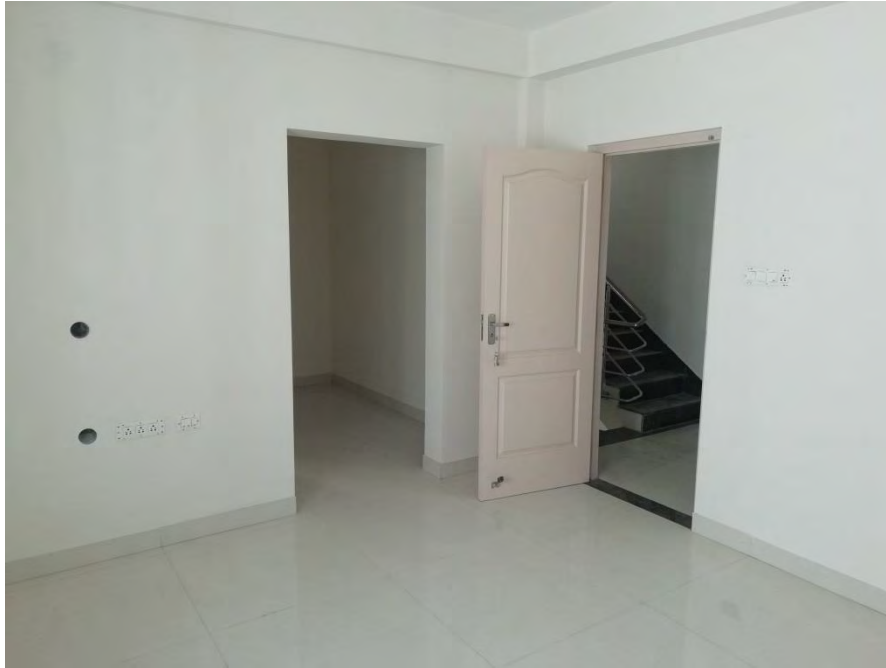
Flooring and painting completed
