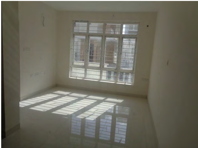
Flooring and painting completed
