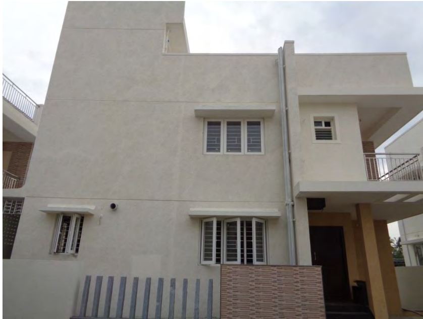
Flooring and painting completed
