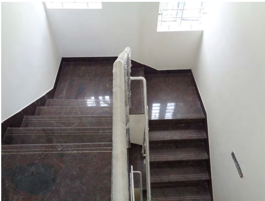
Flooring and painting completed
