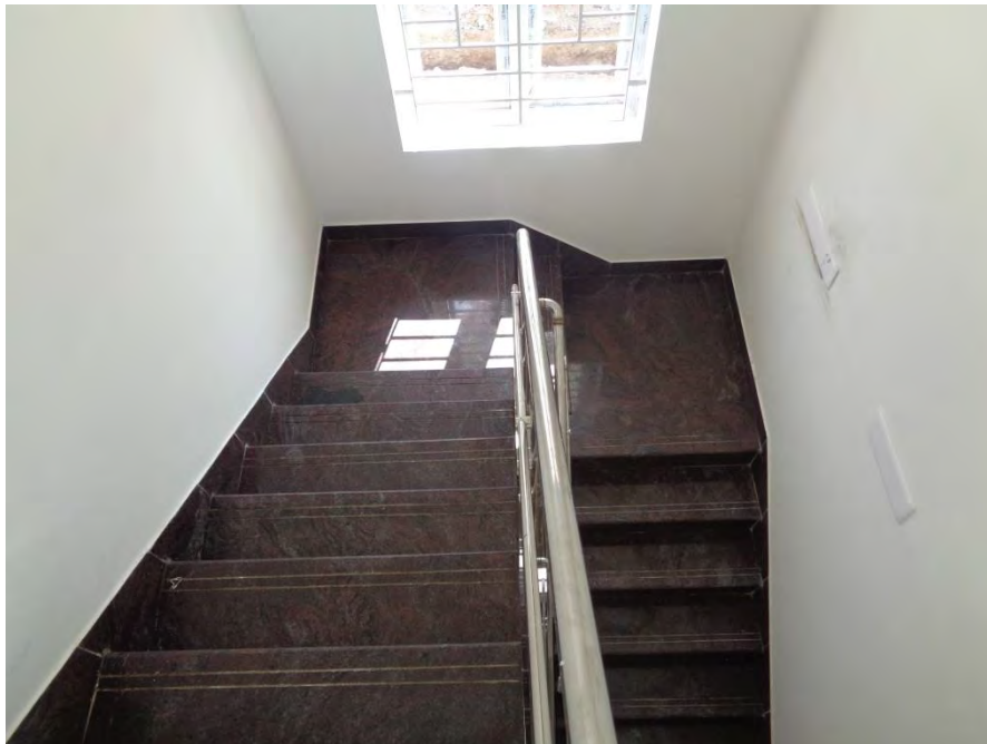
Flooring and painting completed
