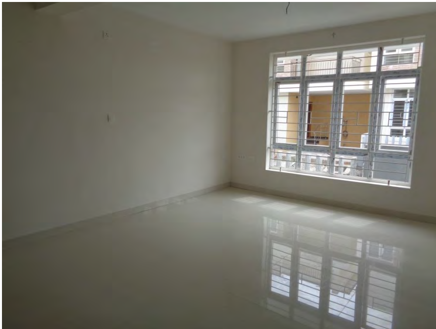
Flooring and painting completed
