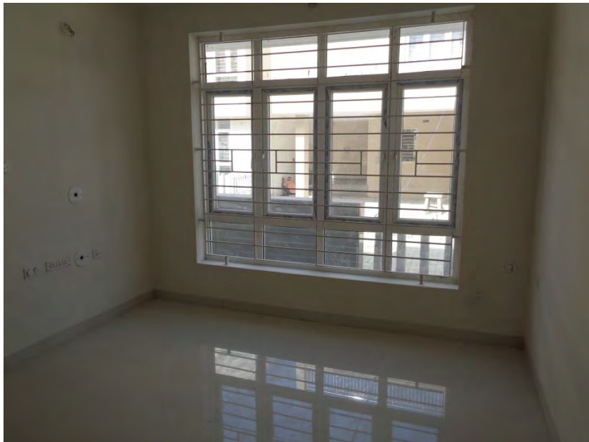
Flooring and painting completed
