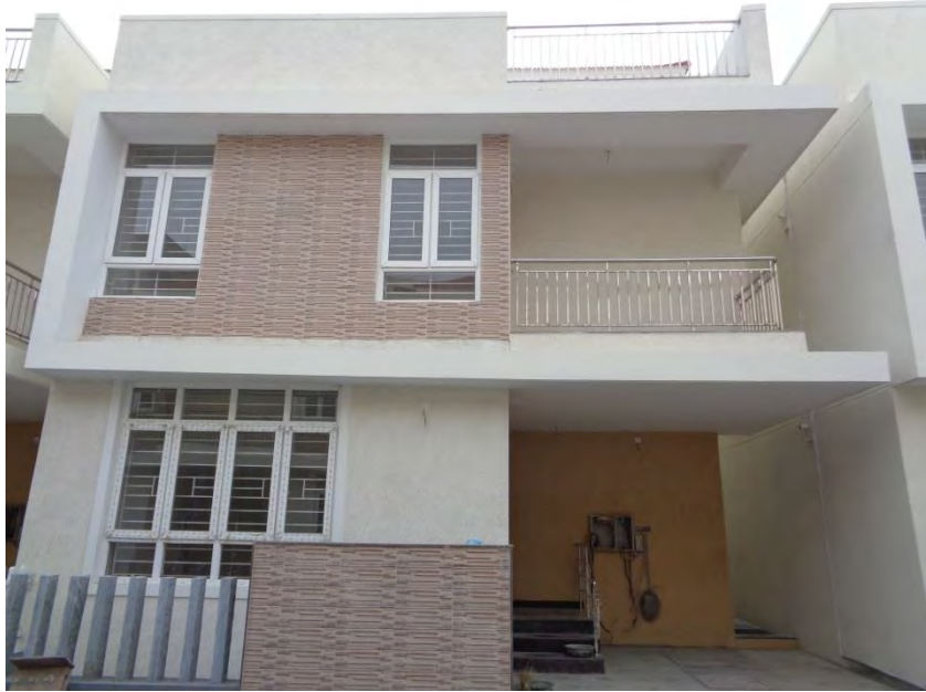
Flooring and painting completed
