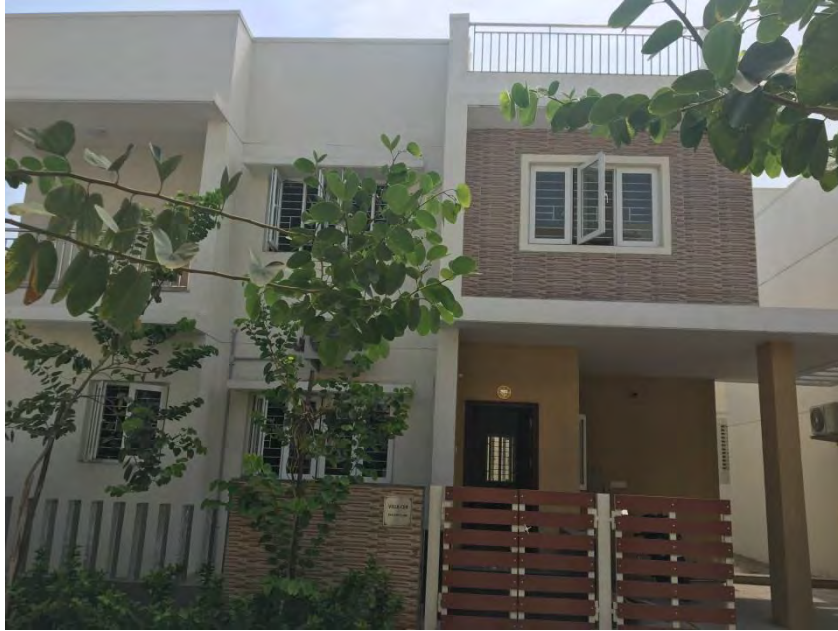
Flooring and painting Completed
