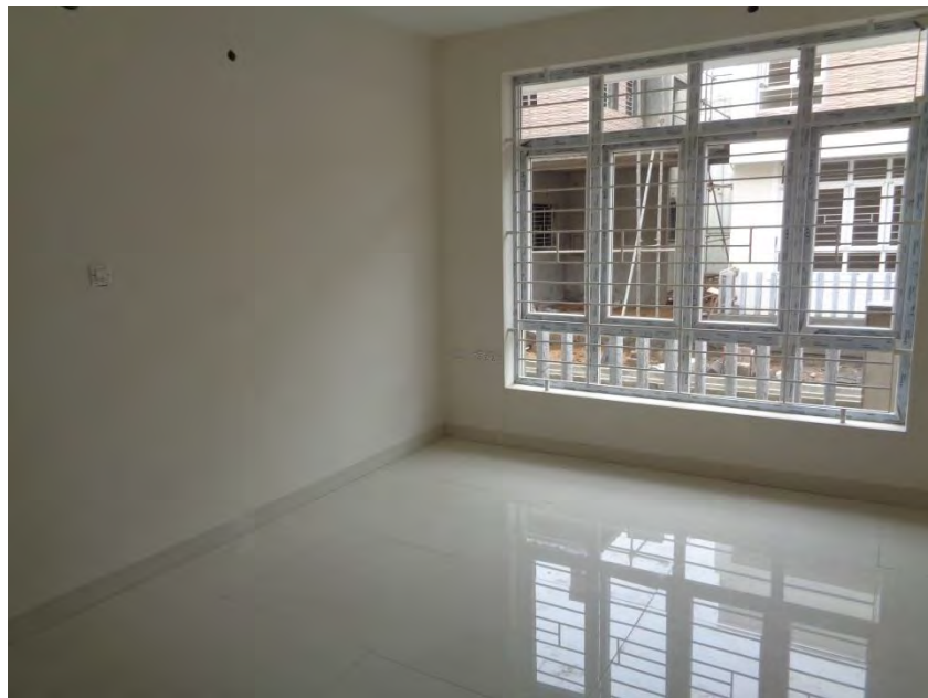
Flooring and painting completed
