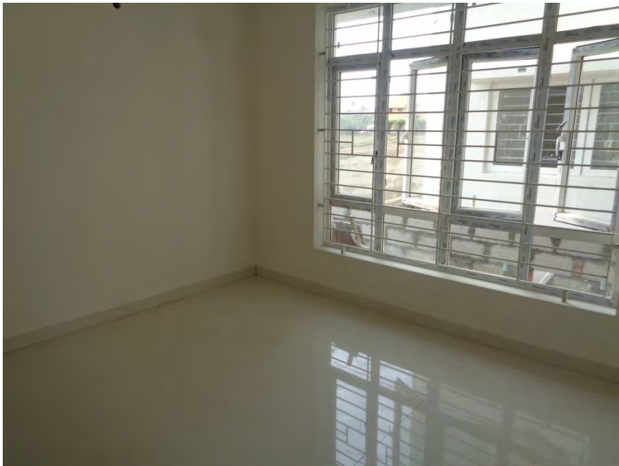
Flooring and painting completed
