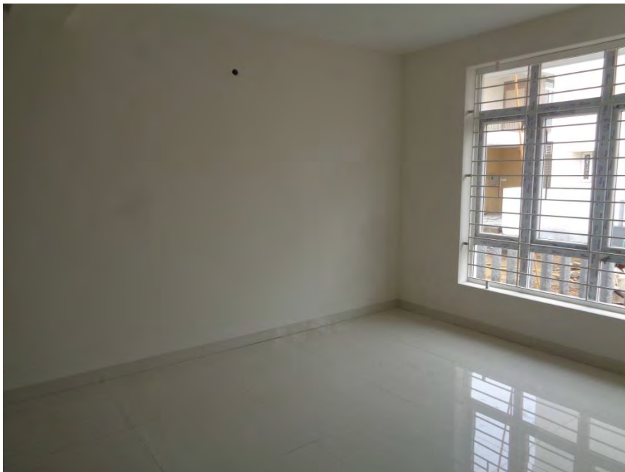
Flooring and painting completed
