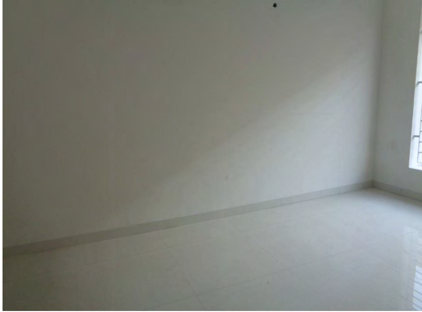
Flooring and painting completed
