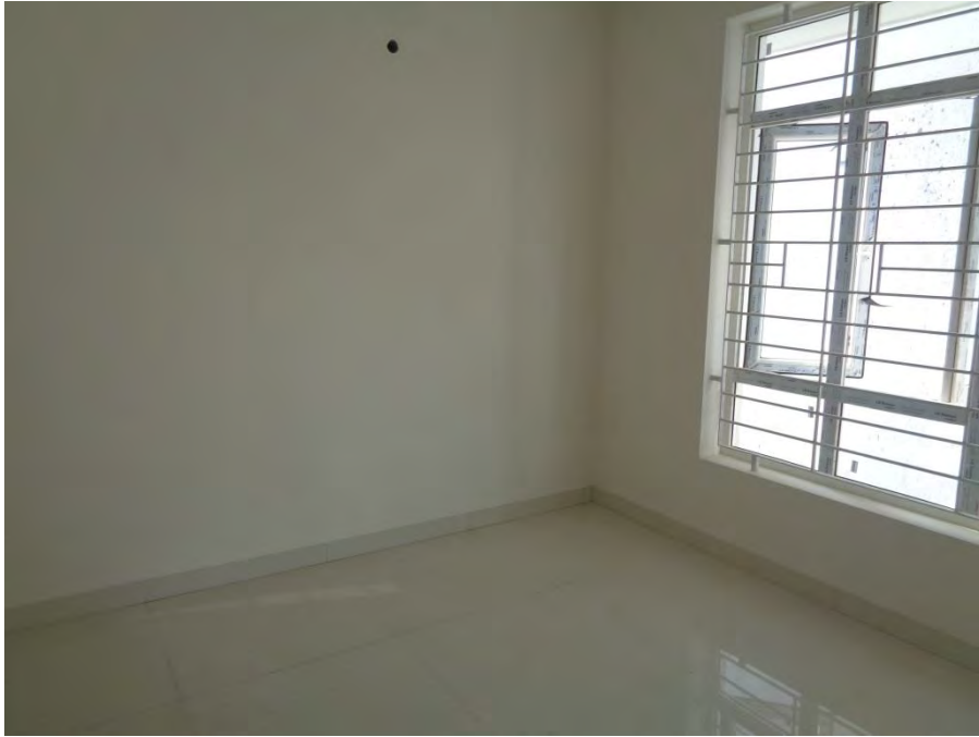
Flooring and painting completed
