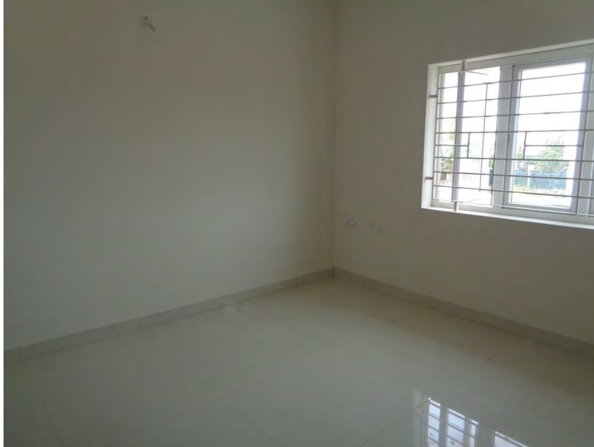
Flooring and painting completed
