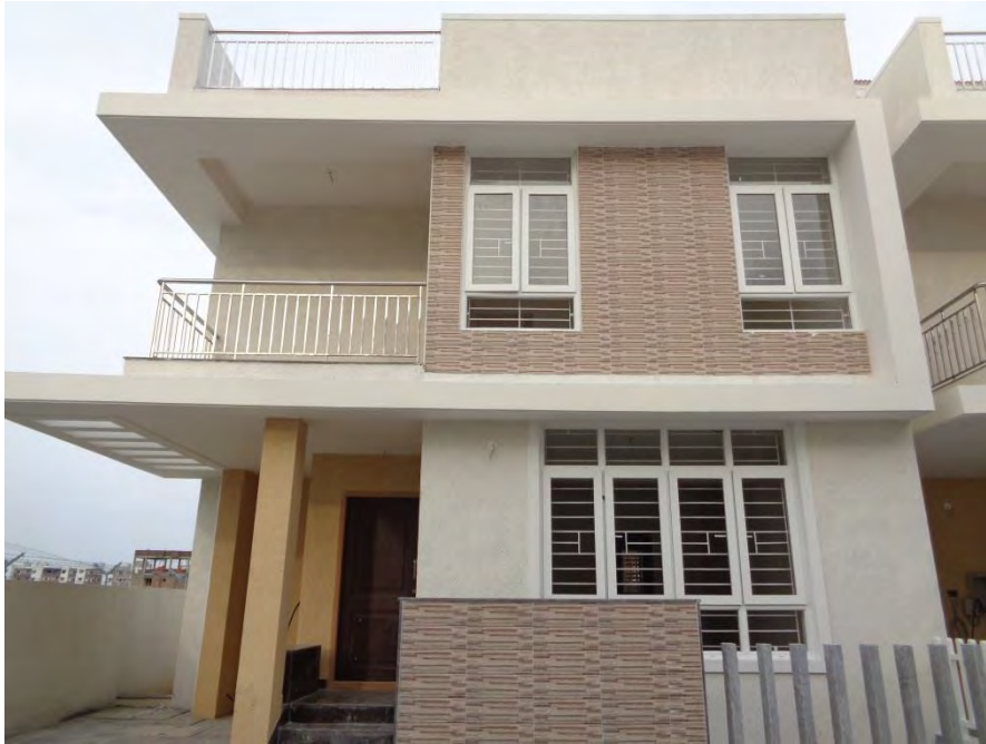
Flooring and painting completed
