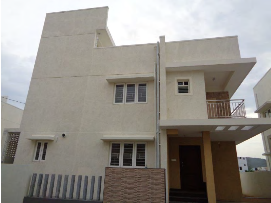
Flooring and painting completed
