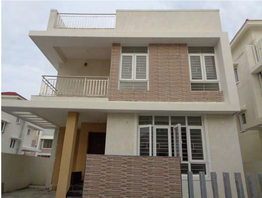
Flooring and painting completed
