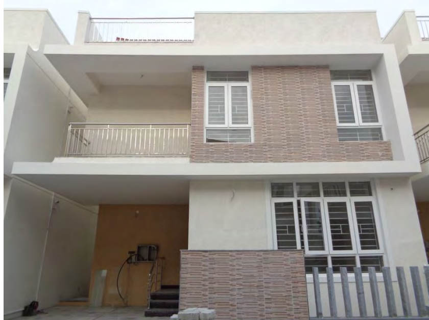
Flooring and painting completed
