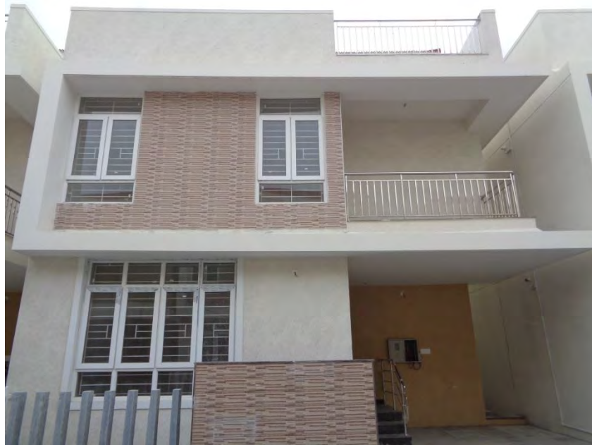
Flooring and painting completed
