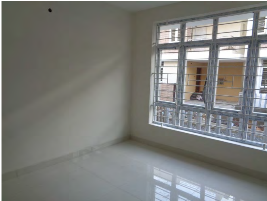
Flooring and painting completed
