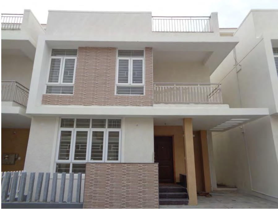
Flooring and painting completed
