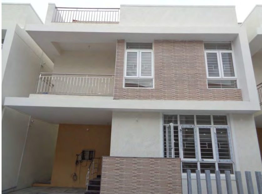
Flooring and painting completed
