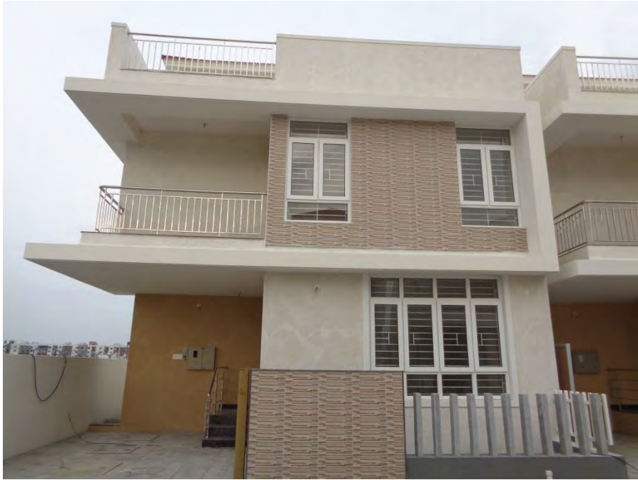
Flooring and painting completed
