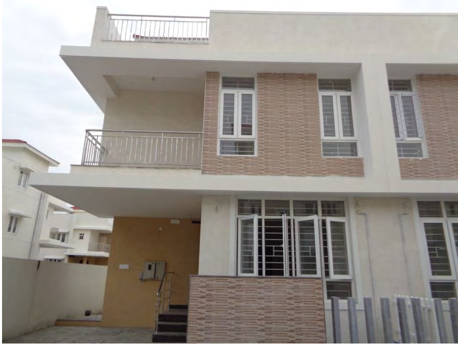
Flooring and painting completed
