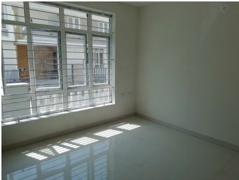
Flooring and painting completed
