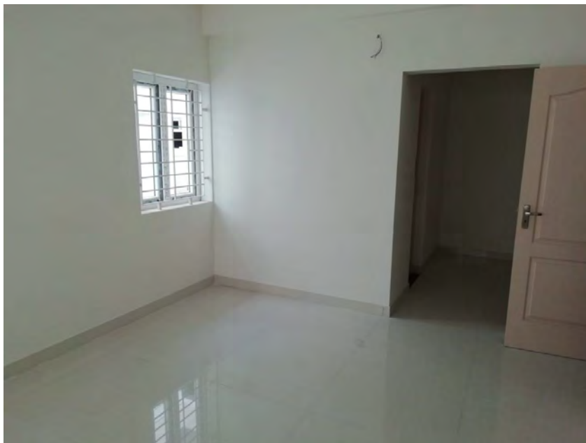
Flooring and painting completed
