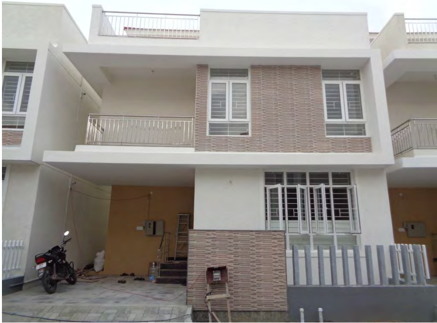
Flooring and painting completed
