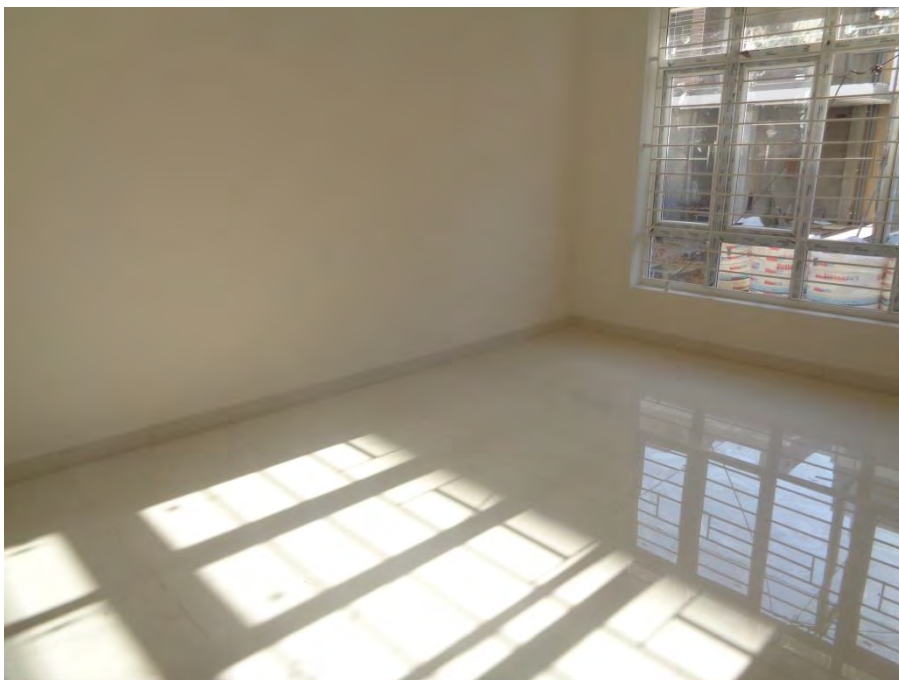
Flooring and painting completed
