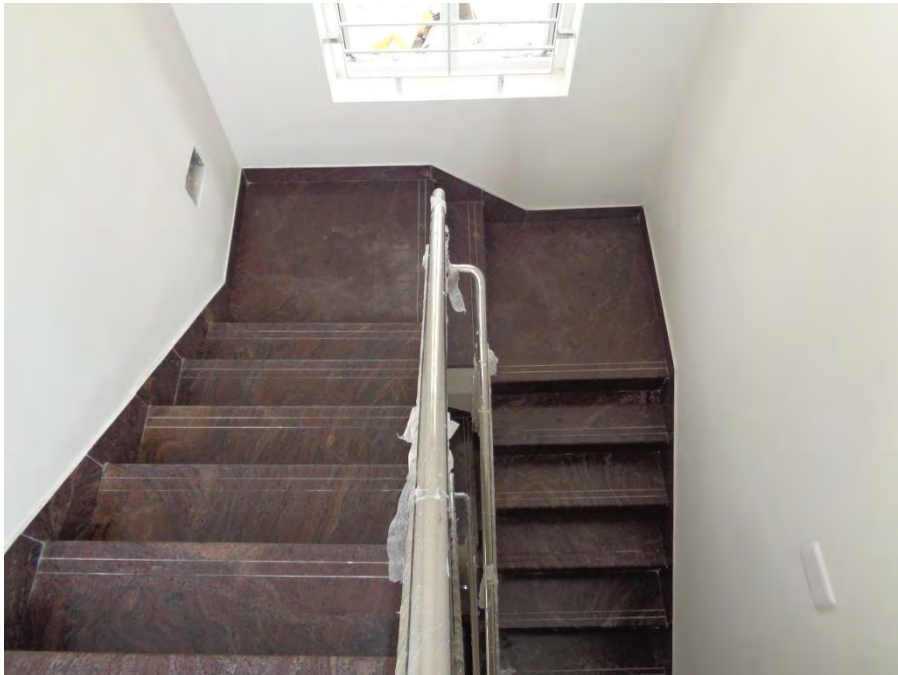
Flooring and painting completed
