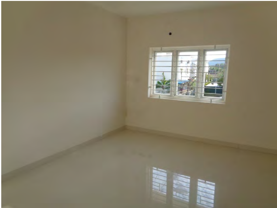
Flooring and painting completed
