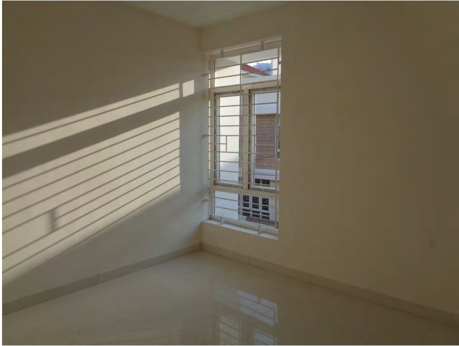
Flooring and painting completed
