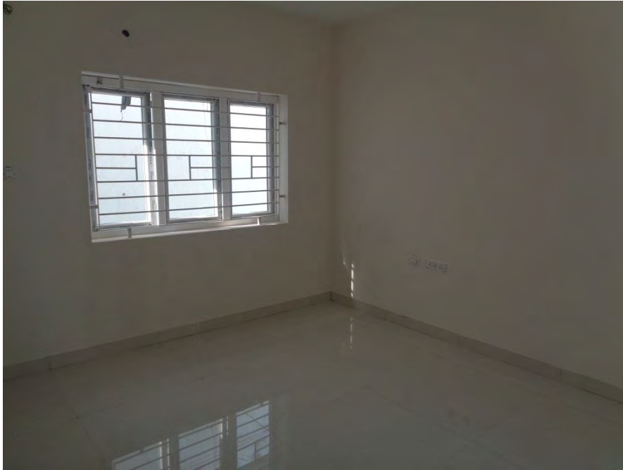
Flooring and painting completed
