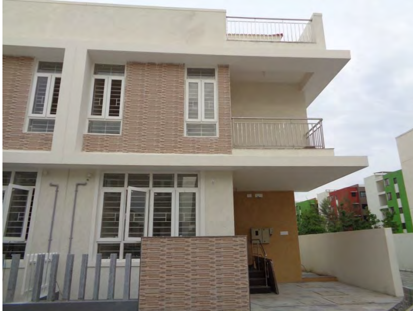
Flooring and painting completed
