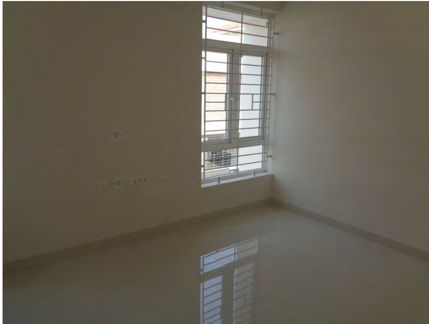
Flooring and painting completed
