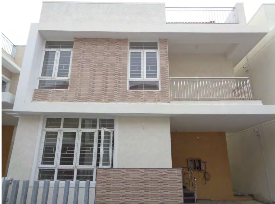
Flooring and painting completed
