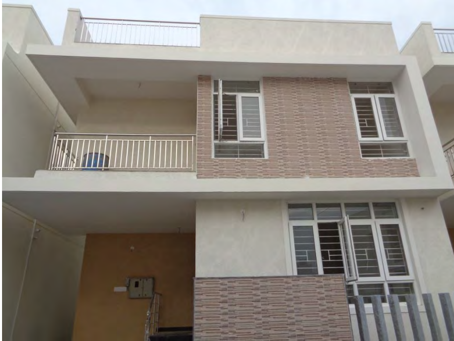
Flooring and painting completed
