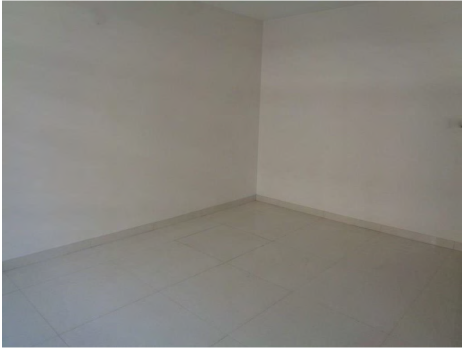
Flooring and painting completed
