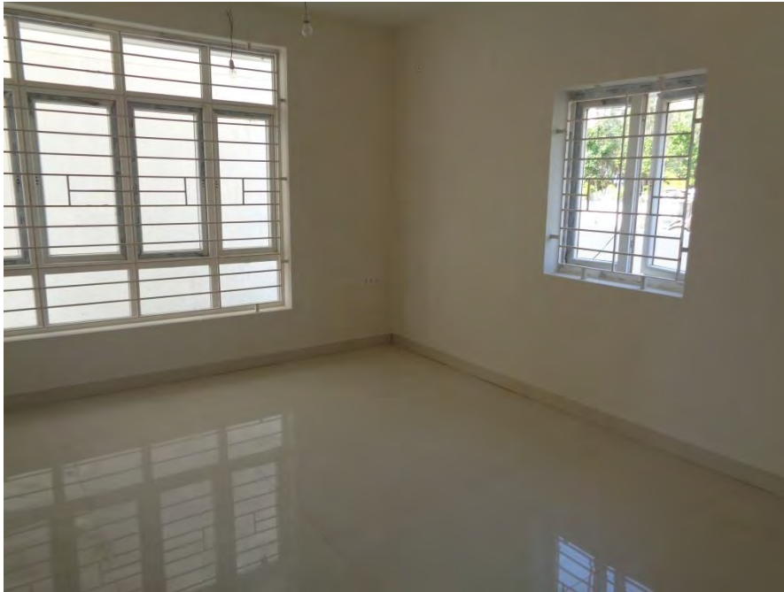
Flooring and painting completed
