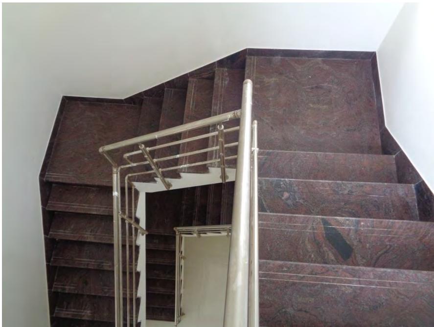
Flooring and painting completed
