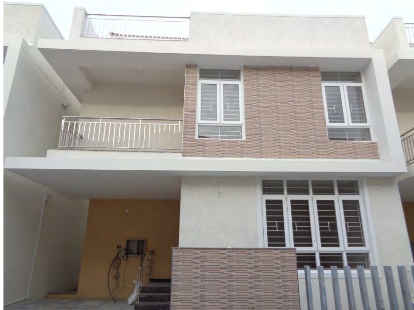
Flooring and painting completed
