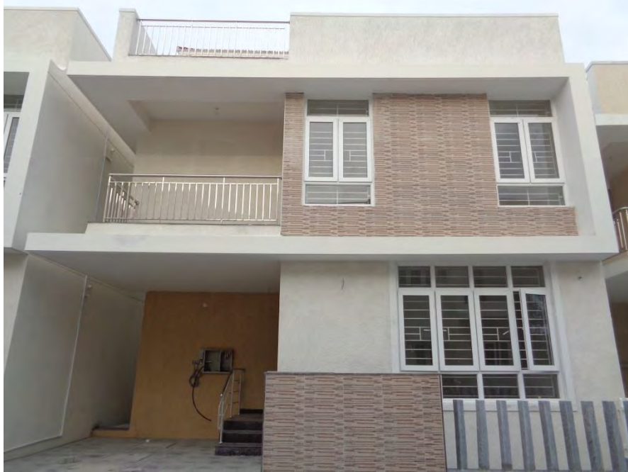
Flooring and painting completed
