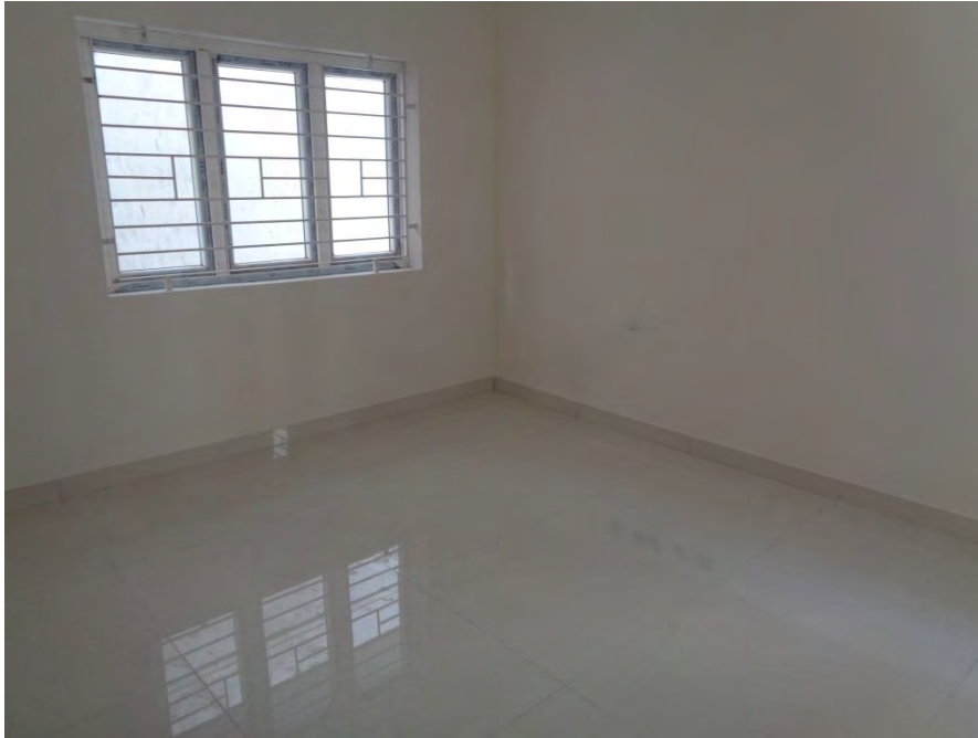
Flooring and painting completed
