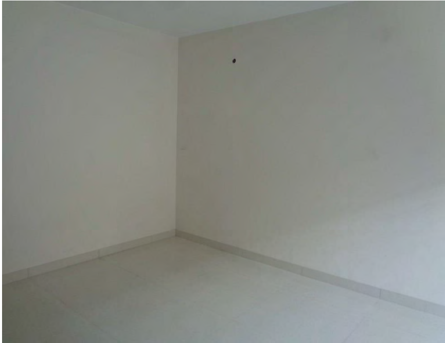
Flooring and painting completed
