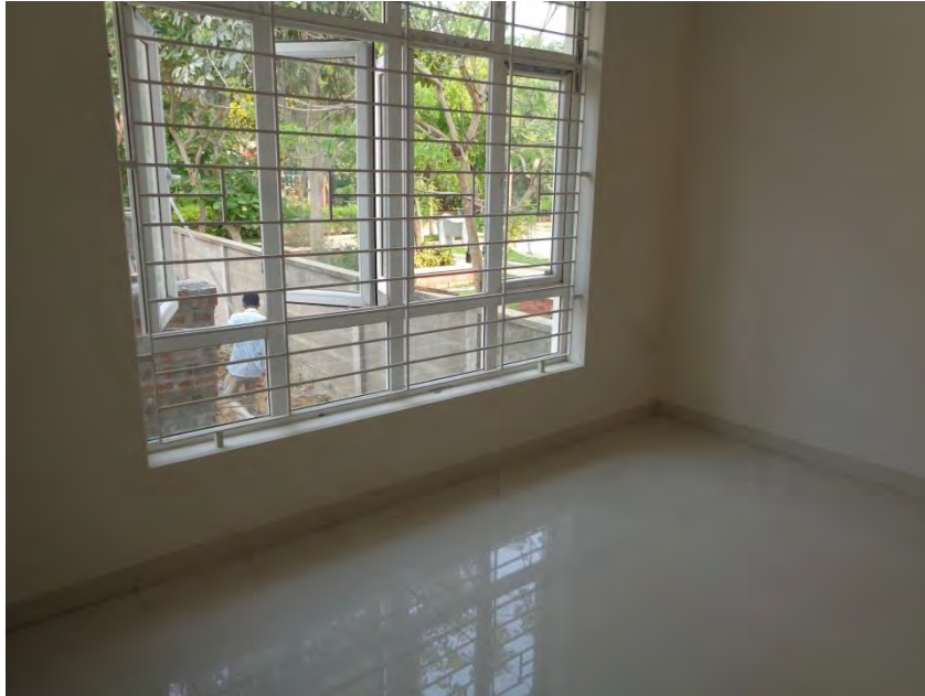
Flooring and painting completed
