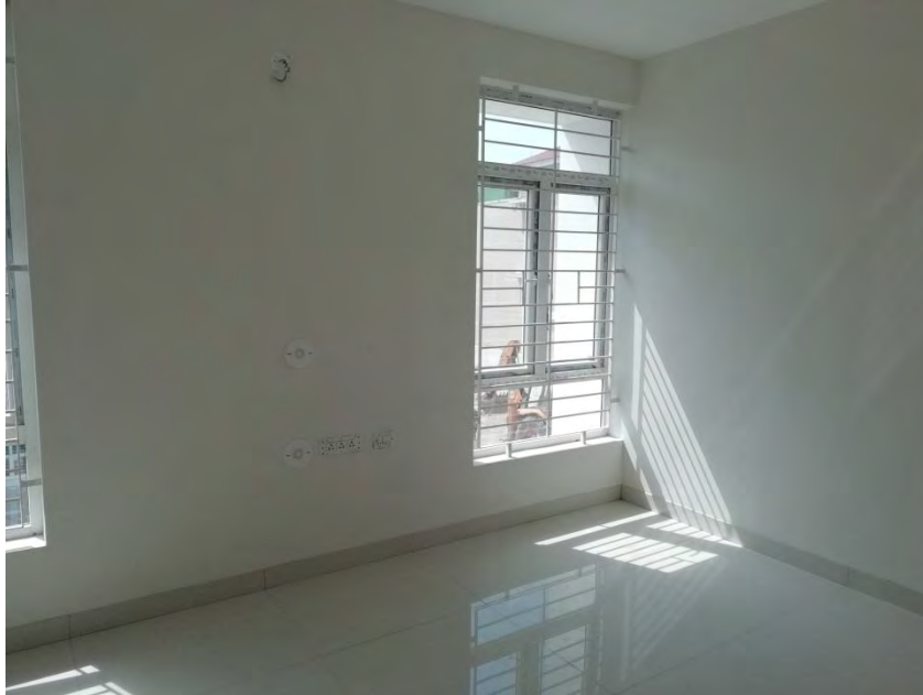
Flooring and painting completed
