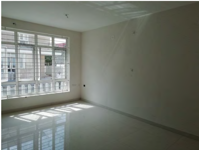
Flooring and painting completed
