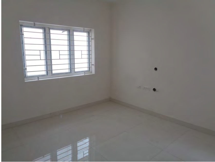
Flooring and painting completed
