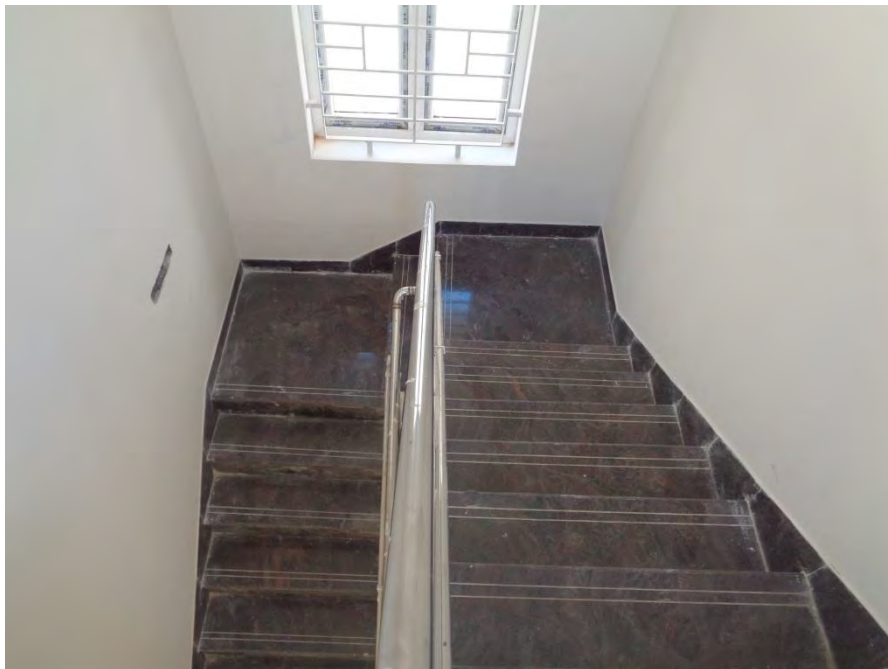
Flooring and painting completed
