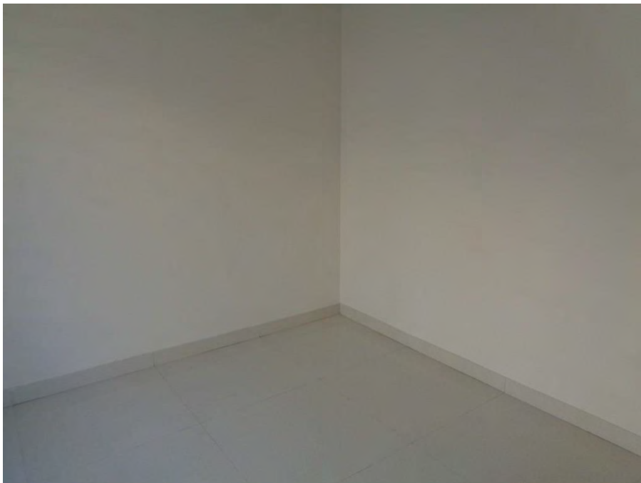
Flooring and painting completed
