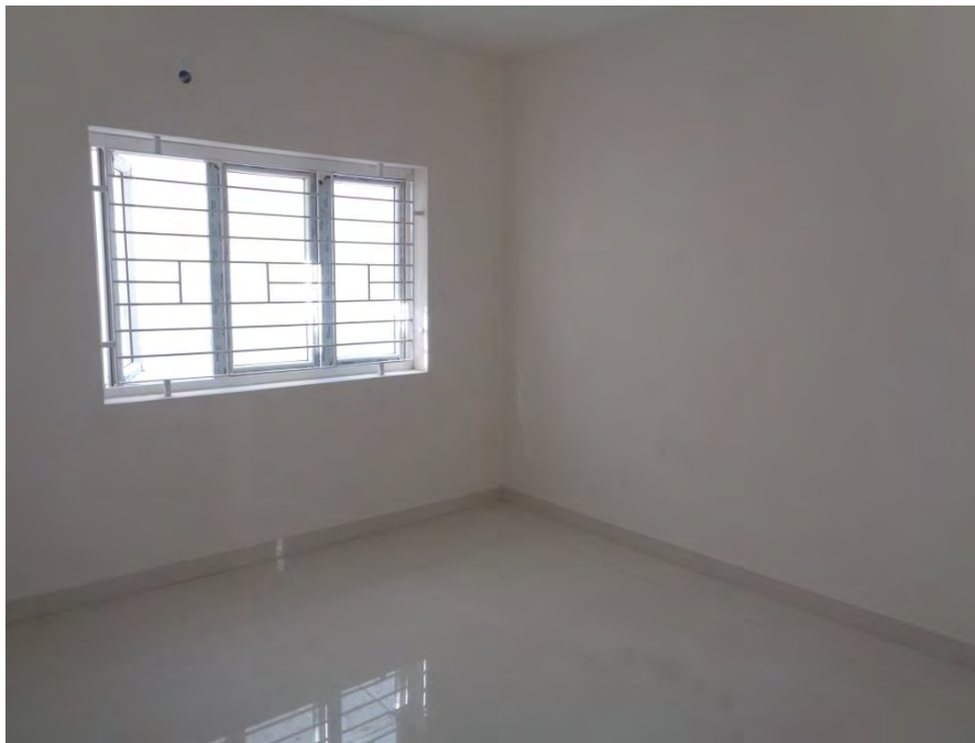
Flooring and painting completed
