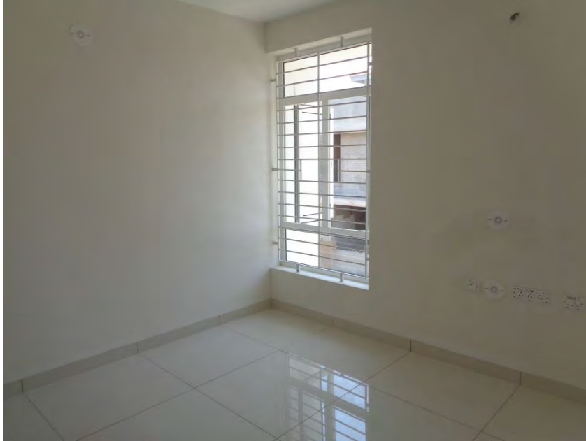
Flooring and painting completed
