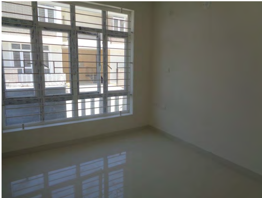
Flooring and painting completed
