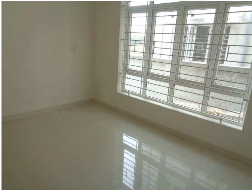
Flooring and painting completed
