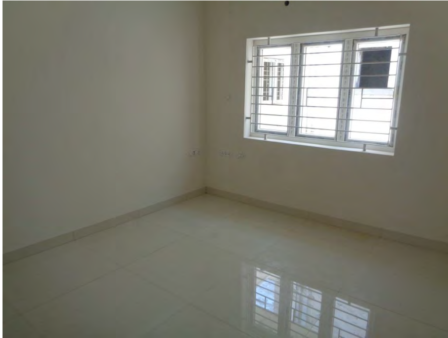
Flooring and painting completed
