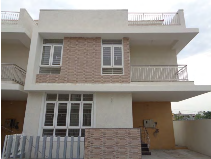
Flooring and painting completed
