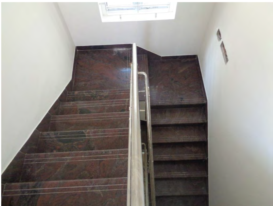
Flooring and painting completed
