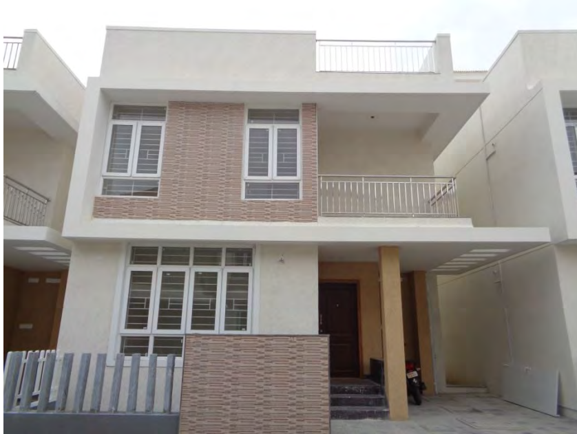
Flooring and painting completed
