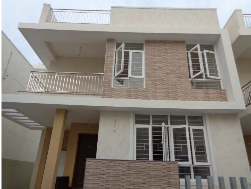
Flooring and painting completed
