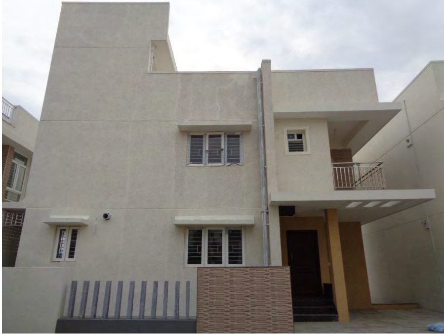
Flooring and painting completed
