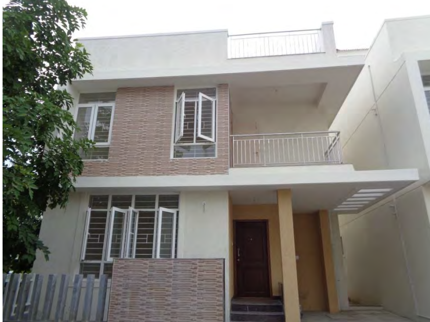
Flooring and painting completed
