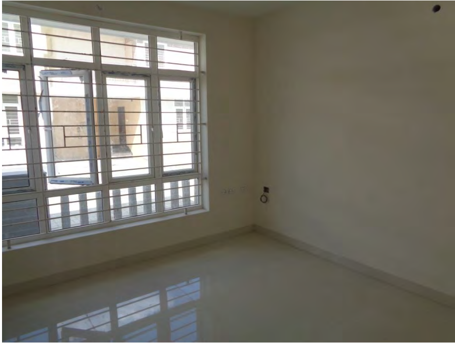
Flooring and painting completed
