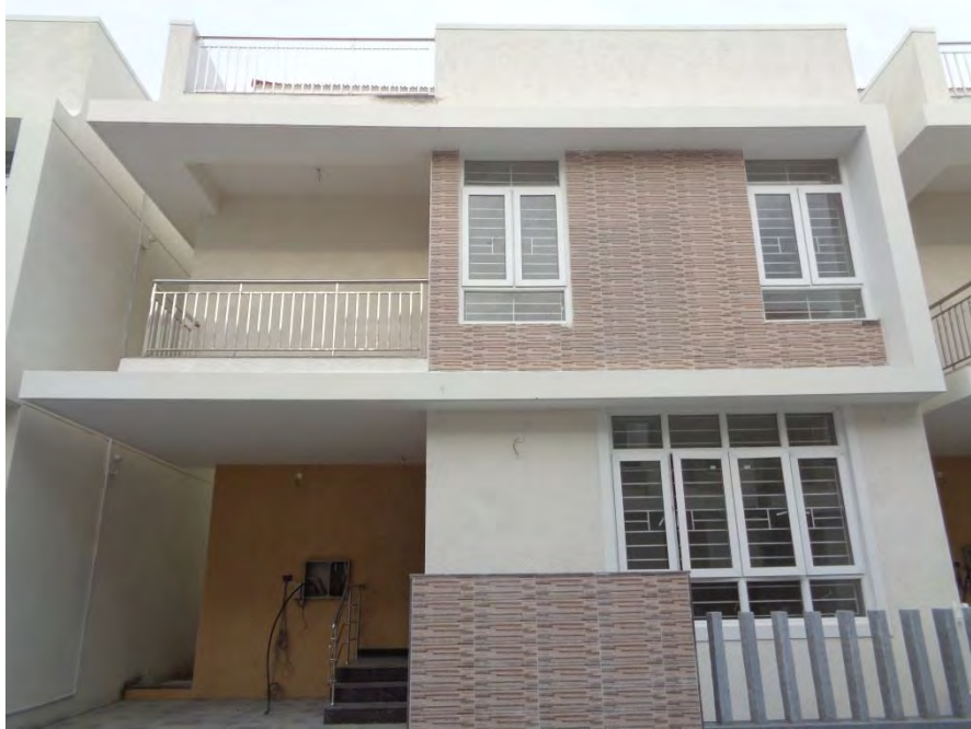
Flooring and painting completed
