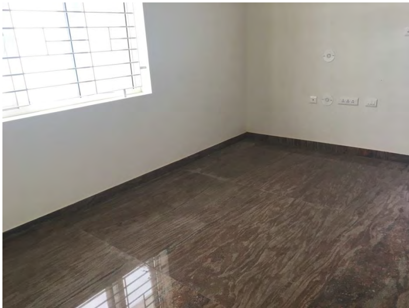
Flooring and painting Completed
