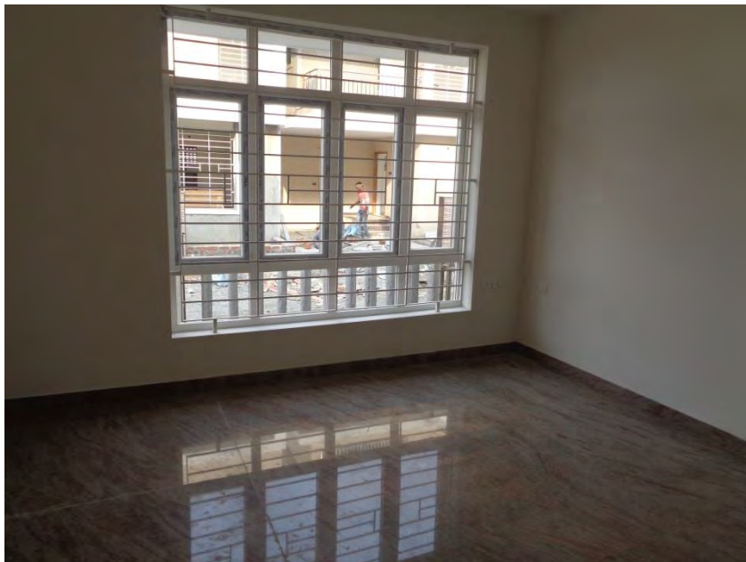
Flooring and painting completed
