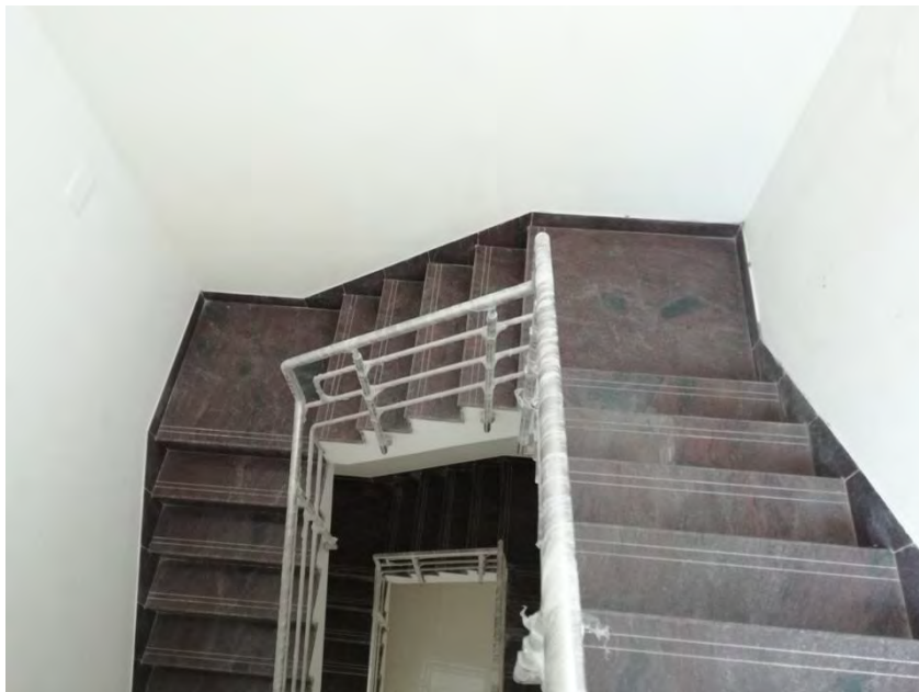
Flooring and painting completed
