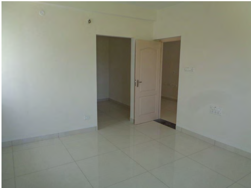
Flooring and painting completed
