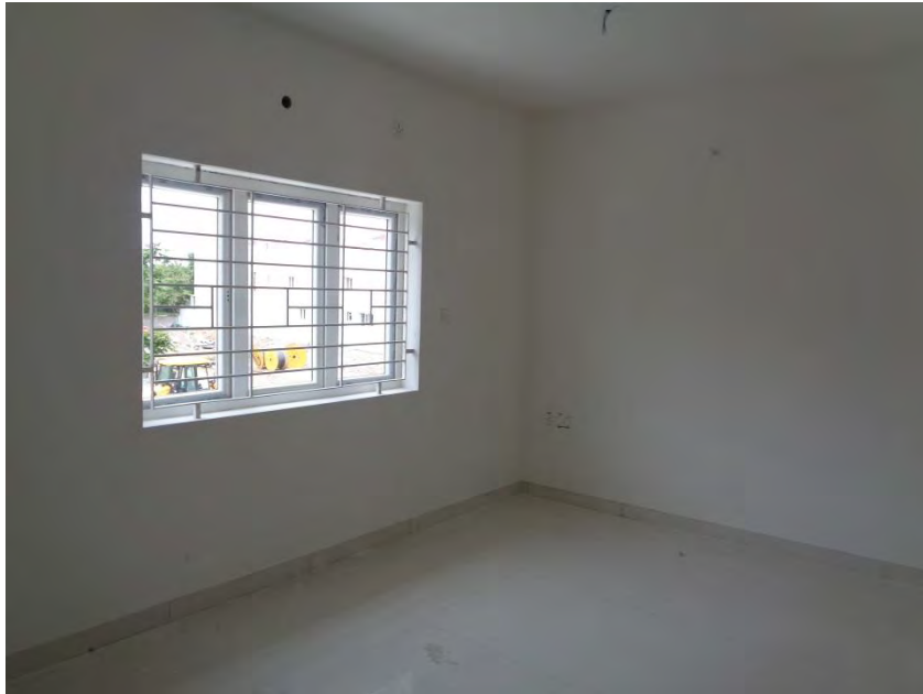
Flooring and painting Completed
