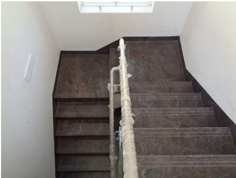
Flooring and painting completed
