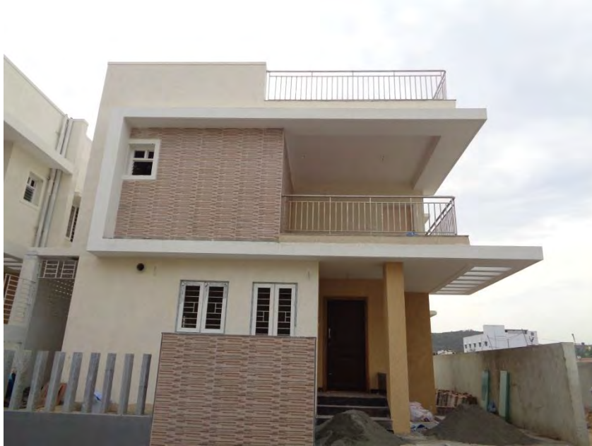
Flooring and painting completed
