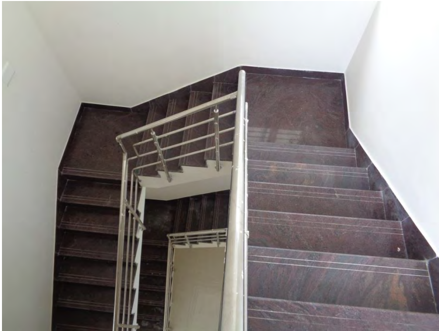
Flooring and painting completed
