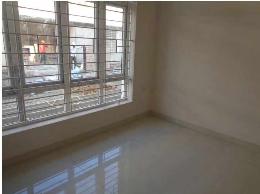
Flooring and painting completed
