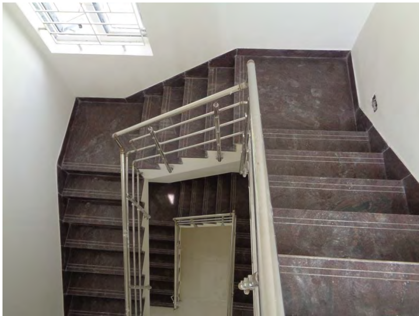
Flooring and painting completed
