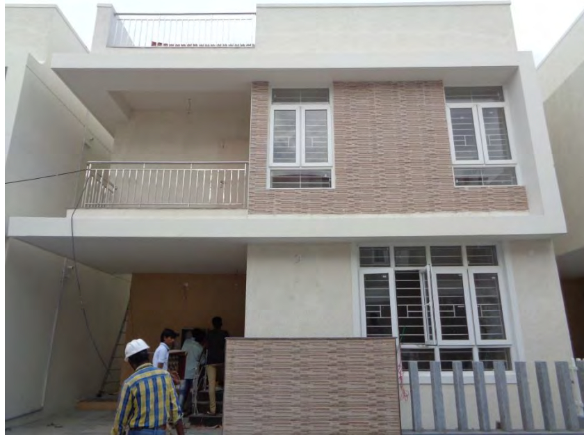
Flooring and painting completed
