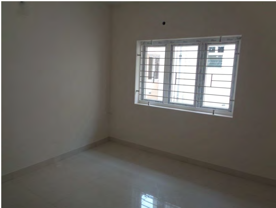
Flooring and painting completed
