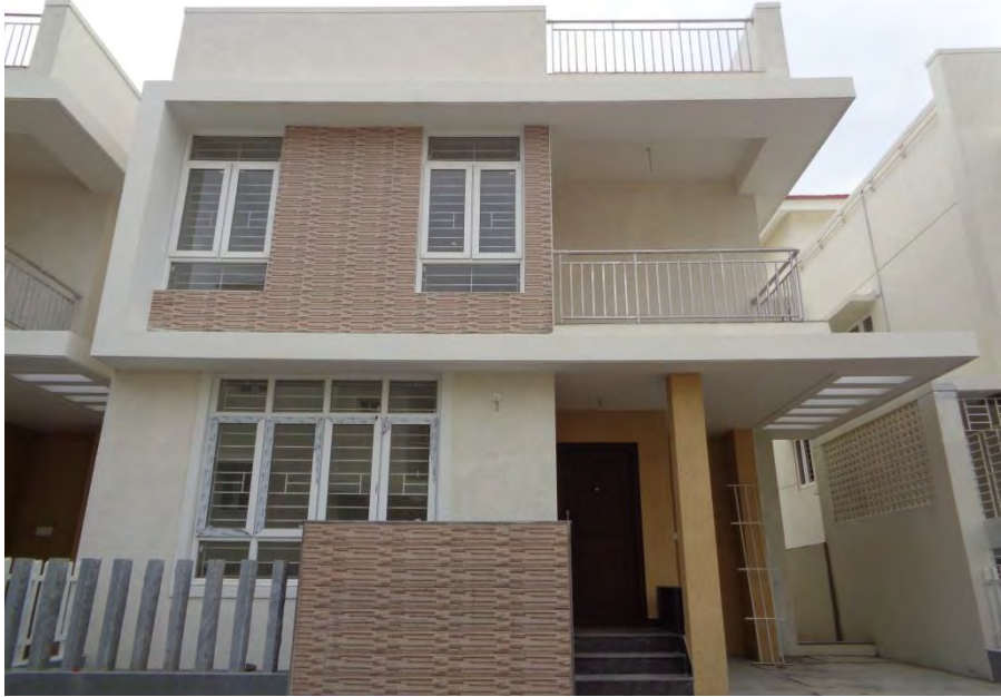
Flooring and painting completed
