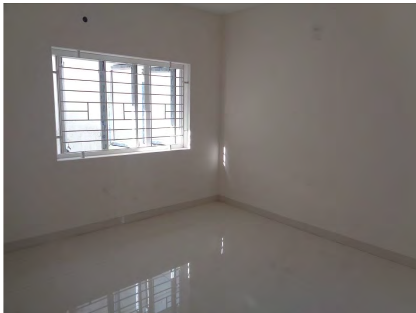
Flooring and painting completed
