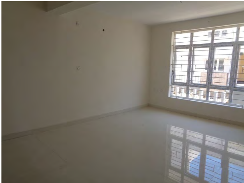
Flooring and painting completed
