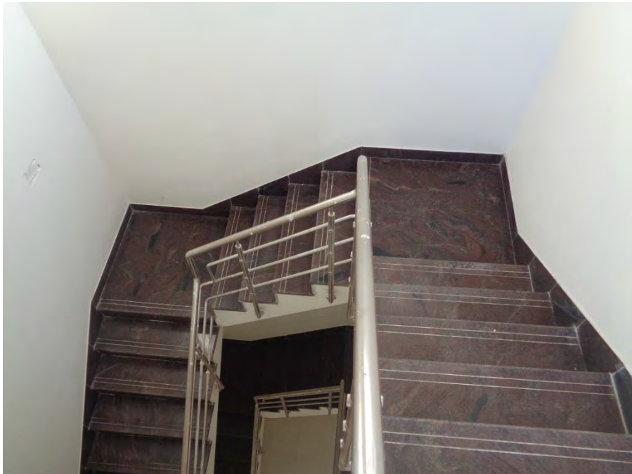
Flooring and painting completed
