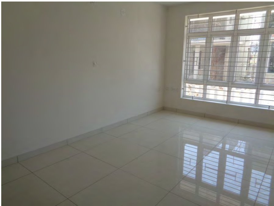
Flooring and painting completed
