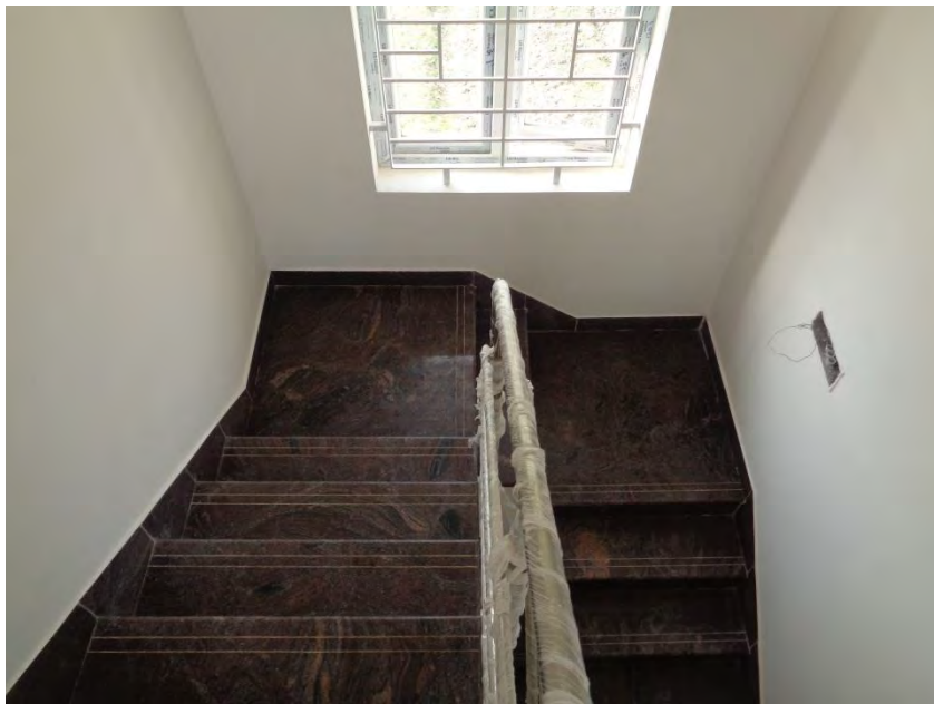
Flooring and painting completed
