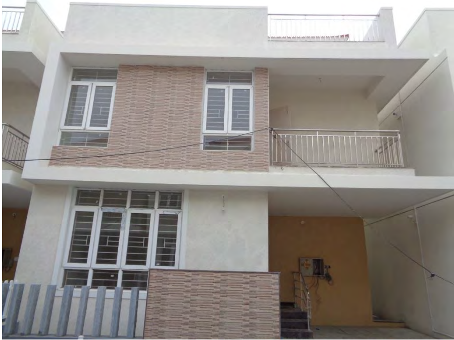
Flooring and painting completed
