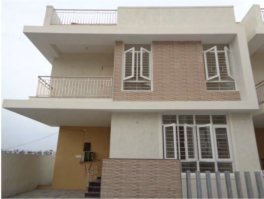
Flooring and painting completed
