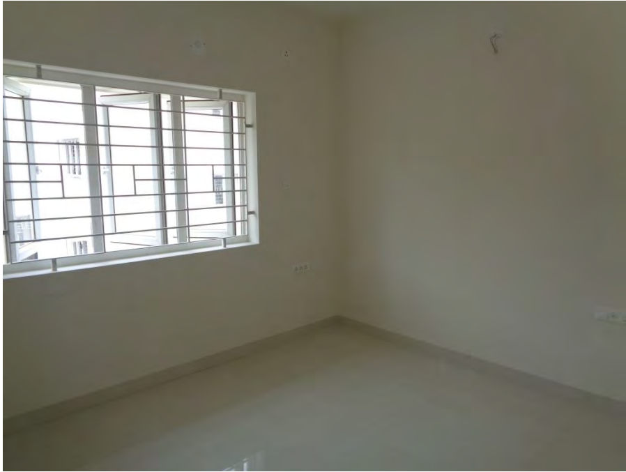
Flooring and painting completed
