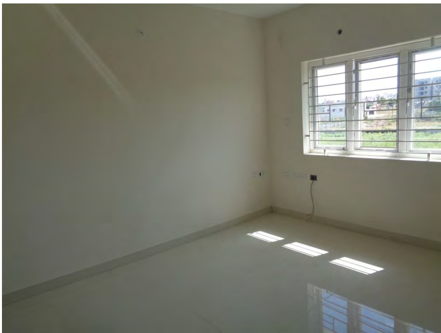
Flooring and painting completed
