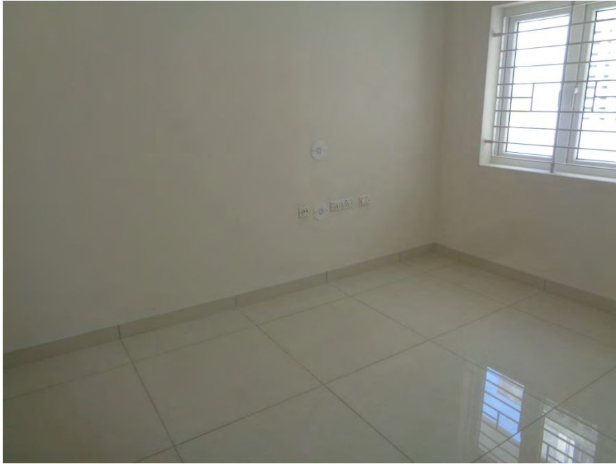
Flooring and painting completed
