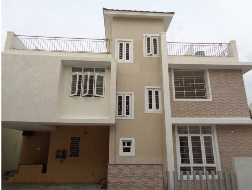
Flooring and painting completed
