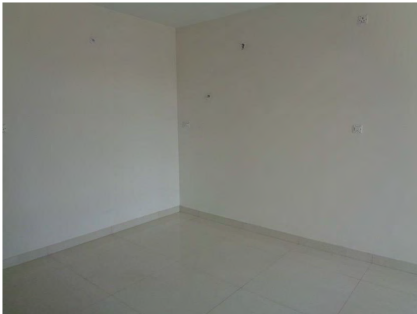
Flooring and painting completed
