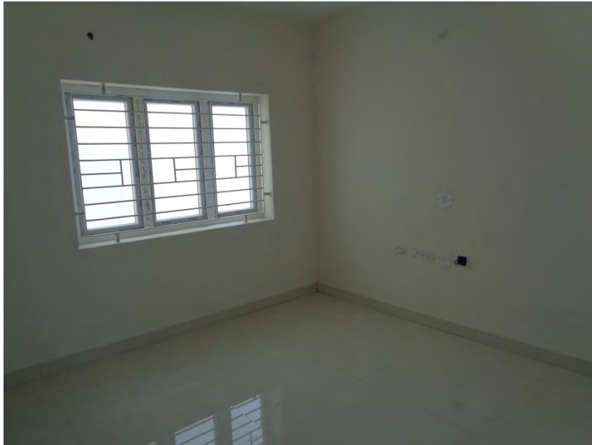
Flooring and painting completed
