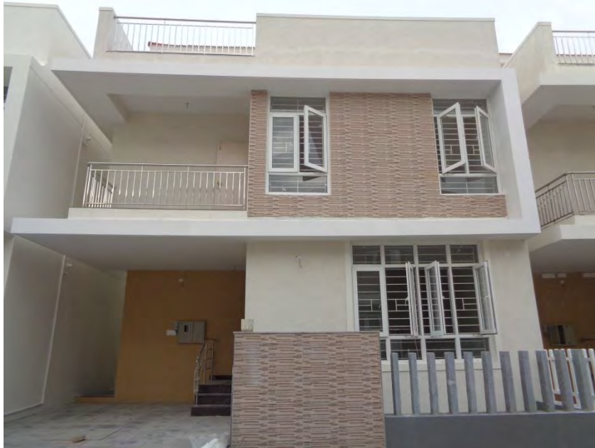
Flooring and painting completed
