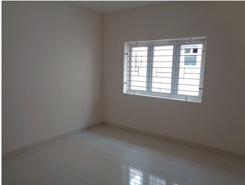
Flooring and painting completed
