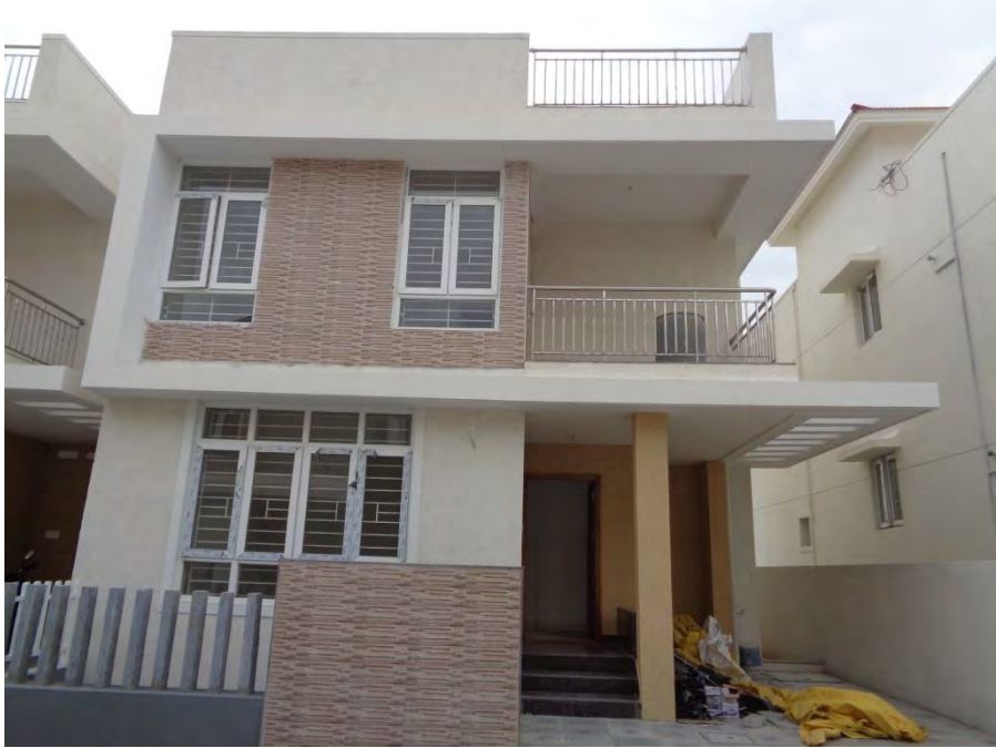
Flooring and painting completed
