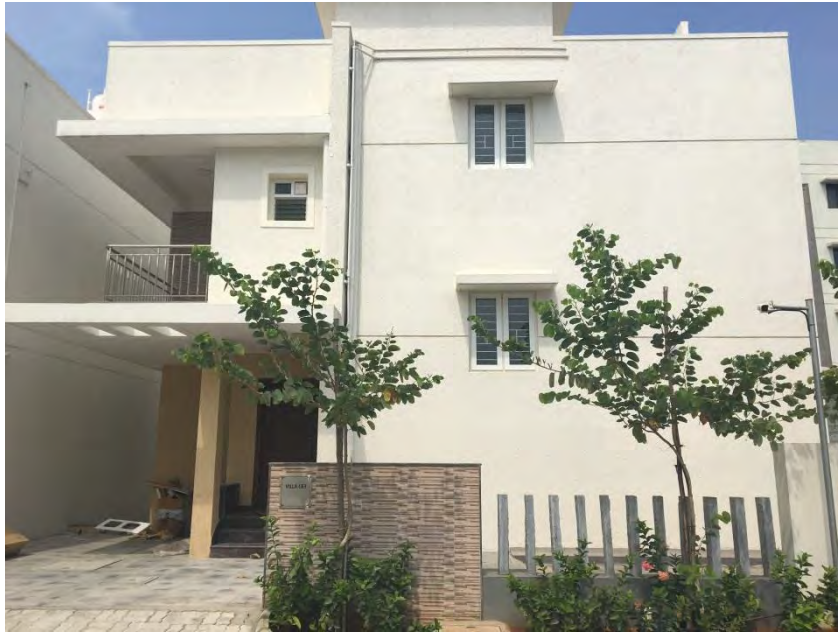
Flooring and painting Completed
