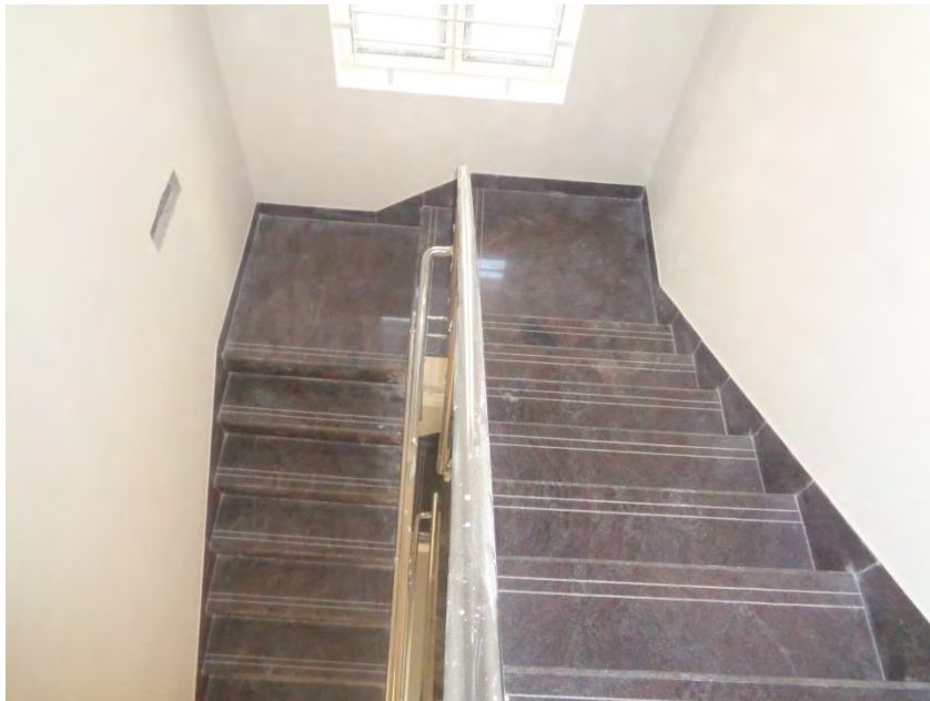
Flooring and painting completed
