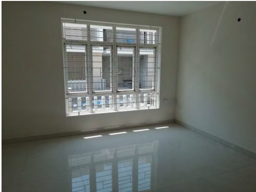
Flooring and painting completed
