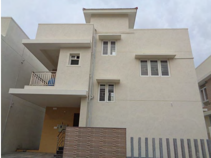
Flooring and painting completed
