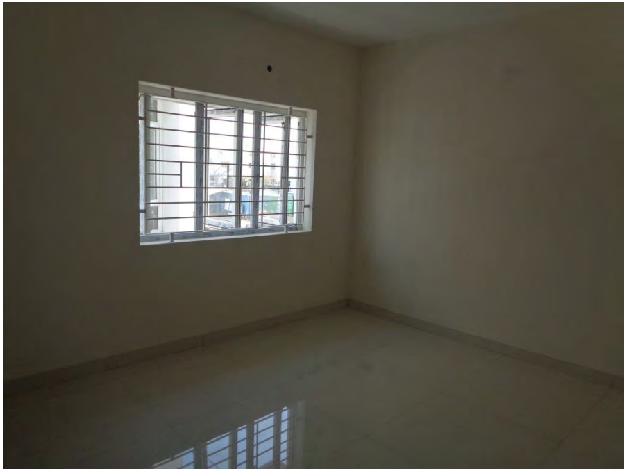
Flooring and painting completed
