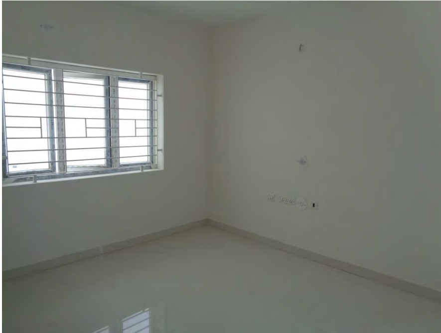
Flooring and painting completed
