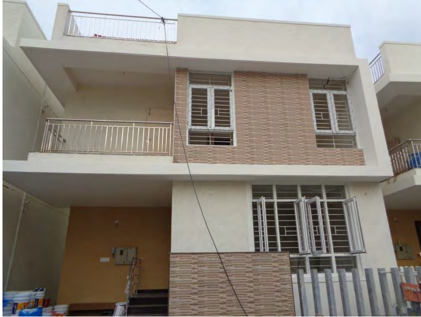
Flooring and painting completed
