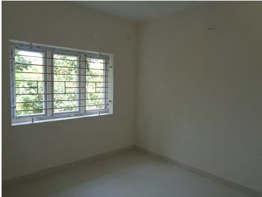
Flooring and painting Completed
