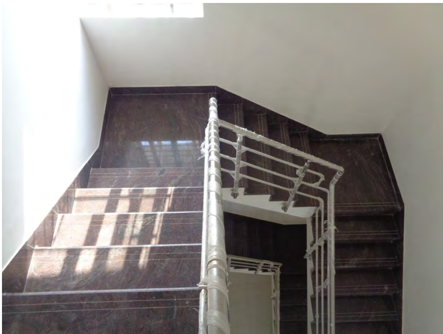
Flooring and painting completed
