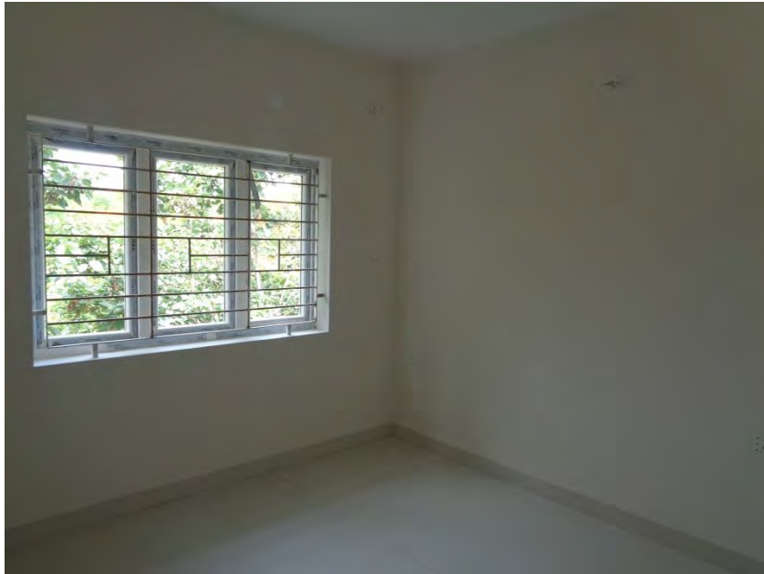
Flooring and painting completed
