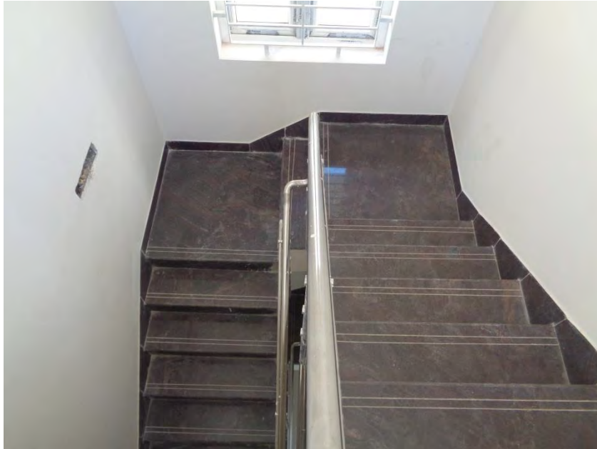
Flooring and painting completed
