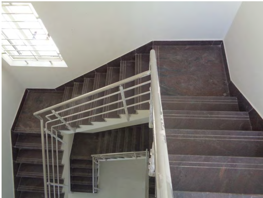
Flooring and painting completed
