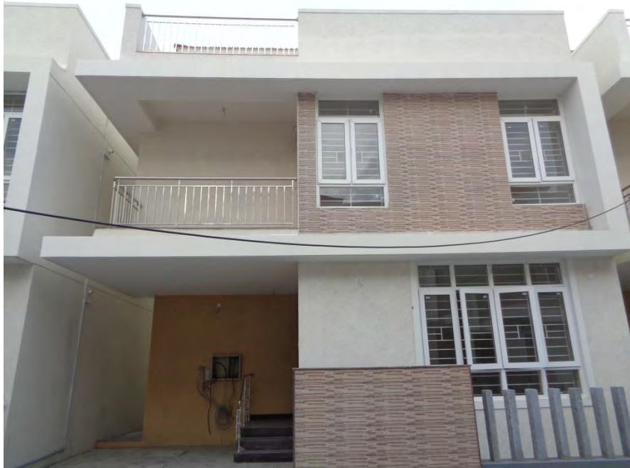
Flooring and painting completed
