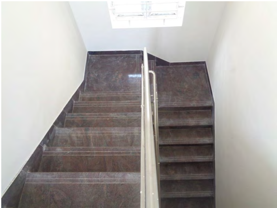
Flooring and painting completed
