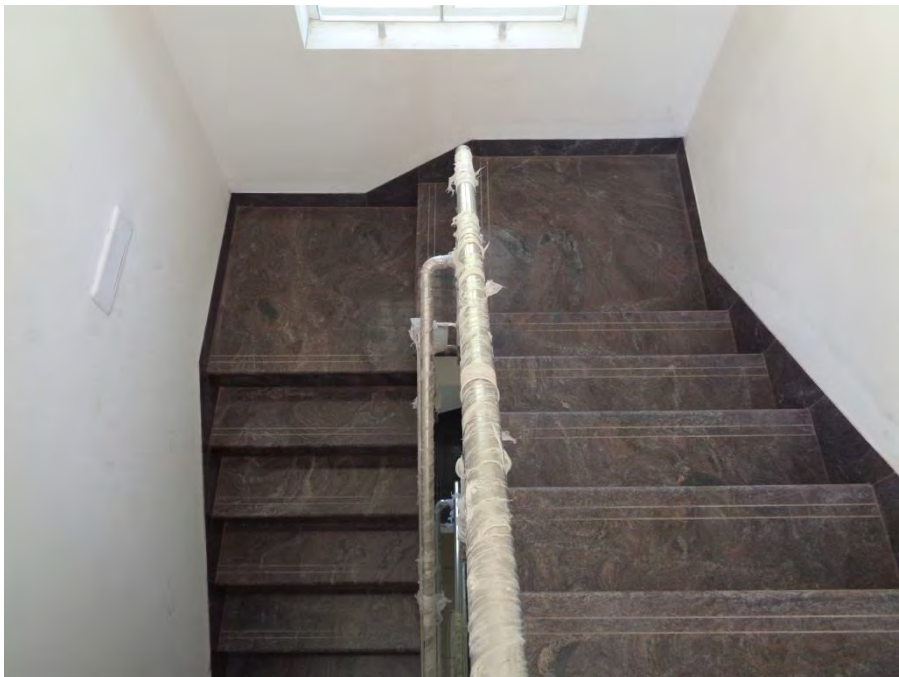
Flooring and painting completed
