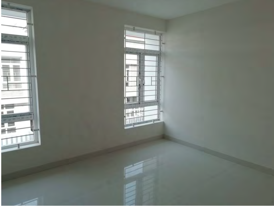
Flooring and painting completed
