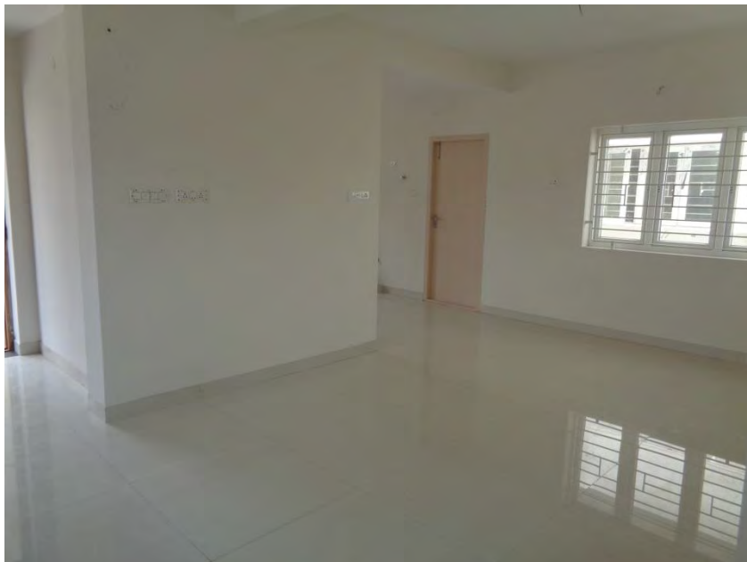
Flooring and painting completed
