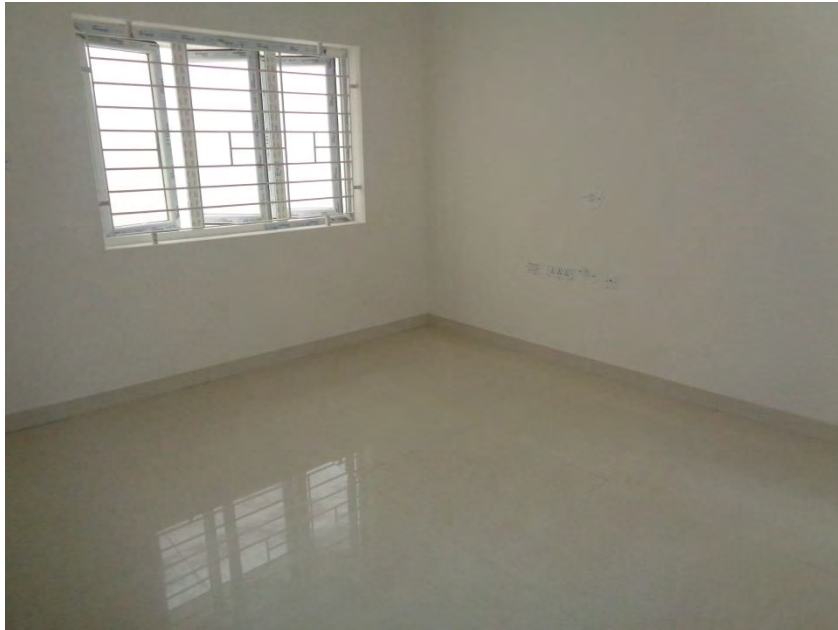
Flooring and painting completed
