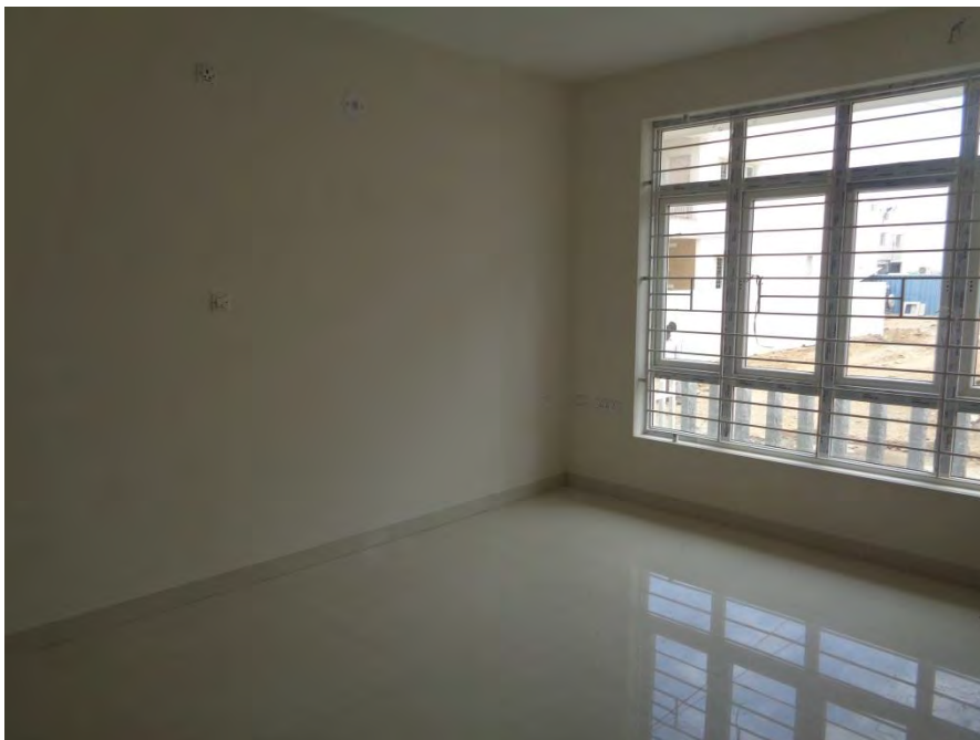
Flooring and painting completed
