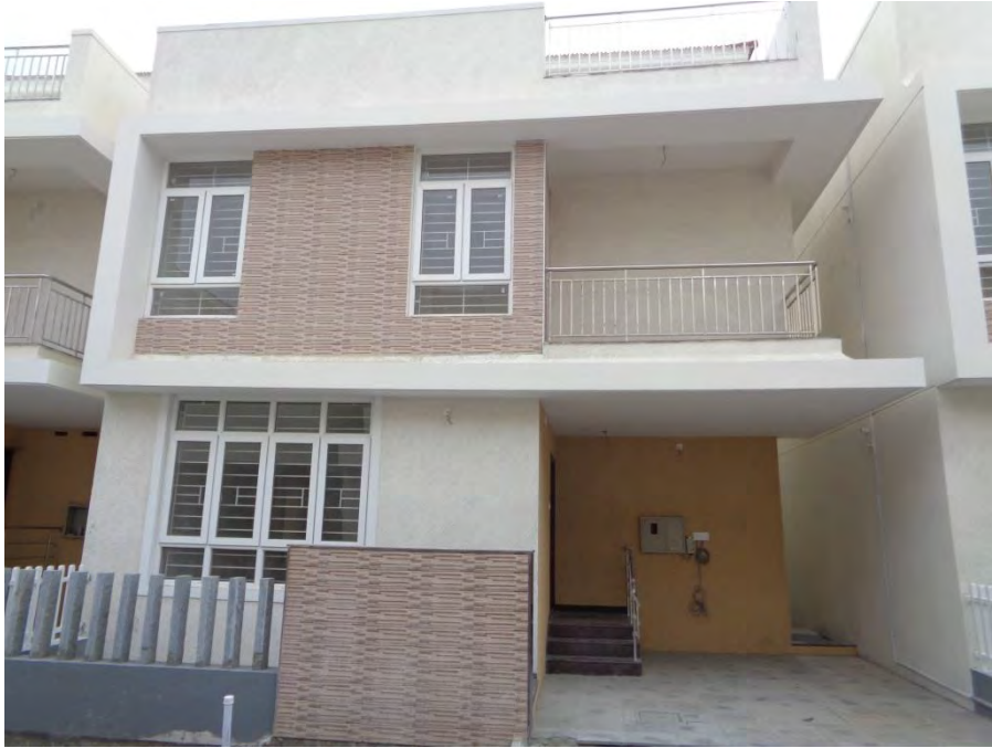
Flooring and painting completed
