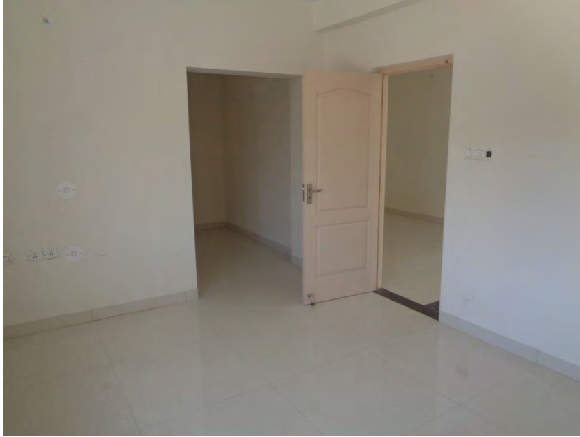
Flooring and painting completed
