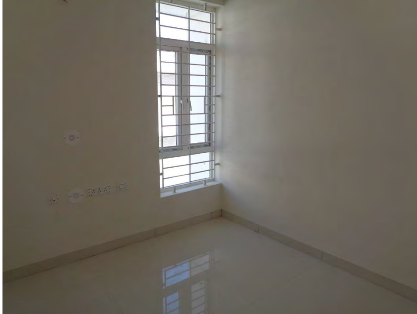
Flooring and painting completed
