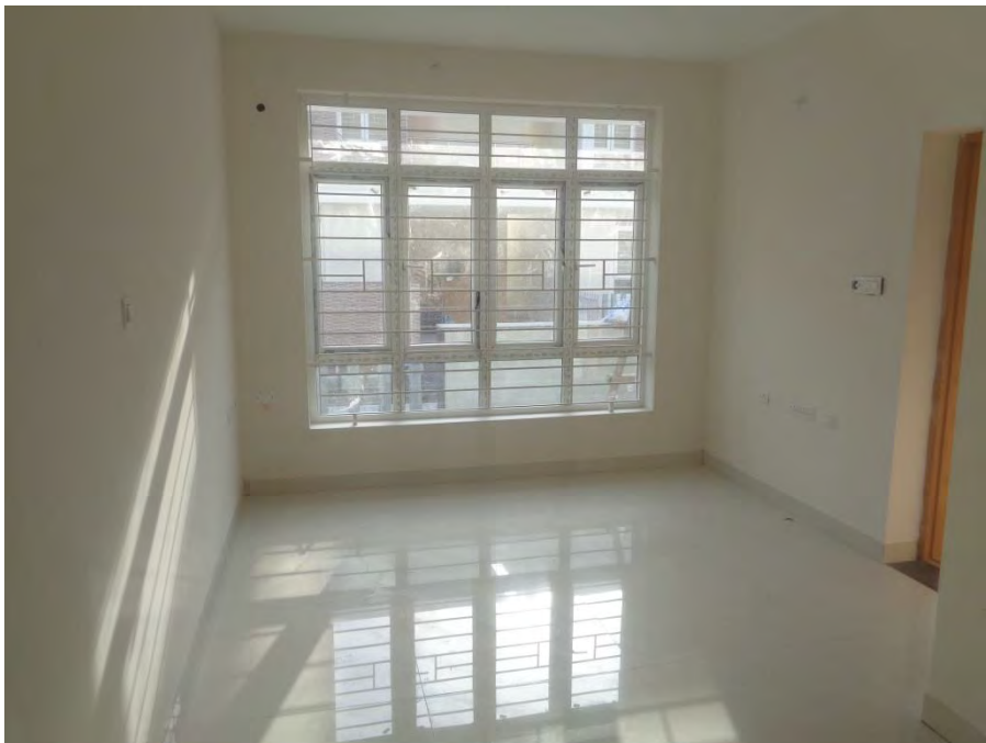
Flooring and painting completed
