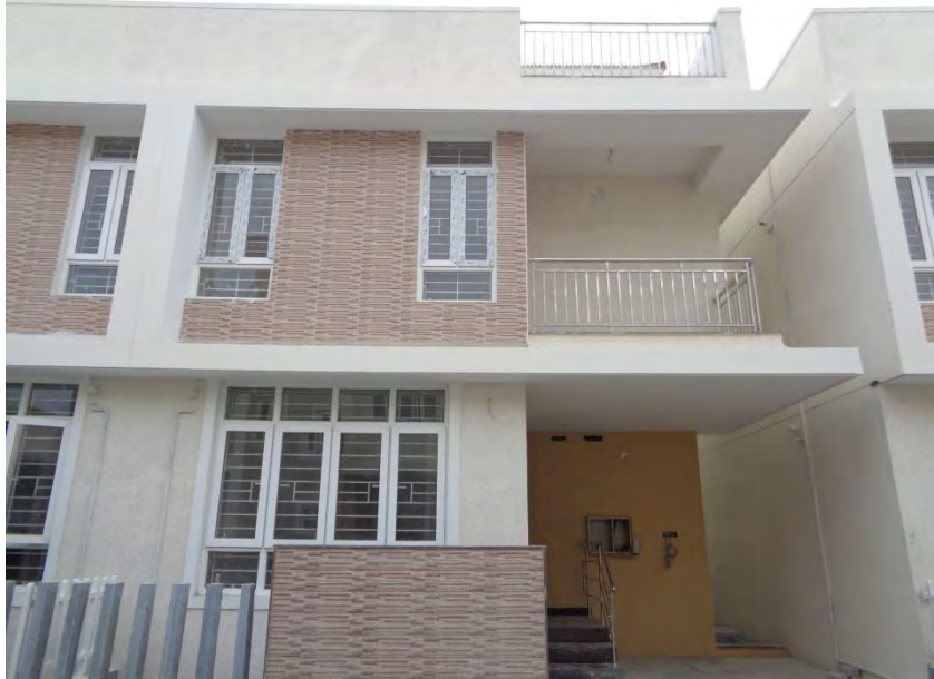
Flooring and painting completed
