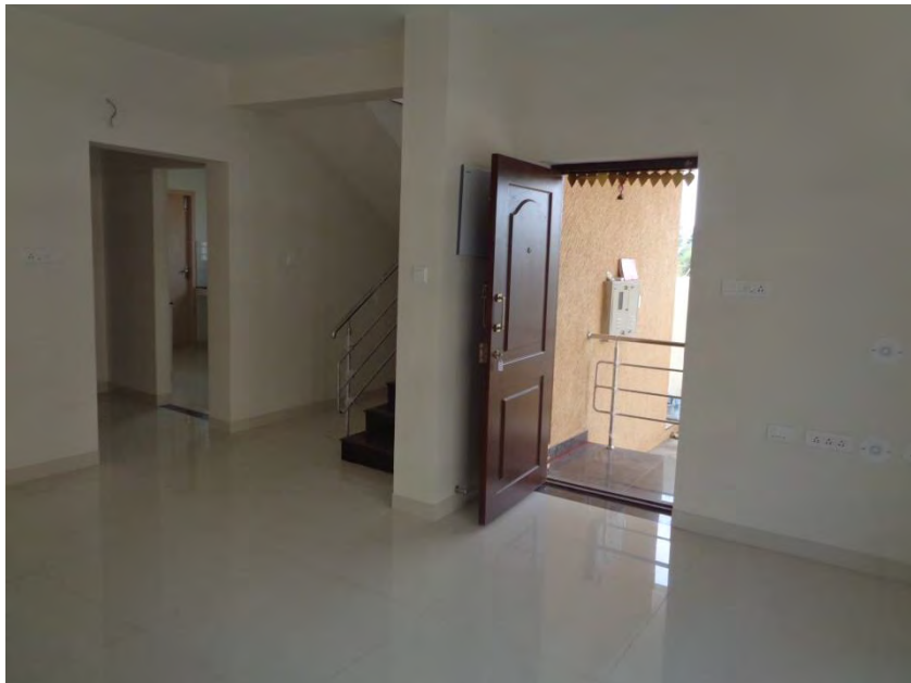
Flooring and painting completed
