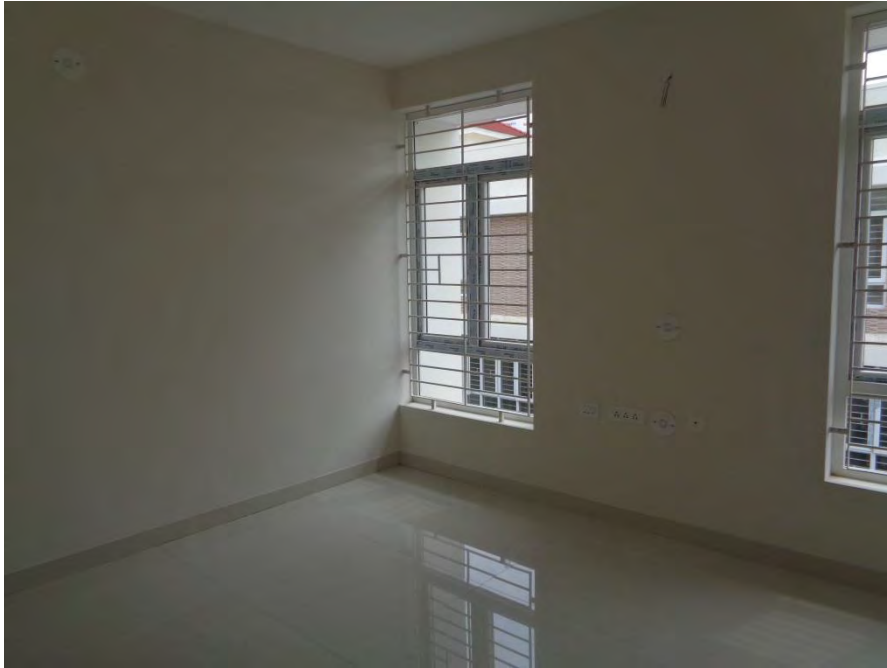
Flooring and painting completed
