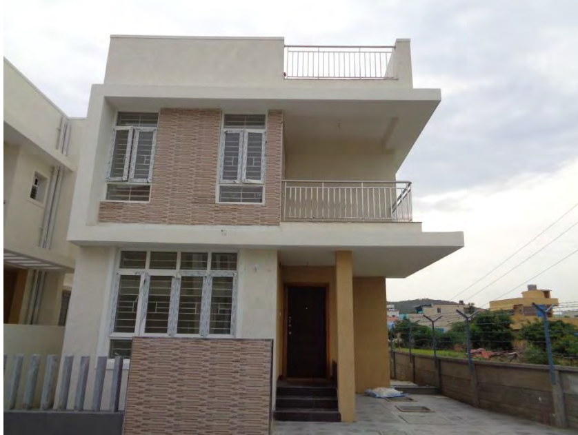
Flooring and painting completed
