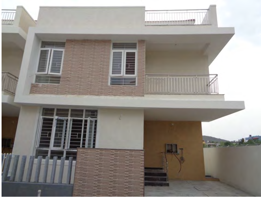
Flooring and painting completed
