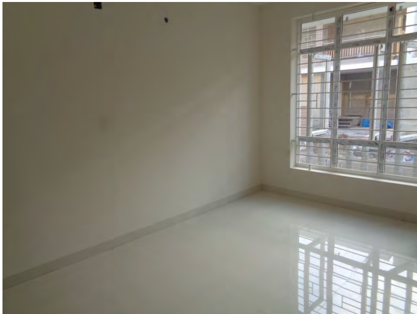
Flooring and painting completed
