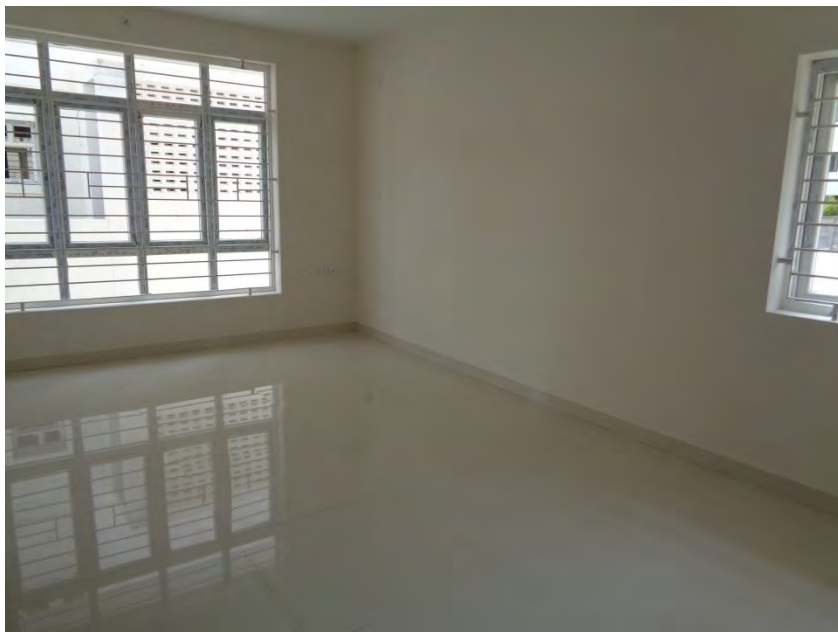
Flooring and painting Completed
