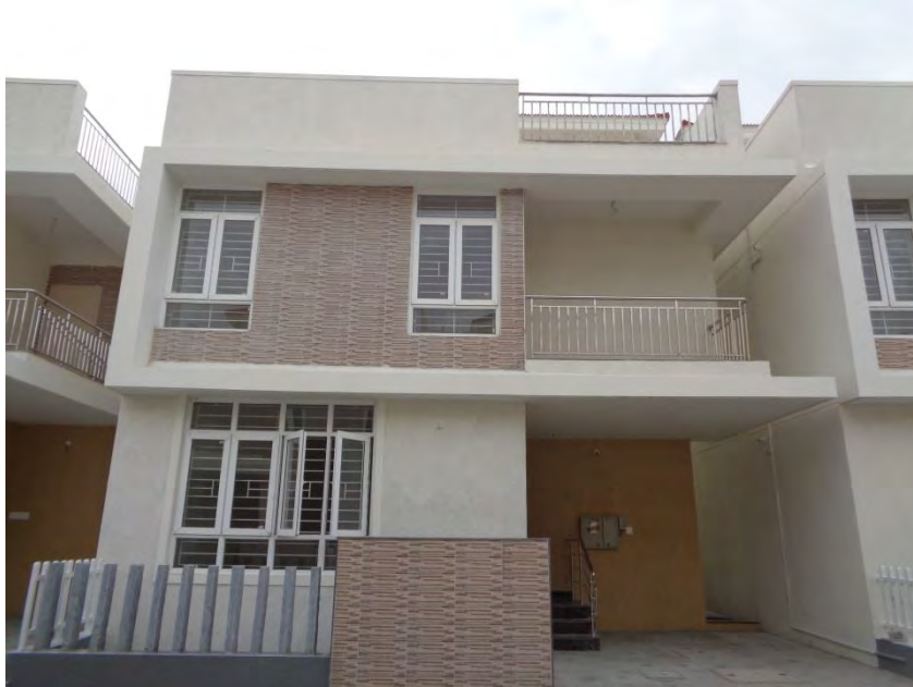
Flooring and painting completed
