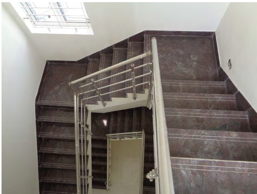
Flooring and painting completed
