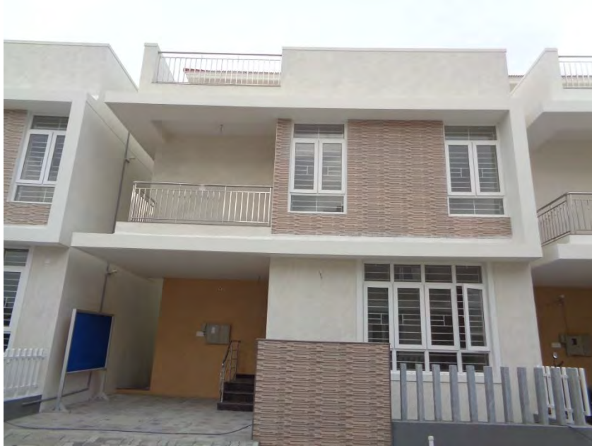
Flooring and painting completed
