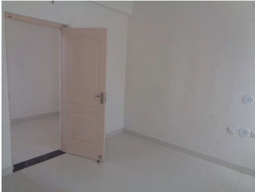
Flooring and painting completed
