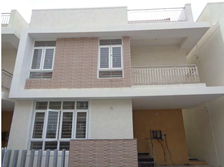
Flooring and painting completed
