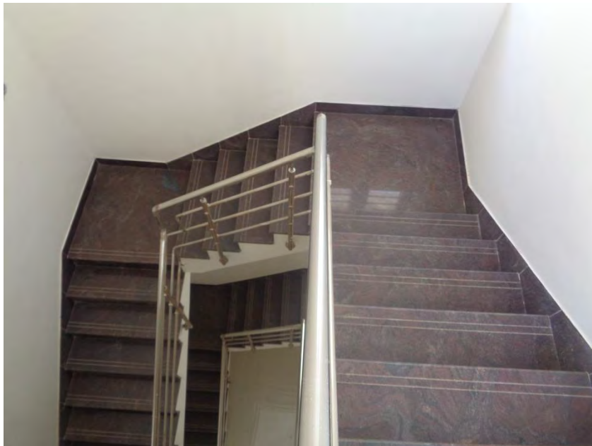
Flooring and painting completed
