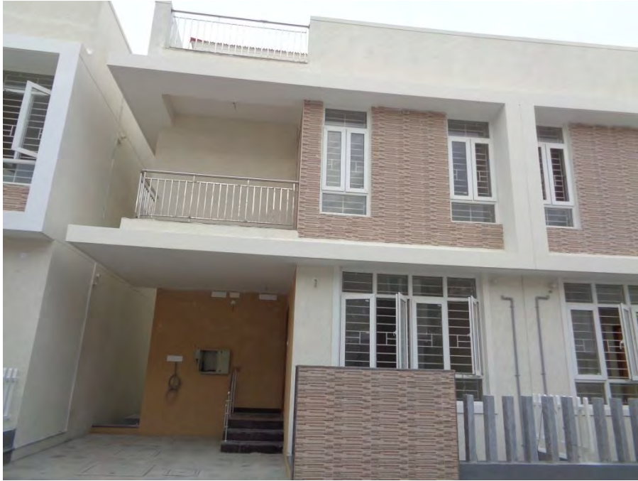
Flooring and painting completed
