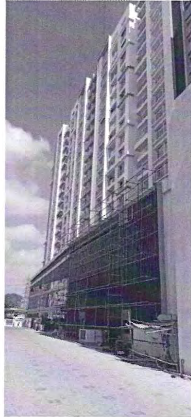
A & B WING – SOUTH SIDE
