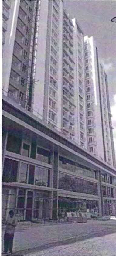
A & B WING - NORTH SIDE
