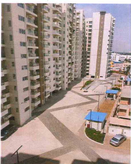
A-BLOCK NORTH DRIVEWAY
