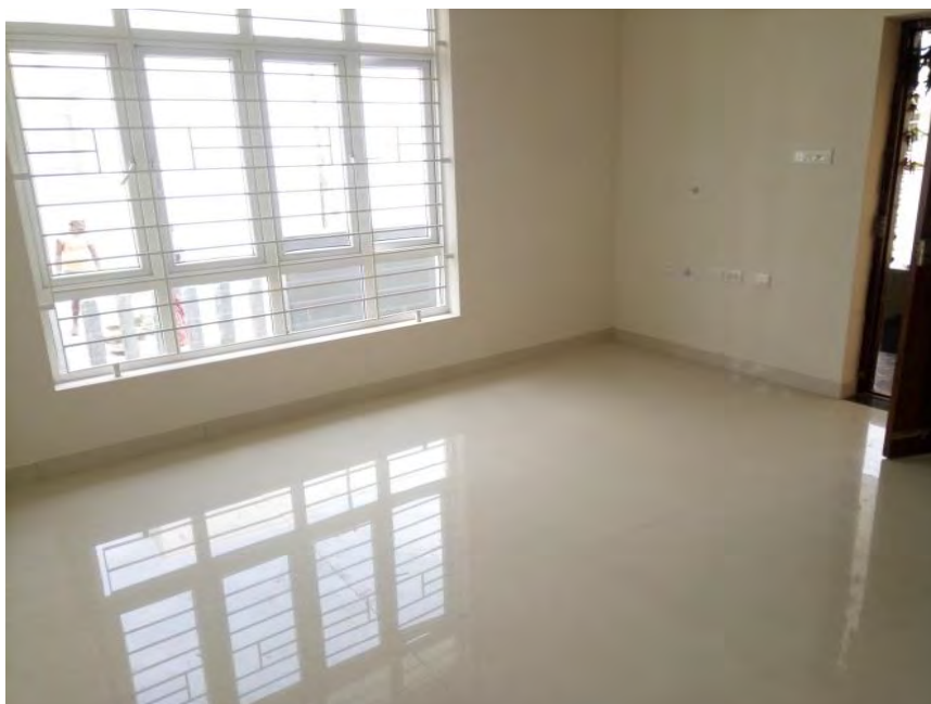
Flooring and painting Completed
