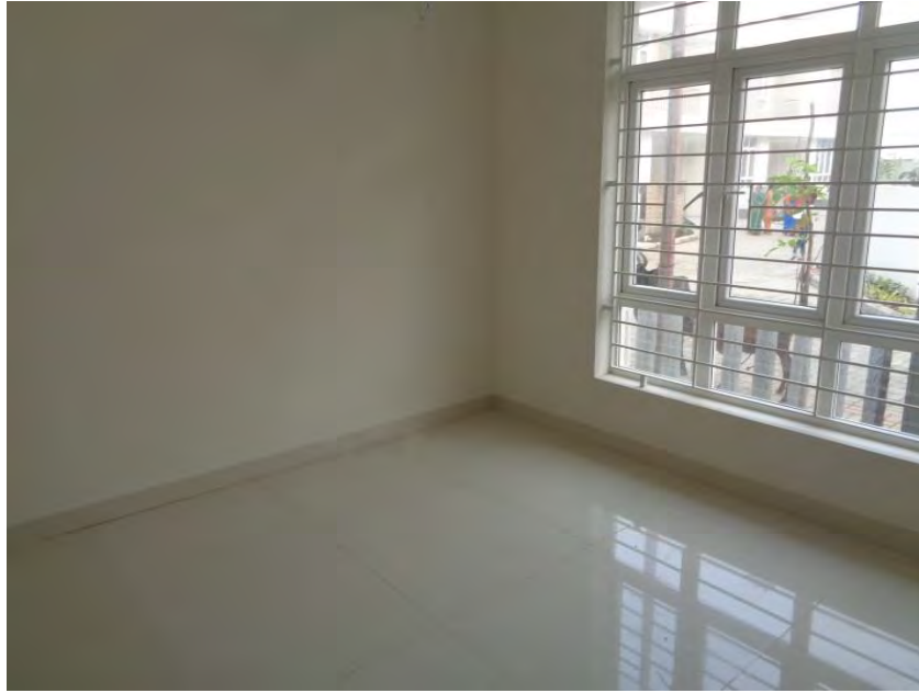
Flooring and painting Completed
