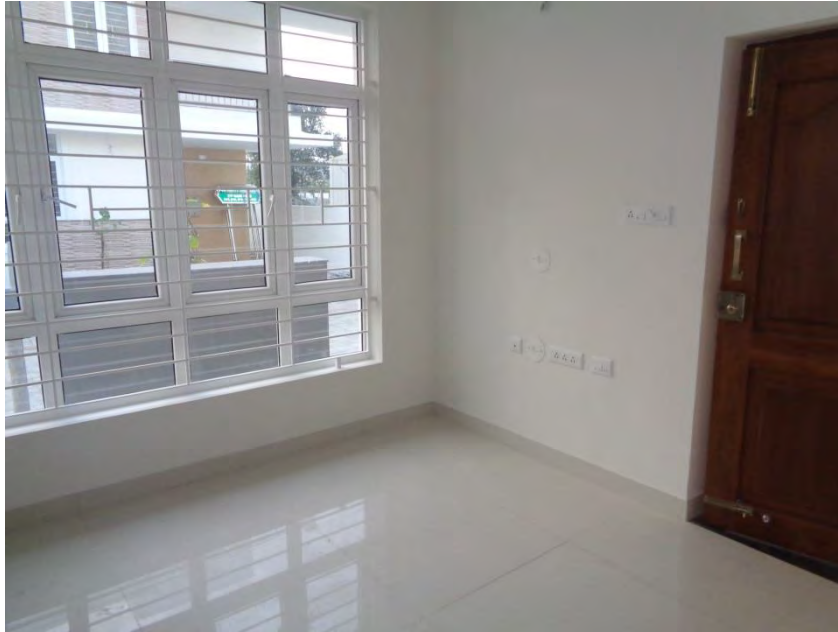
Flooring and painting COMPLETED
