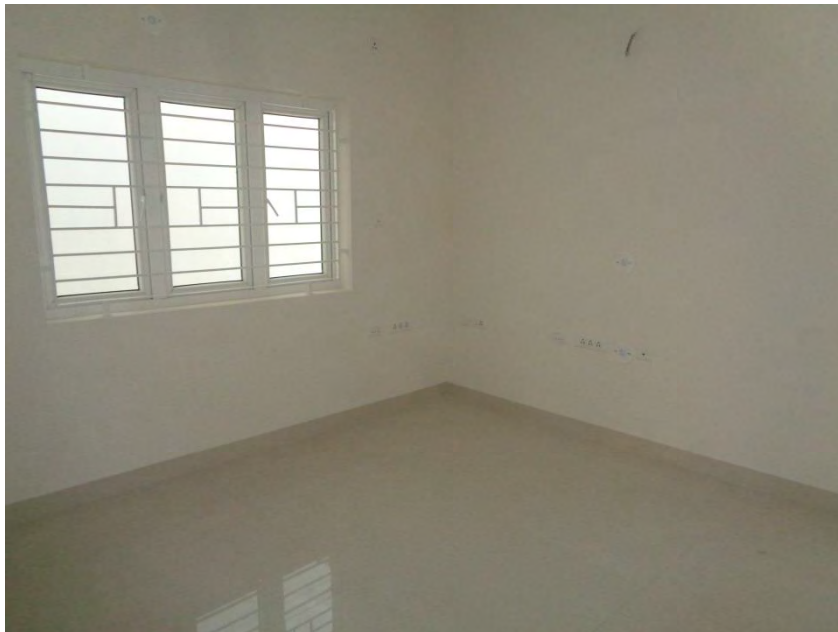
Flooring and painting COMPLETED
