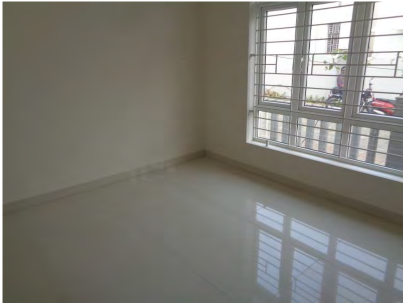
Flooring and painting Completed
