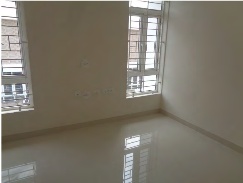
Flooring and painting COMPLETED
