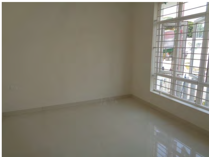
Flooring and painting Completed
