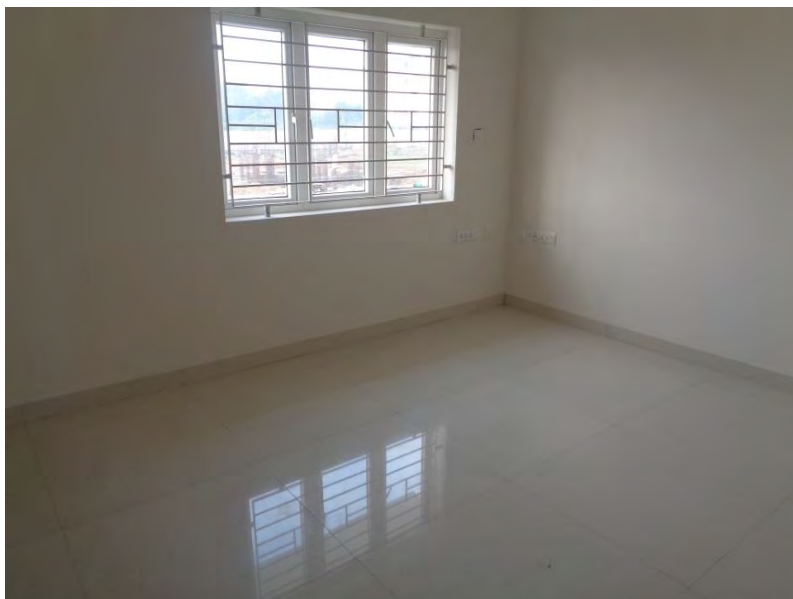
Flooring and painting Completed
