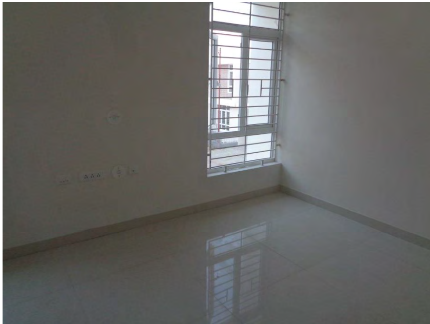
Flooring and painting COMPLETED
