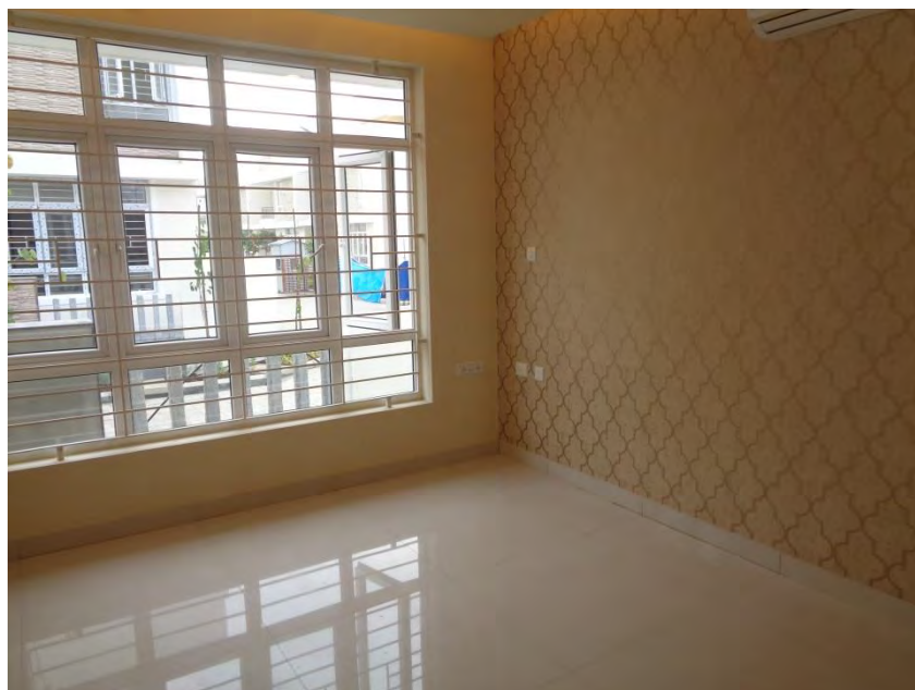
Flooring and painting COMPLETED
