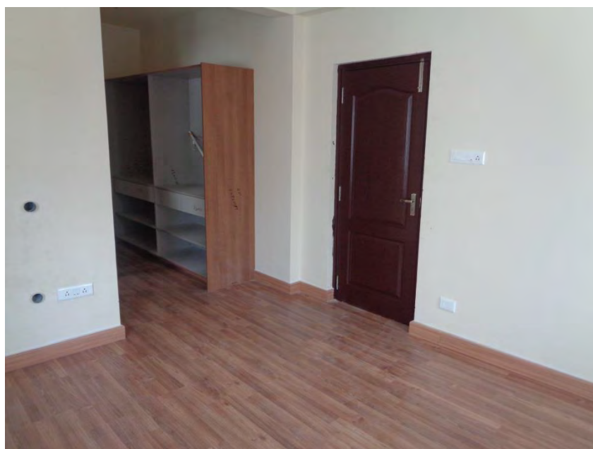
Flooring and painting COMPLETED
