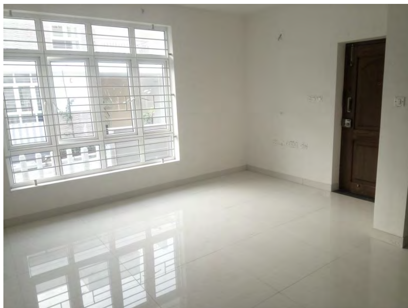
Flooring and painting COMPLETED
