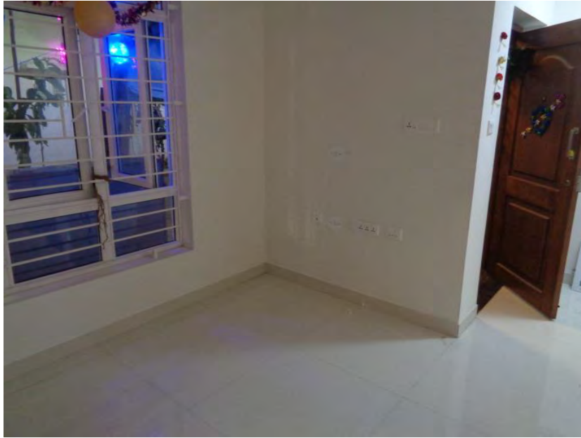
Flooring and painting COMPLETED
