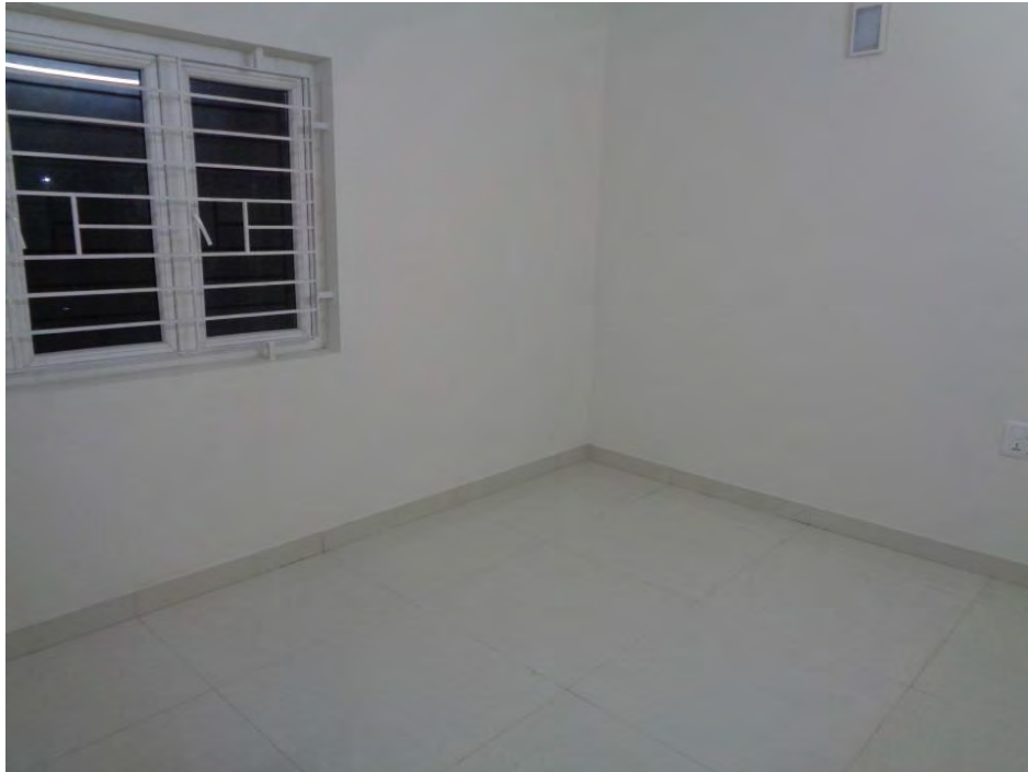
Flooring and painting COMPLETED
