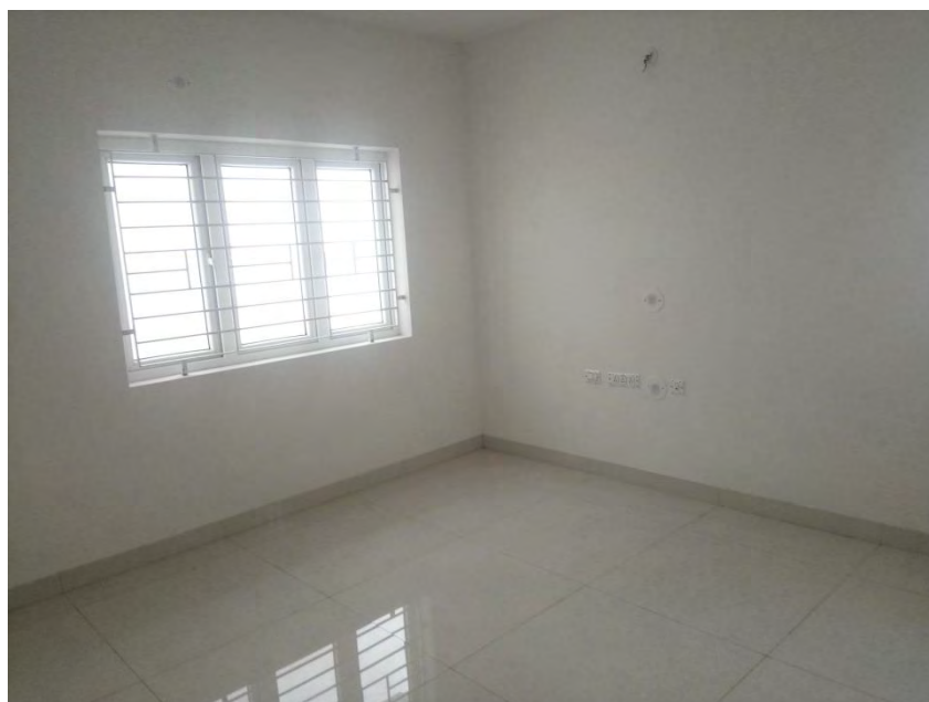
Flooring and painting COMPLETED
