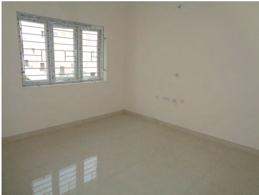
Flooring and painting COMPLETED
