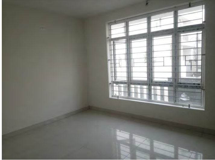
Flooring and painting Completed
