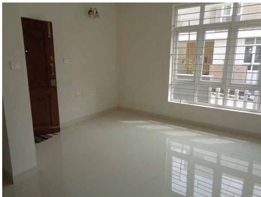
Flooring and painting COMPLETED
