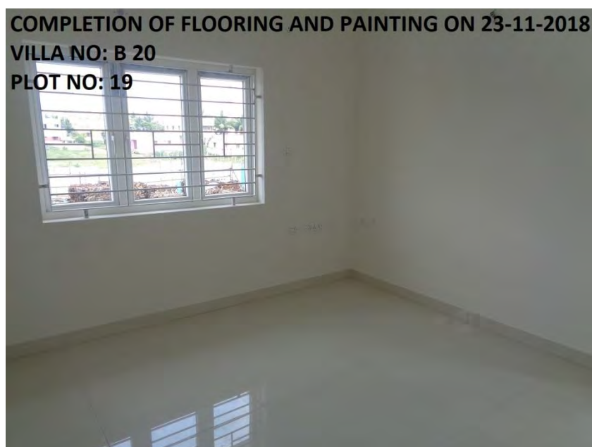
Flooring and painting COMPLETED
