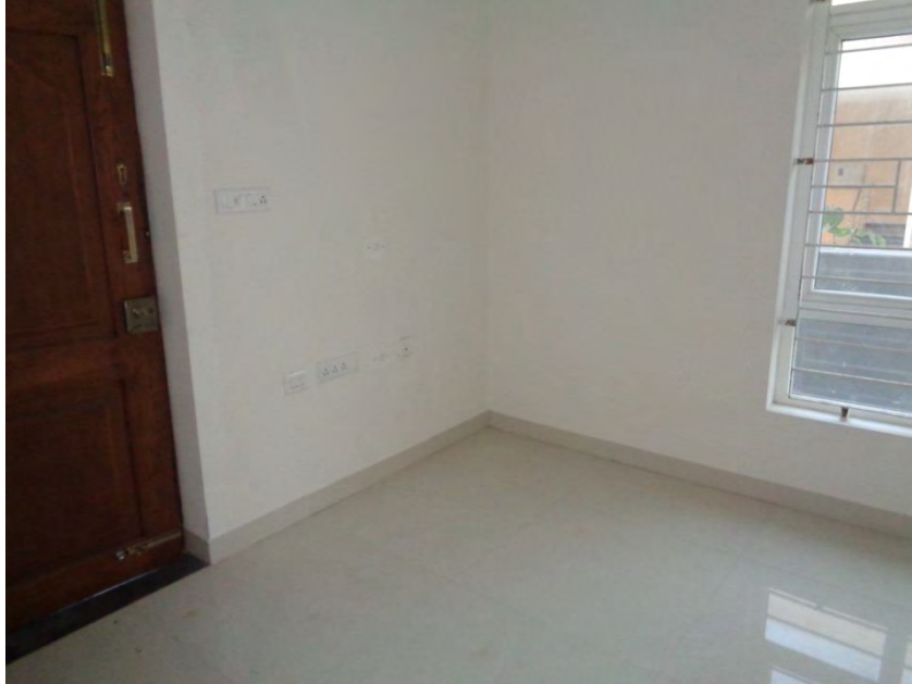
Flooring and painting COMPLETED
