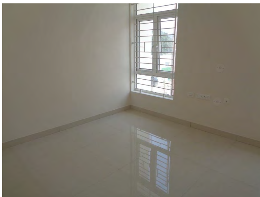
Flooring and painting COMPLETED
