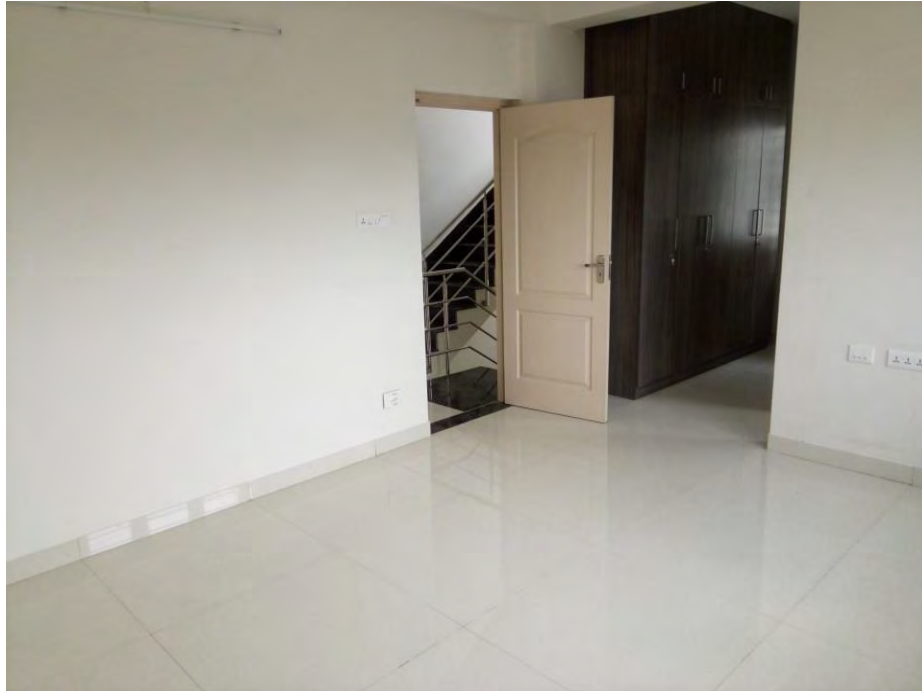
Flooring and painting Completed
