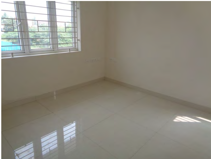
Flooring and painting COMPLETED
