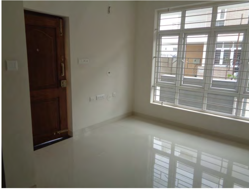
Flooring and painting COMPLETED
