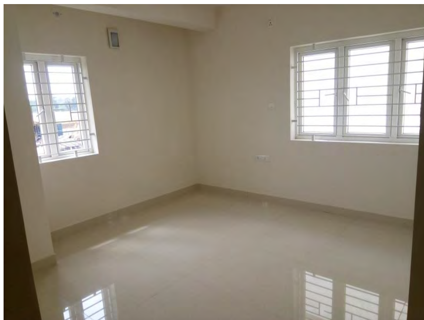
Flooring and painting Completed
