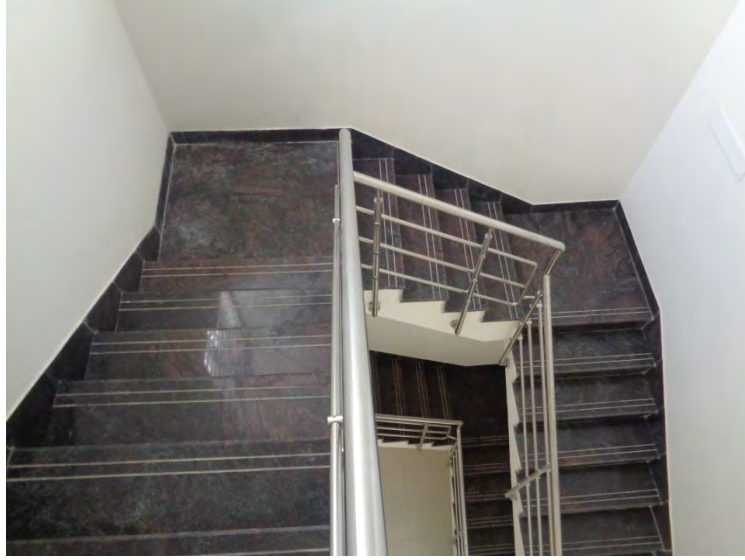
Flooring and painting Completed
