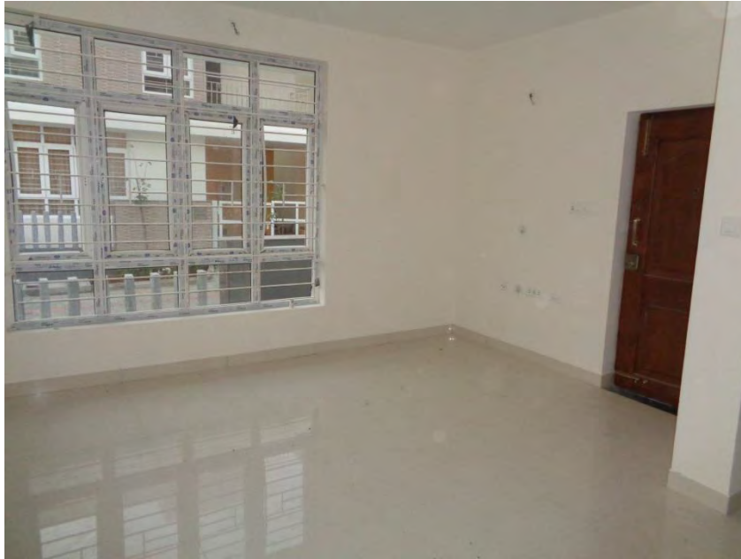
Flooring and painting COMPLETED
