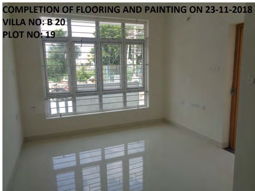
Flooring and painting COMPLETED
