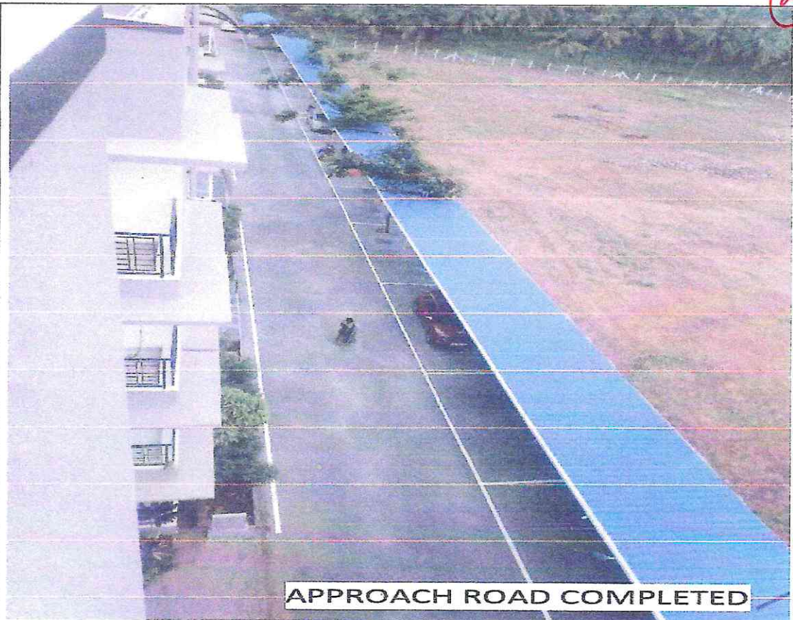
Approach road completed
