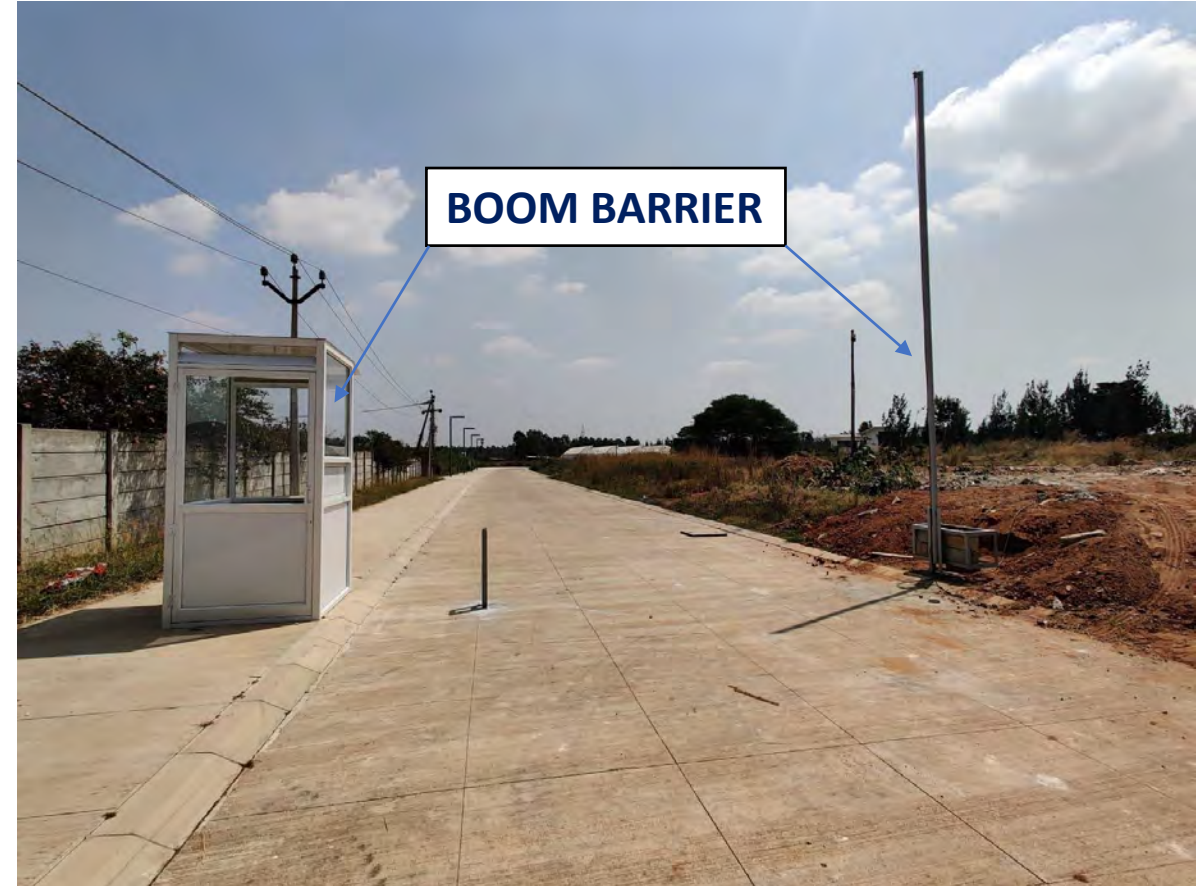
PHASE-4B BOOM BARRIER
