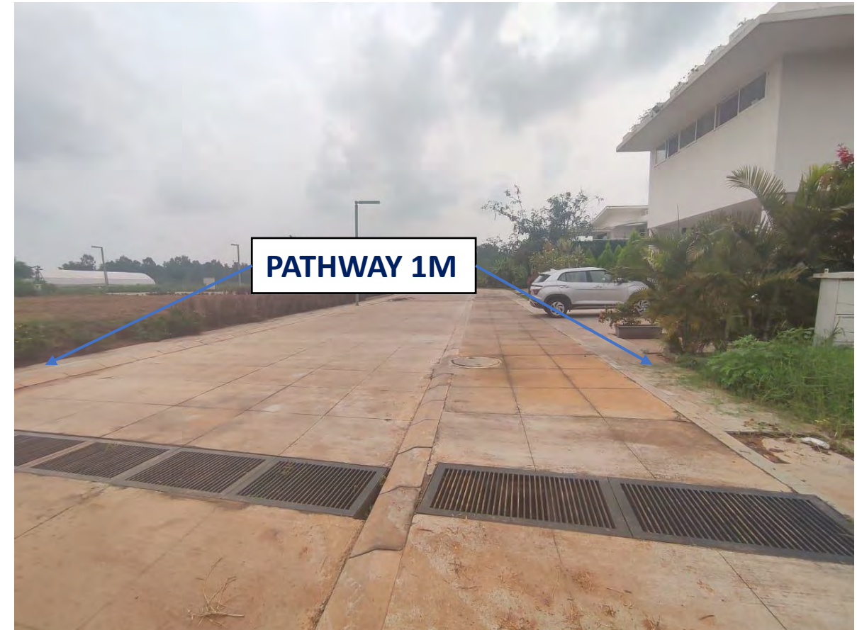
PHASE-4B ROAD ALONG CARPARK AND PATHWAY
