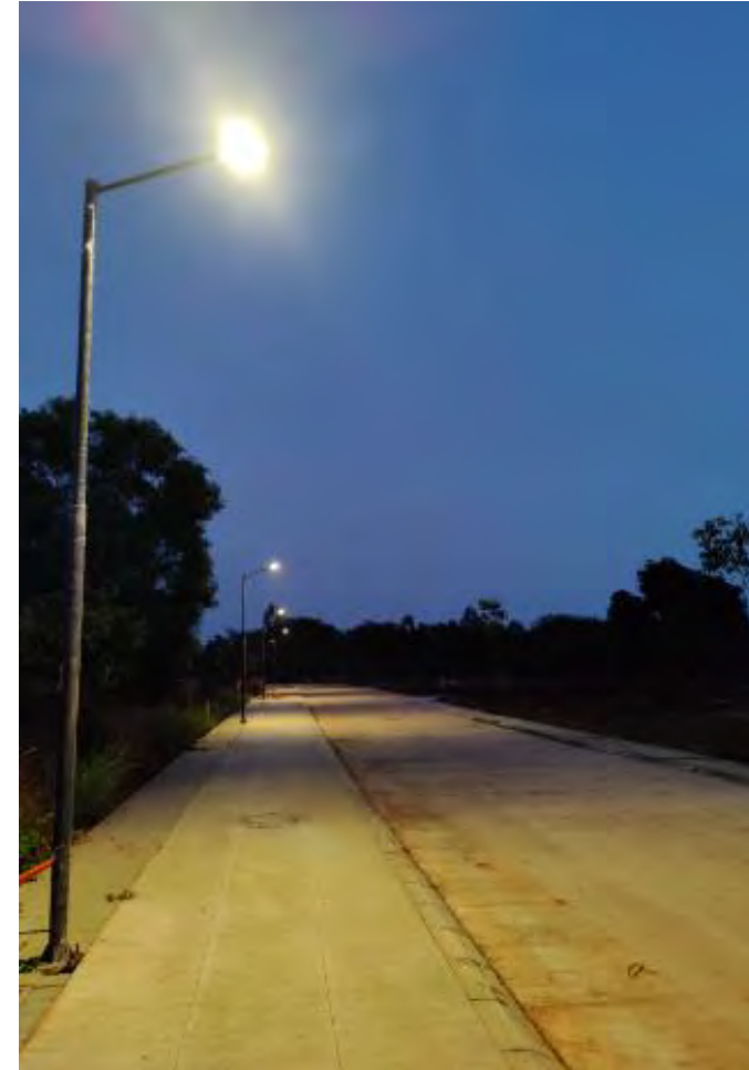
STREET LIGHT WORK
