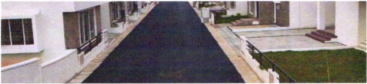
BT COMPLETED IN INTERNAL ROAD
