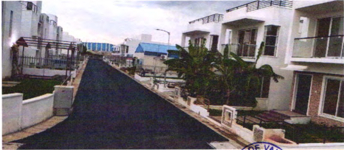
BT COMPLETED IN INTERNAL ROAD
