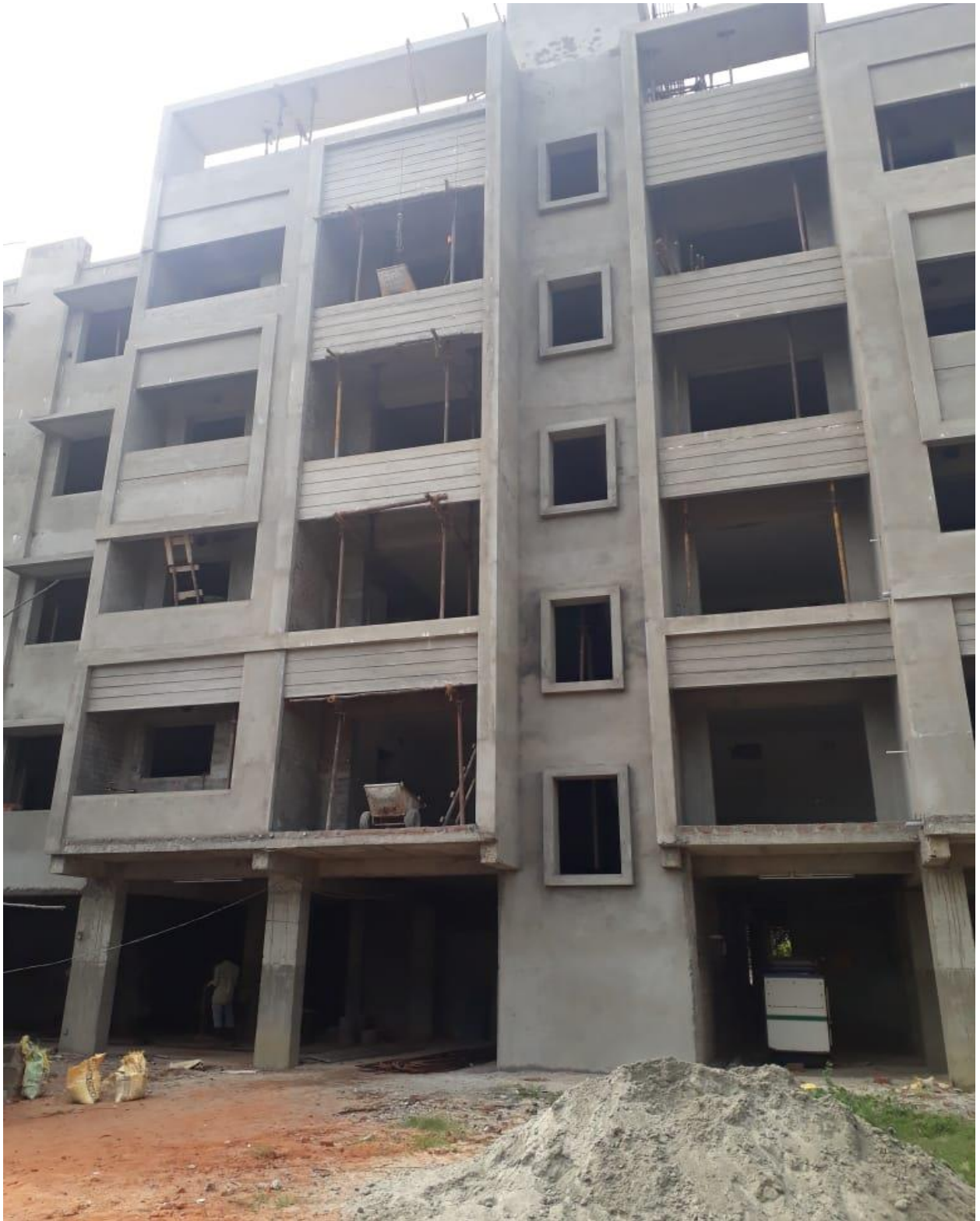
Elevation from the East
