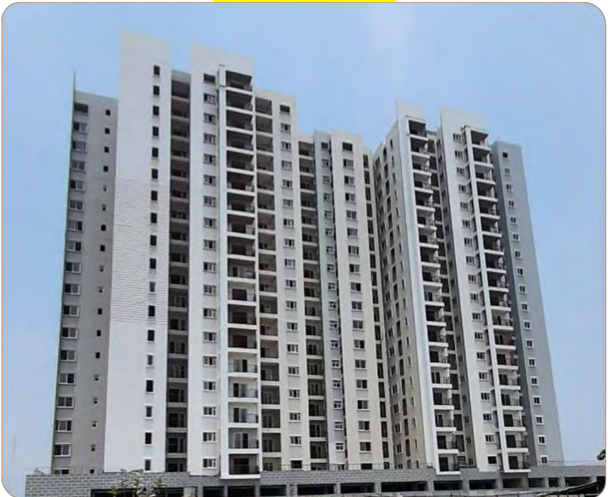
C7 Tower South Side View
