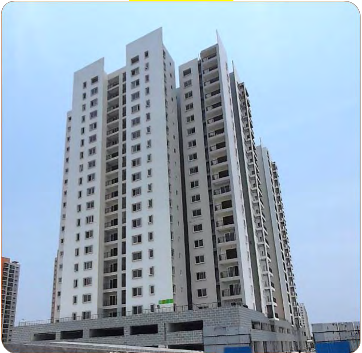
C7 Tower West Side View
