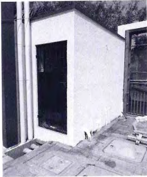
STP plant room and Fire Fighting line:
