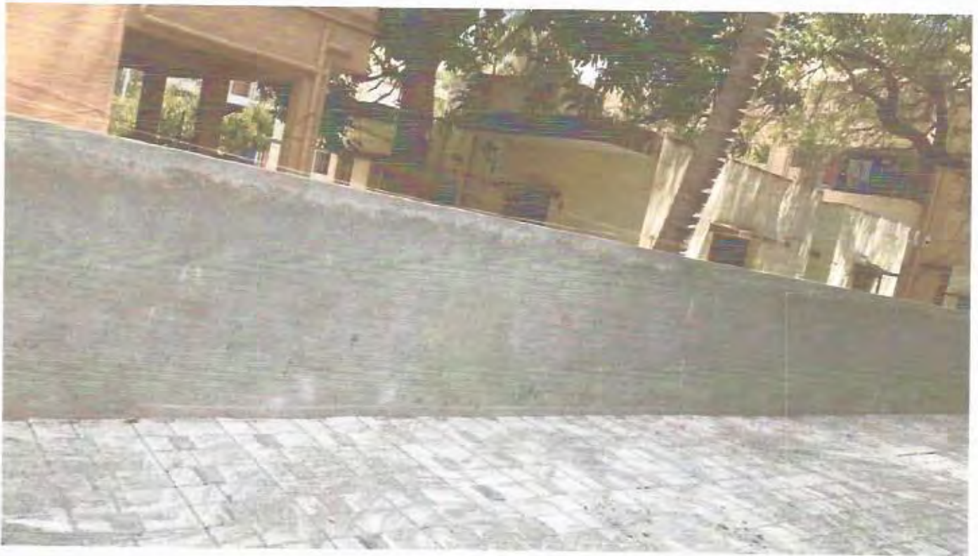
All side compound wall with gate
