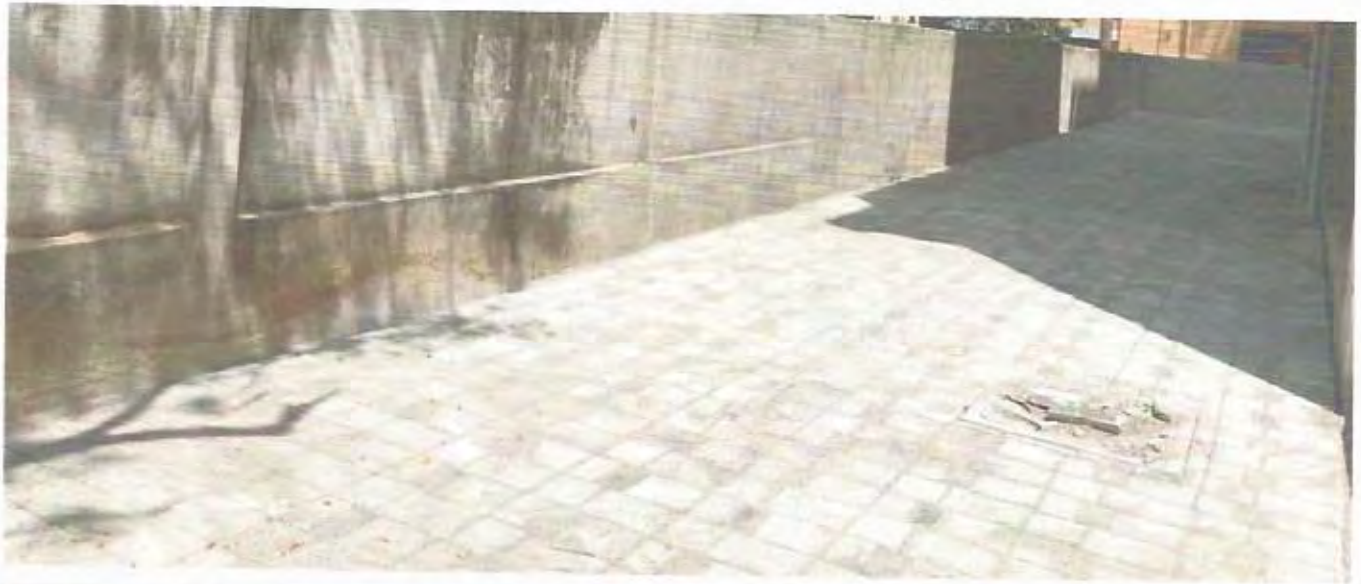
All side compound wall with gate
