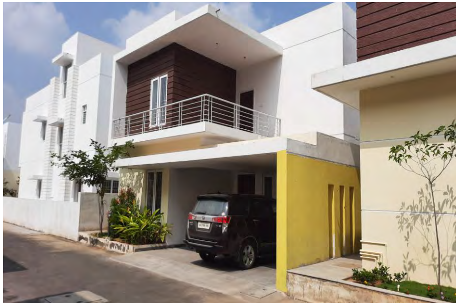
Image Showing: i42 - External painting Completed.
