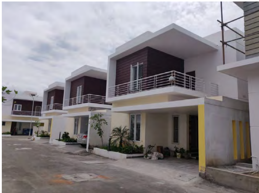
Image Showing: K60 K61 K 62- External painting completed.
