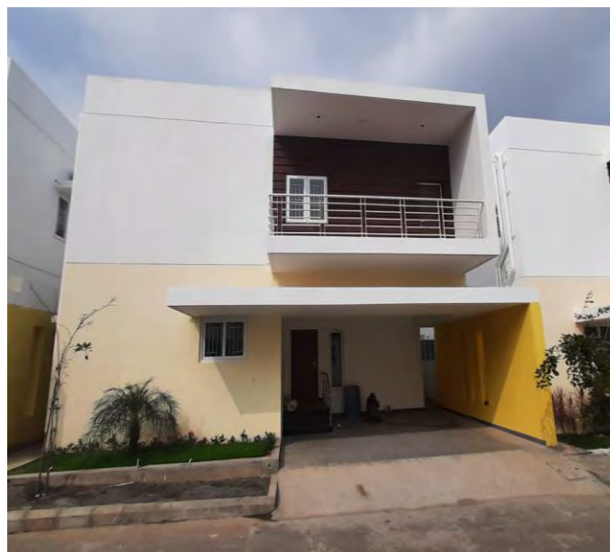
Image Showing: L76 – External painting completed.
