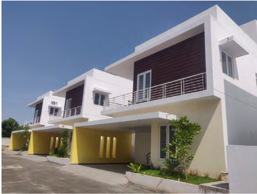
Image Showing: I46, I47, I48 – External painting completed.
