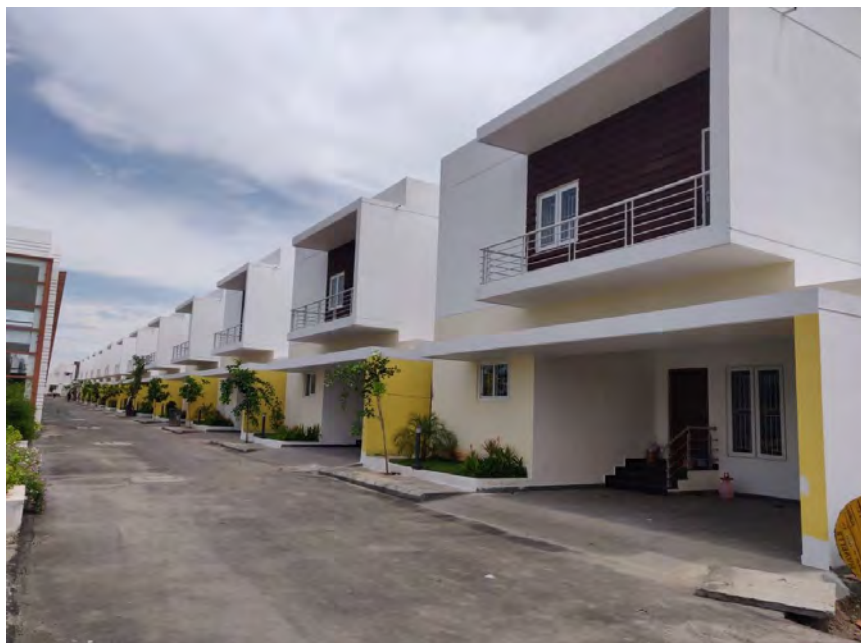
Image Showing: L63 to L67- External painting completed.
