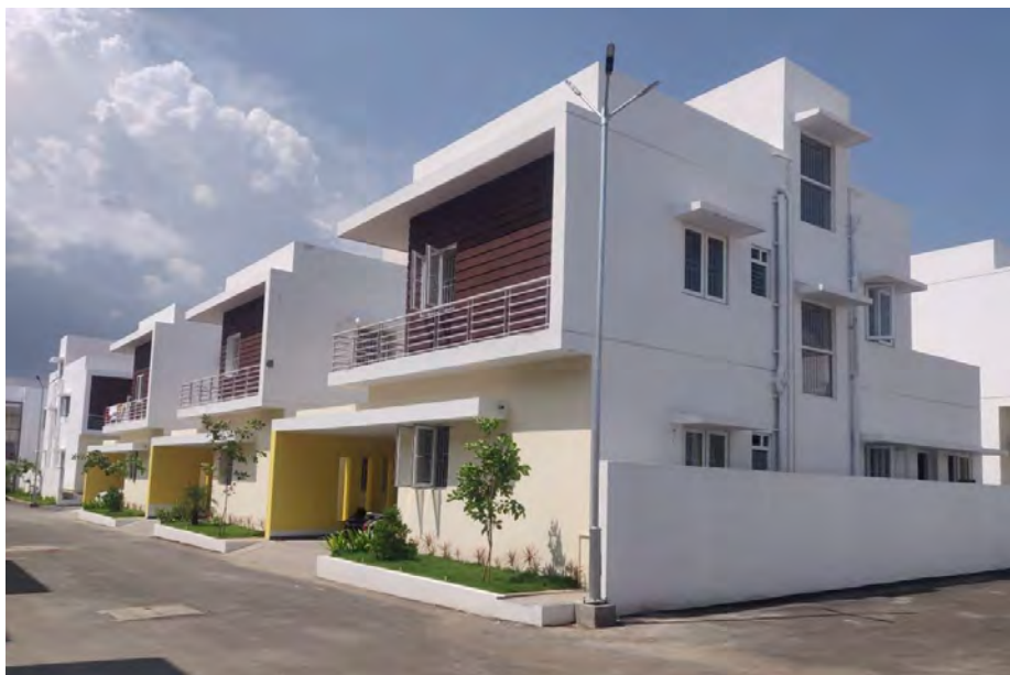
Image Showing: I43, I44, I45- External painting completed
