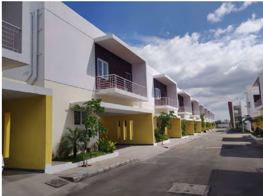
Image Showing: L75 to L68- External painting completed.
