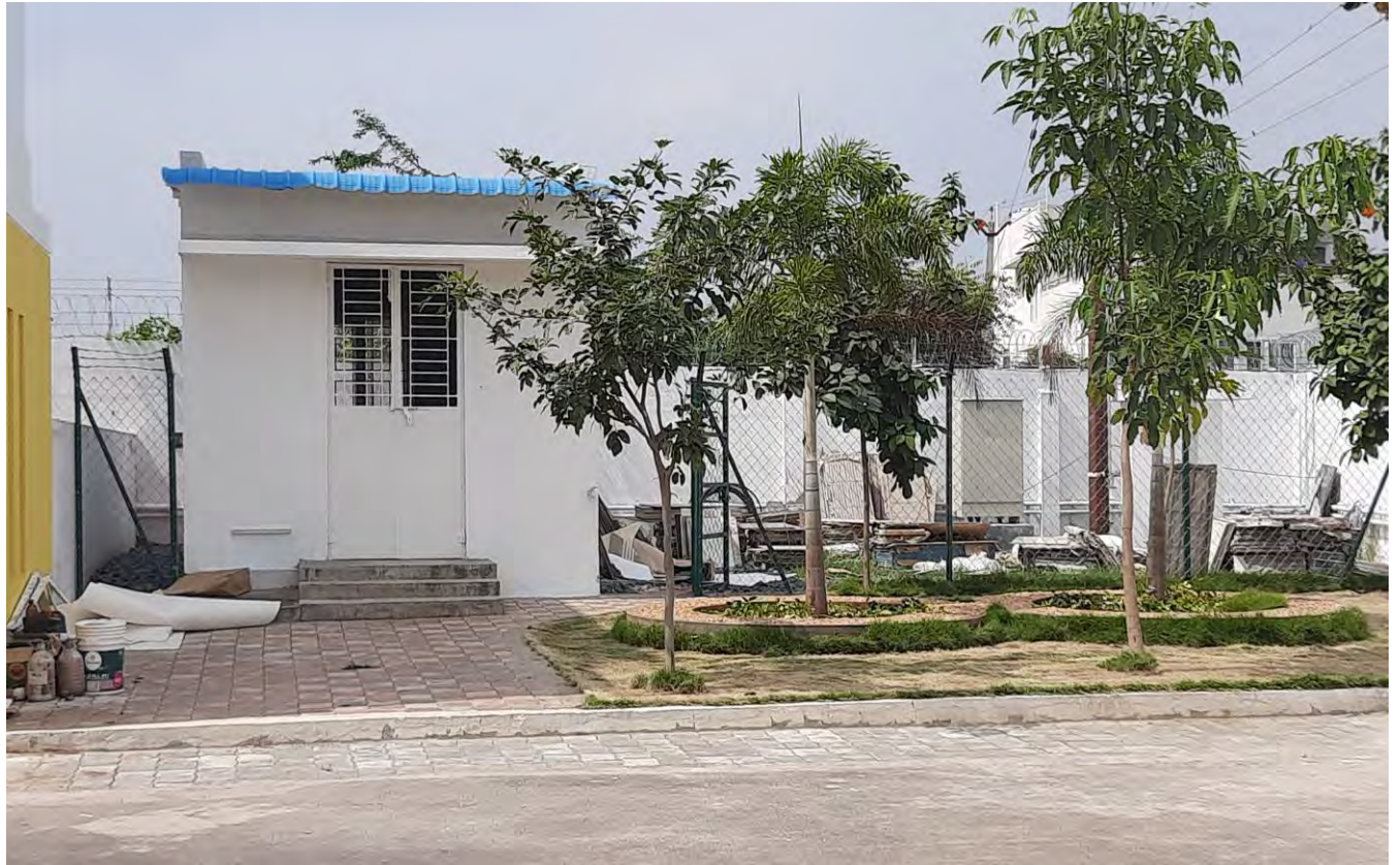
Image Showing: - EB room
