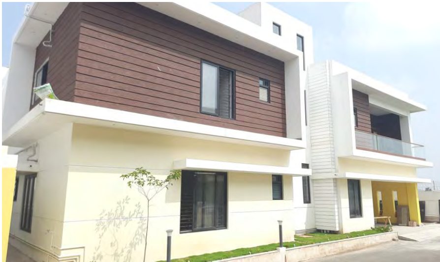
Image Showing: I40 & 41 –External emulsion work completed
