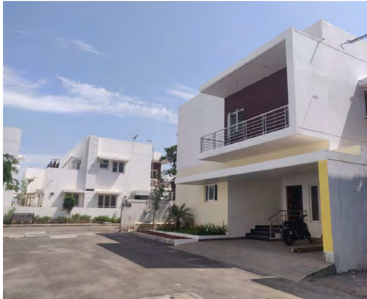
Image Showing: L77- External painting completed.
