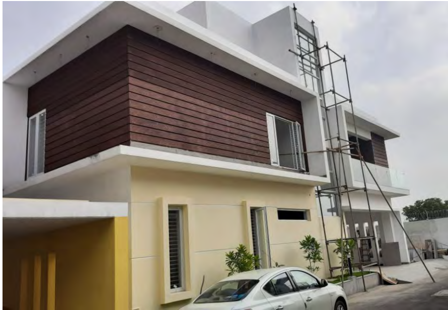
Image Showing: K58&59 External painting completed.
