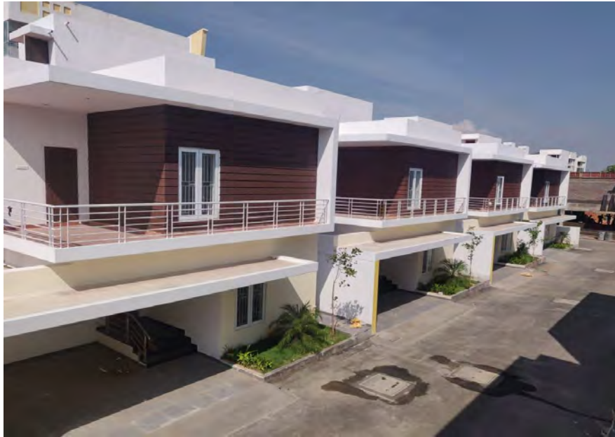
Image Showing: H36, H37, H38, H39 – External Emulsion work Completed
