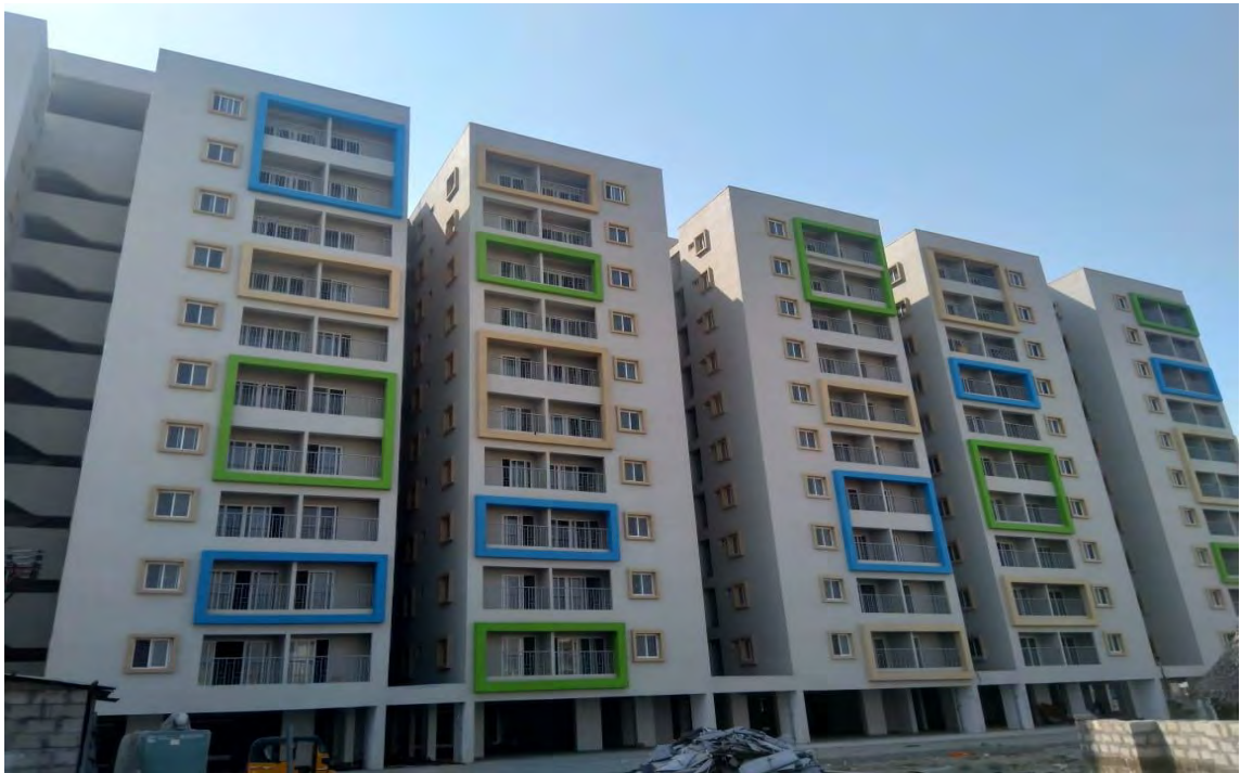
View of C1 Block East Side Elevation
