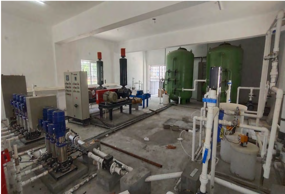
STP-1 – Erection & Commissioning completed.
