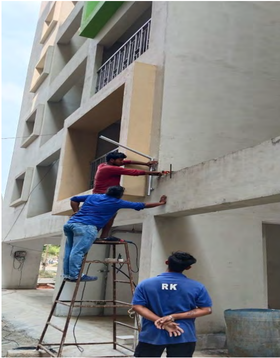
Fixing of Street Light Poles & Wall Brackets in and around D-Type Blocks
