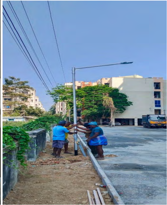
Fixing of Street Light Poles & Wall Brackets in and around D-Type Blocks
