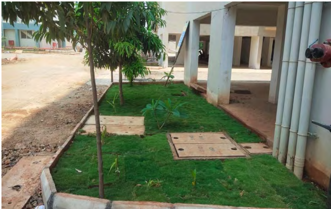
Landscaping work in D2 Block
