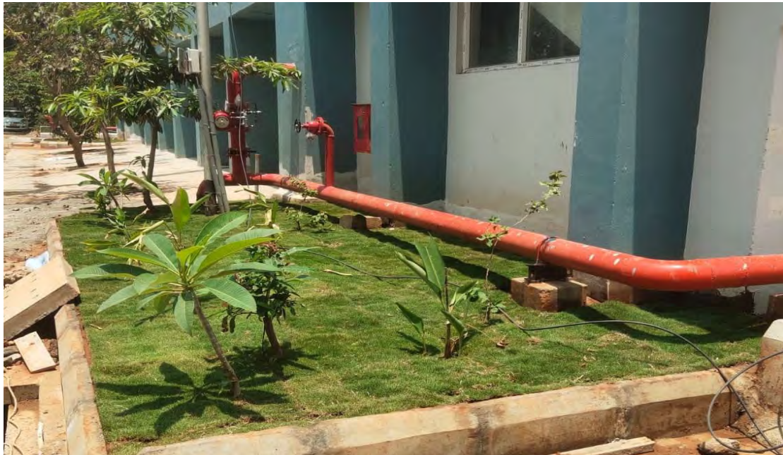
Landscaping work in Community Hall
