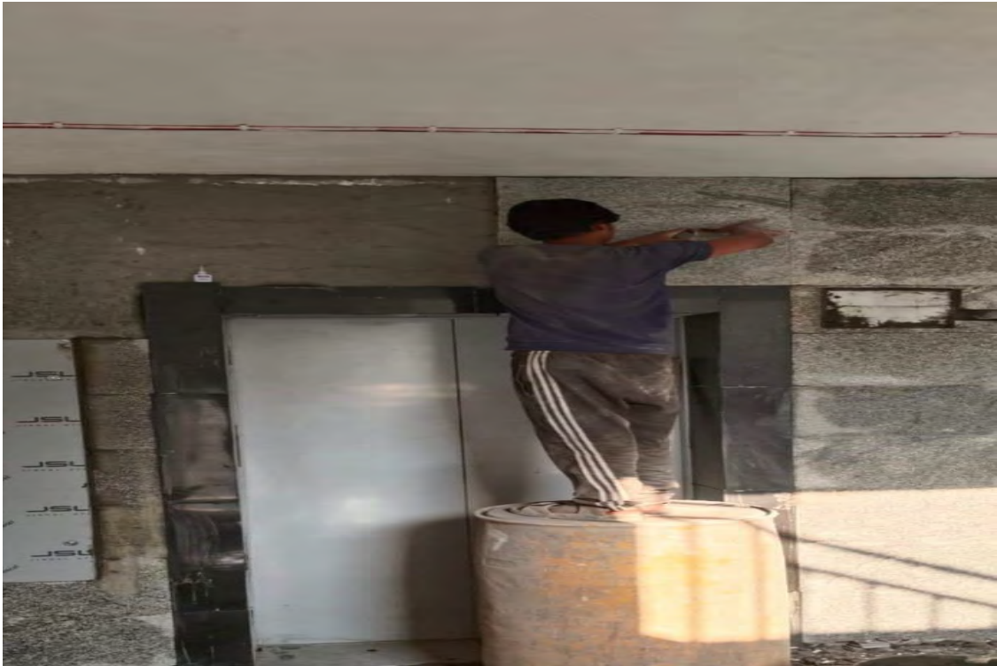
Lift Cladding works in B2 Block
