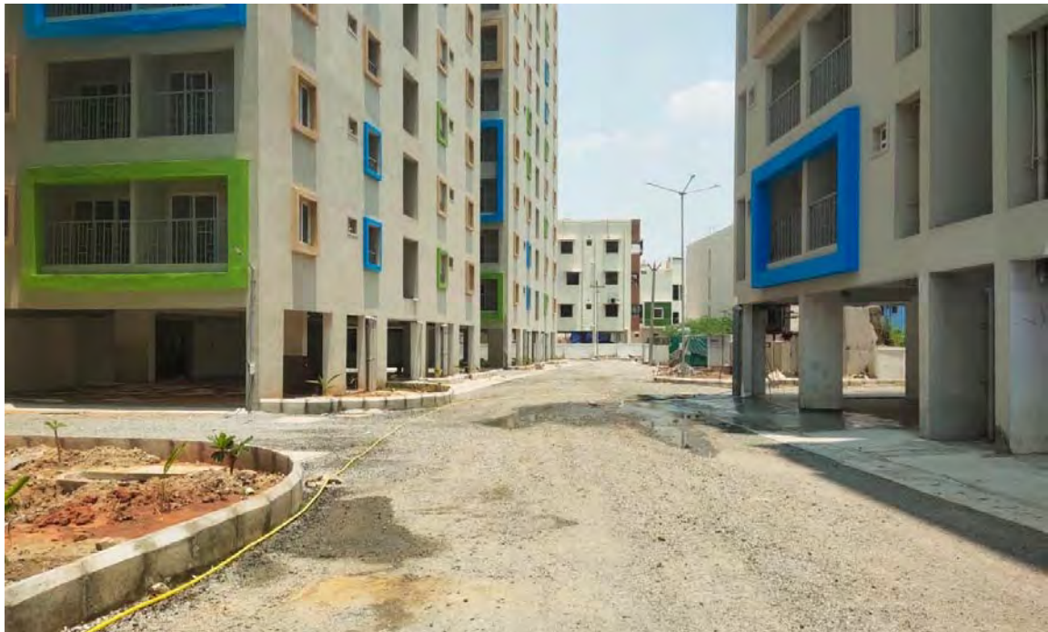
Road Second Layer (W.M.M) completed in South side of Block - C1,C2,C3
