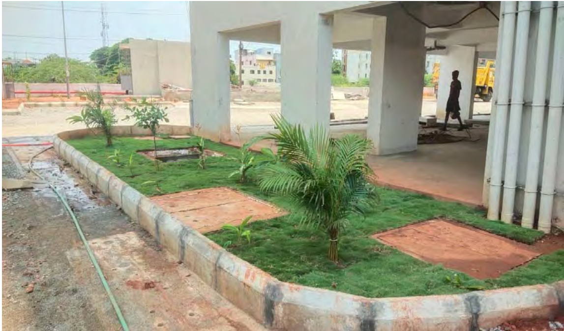
Landscaping work in D1 Block
