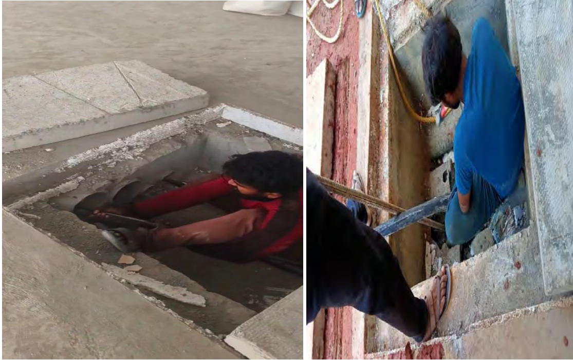
Laying of Electrical Cables from Transformer to Electrical Panel in Each Blocks
