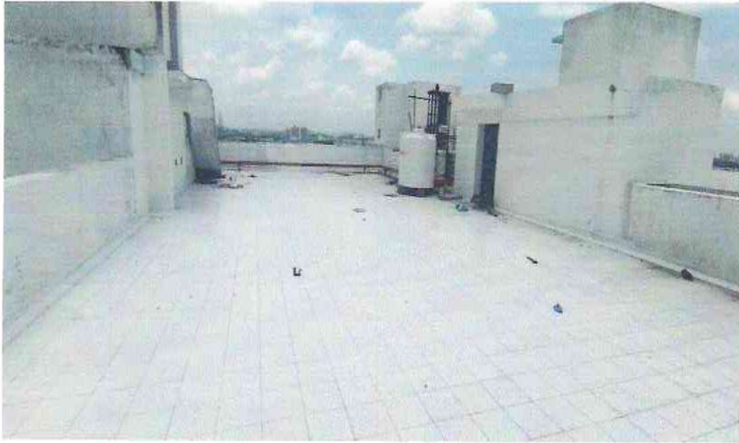
9. Terrace Weather Proofing Completion.
