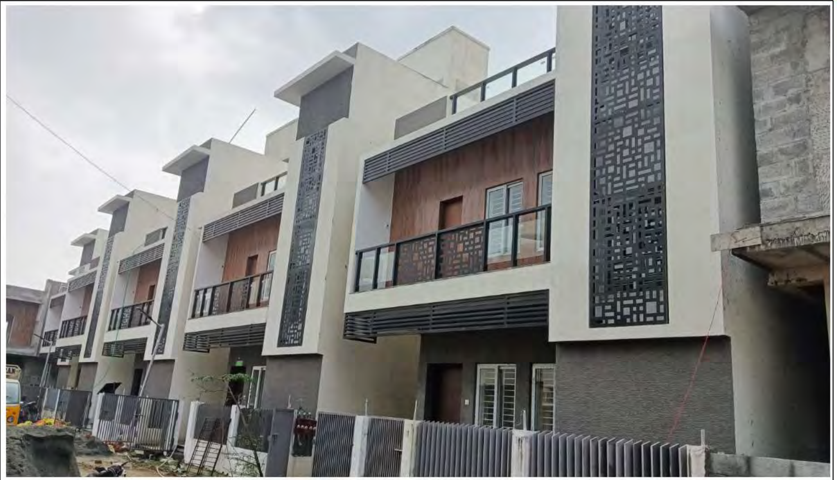
Villa 39-43 – 100% work completed
