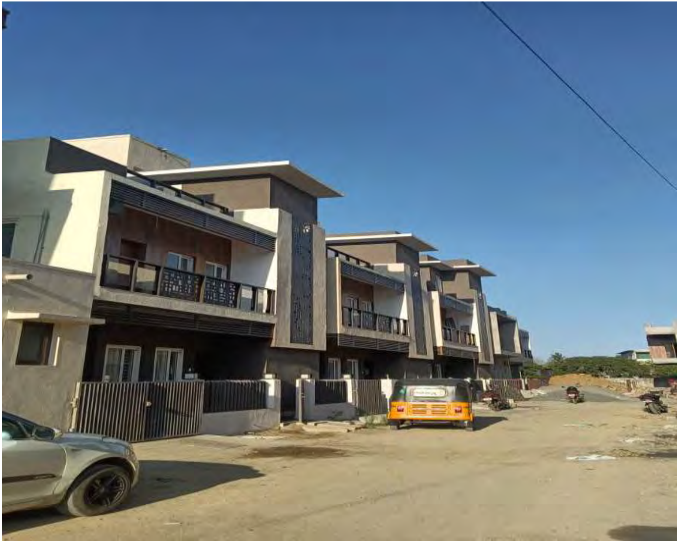
Villa 18-22 – 100% work completed
