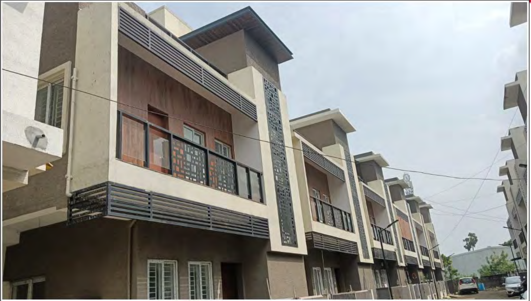
Villa 31-36 – 100% work completed
