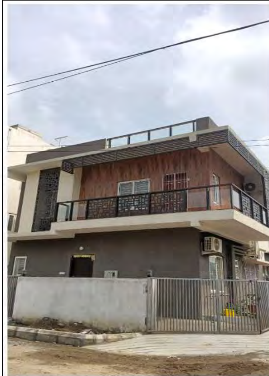
Villa 9 – 100% work completed
