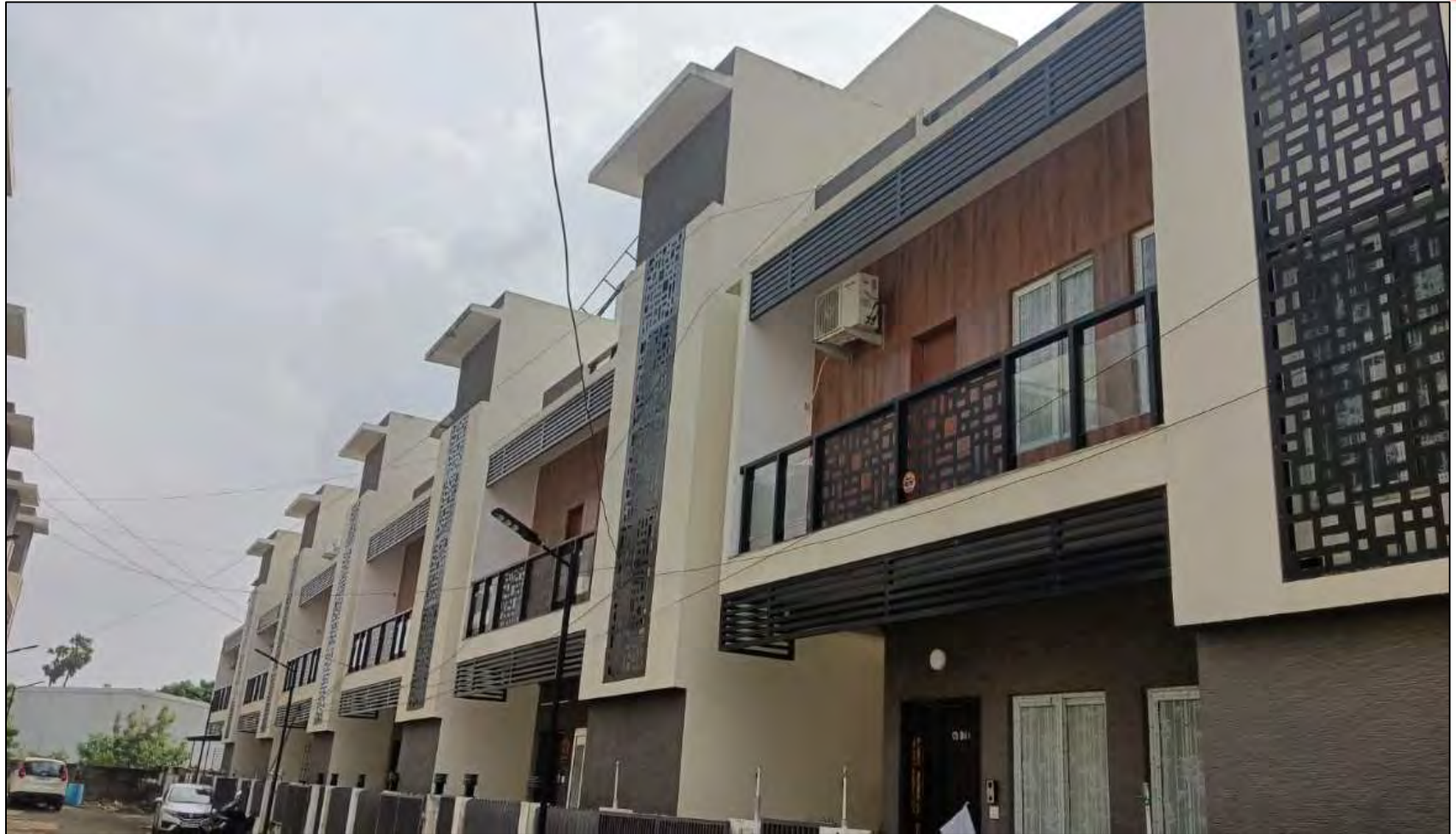
Villa 25-30 – 100% work completed
