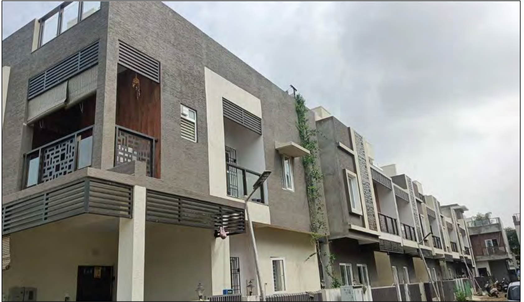
Villa 73-79 – 100% work completed
