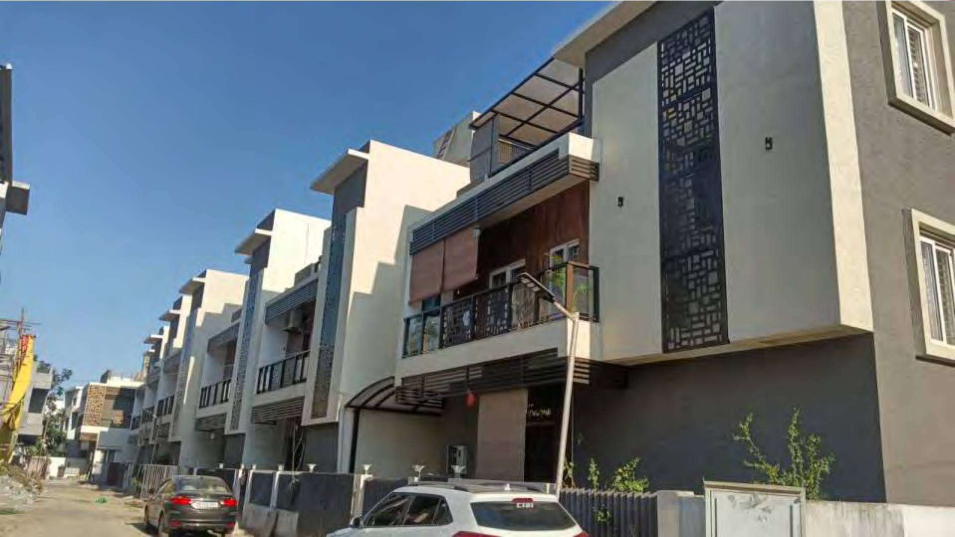
Villa 80 - 86 – 100% Work Completed
