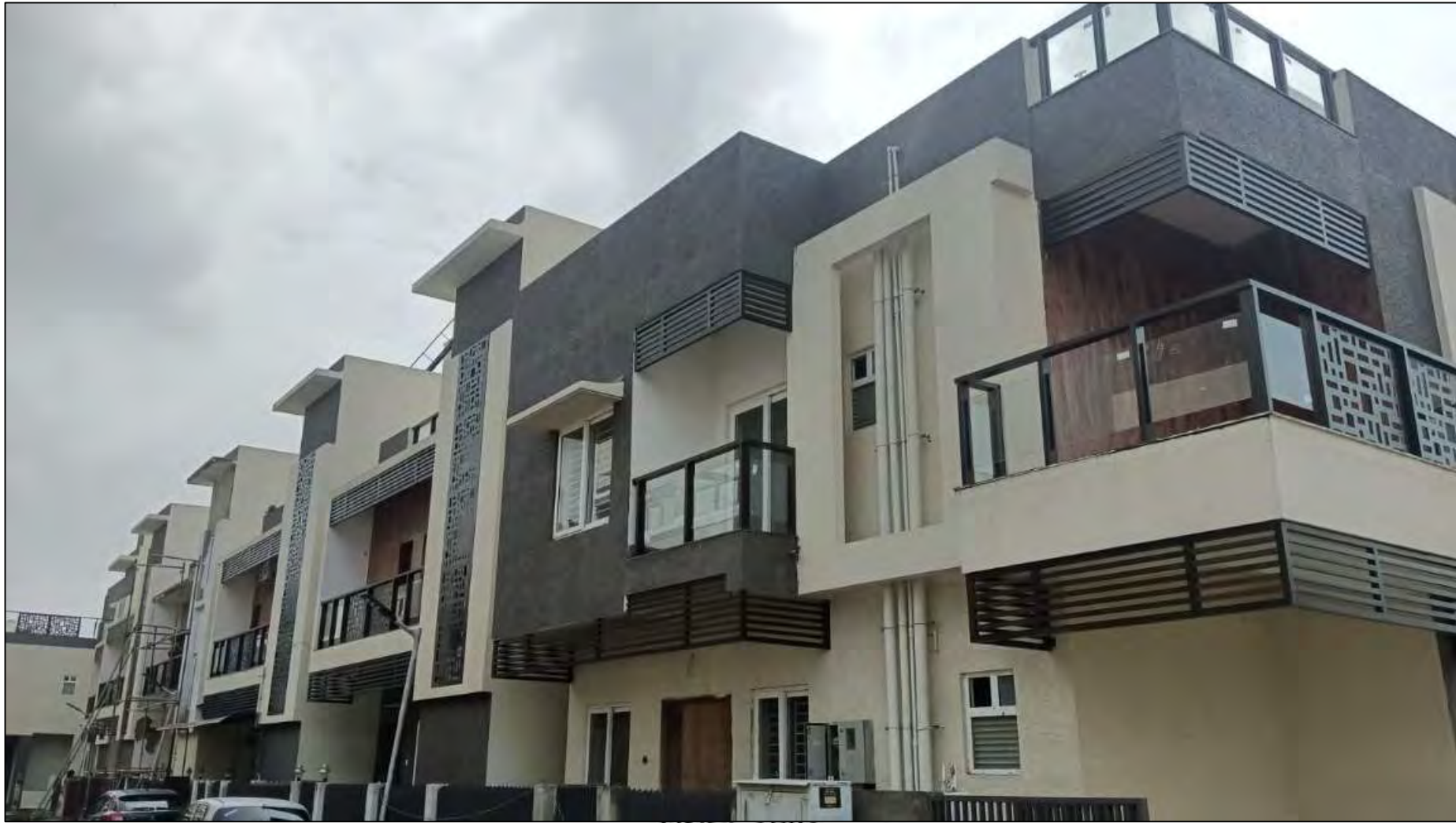
Villa 69-71 – 100% work completed
