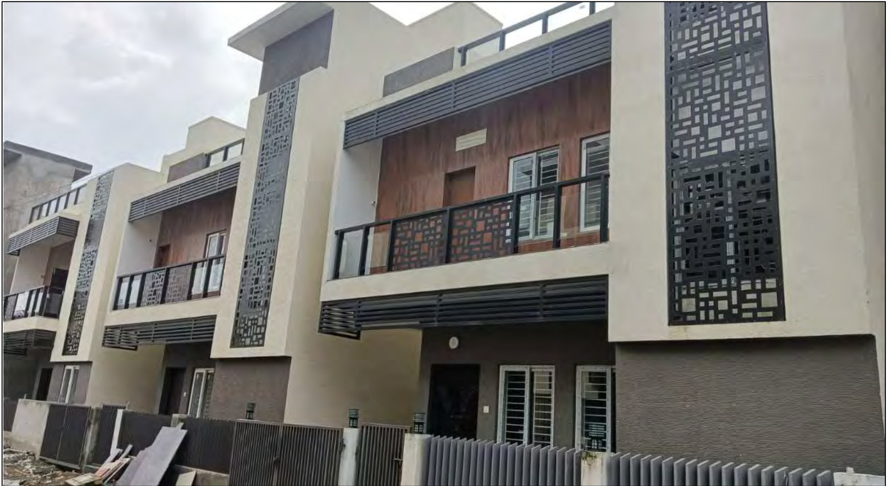
Villa 95 - 97 – 100% work completed
