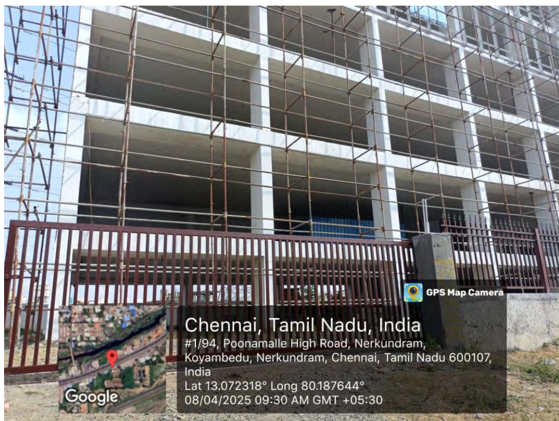
Gate view as on 08/04/2025
