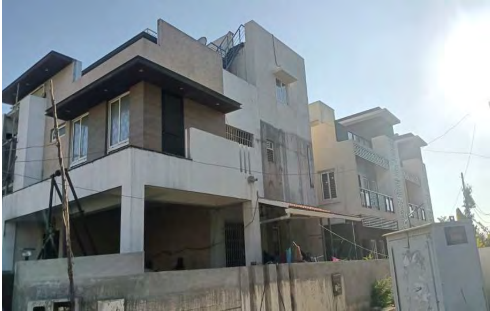
Villa 124-126 works completed
