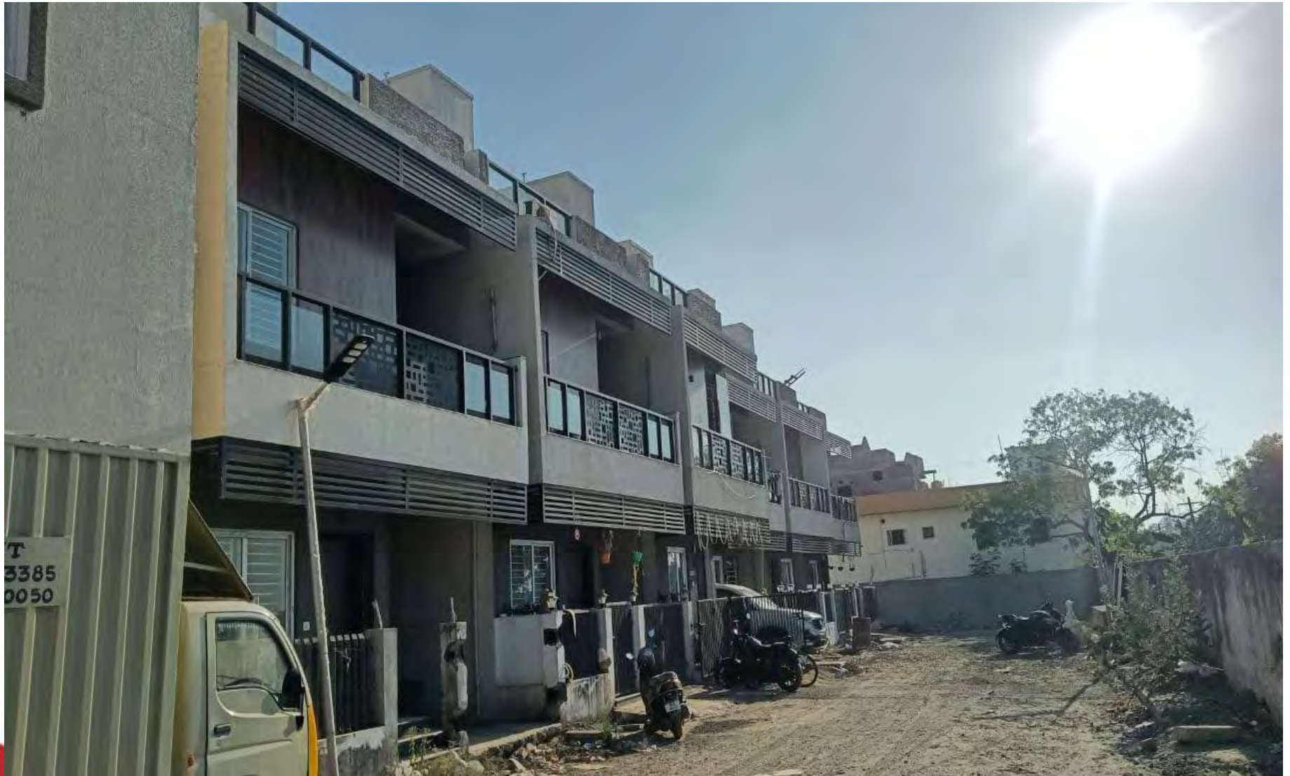
Villa 157 – 162 - 100% Work Completed
