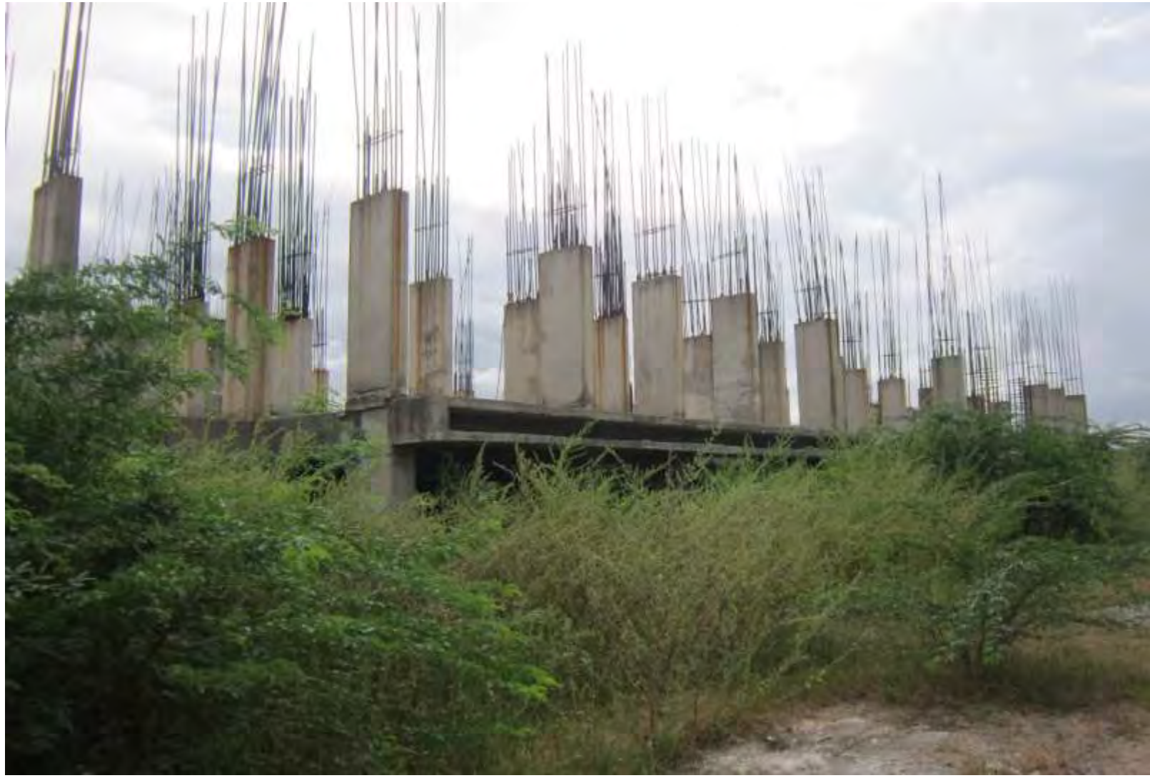
Block D – 1 st floor slab completed and 1 st floor column concrete completed
