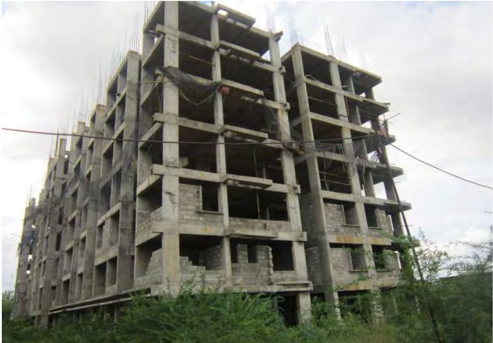
Block A – 7 th floor column and 8 th floor slab shuttering work
