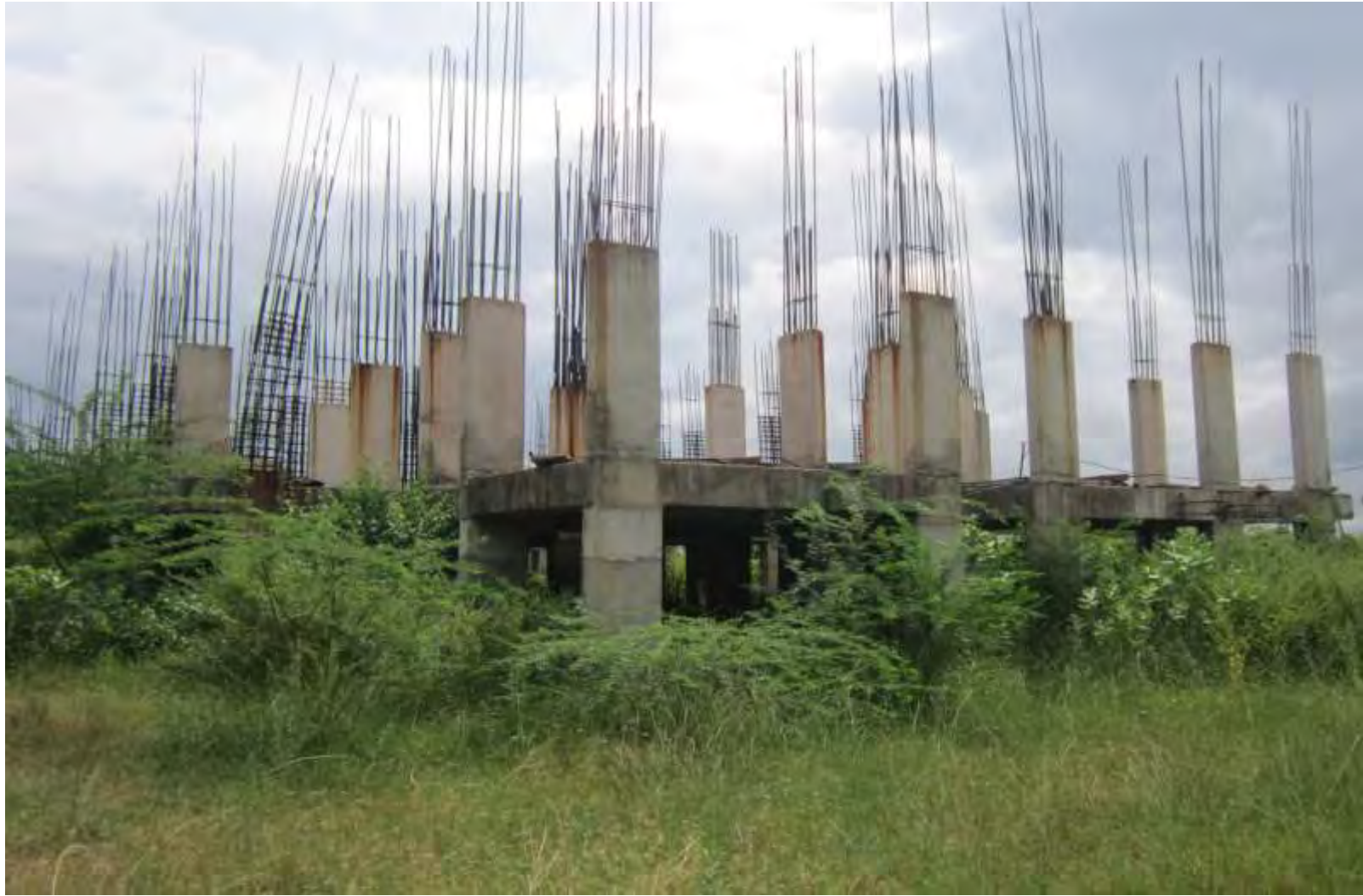
Block C – 1 st floor slab concrete pour 1 and pour 2 completed and 1 st floor slab Shuttering work
