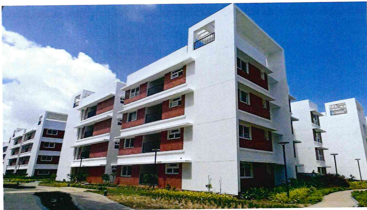
TOWER-6 South East view
