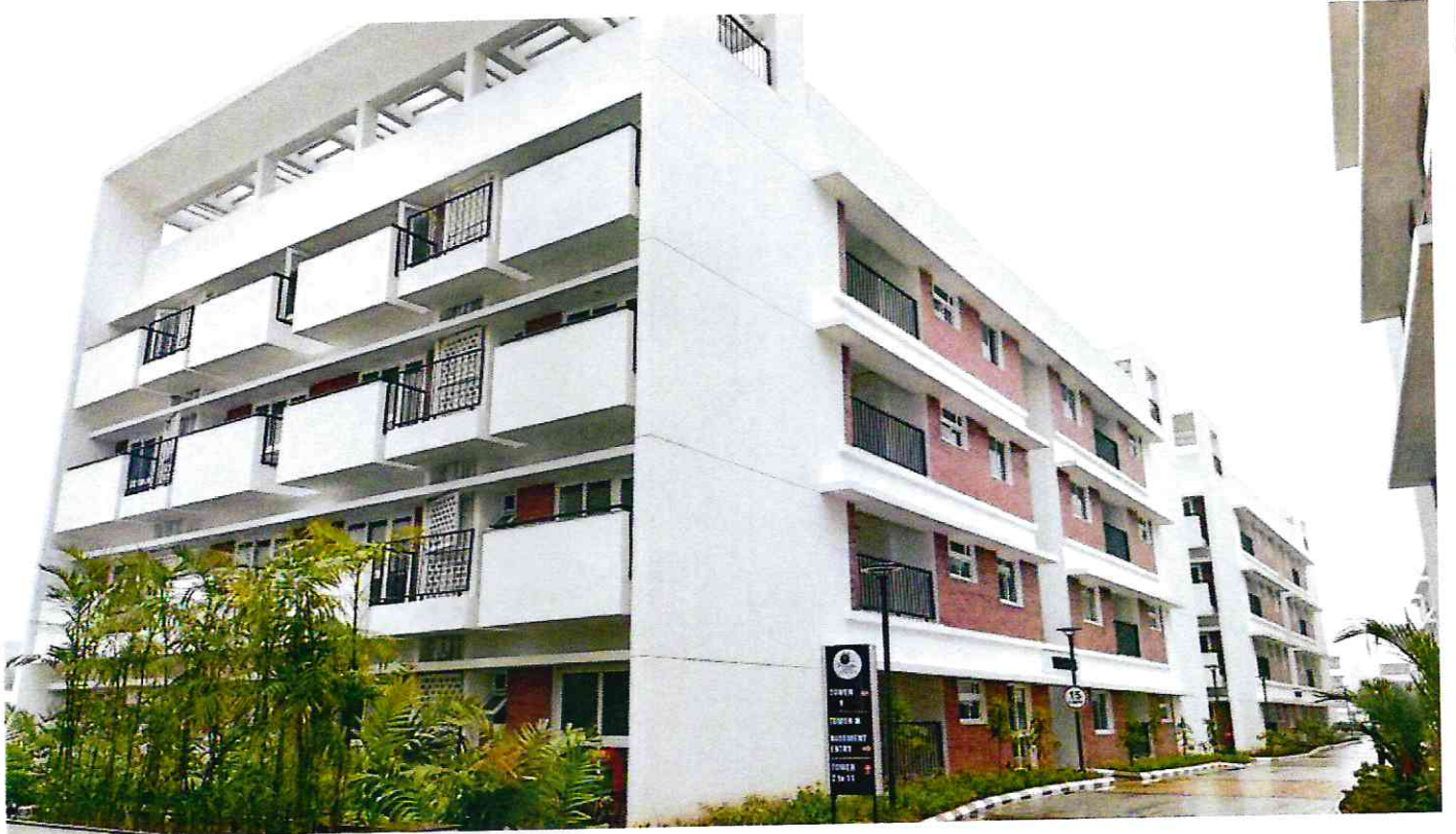
TOWER-1 South West view
