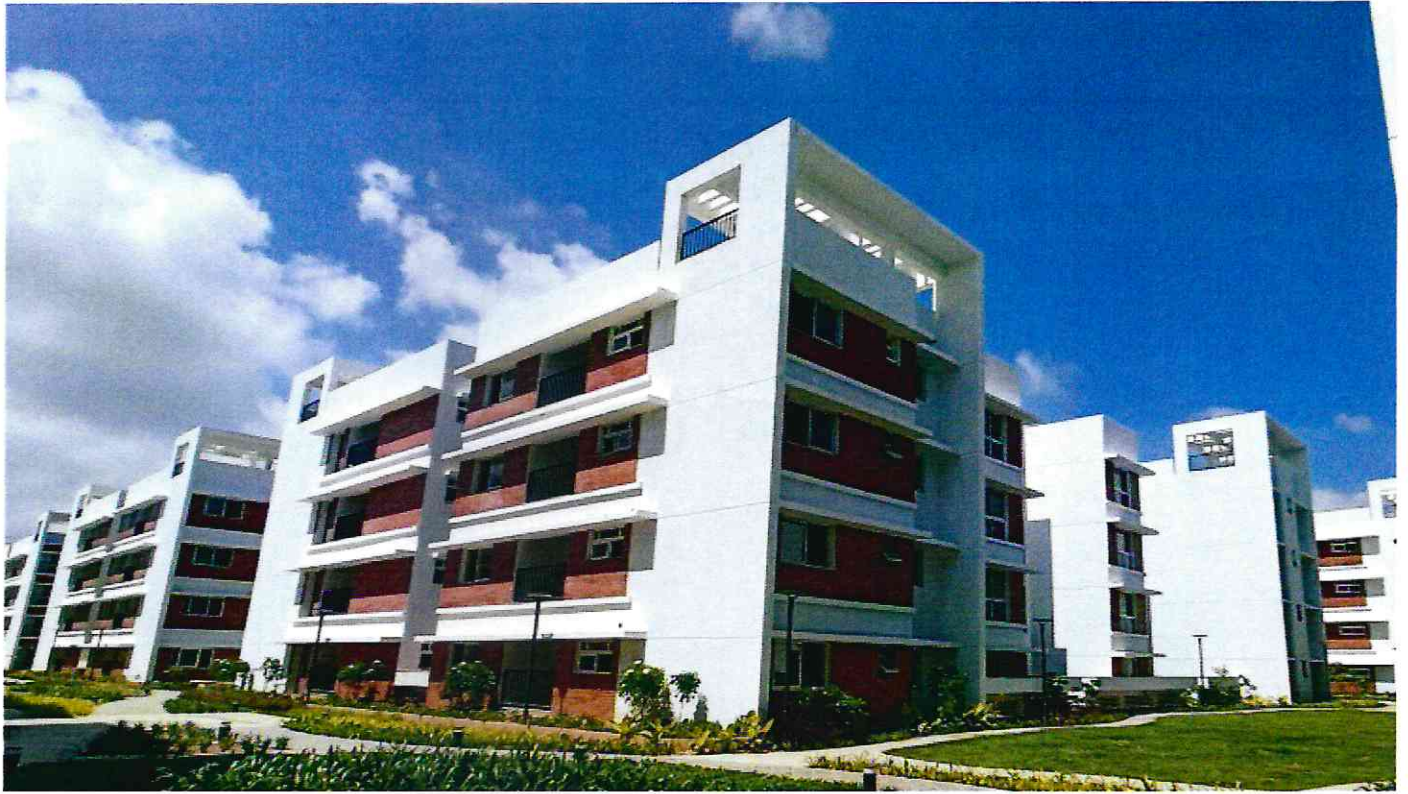
TOWER-7 South East view
