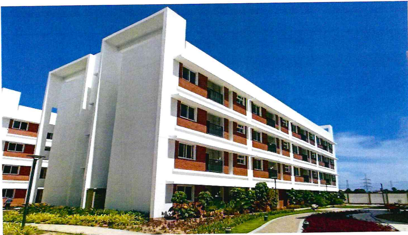
TOWER-5 South East view
