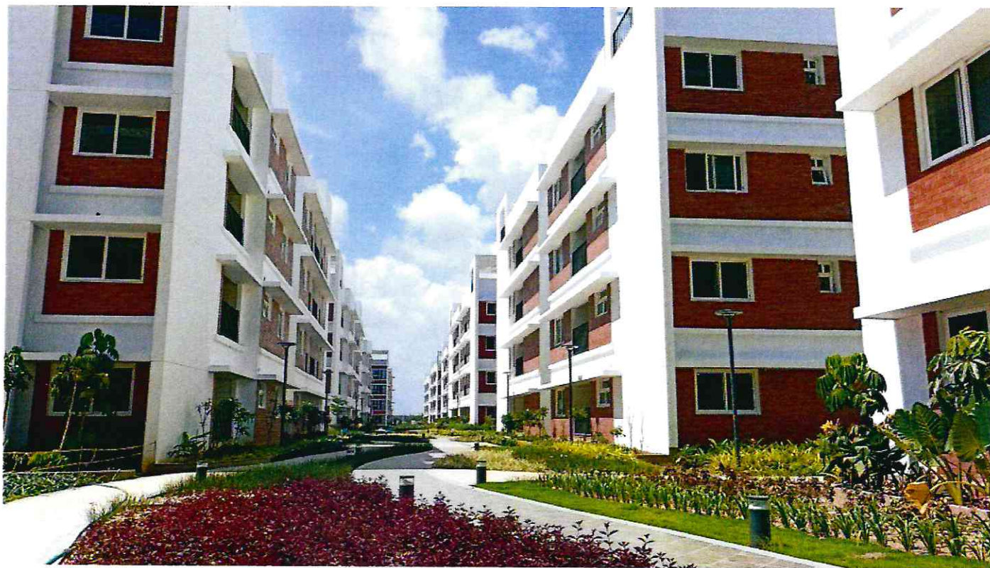
Celebrity walkway between T11 & T5 (East to West)
