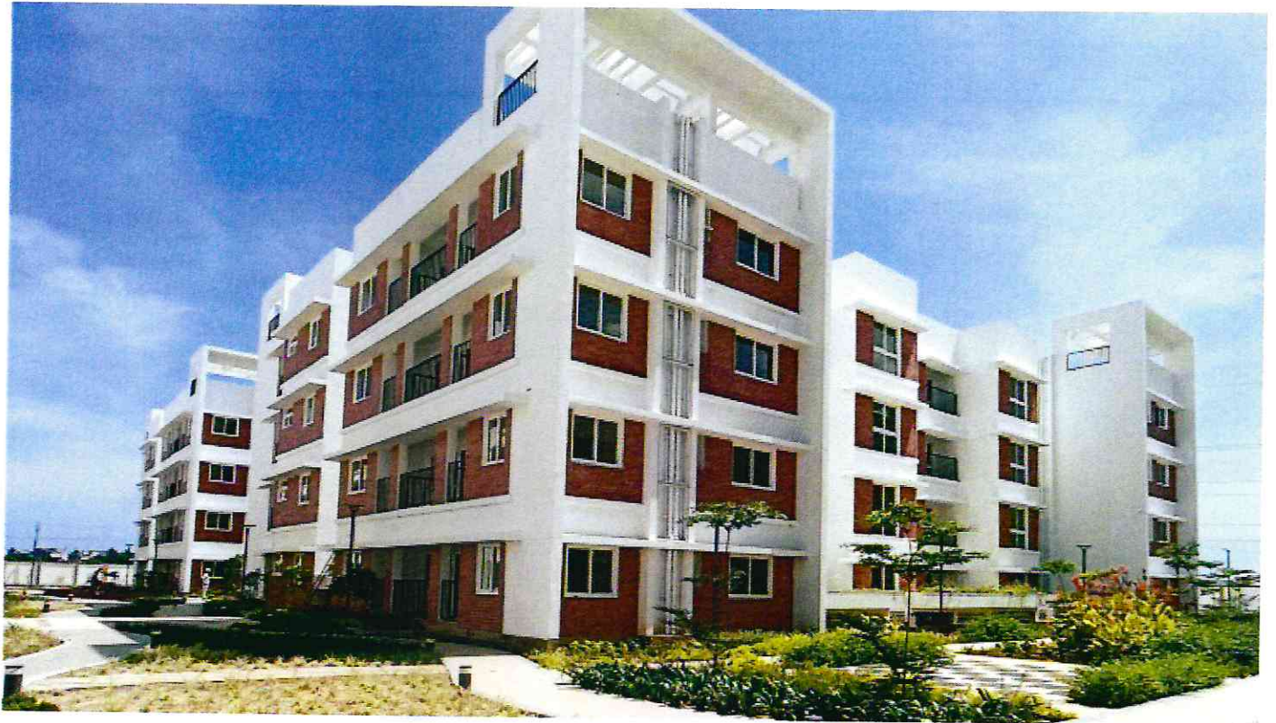
TOWER-11 North West view
