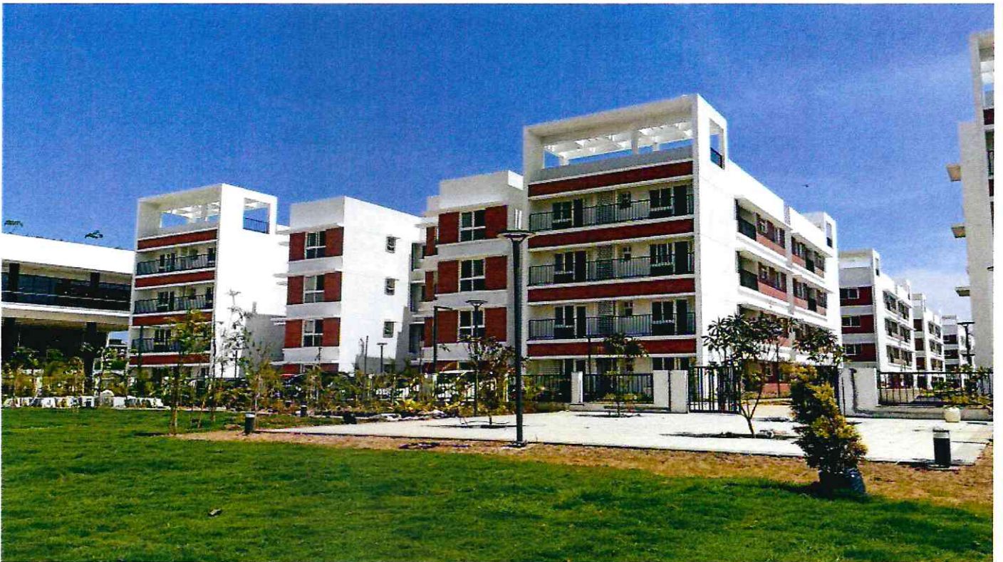
TOWER-8 South West view
