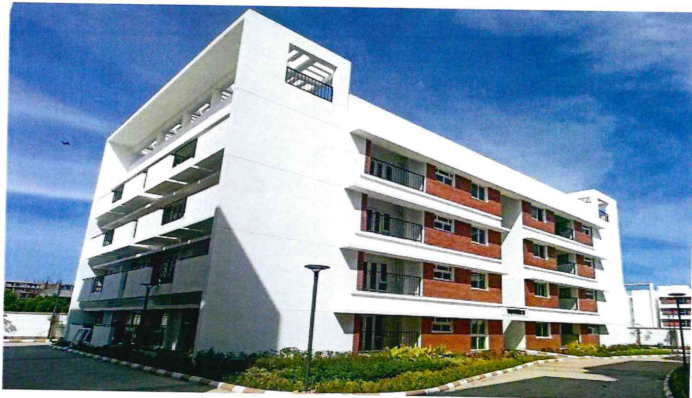
TOWER-3 South West view
