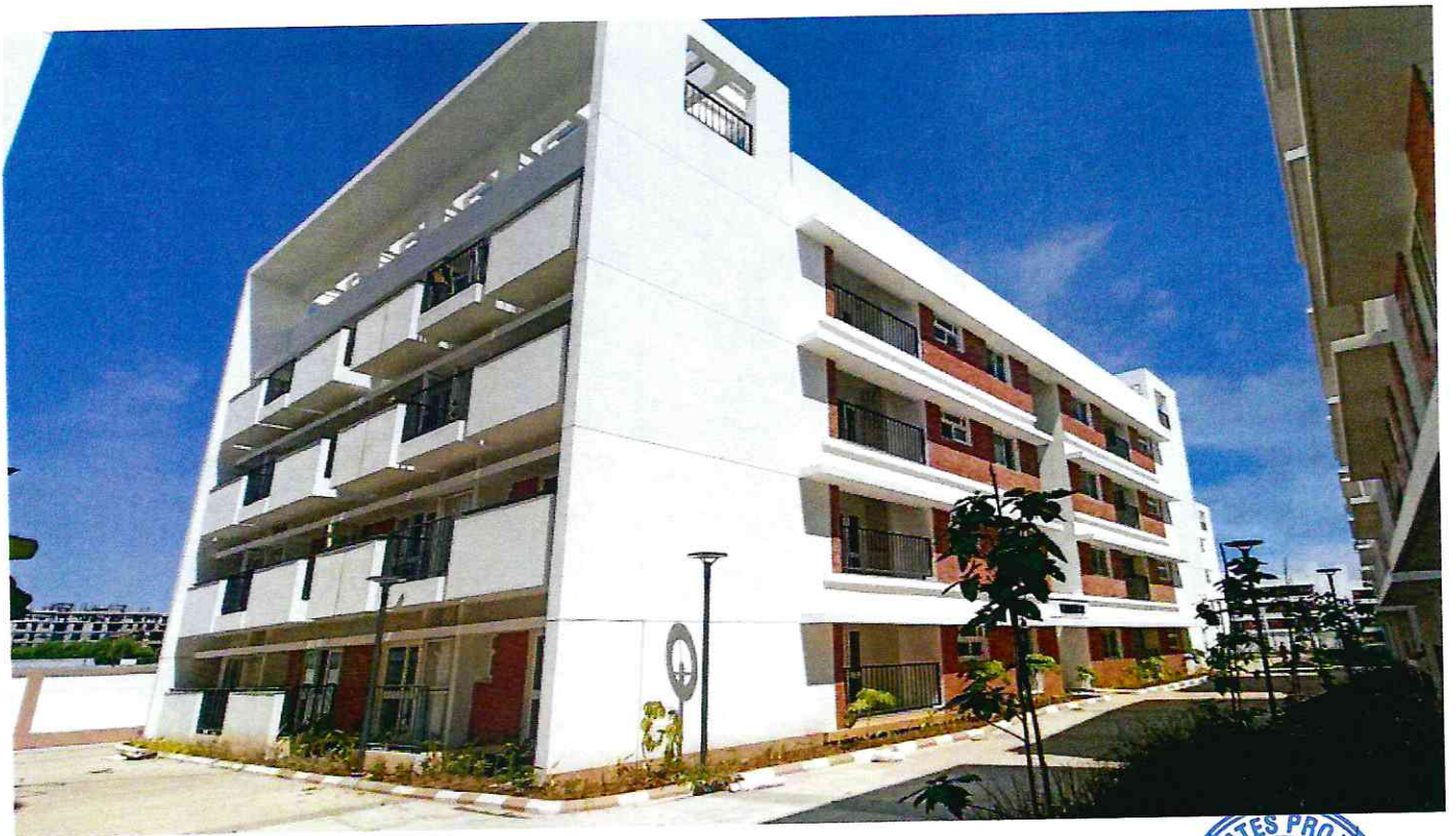
TOWER-2 South West view
