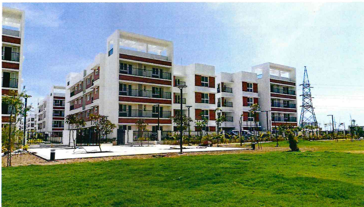
TOWER-9 North West view
