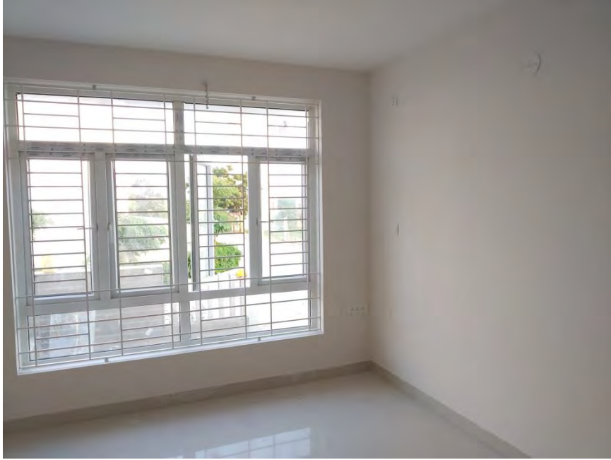
Flooring and painting Completed
