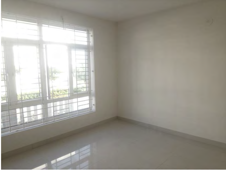
Flooring and painting Completed
