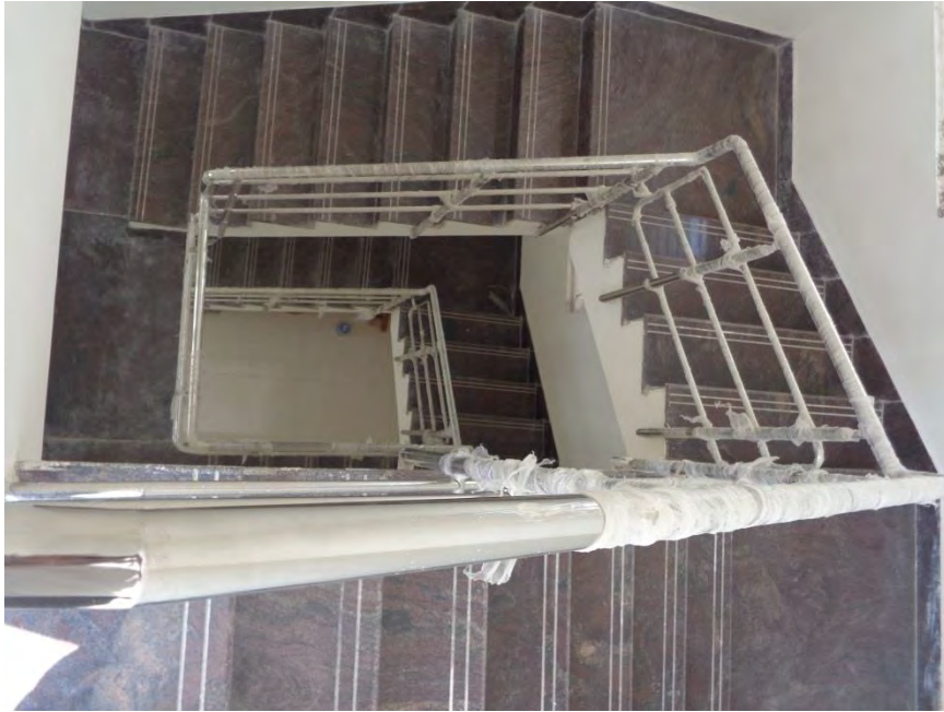
Flooring and painting Completed
