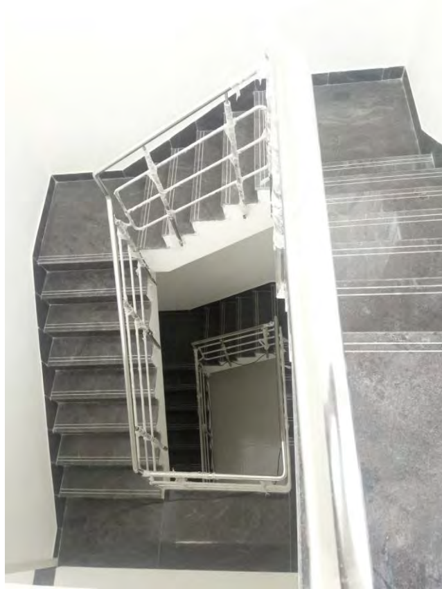
Flooring and painting Completed
