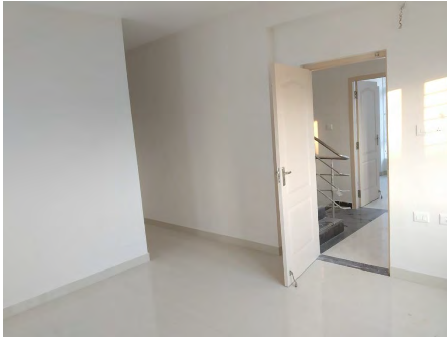
Flooring and painting Completed
