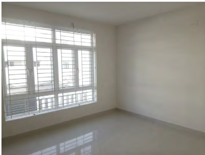
Flooring and painting Completed
