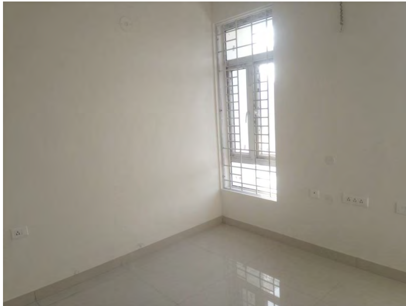
Flooring and painting Completed
