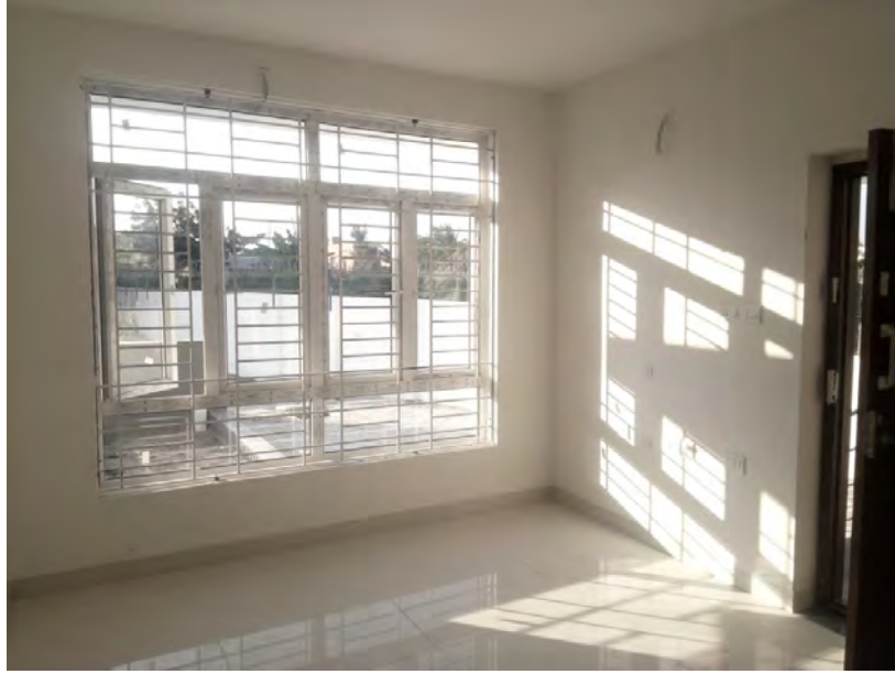
Flooring and painting Completed
