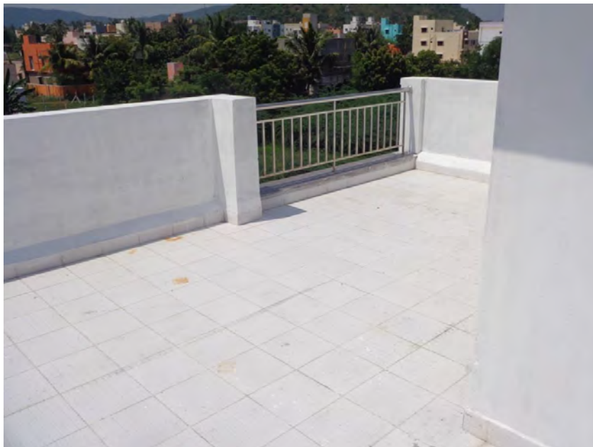
Flooring and painting Completed
