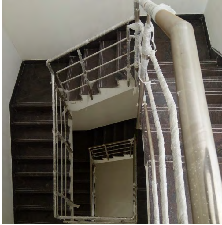
Flooring and painting Completed
