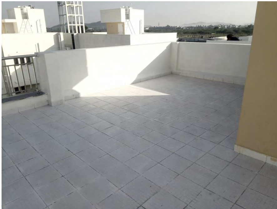
Flooring and painting Completed
