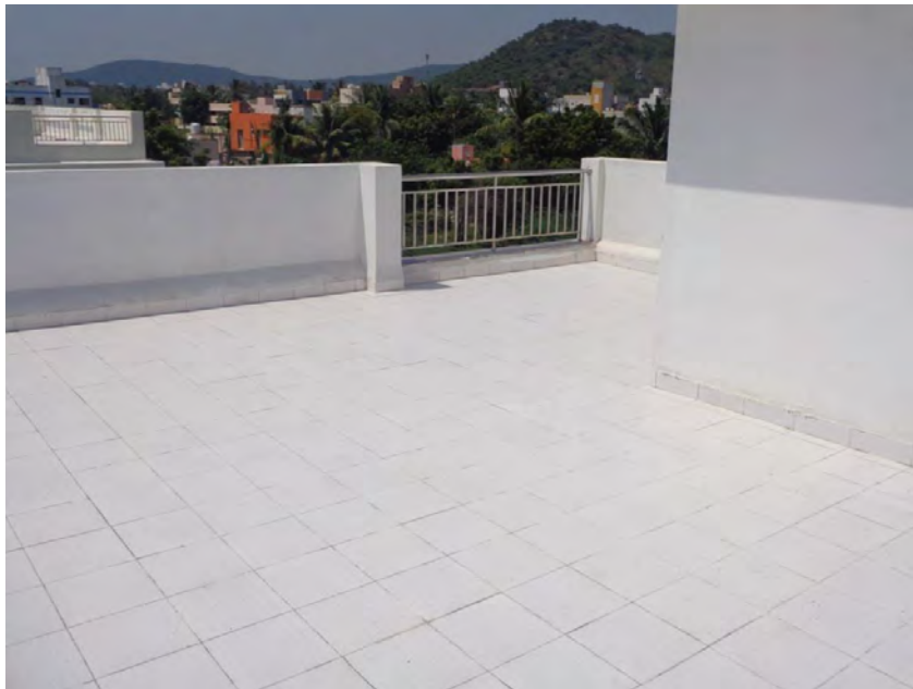
Flooring and painting Completed
