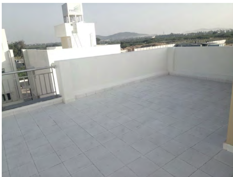
Flooring and painting Completed
