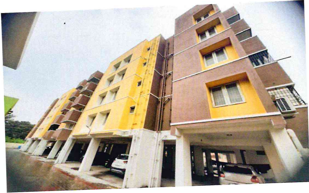
Back view - West side
