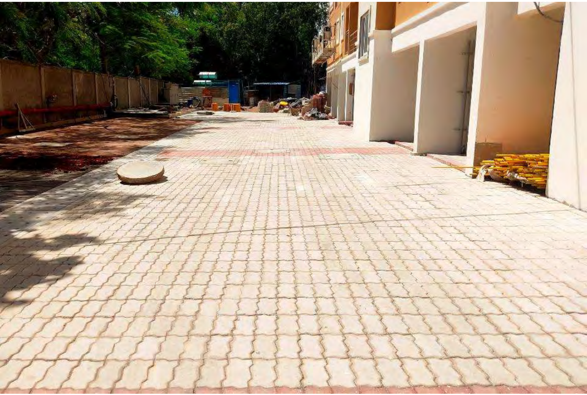
External Driveway Block D : Zig-Zag Paver completed & Grass Paver in Progress. Photo 1 of 2.
