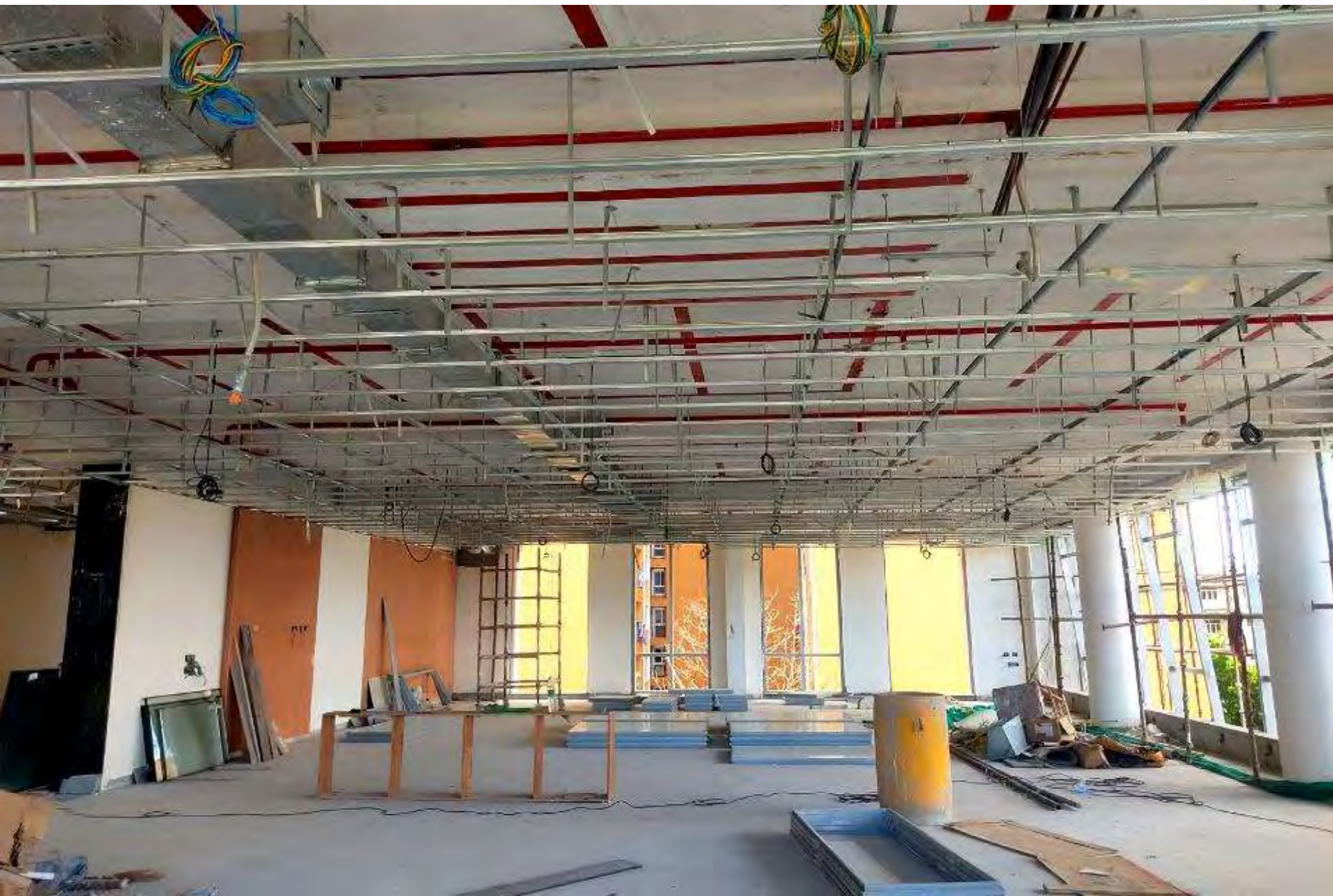
Clubhouse : Interior work in progress. Photo 2 of 2.
