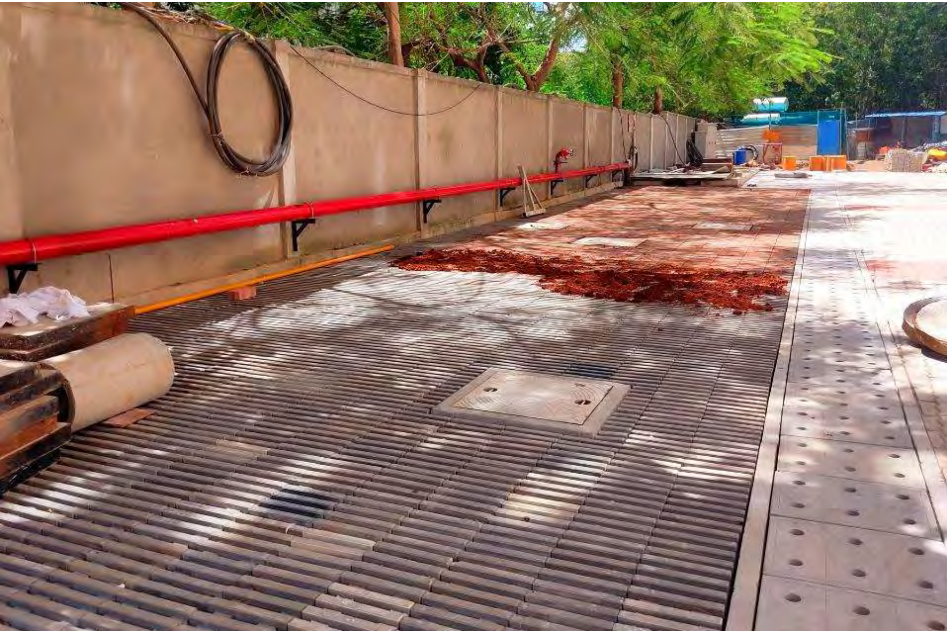
External Driveway Block D : Zig-Zag Paver completed & Grass Paver in Progress. Photo 2 of 2.
