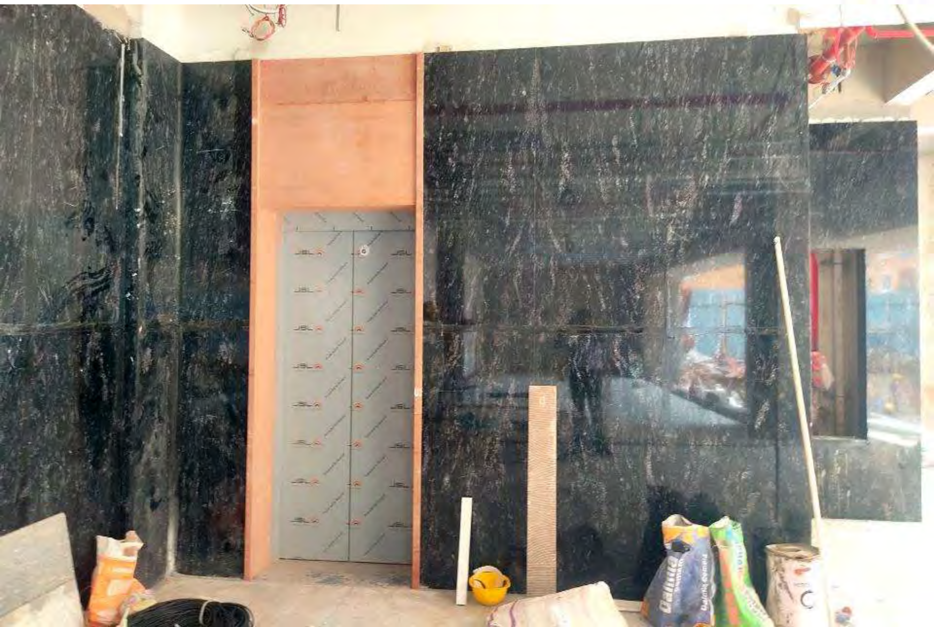
Clubhouse : Wall cladding work is completed.
