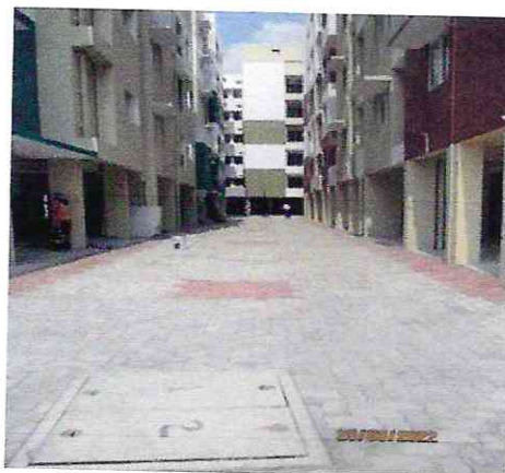
Paver Road work is completed COMPLETED
