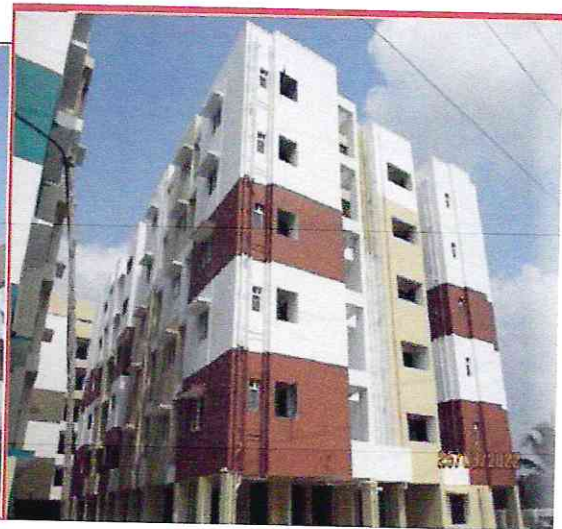
External Painting Work Completed – B
