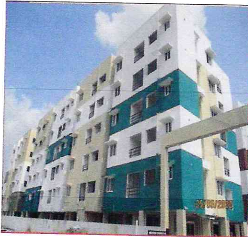
External Painting Work Completed – C Block Block
