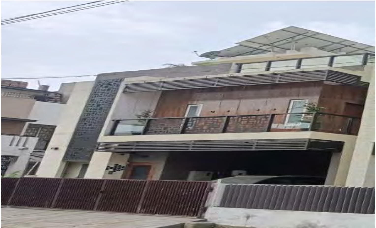
Villa 122 – 100% work completed
