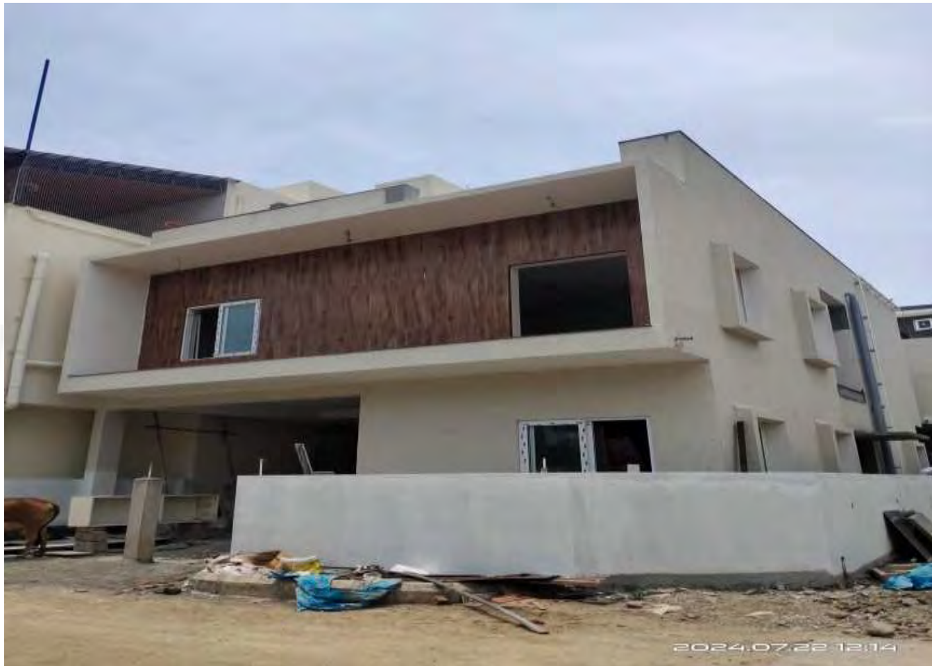
Villa 103 – 95% completed. Elevation in Progress
