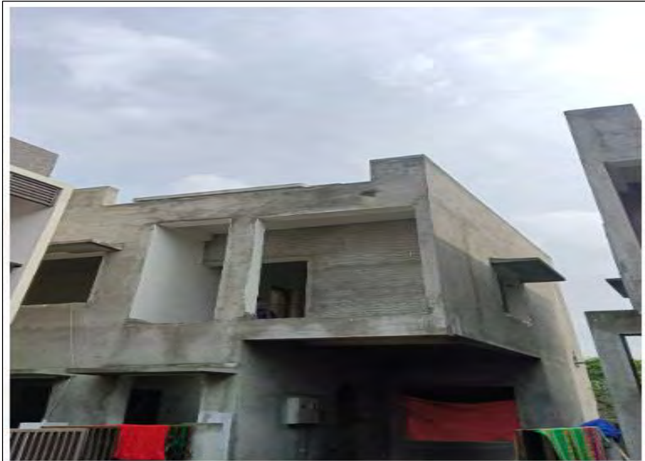
Villa 45 – Tiling & painting in progress
