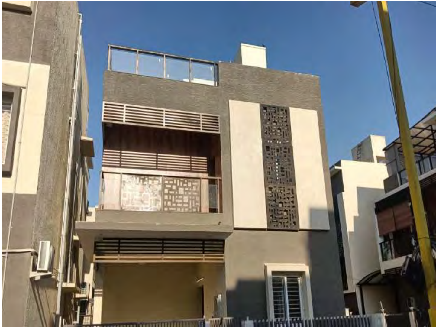
Villa 93 – 100% work completed
