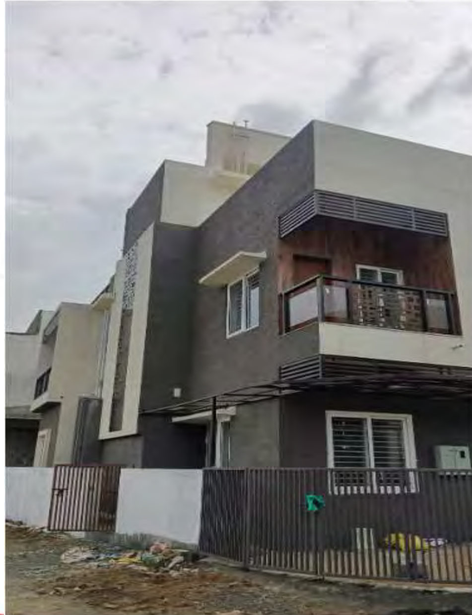
Villa 111 – 100% work completed
