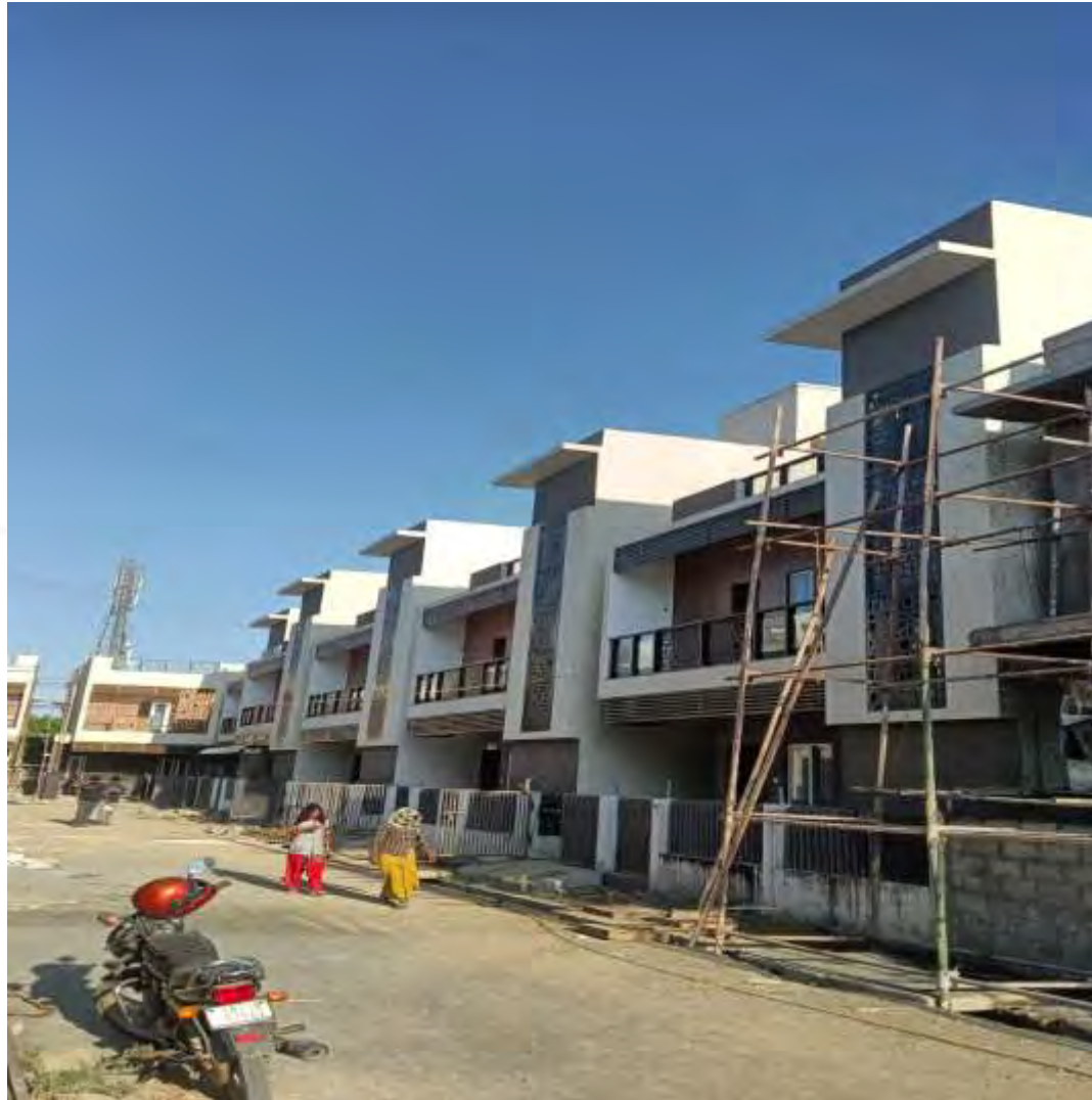
Villa 44 – 100% work completed
