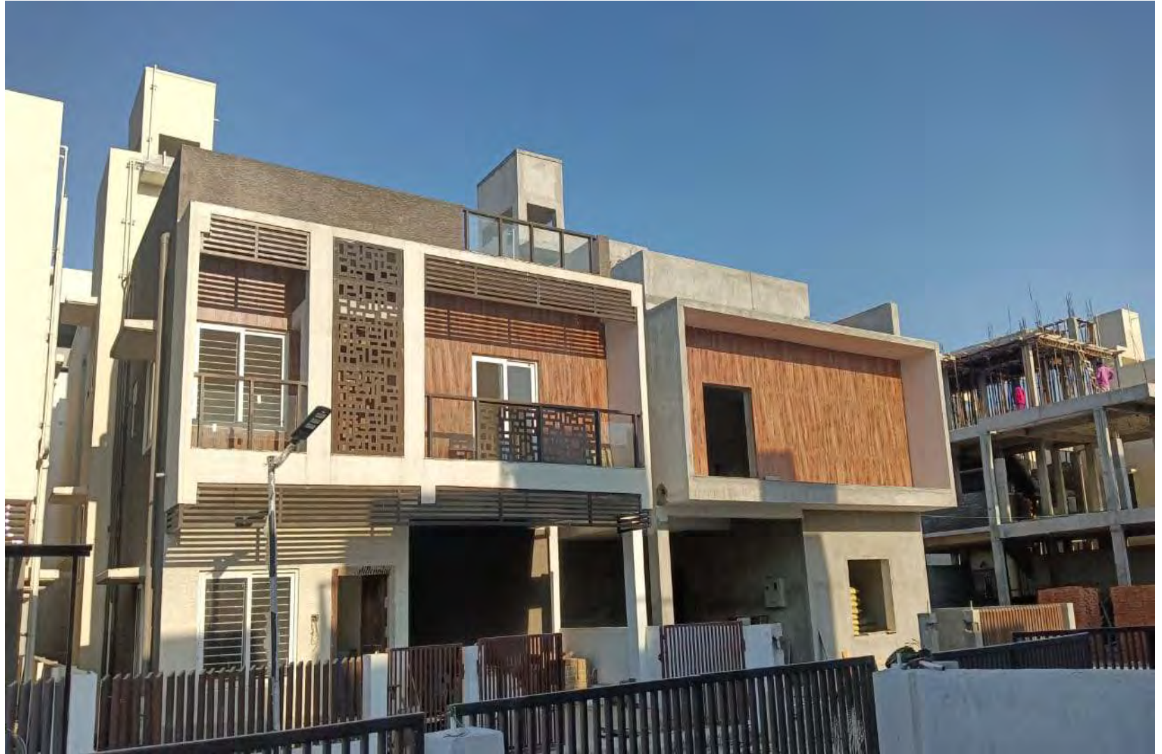
Villa 109 – Internal Plumbing works completed V-110 -100% Completed
