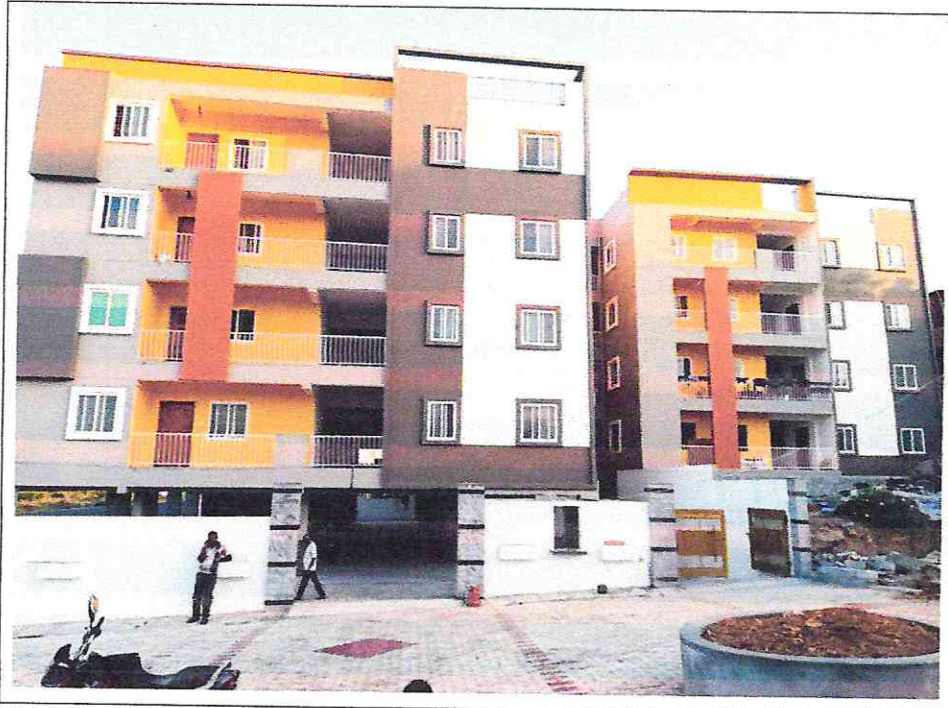
View from North
