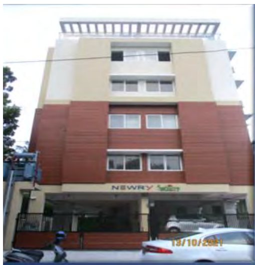
External Finishing work is completed
