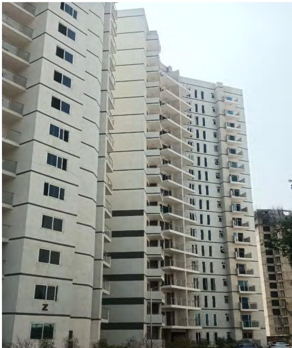
Y tower – Civil & MEP finishes under progress
