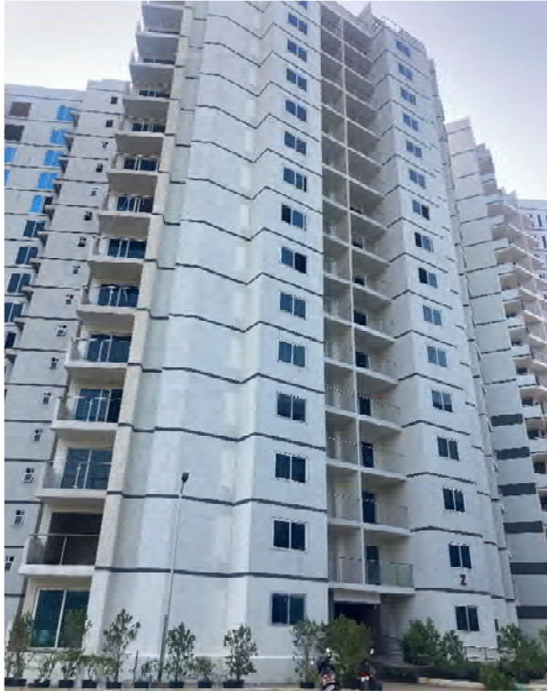
Z tower – Civil & MEP finishes under progress
