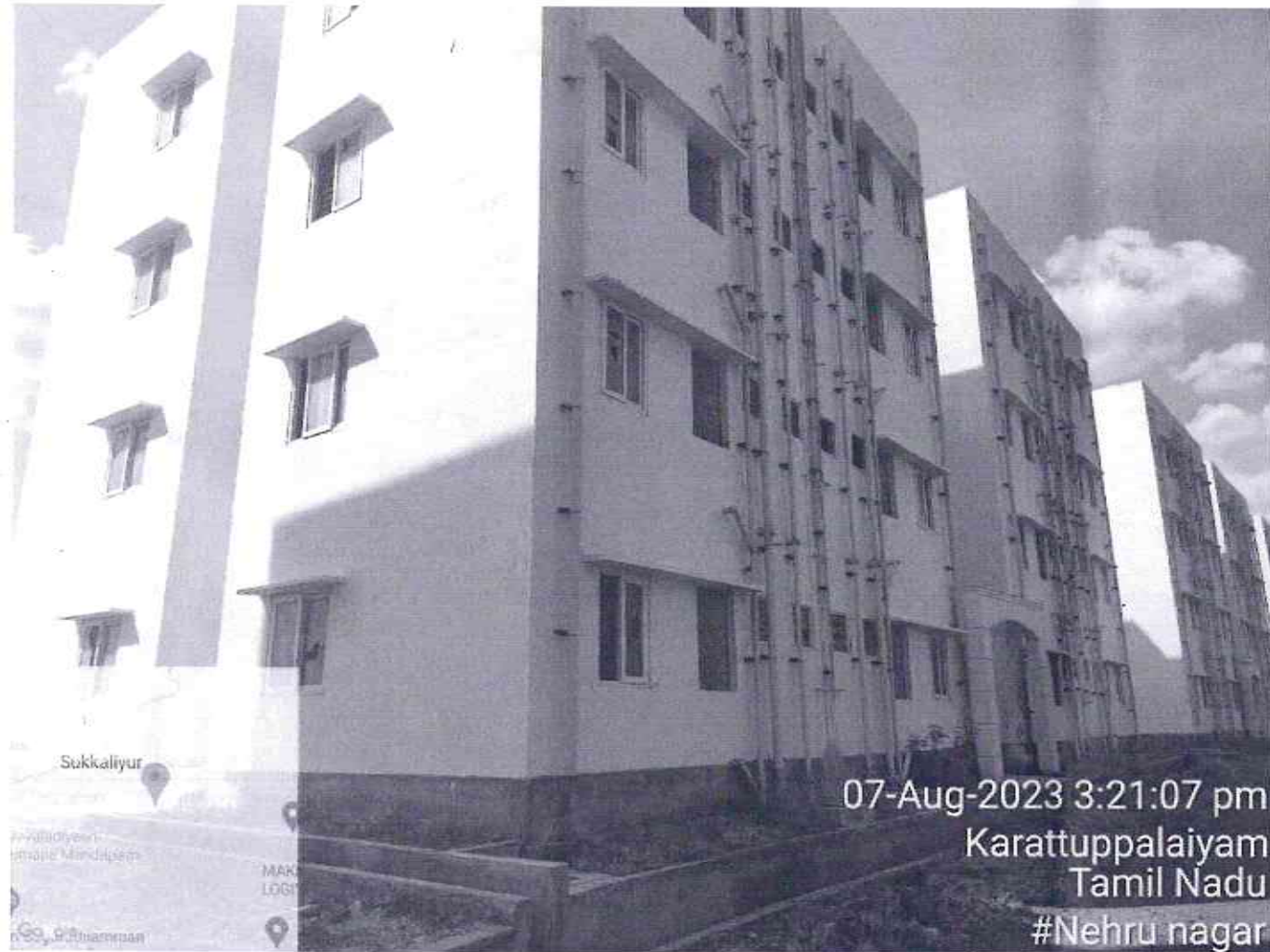
Rear View of Block 9
