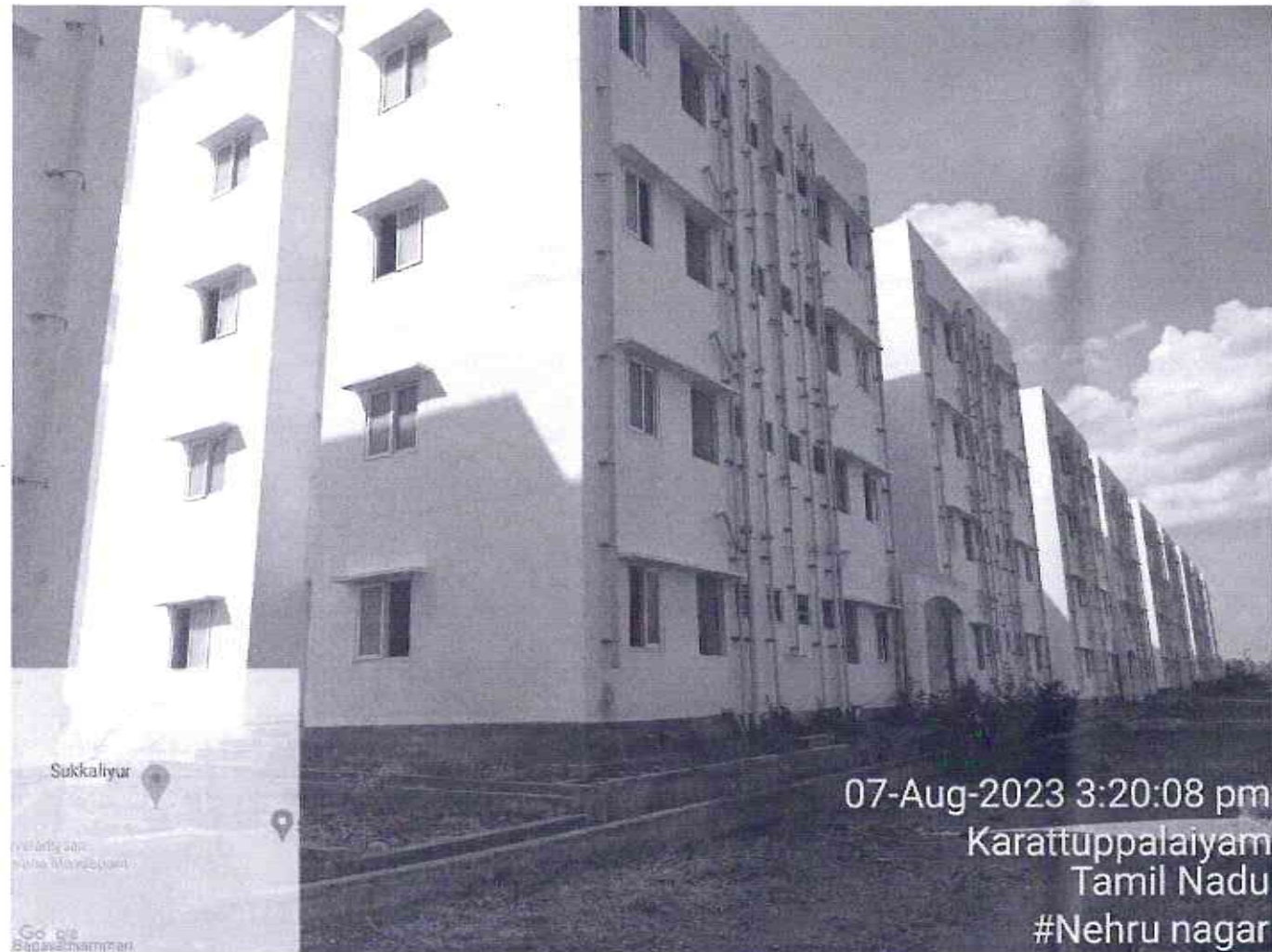
Rear View of Block 7
