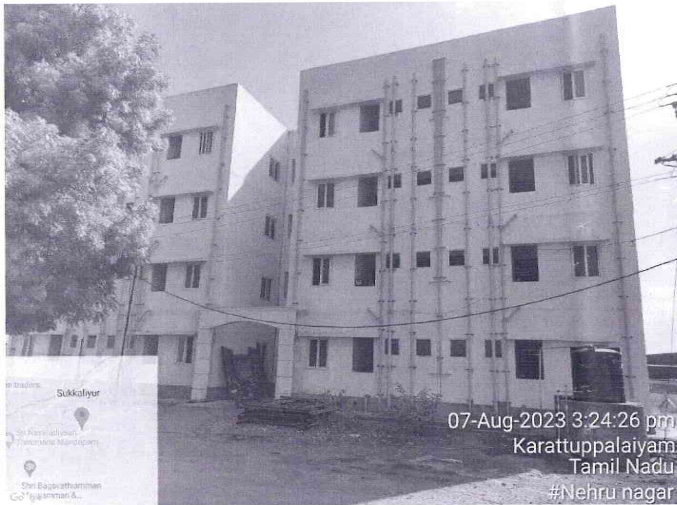
Rear View of Block 14
