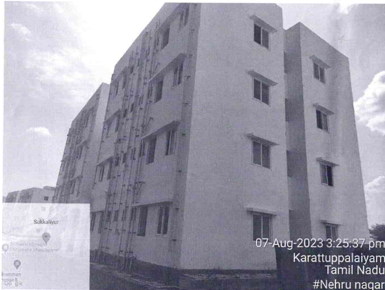
Rear View of Block 15
