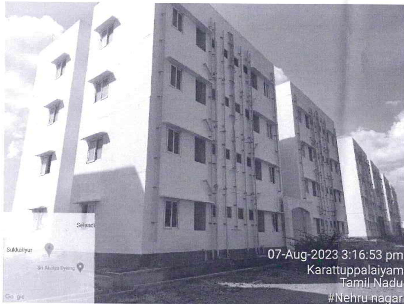
Rear View of Block 3
