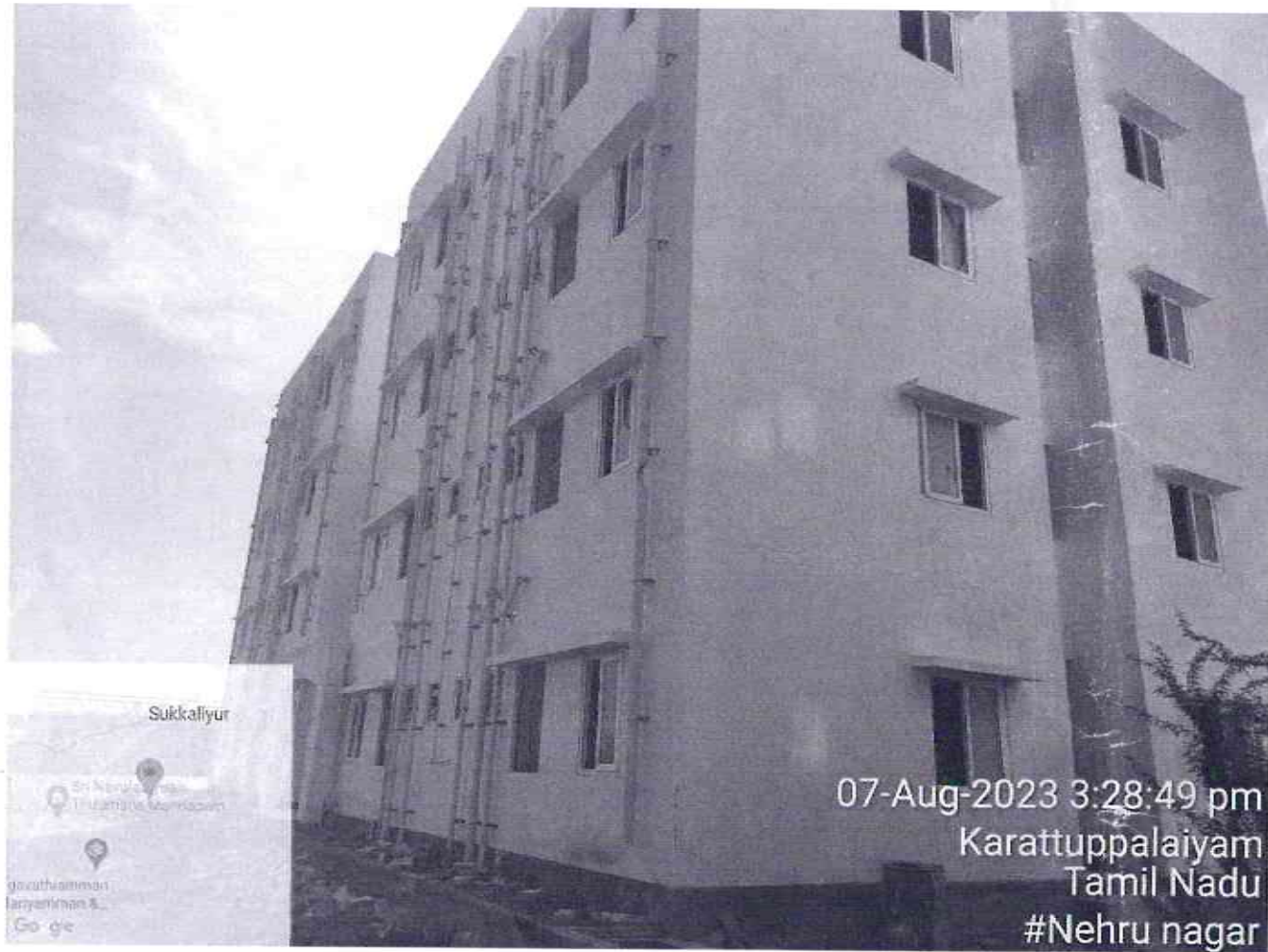
Rear View of Block 20
