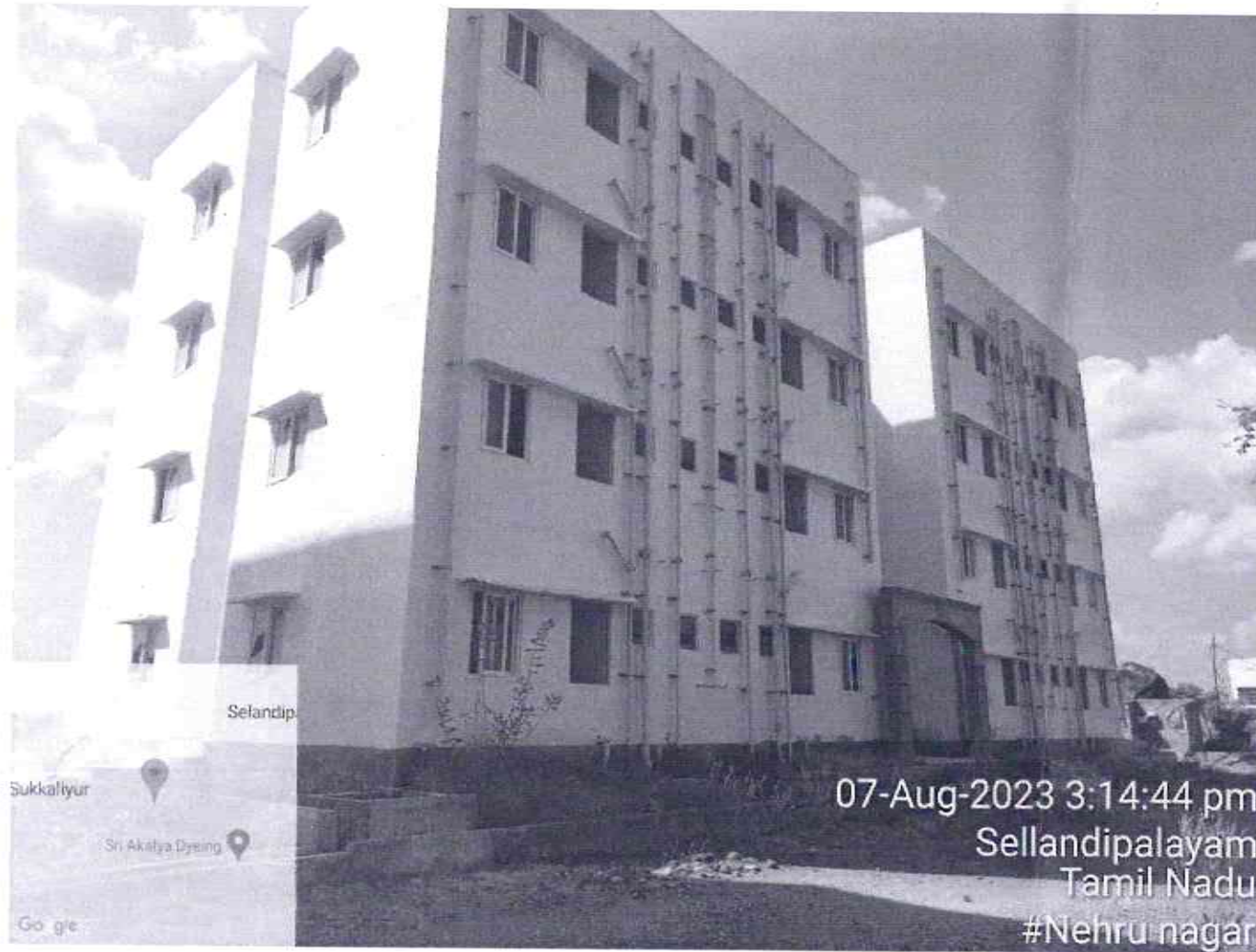
Rear View of Block 1
