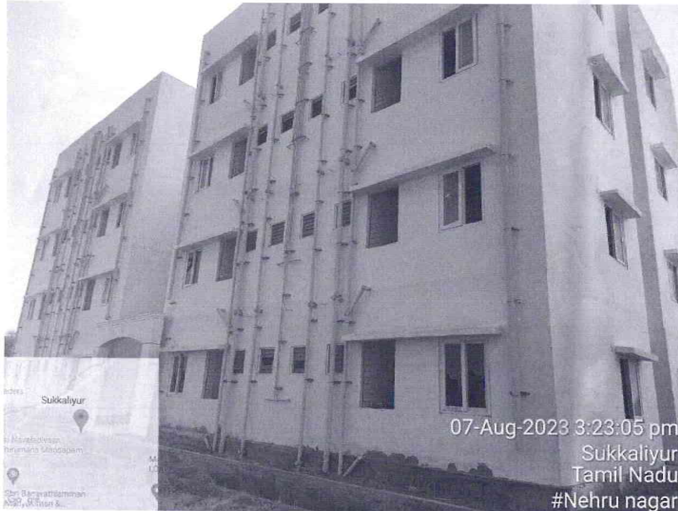
Rear View of Block 13
