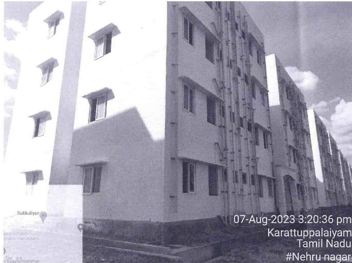
Rear View of Block 8
