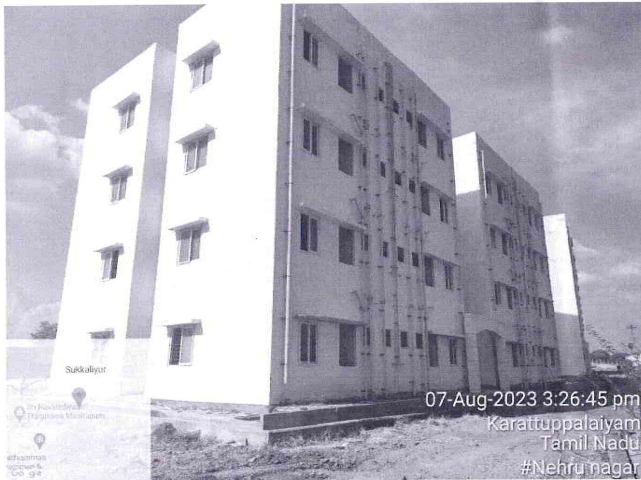
Rear View of Block 16
