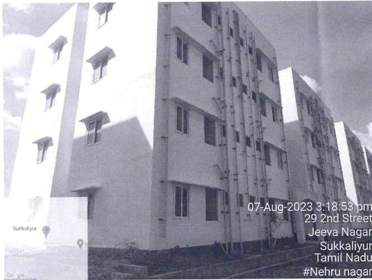
Rear View of Block 4
