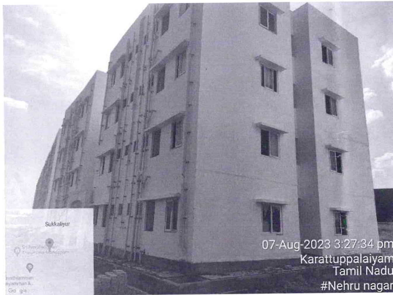
Rear View of Block 18
