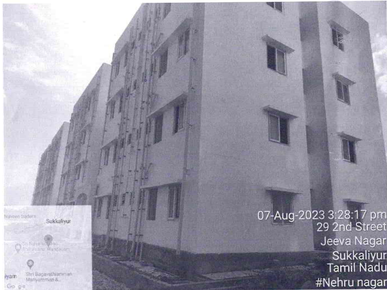
Rear View of Block 19
