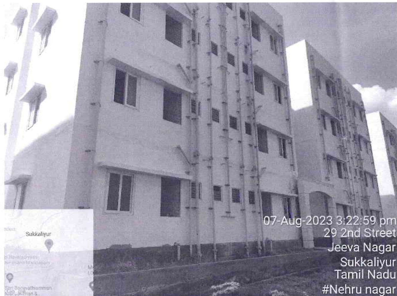
Rear View of Block 12
