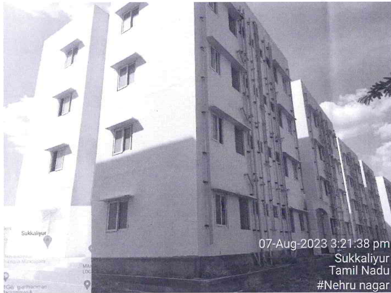
Rear View of Block 10
