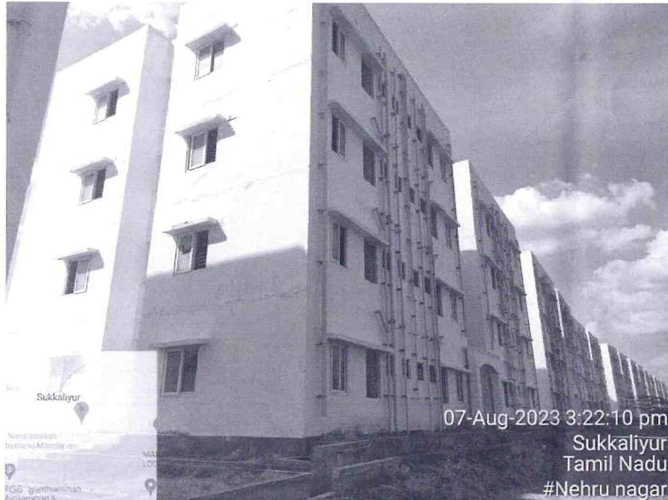
Rear View of Block 11
