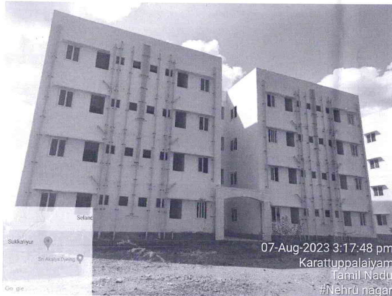
Rear View of Block 5
