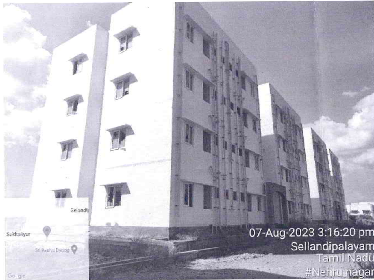
Rear View of Block 2
