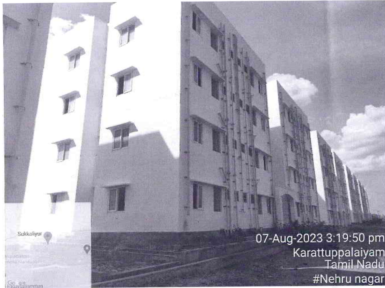
Rear View of Block 6
