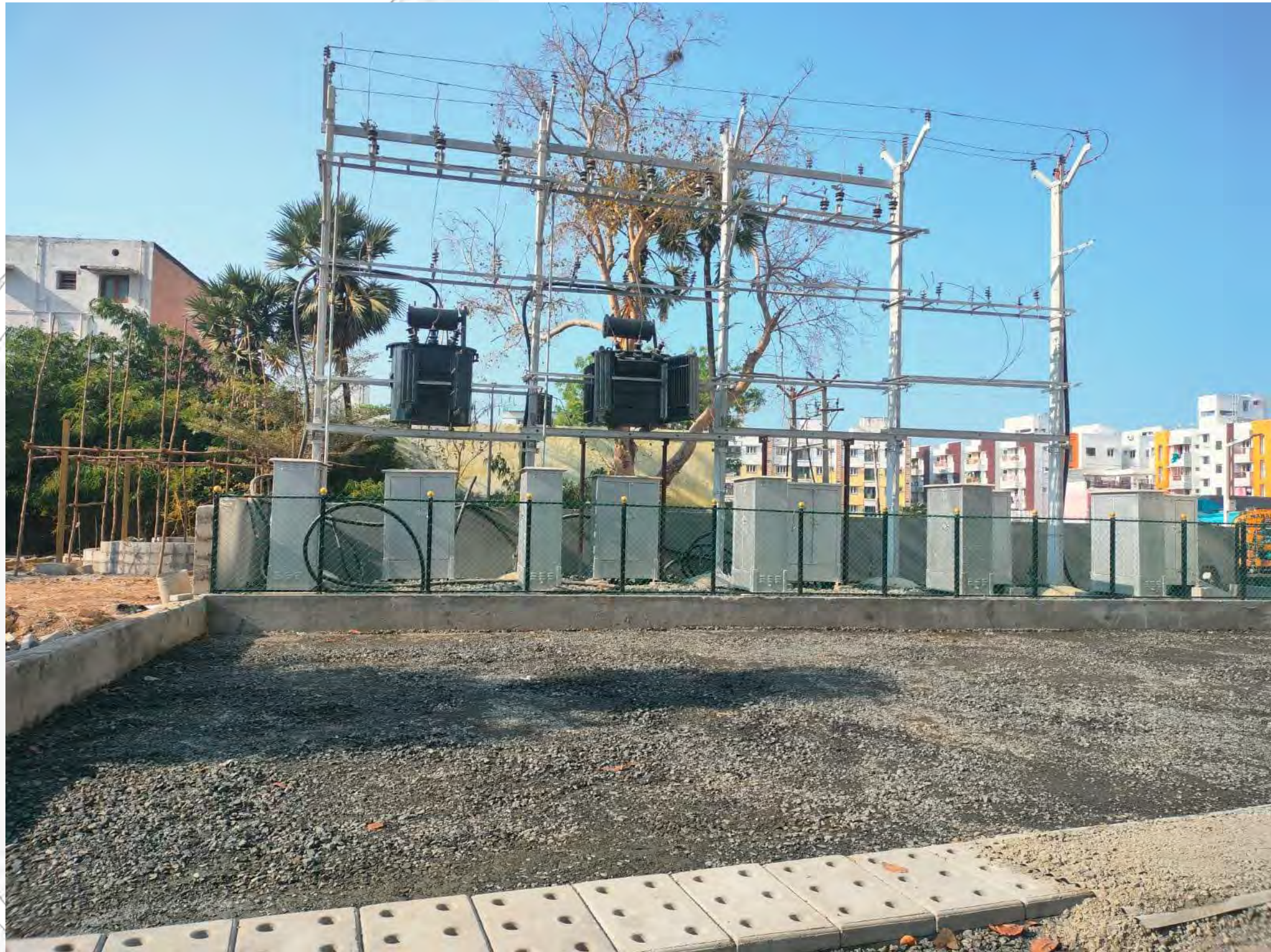
Transformer Yard Work Completed
