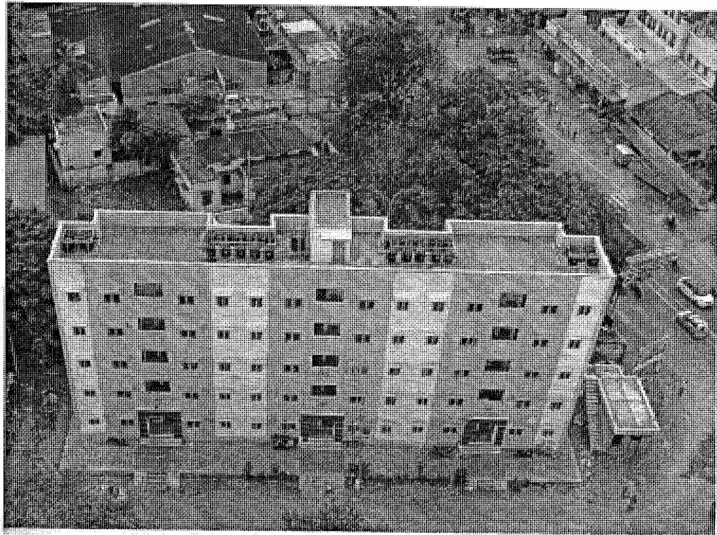
CONSTRUCTION OF 100 TENEMENTS AT KALLAMEDU IN COIMBATORE
