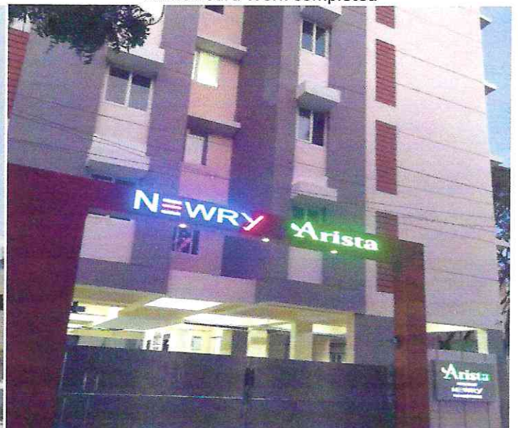
Entrance - Shera Plank Name Board Work Completed
