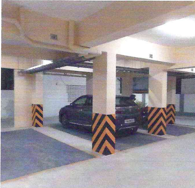
Car Park Marking Completed
