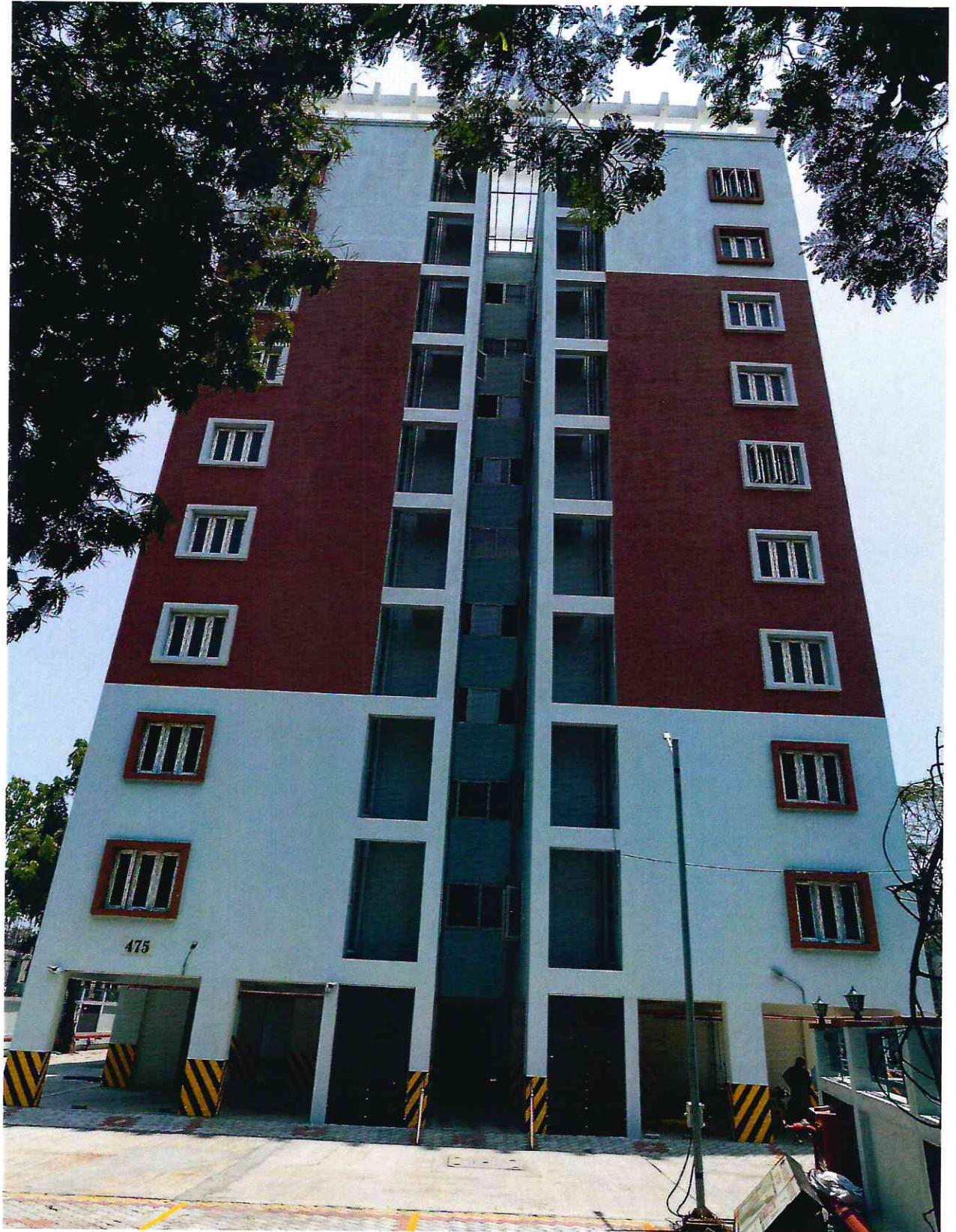
Construction of Stilt Floor + 9 Floors with 108 dwelling units, abutting Cemetery Road and East Club Road, Shenoy Nagar, Chennai.
