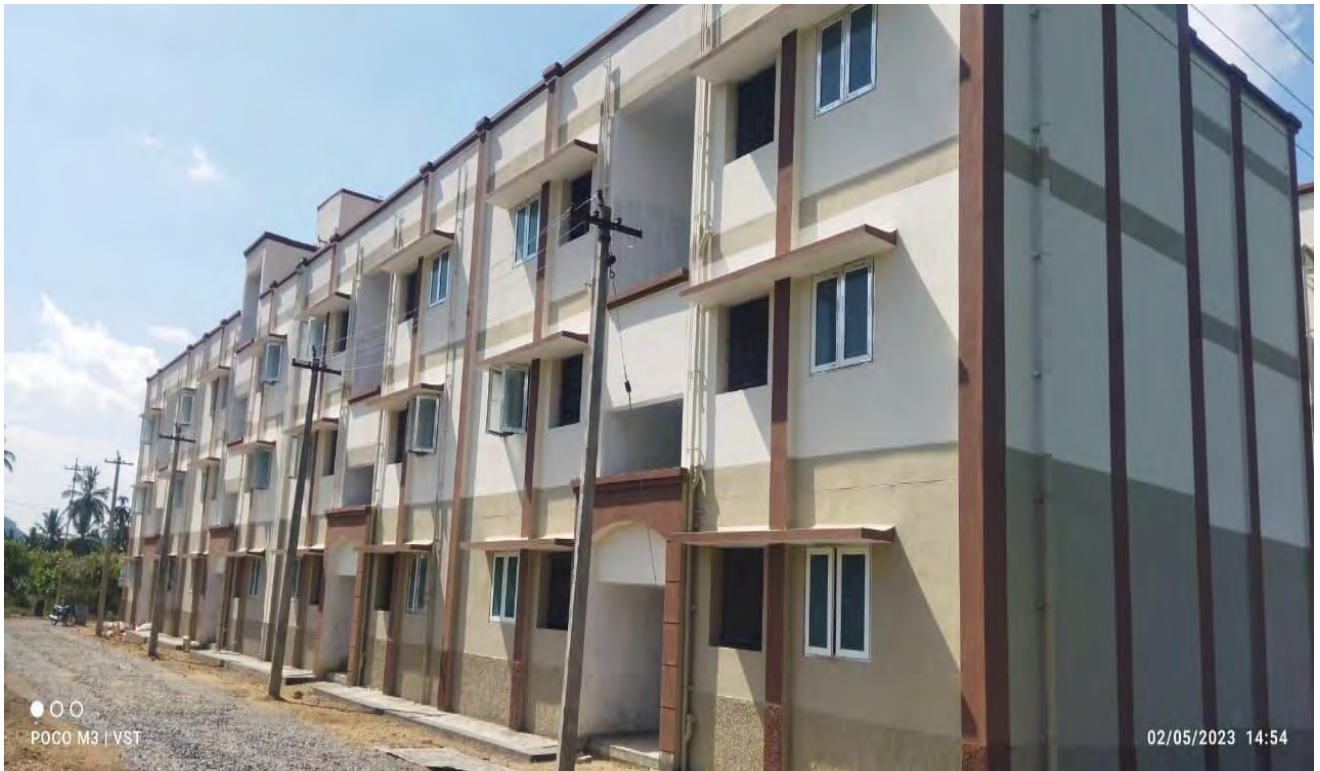
Construction of 192 tenements at Molayanur in Pappireddipatty town
