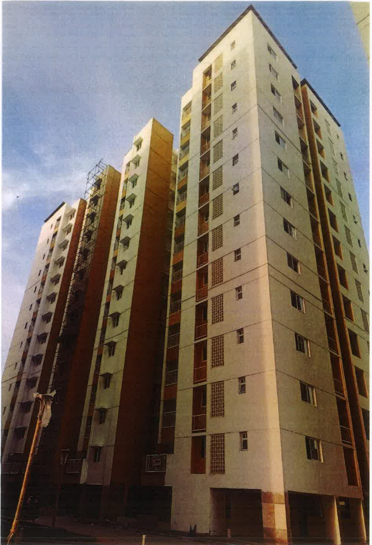
External Painting Works in Progress
