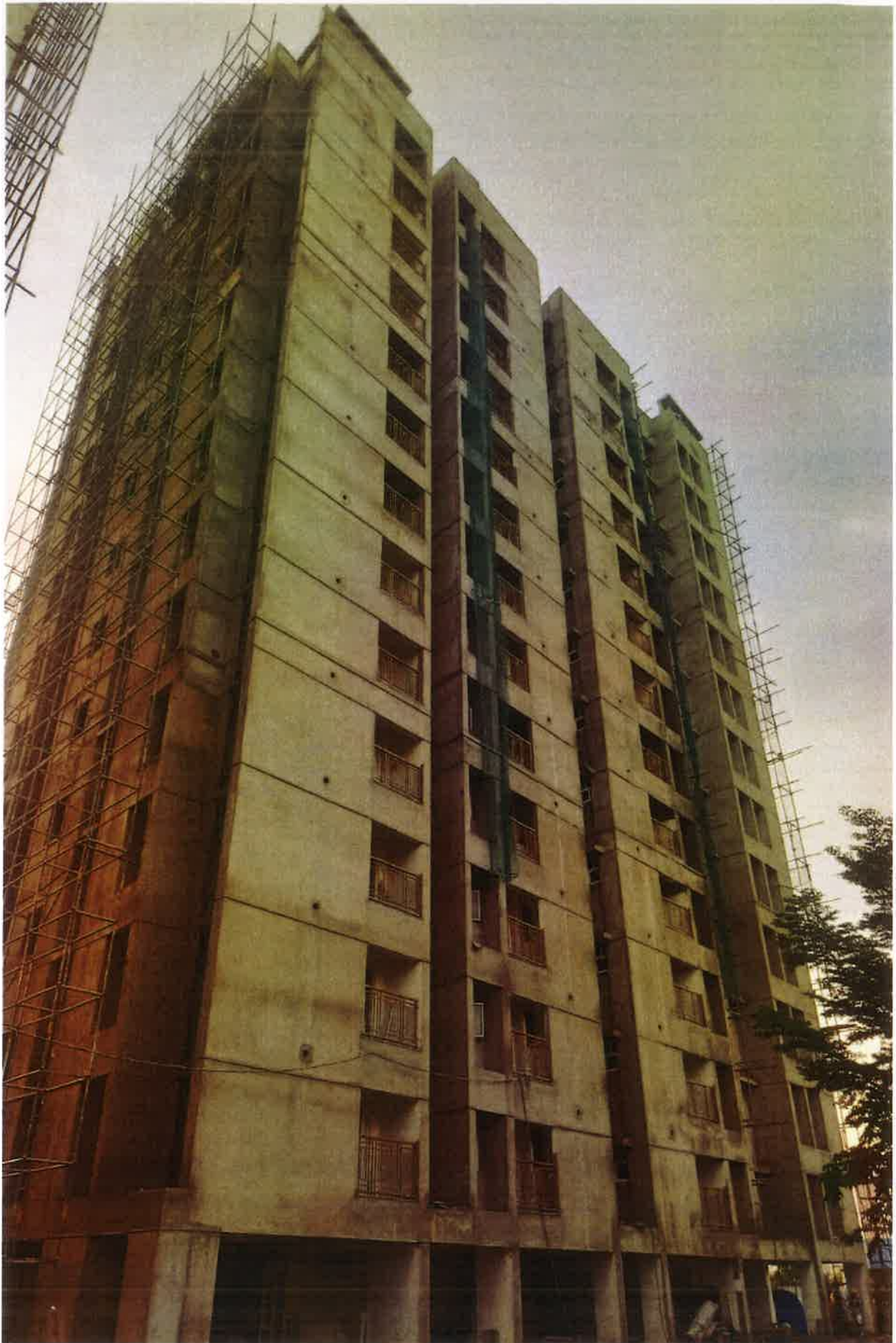
External Plastering Works in Progress
