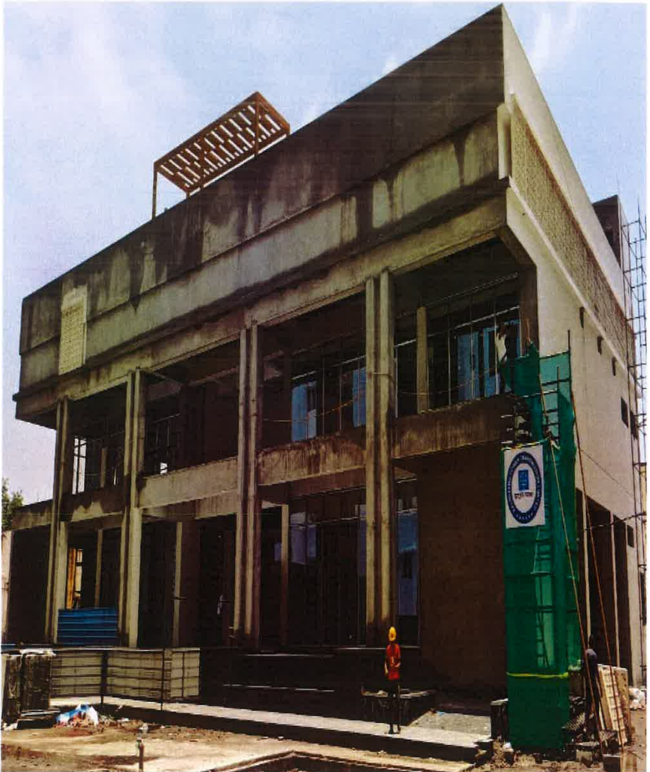
External Painting Works in Progress
