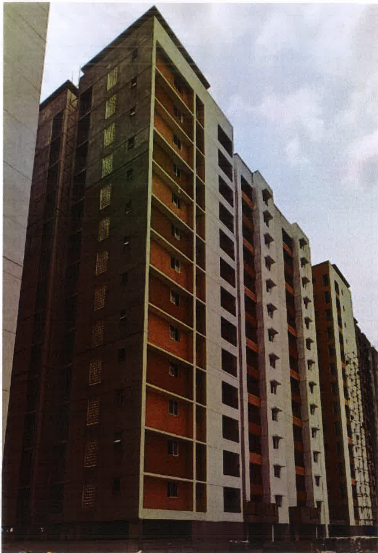
External Painting work in progress
