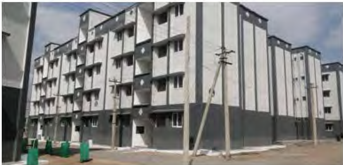
Physical Progress - Block B – Elevation View
