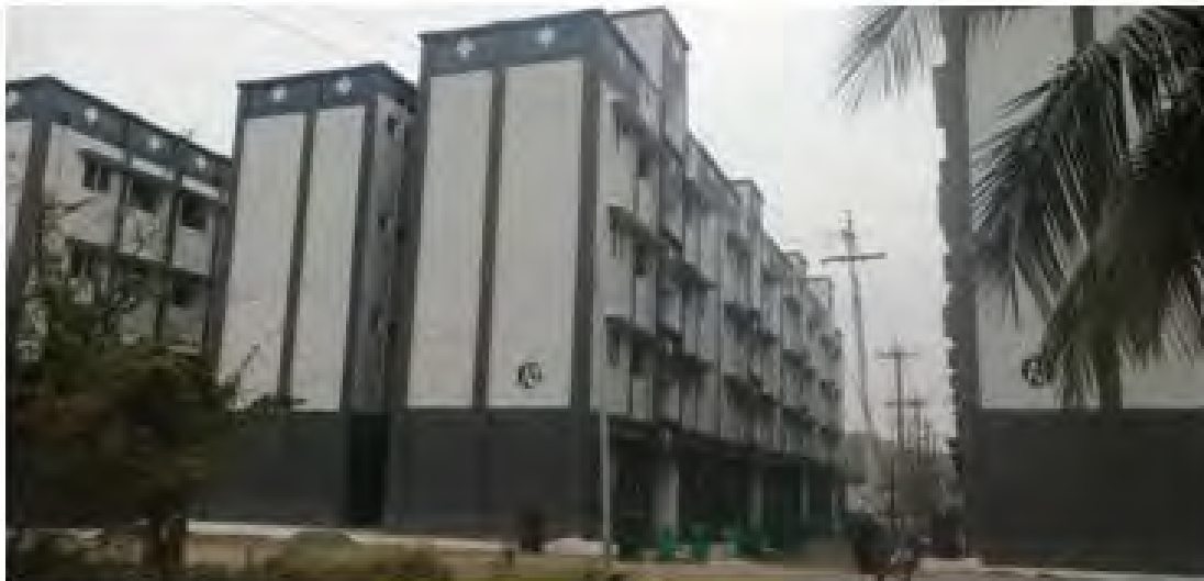
Physical Progress - Block A2 – Elevation View
