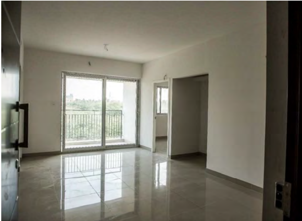
Block – C: Sixth Floor Internal Painting Work in Progress
