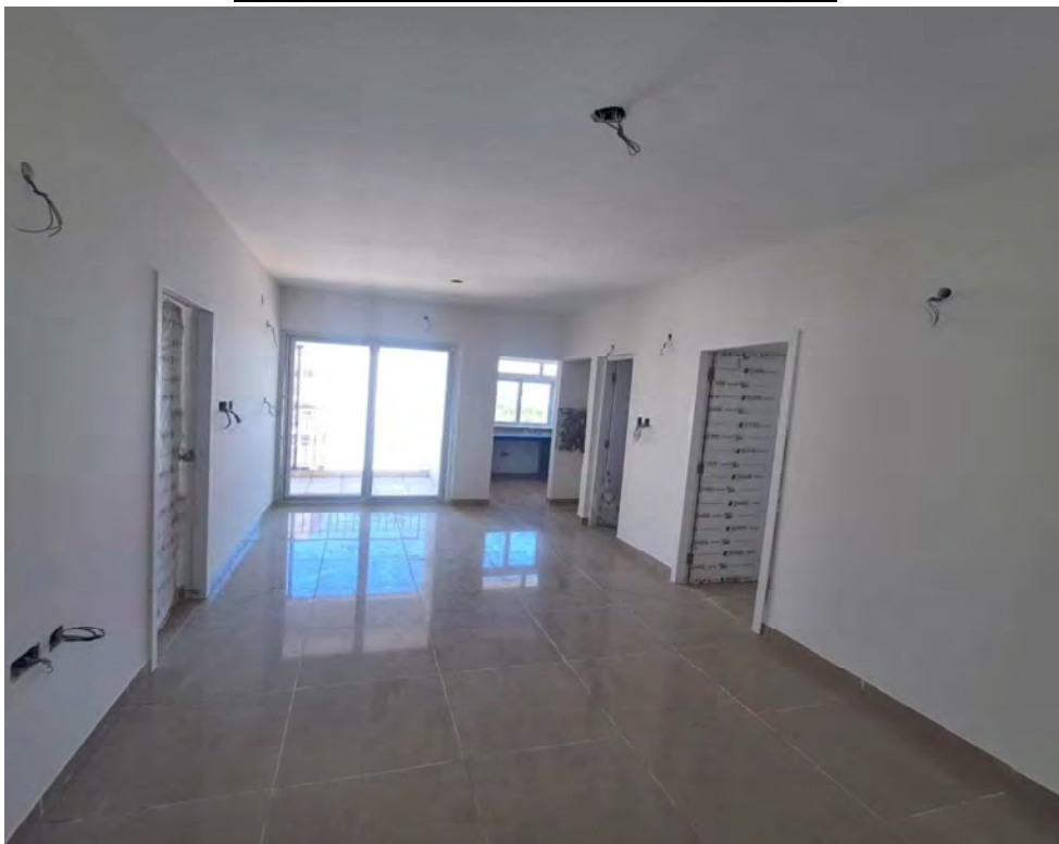
Block – D: First Floor Painting Work in Progress
