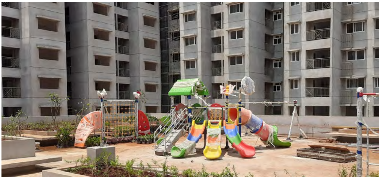
Tower B – Pic 4 – Play Equipment
