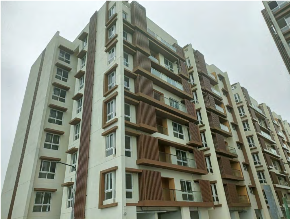
Block 6: Tower J -External & Common area Painting in progress.
