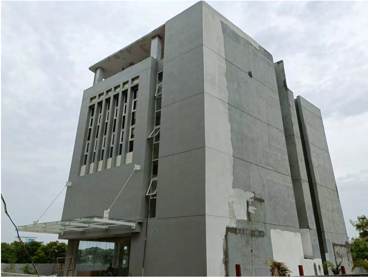
Block 7 : Club House – External Painting work in progress
