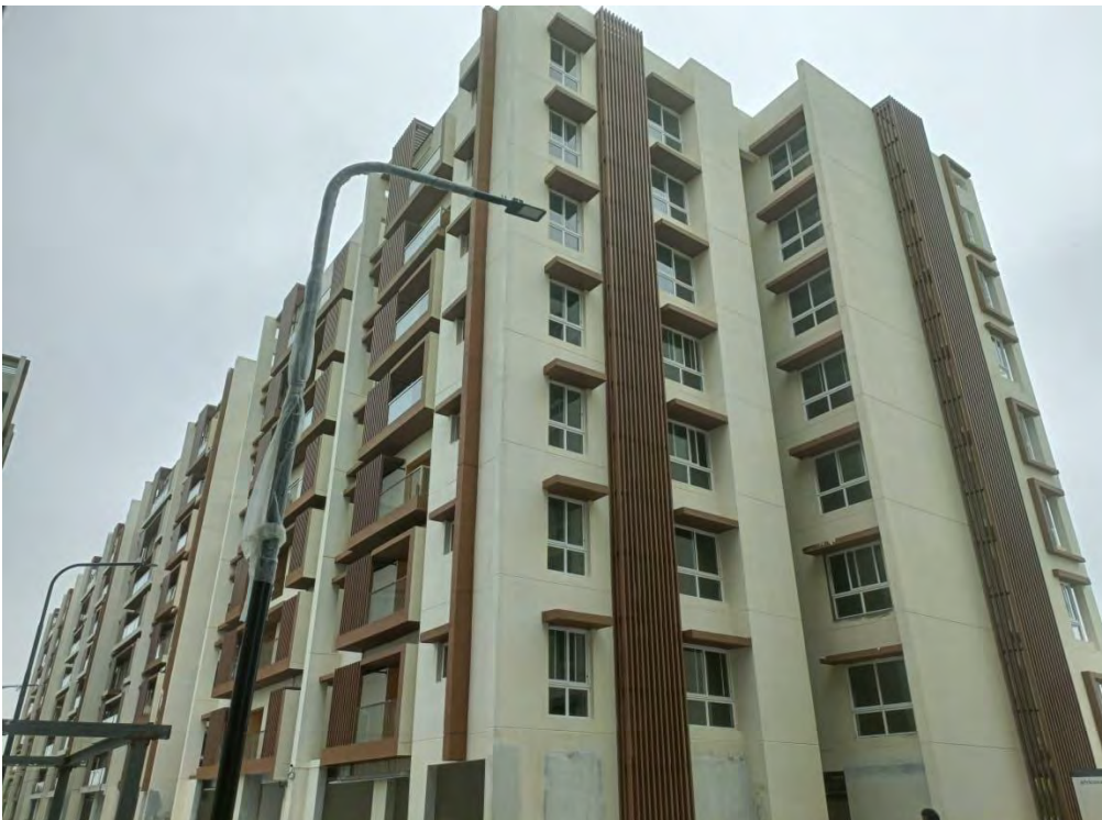
Block 6 : Tower G – External & Common area Painting in progress
