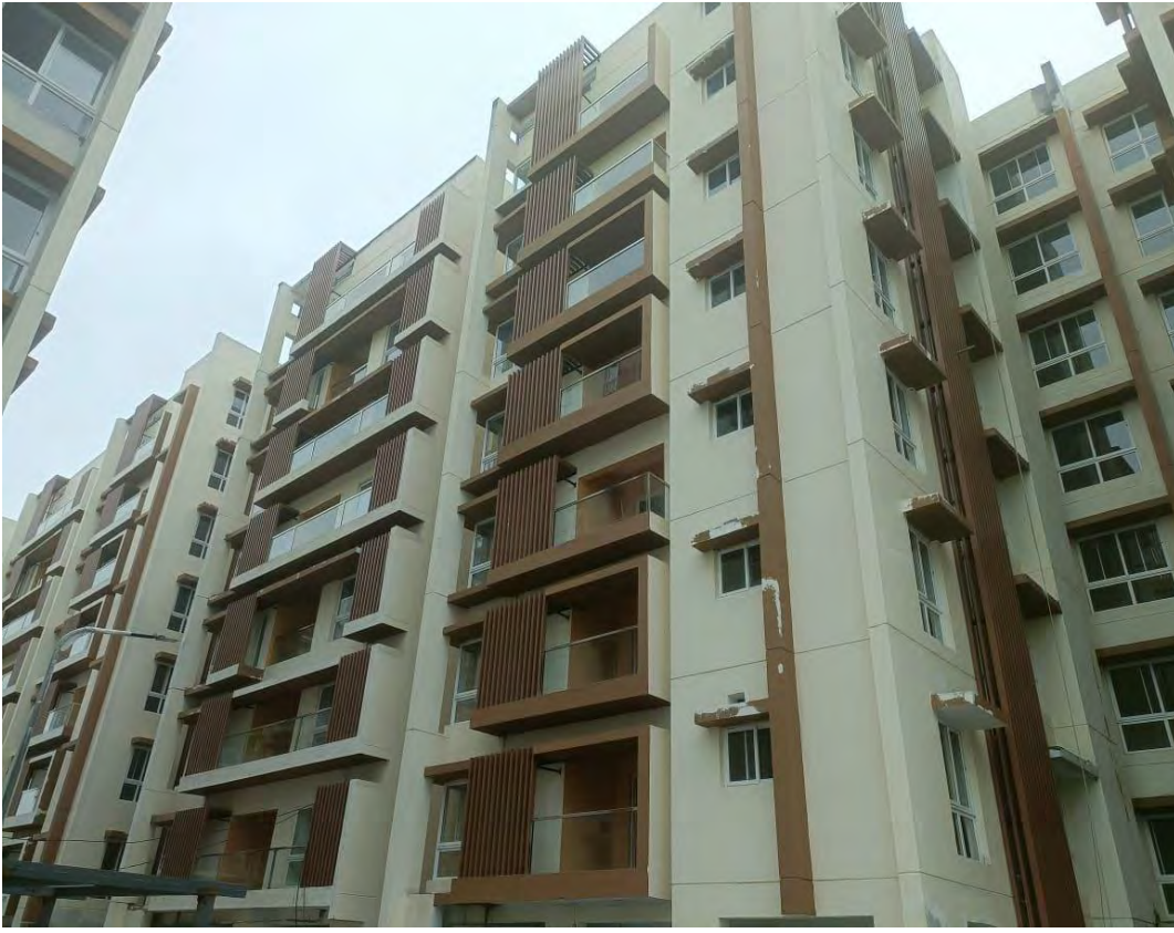
Block 6 : Tower H – External & Common area Painting in progress
