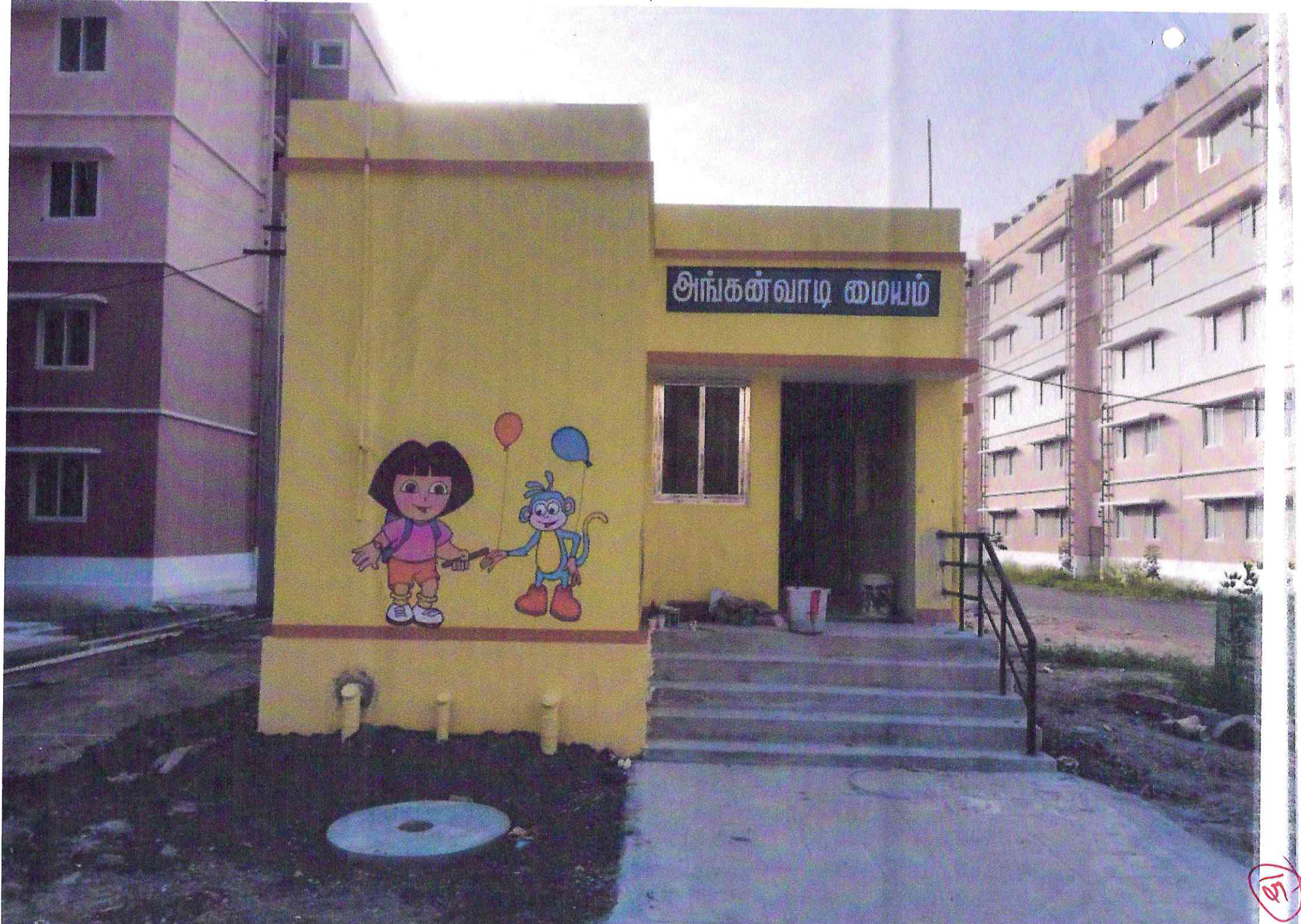
N/w: Construction of 1500 S.km Tenements @ Perianaickenpalayam, Coimbatore
