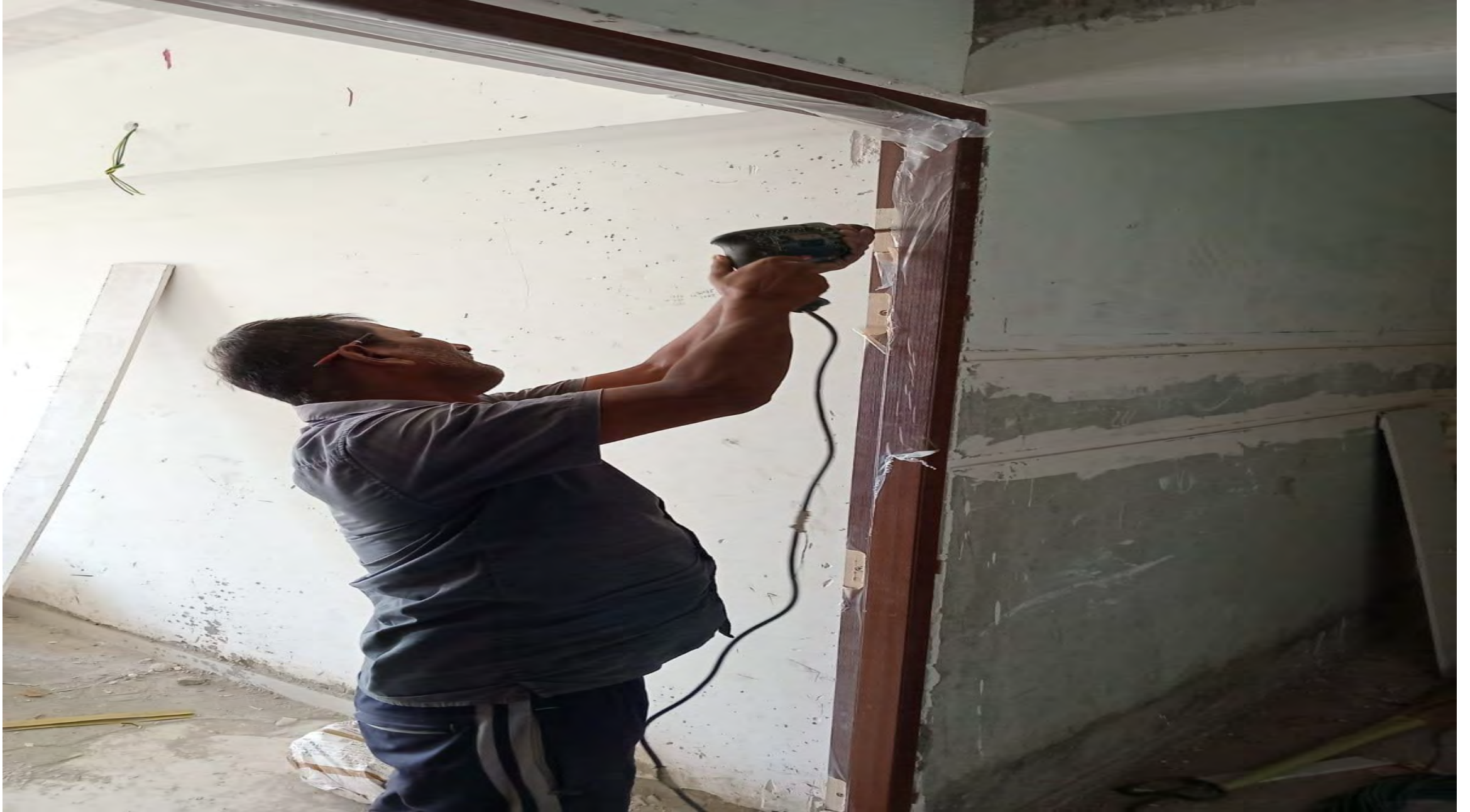
E2 1505 Doors fixing work in progress.
