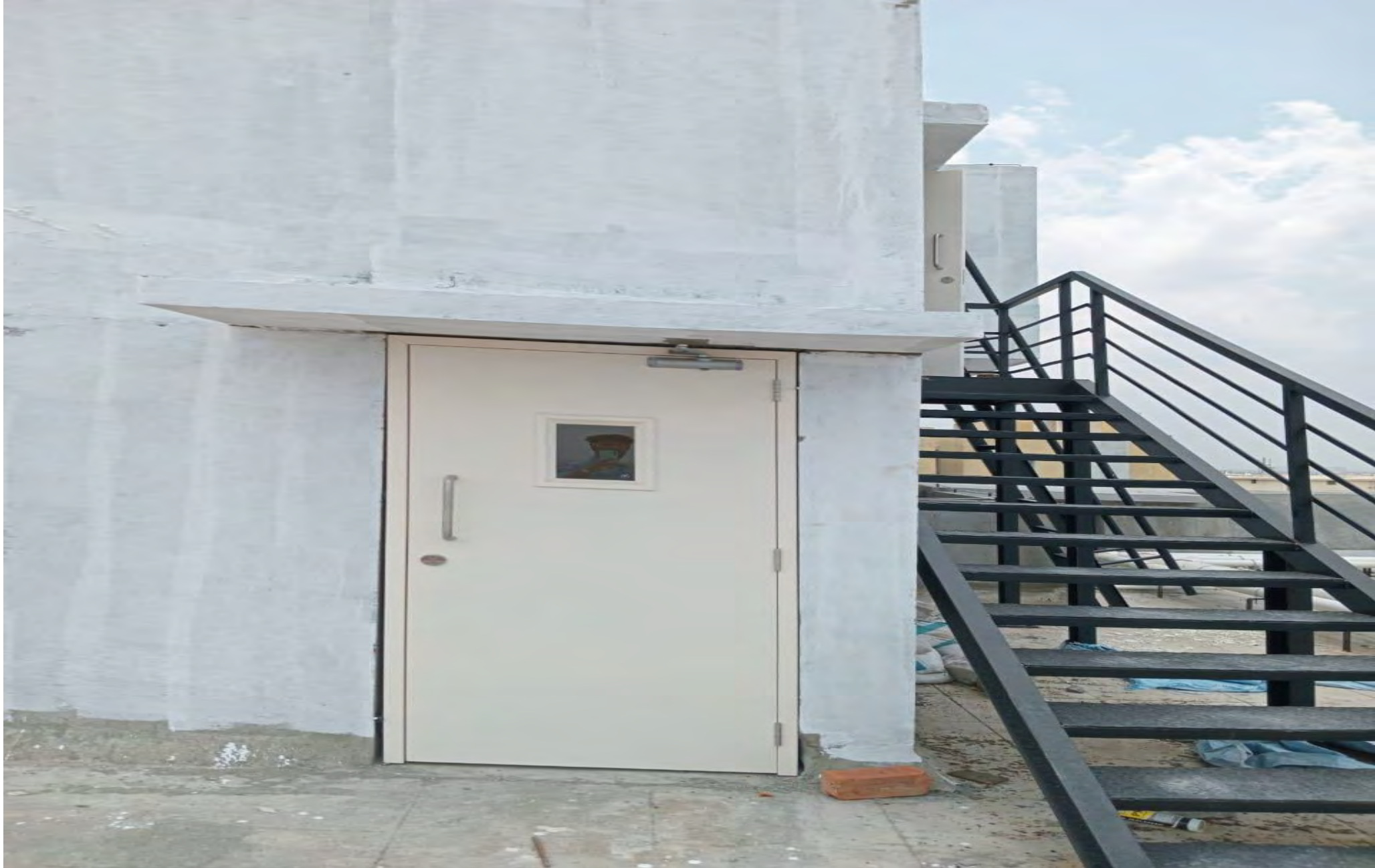
E2 Terrace headroom door fixing work completed.
