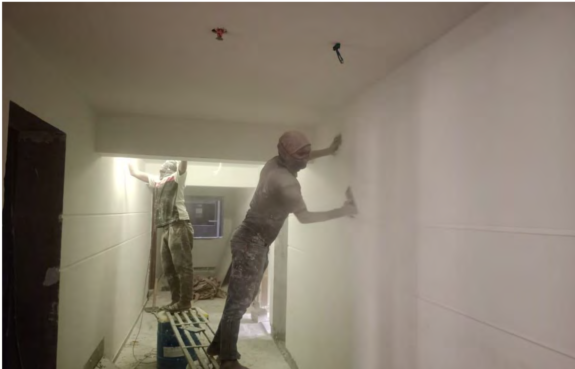
E1 B 3 rd floor corridor putty sanding work in progress.
