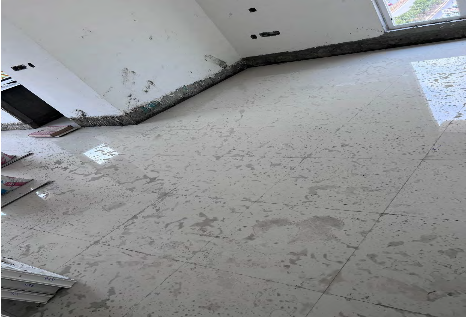
E1 A 1206 Floor tile work.
