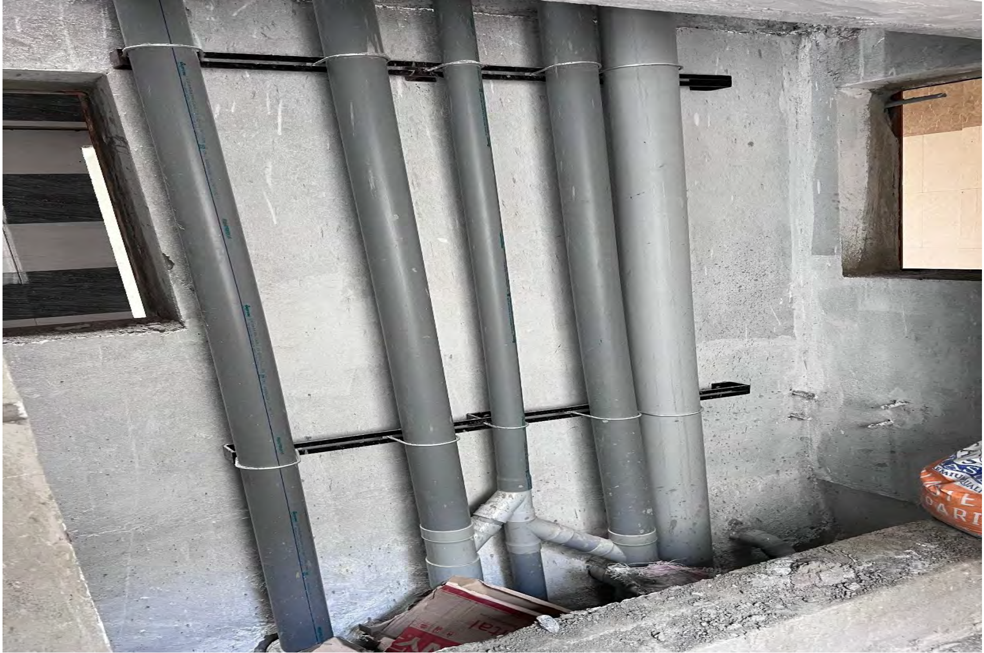
E1 A block plumbing shafts pipe line work.
