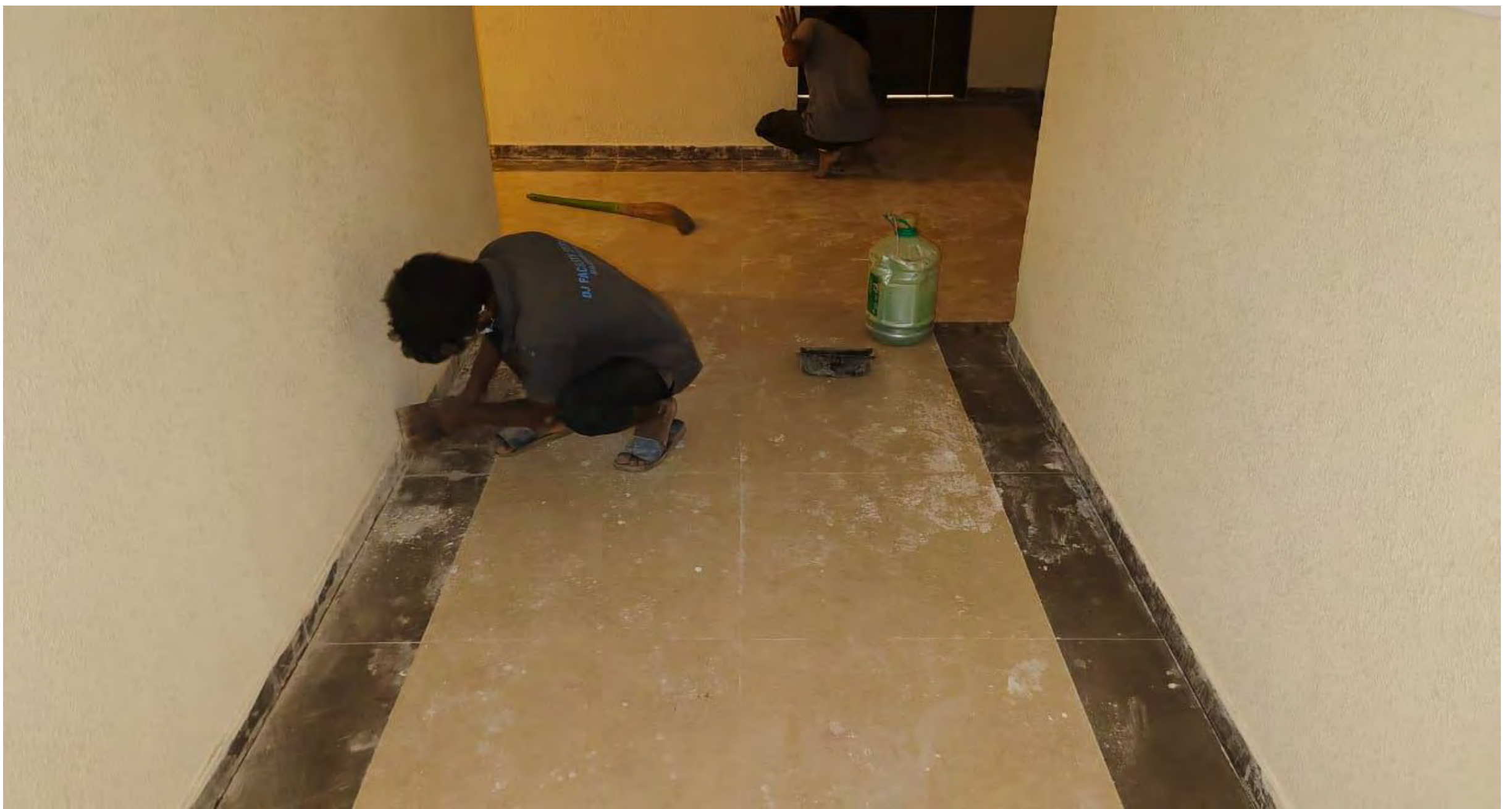
E2 4th floor Deep cleaning work in progress.
