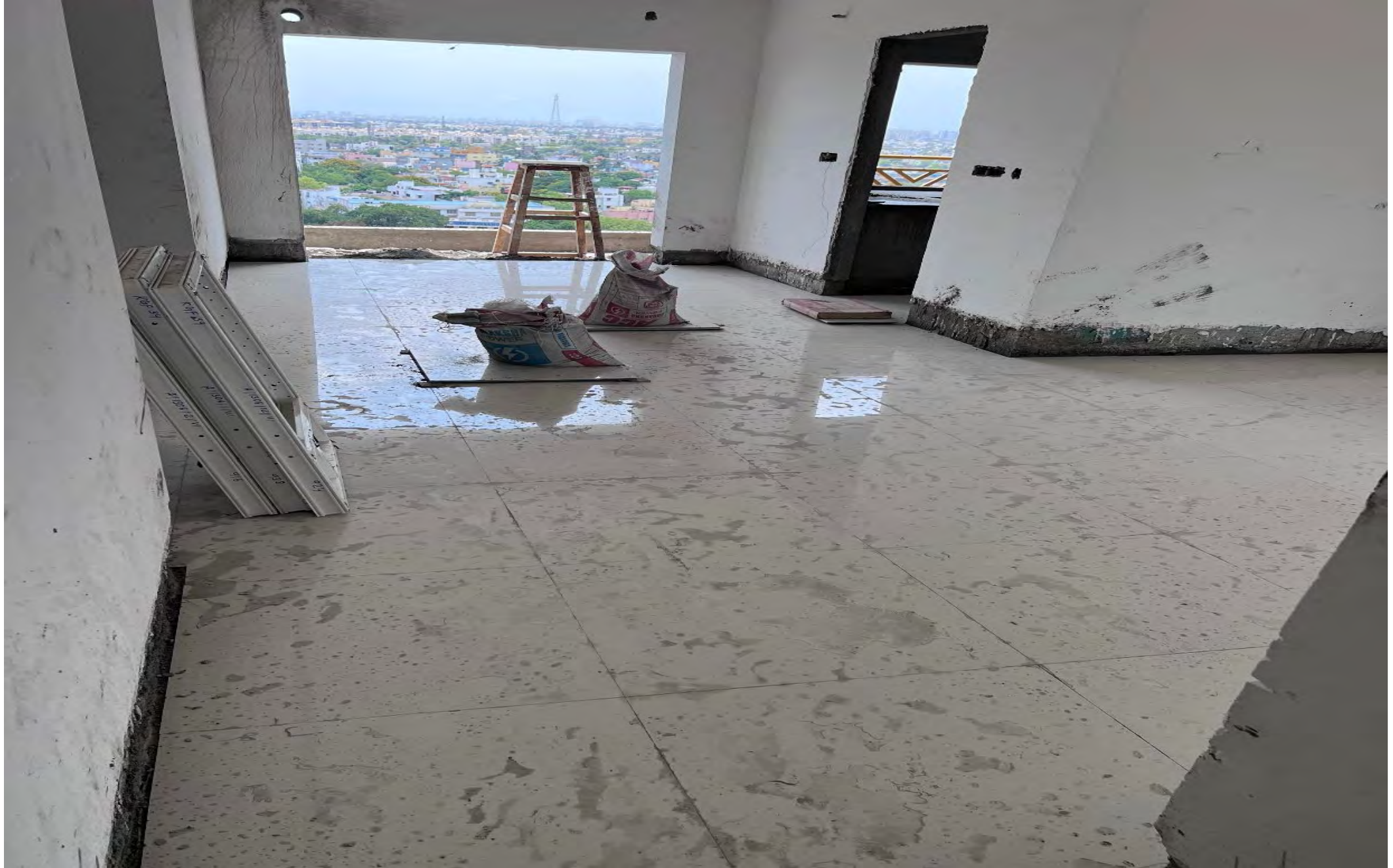
E1 B 1305 main flooring tiling work in progress.
