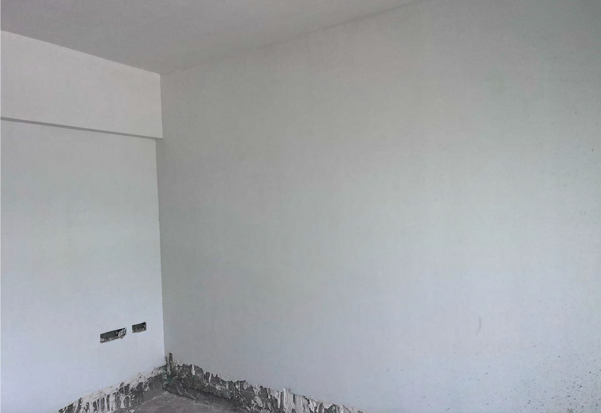
E1 A 14th floor primer applying work in progress.
