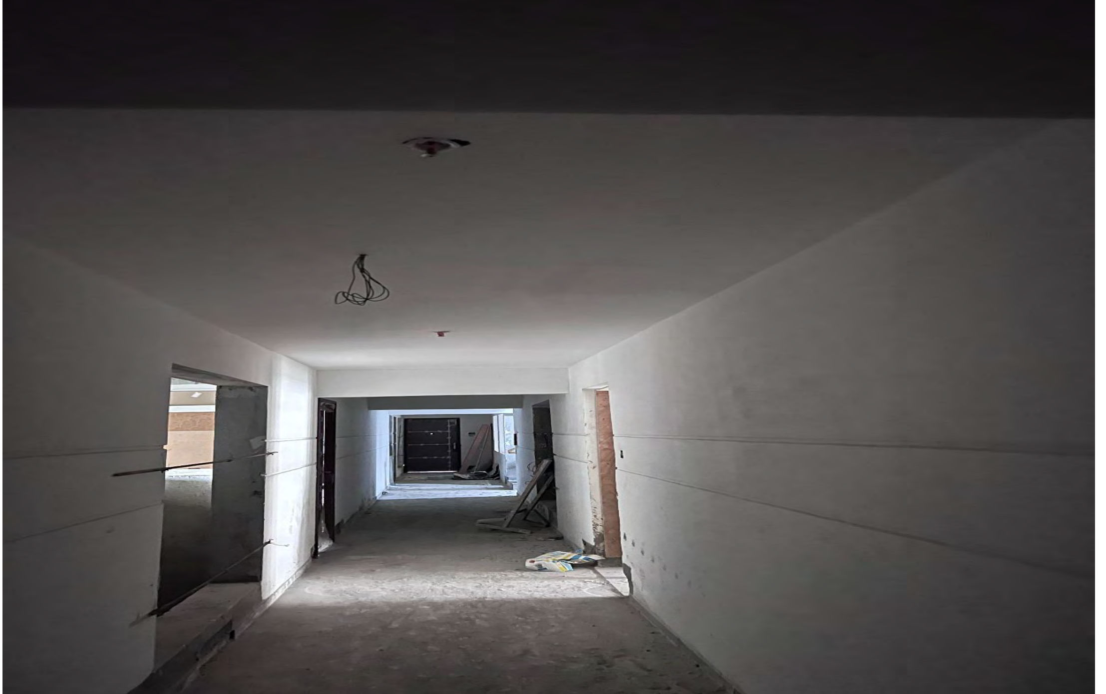
E1 A 4 th floor corridor false ceiling
