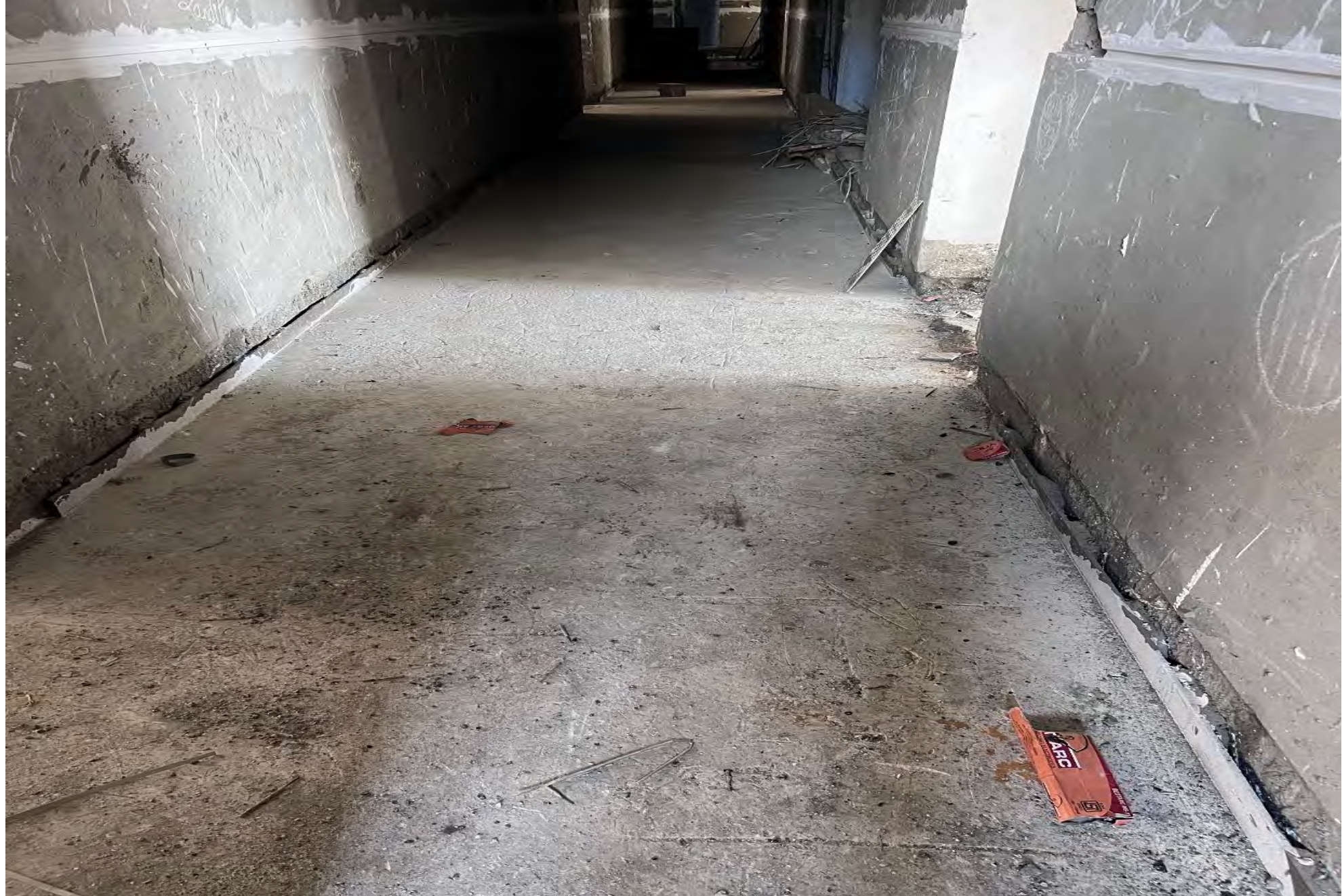
E1 B 13th floor Tile protection work
