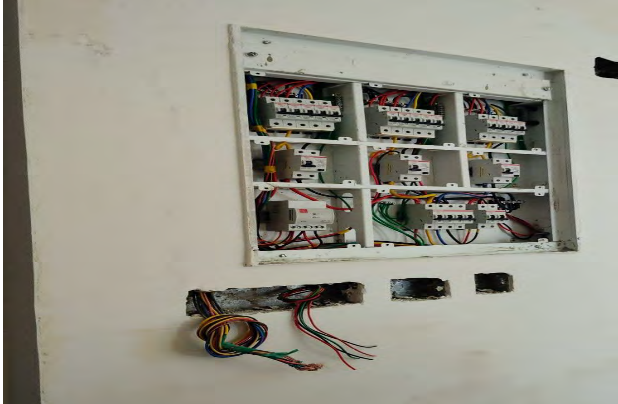
E1 A 104 main DB MCB fixing.
