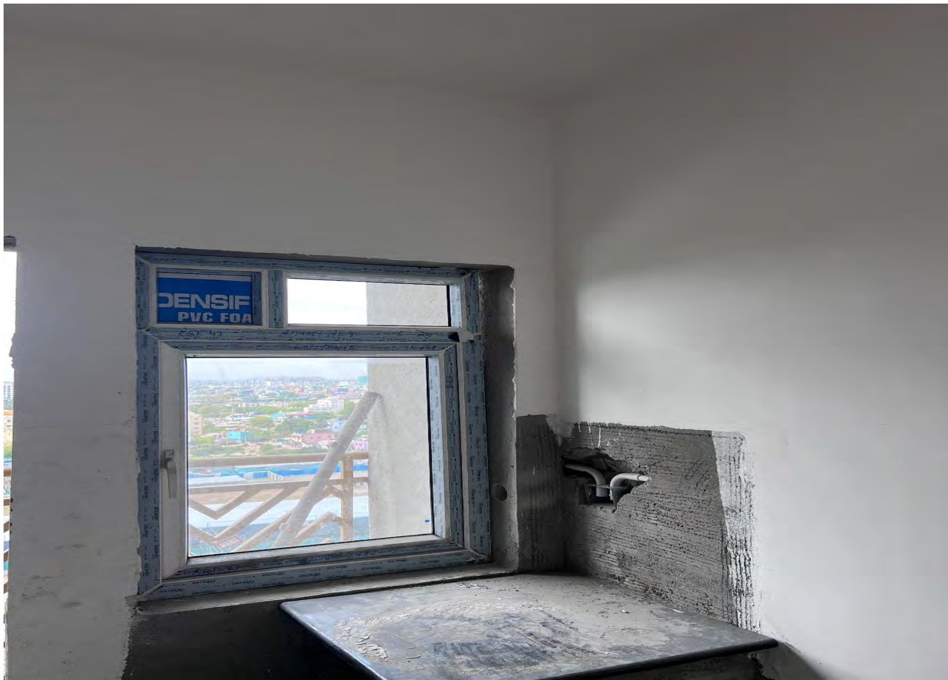
E1 8th floor kitchen window fixing.
