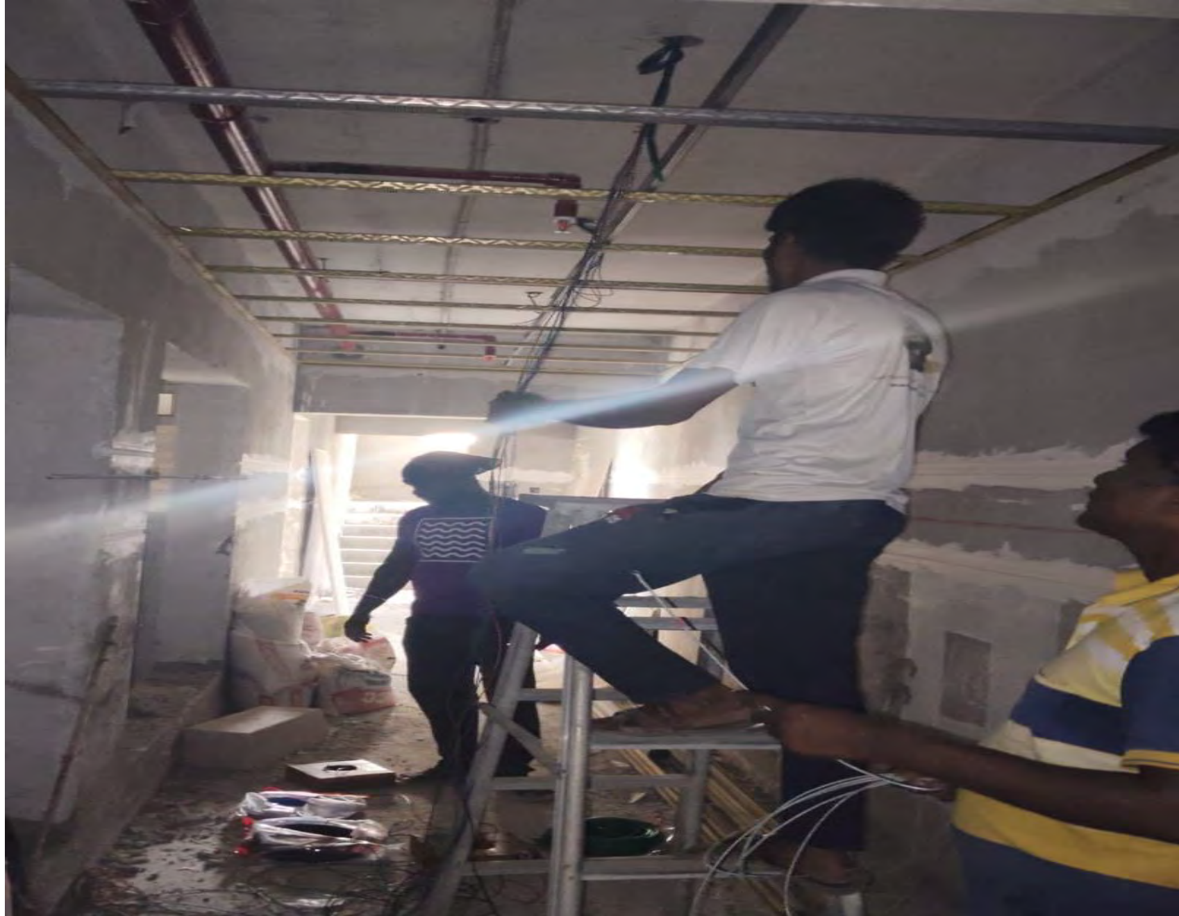
E1 B 6 th floor corridor wiring work in progress.
