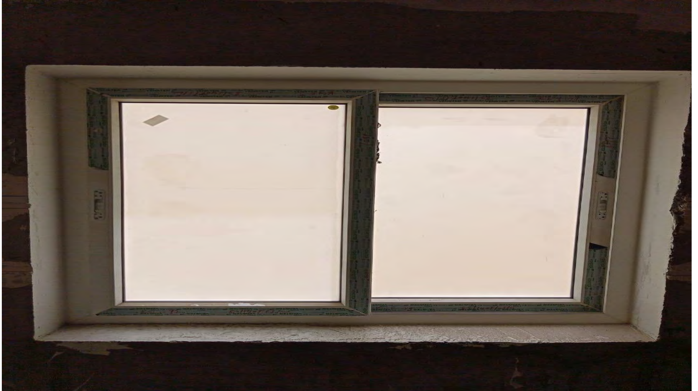
E2 12th floor Corridor windows fixing work in progress.
