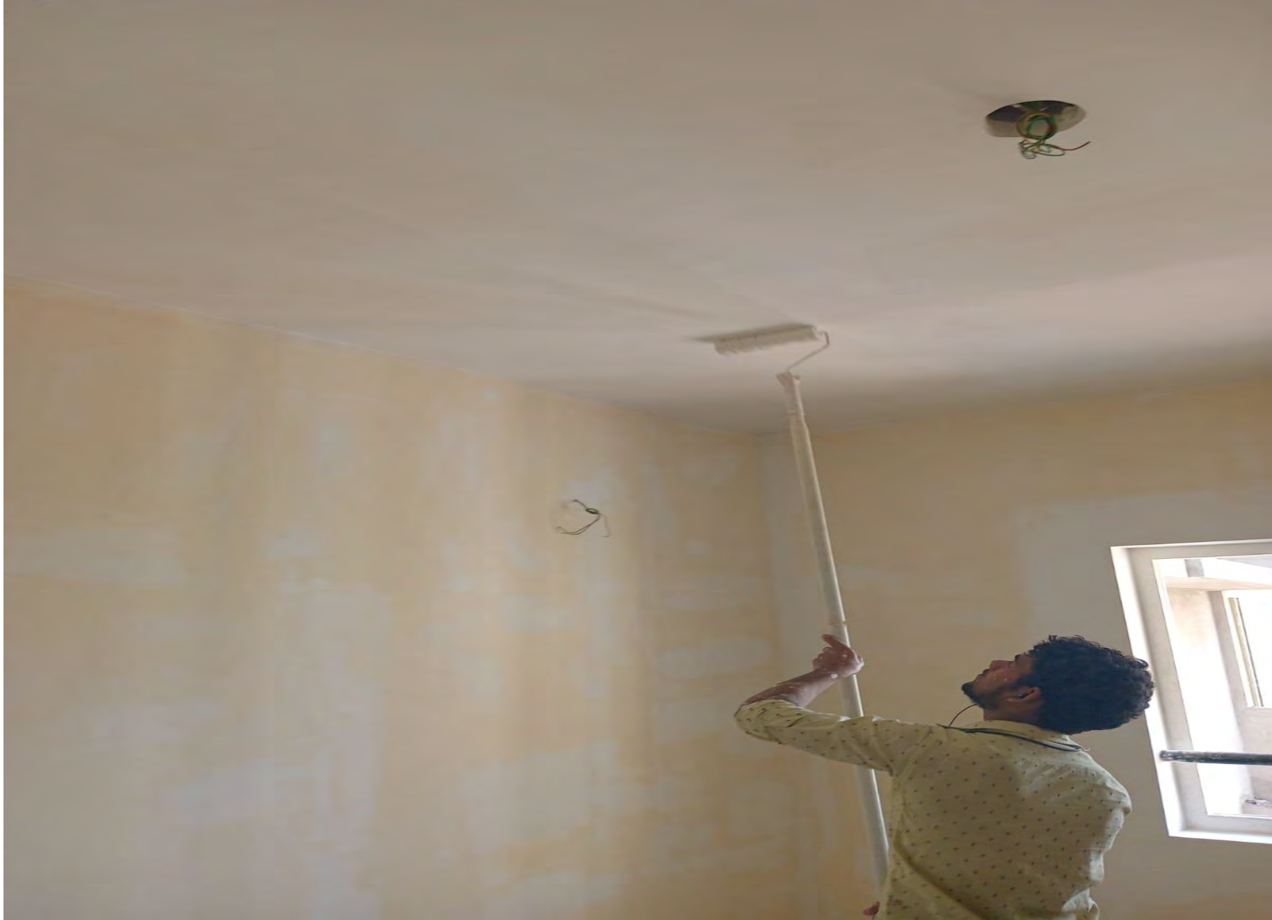
E2 1102 flat final coat painting work in progress
