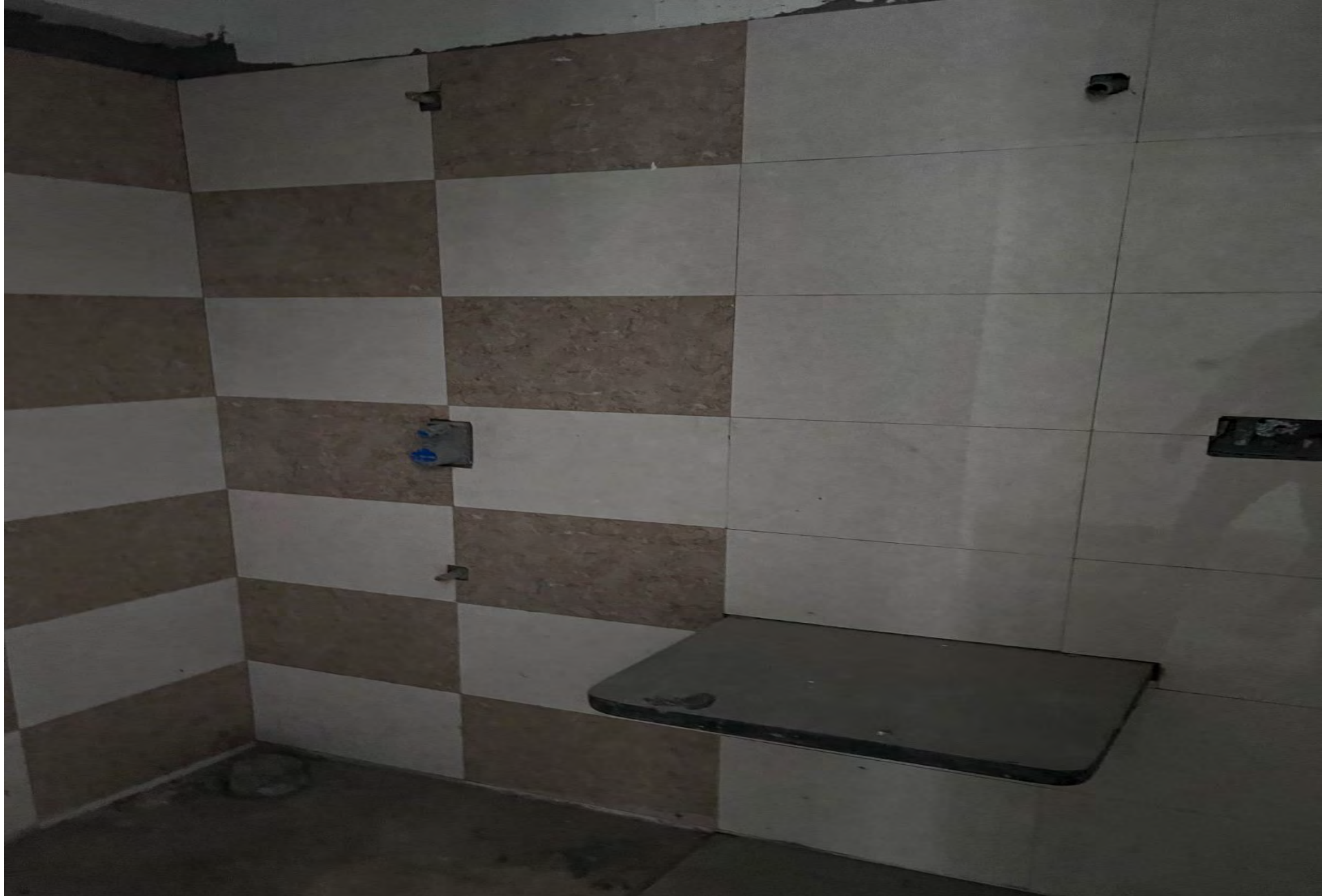
E1 A 13th floor master bathroom counter wash basin granite fixing
