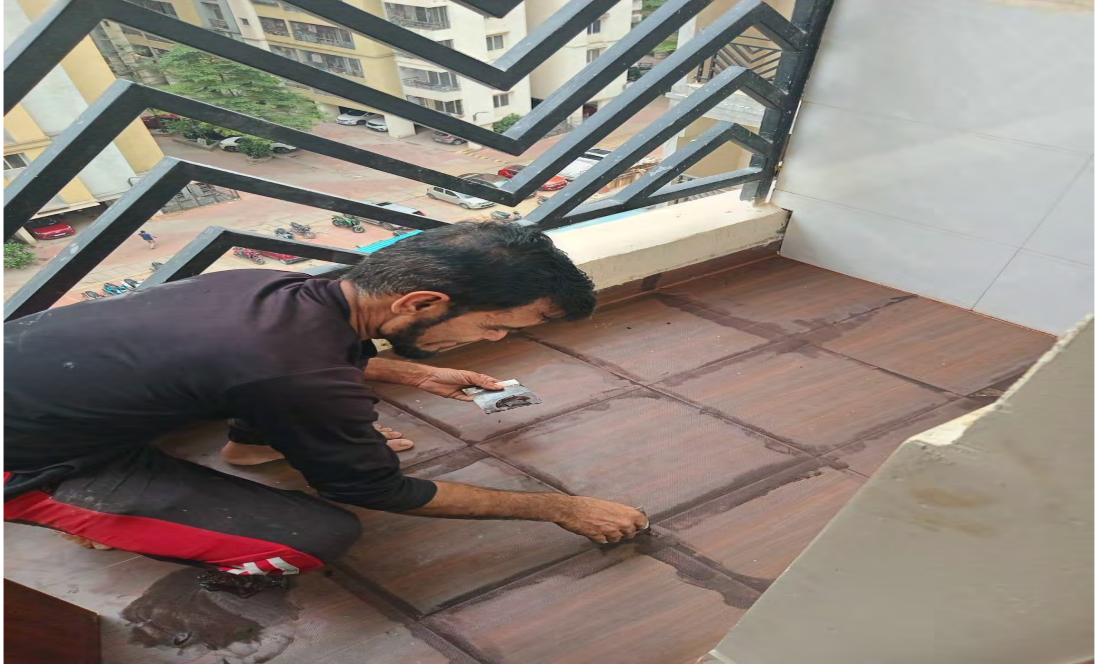
E2 8th floor balcony grouting work in progress
