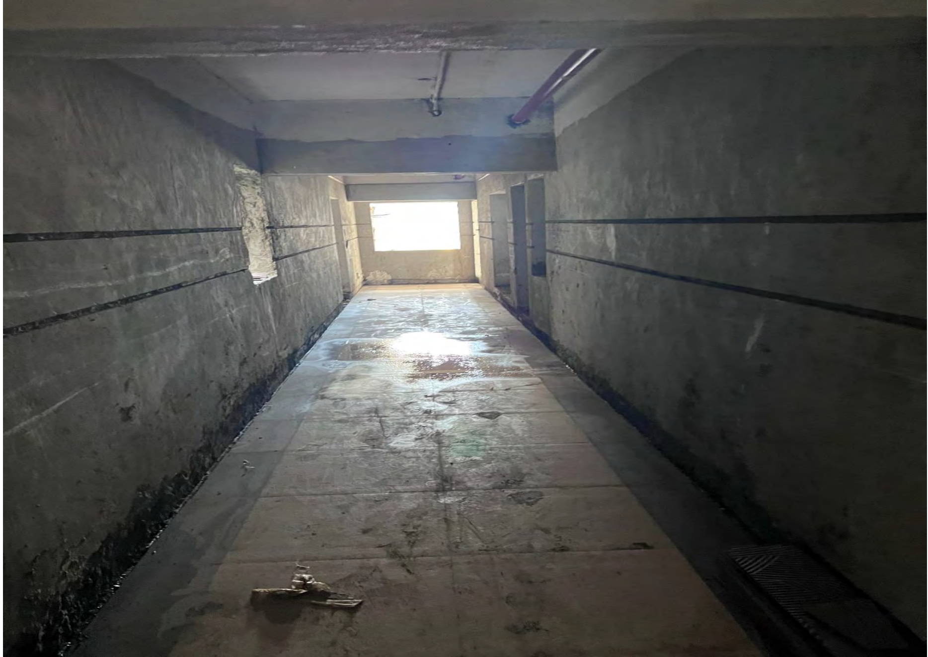
E1 B 12th floor corridor tile work.
