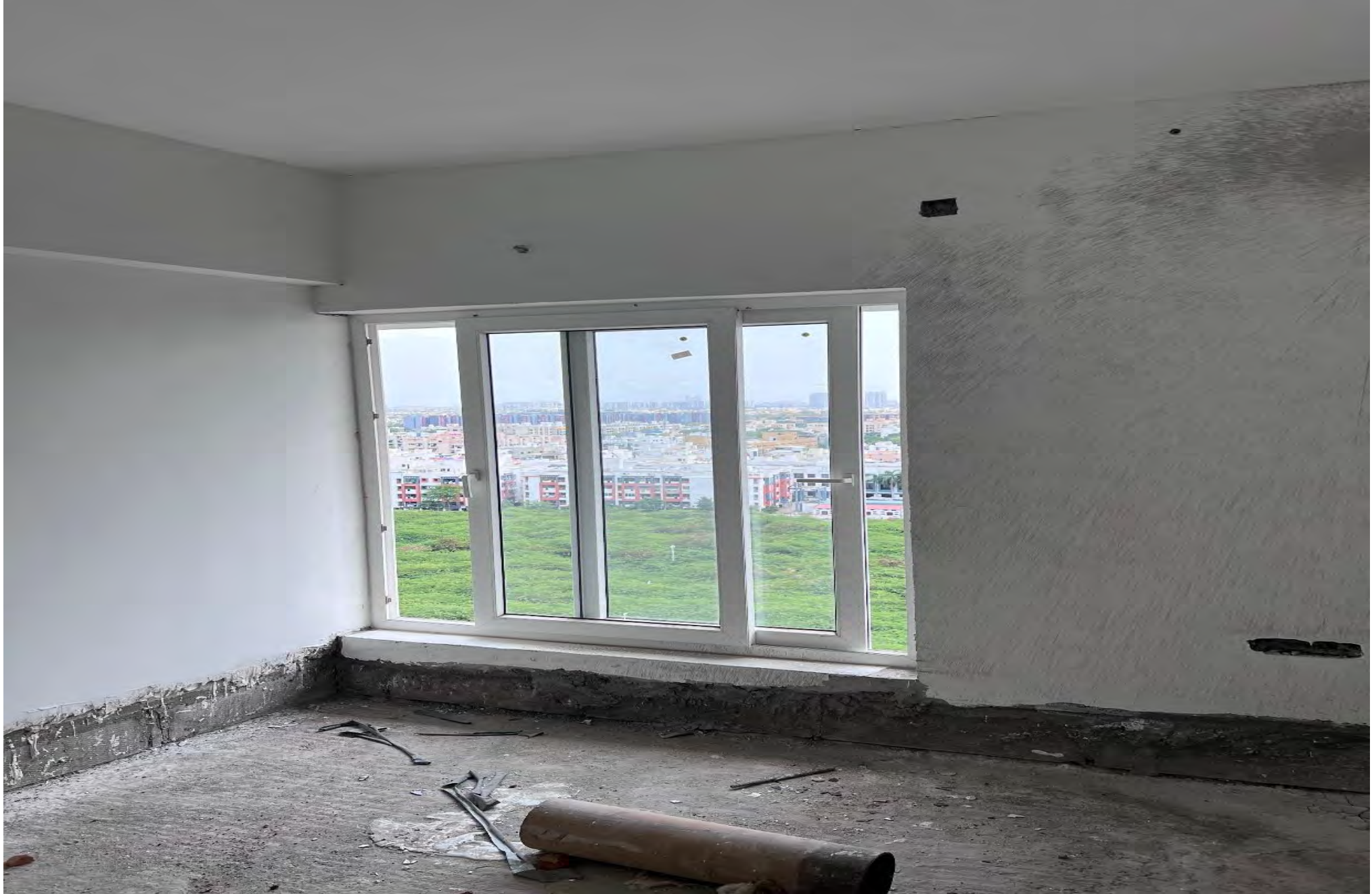
E1 B 13th floor External window shutters.
