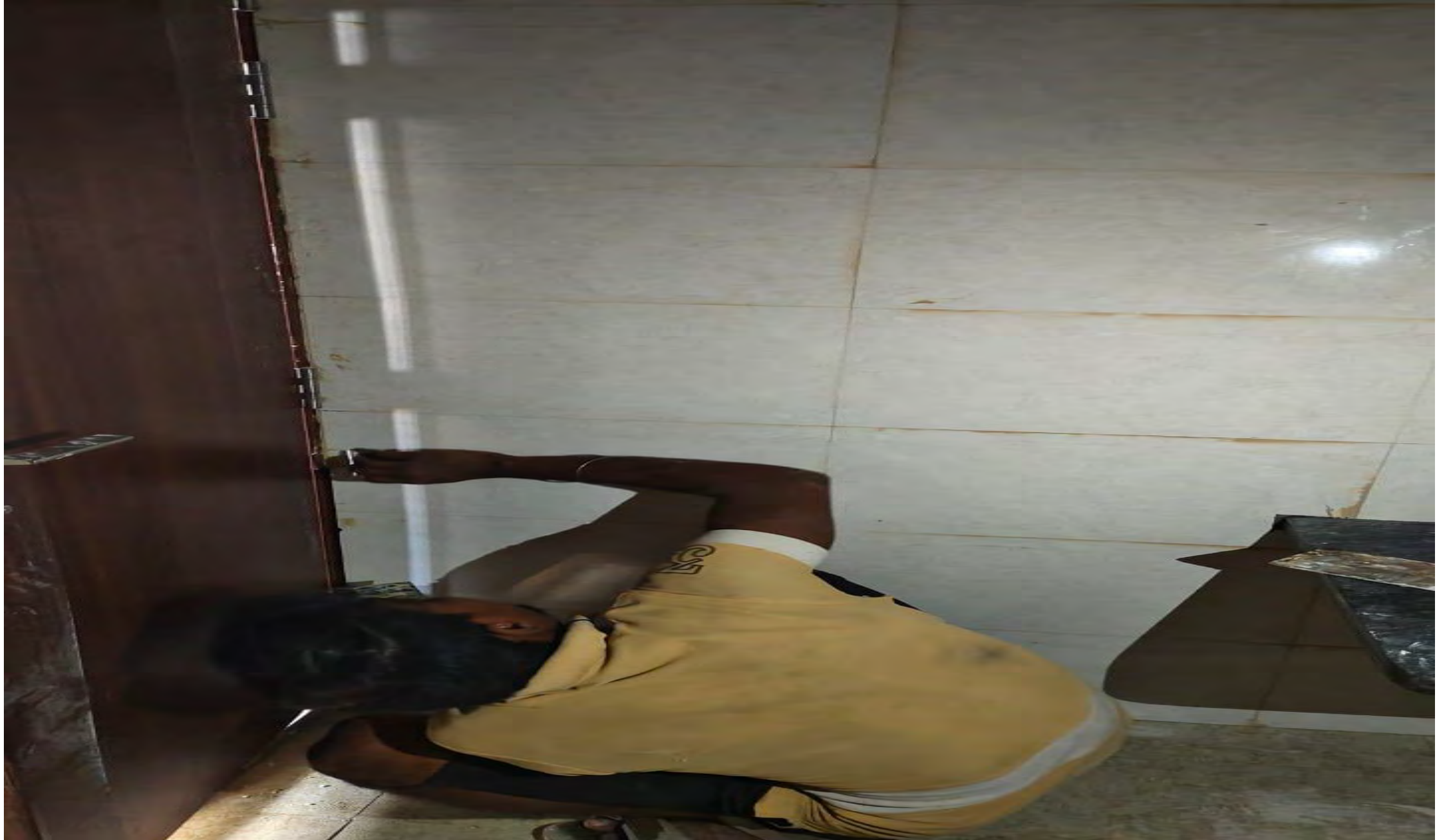
E2 7th floor Grouting work in progress.
