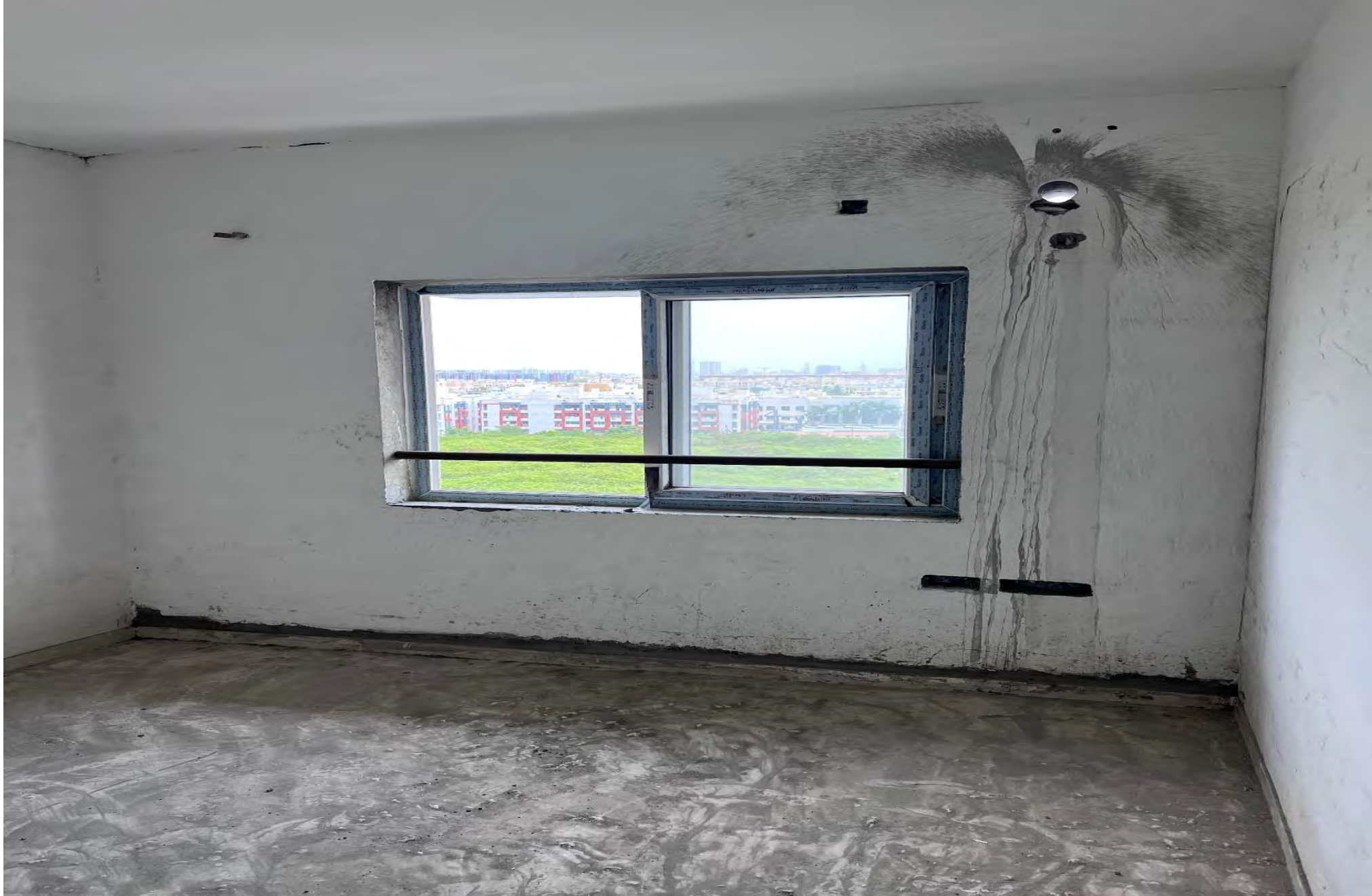
E1 B 15 th floor External windows fixing wip.
