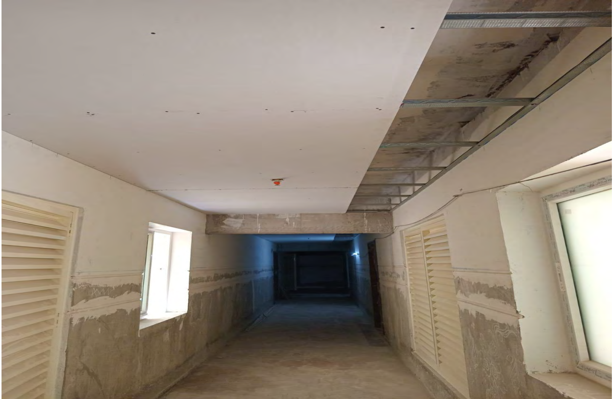
E2 10th floor Corridor false ceiling work in progress.
