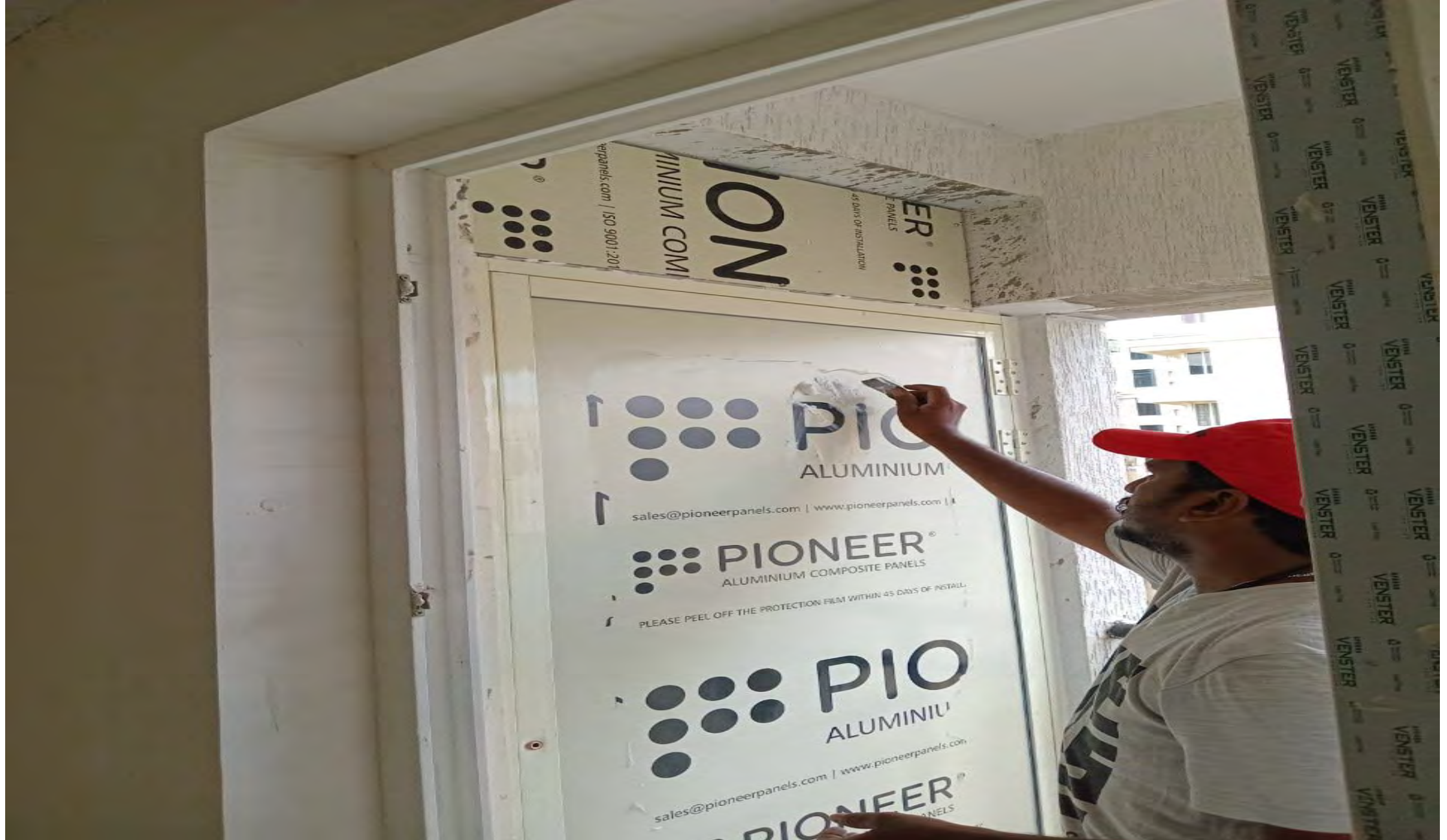
E2 1310 Balcony plumbing shaft ACP doors fixing.
