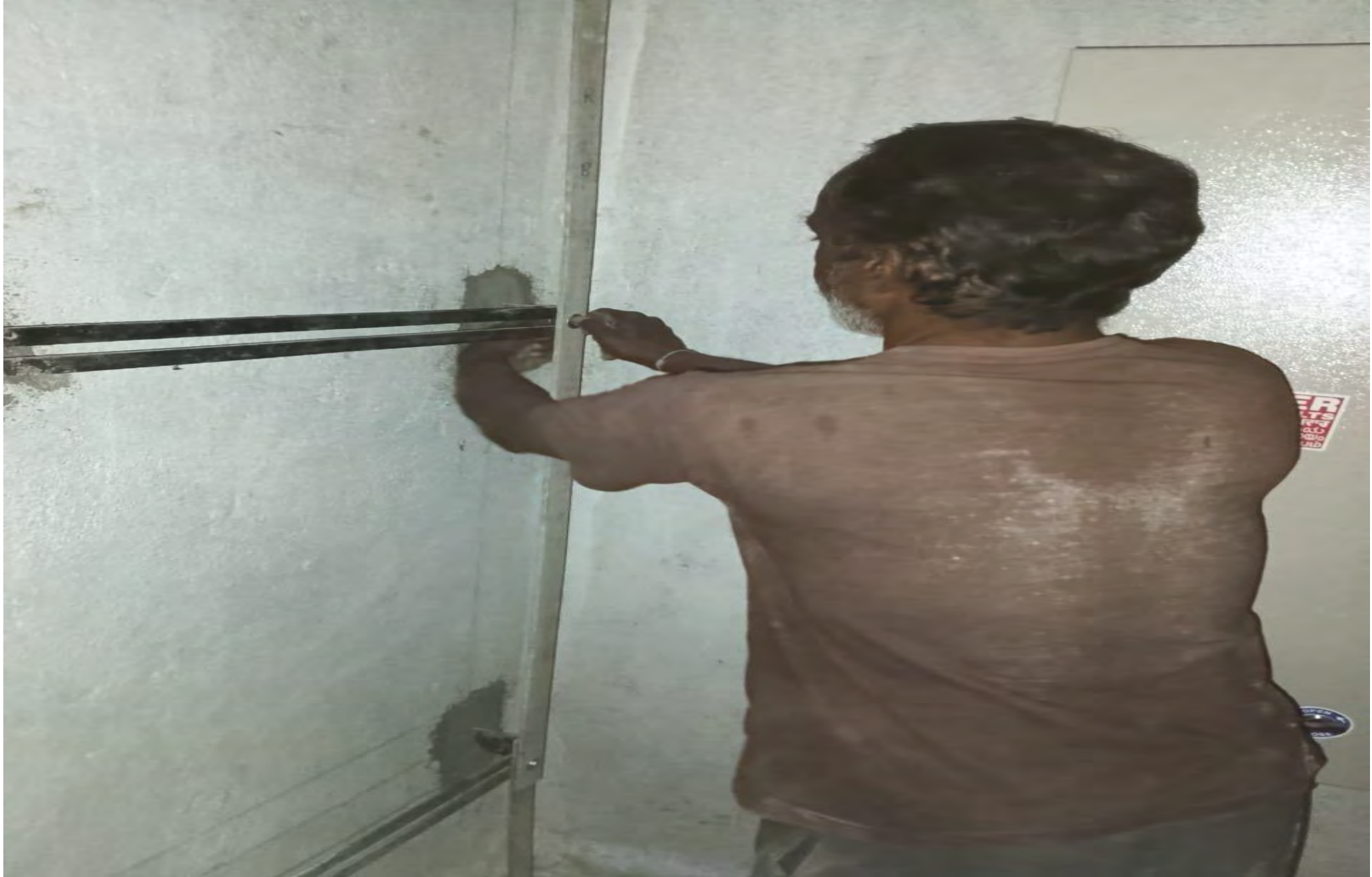
E1 A electrical shaft bracket fixing,
