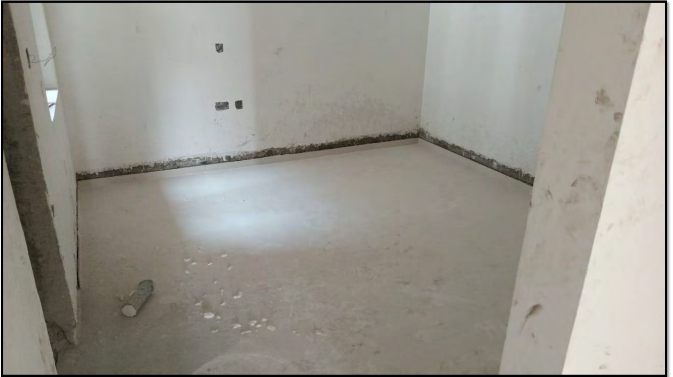
E1 A 12th floor- tile protection work
