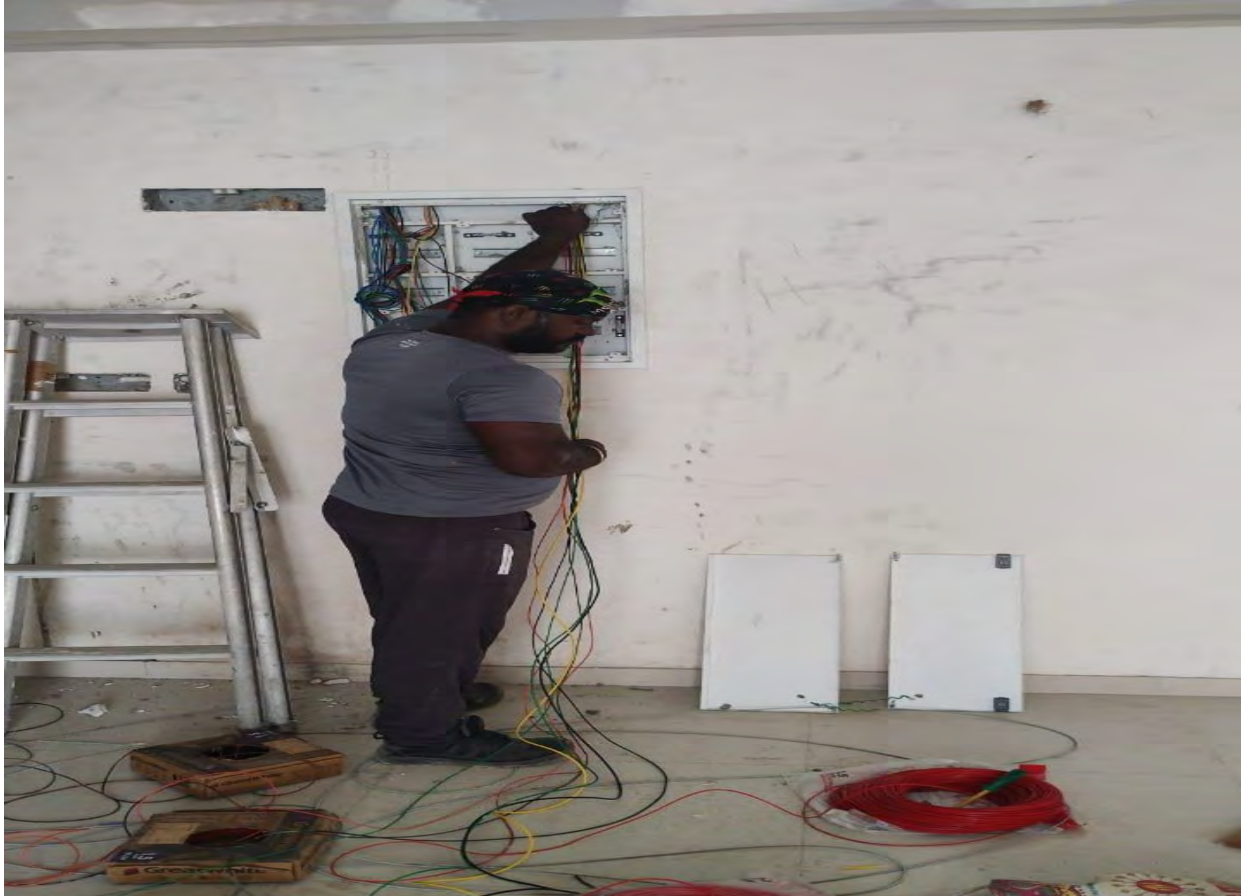
E1 A 206 flat wiring work on progress.
