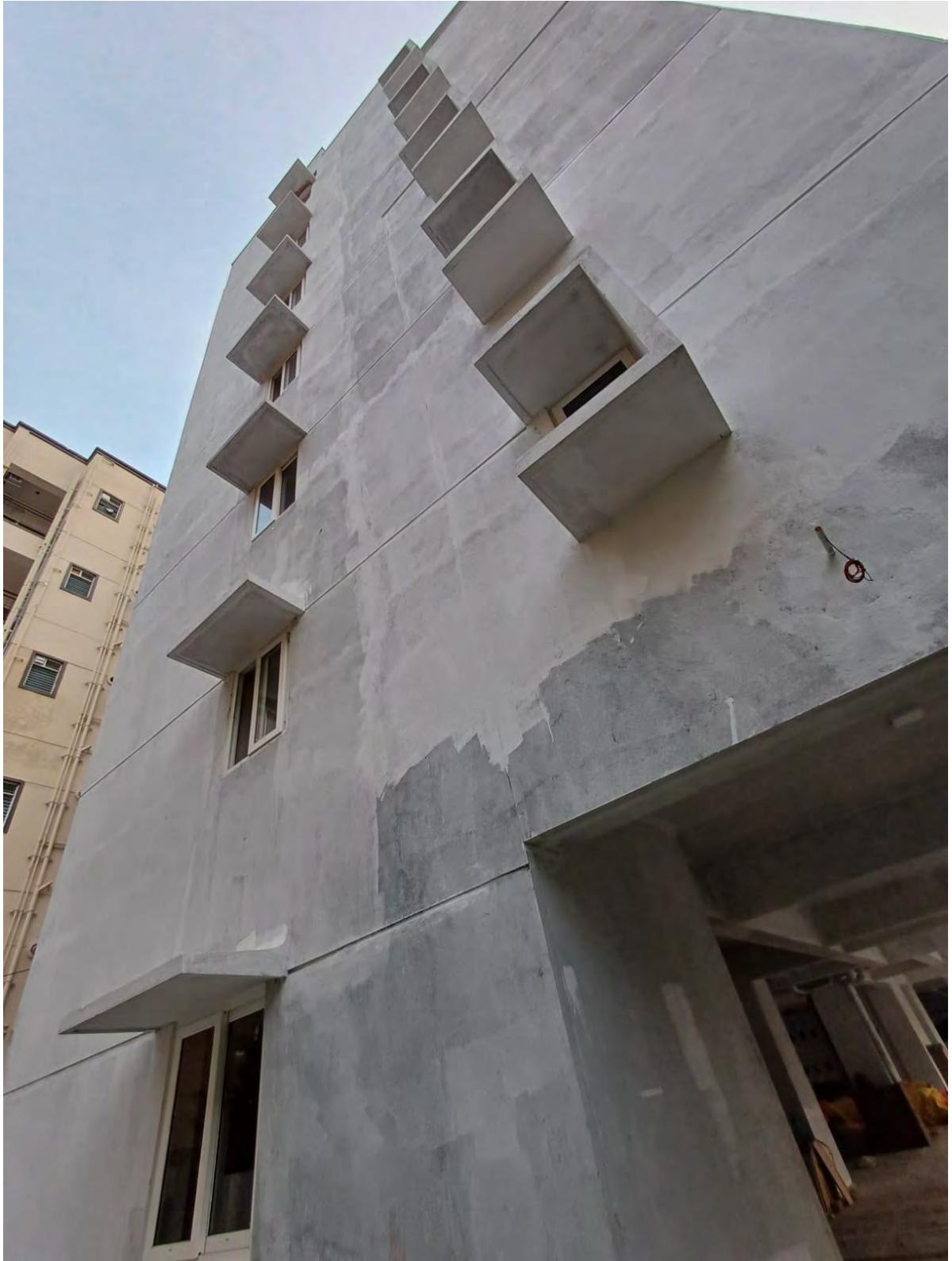
PHOTOGRAPH SHOWING NORTH SIDE ELEVATION - BLOCK – A (14/01/2025)
