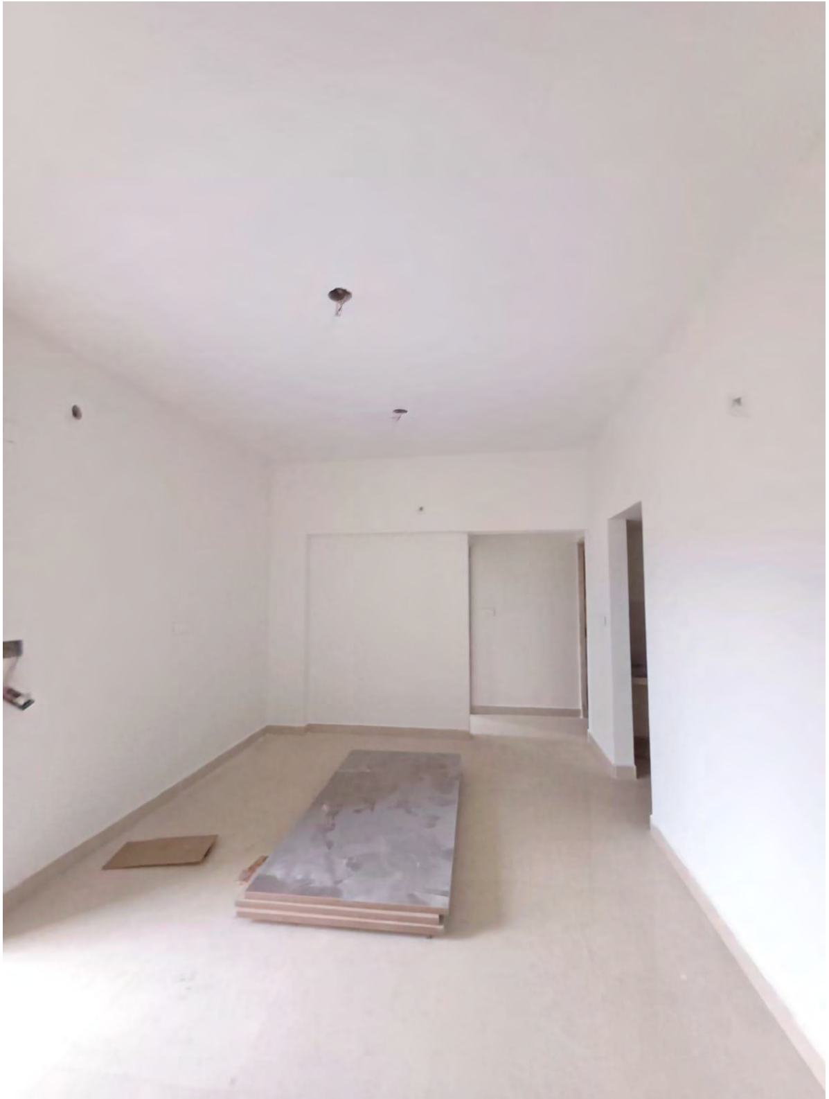
PHOTOGRAPH SHOWING FIFTH FLOOR INNER ROOMS - BLOCK – A (14/01/2025)
