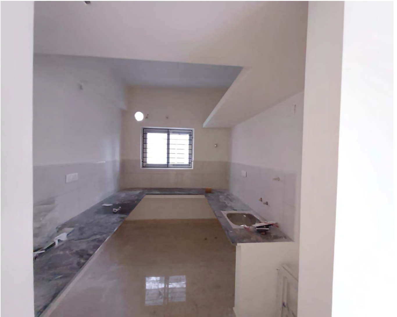
PHOTOGRAPH SHOWING FIFTH FLOOR KITCHEN - BLOCK – A (14/01/2025)
