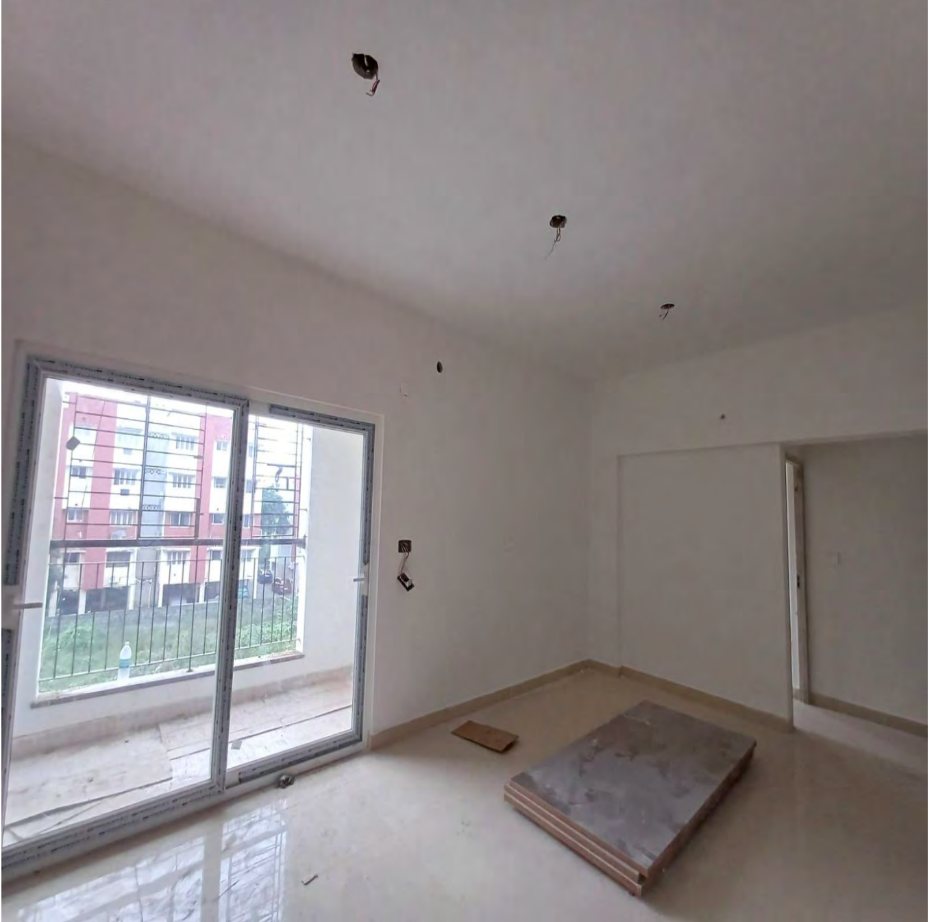
PHOTOGRAPH SHOWING FIFTH FLOOR LIVING ROOM - BLOCK – A (14/01/2025)
