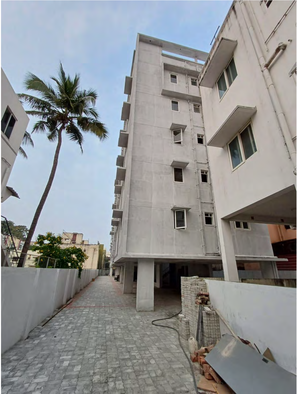
PHOTOGRAPH SHOWING SOUTH SIDE ELEVATION - BLOCK – A (14/01/2025)
