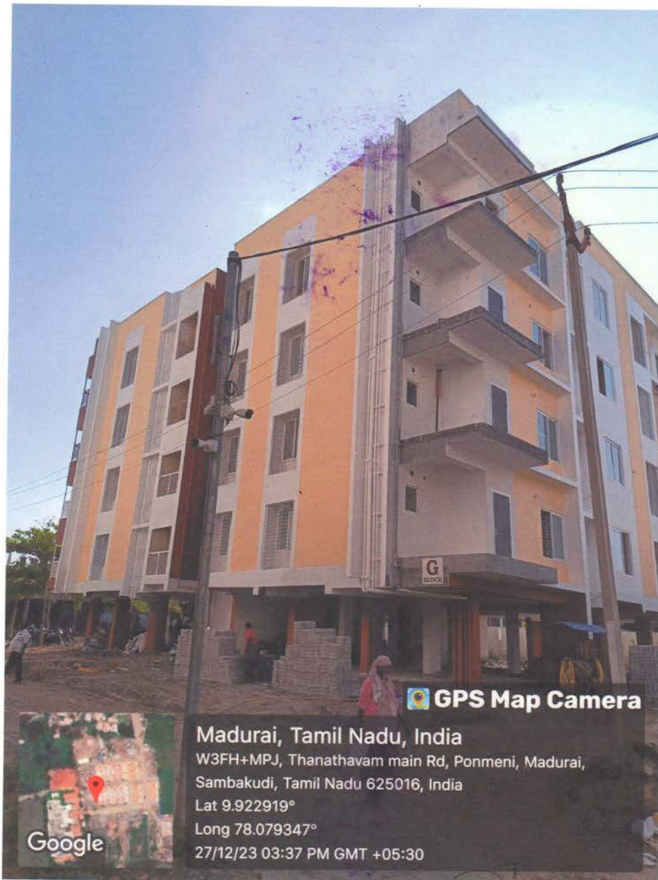
Figure 1: Painting and Completion of Works
