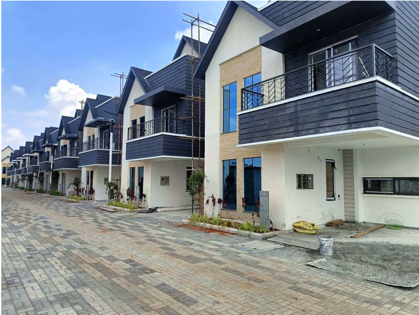
Painting work in progress
