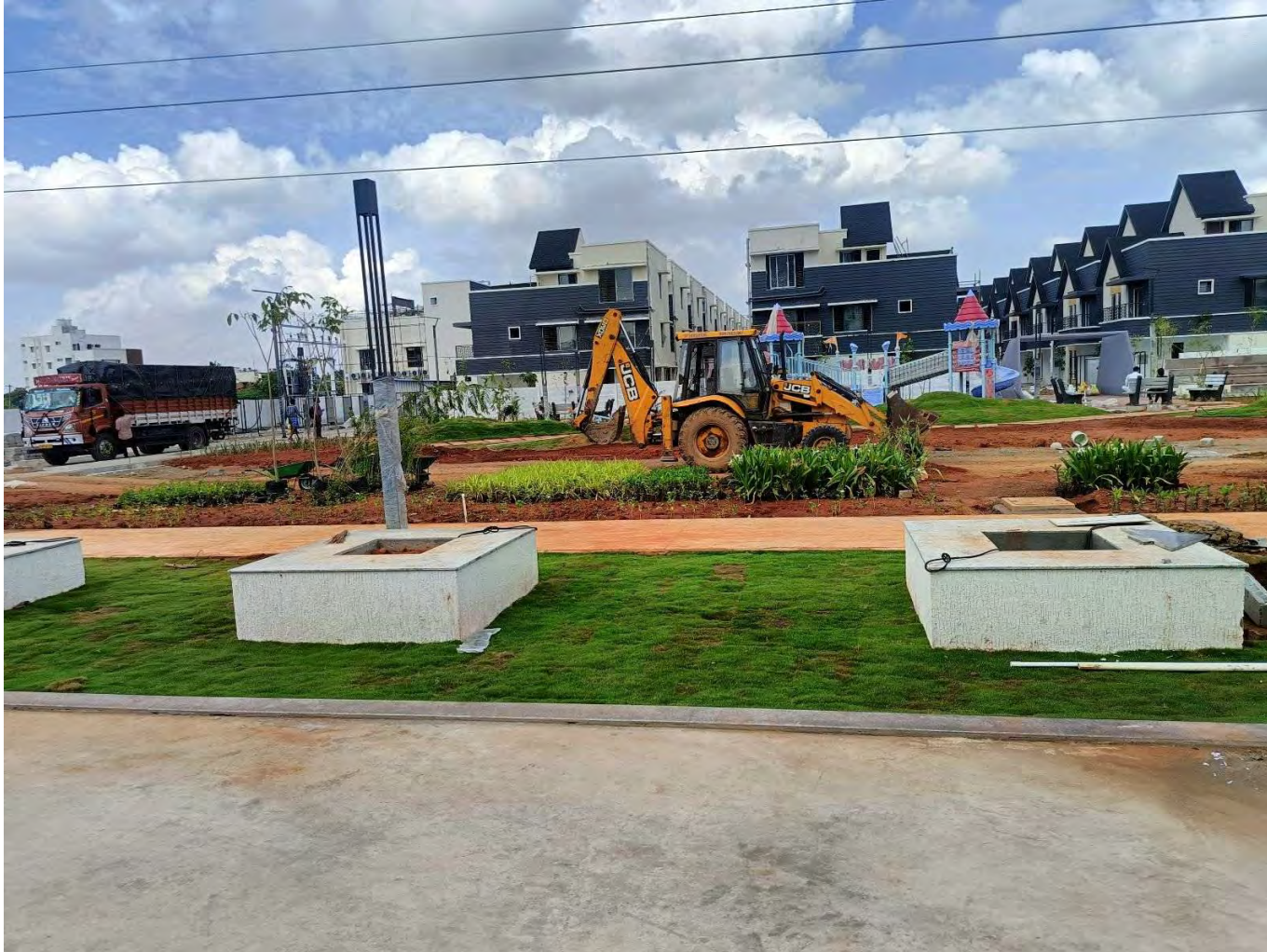
Landscape work in progress
