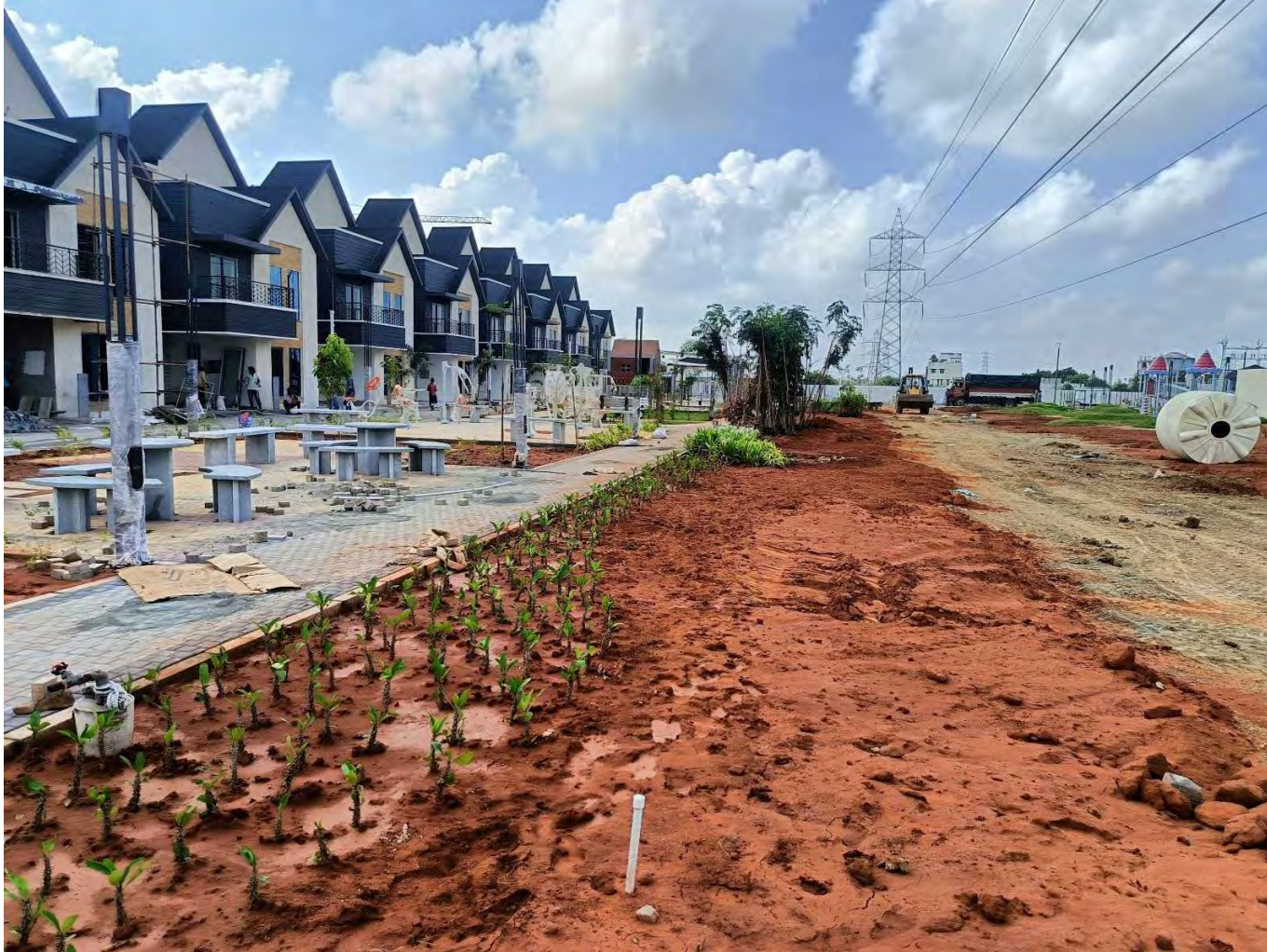
Landscape work in progress
