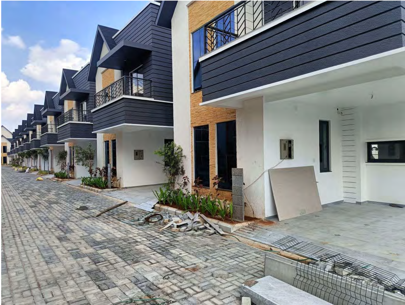
Snag work in progress
