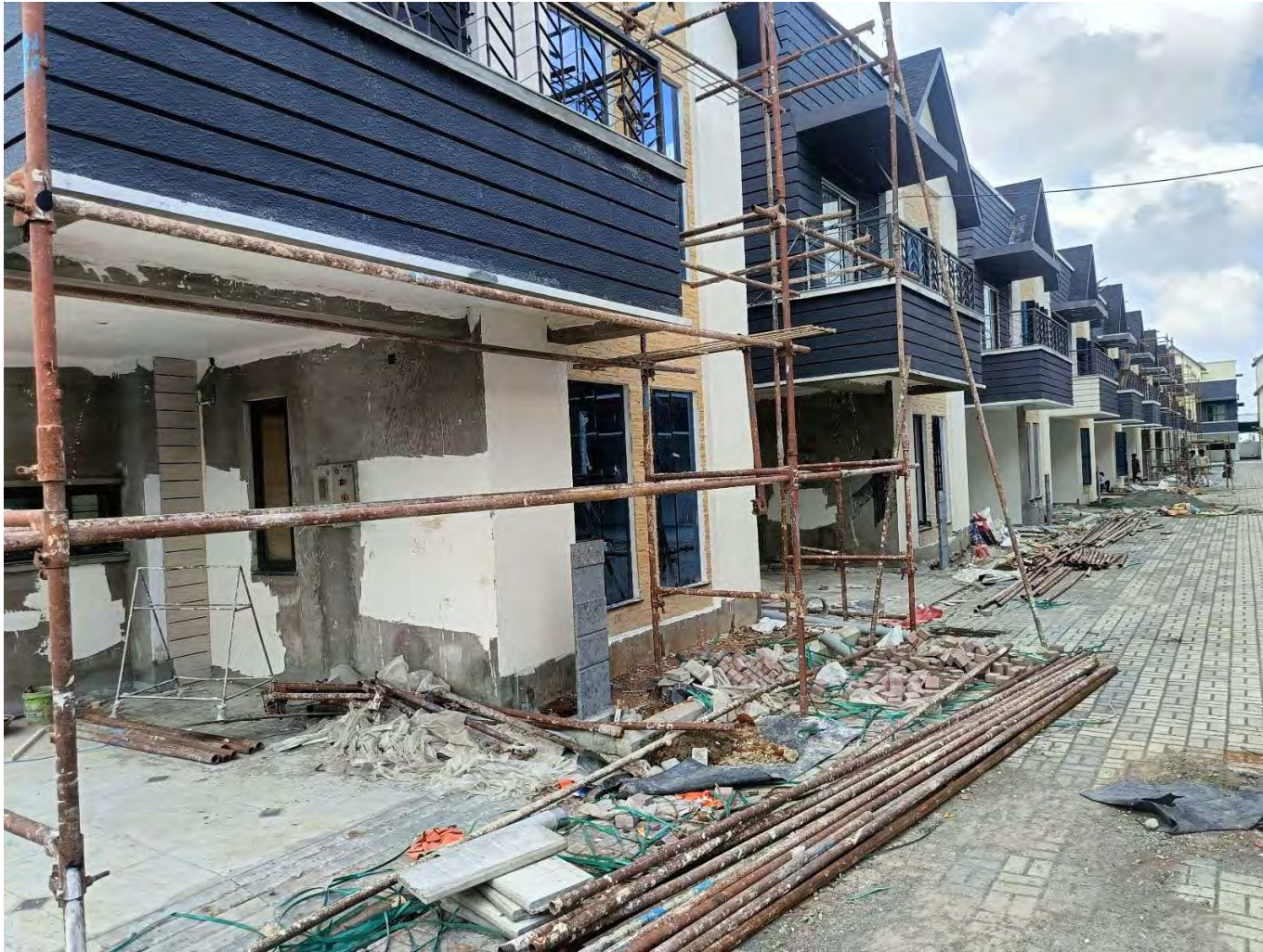
Painting work in progress
