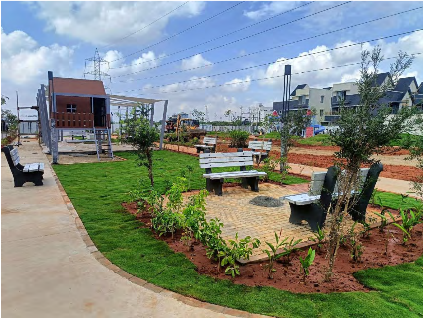
Landscape work in progress
