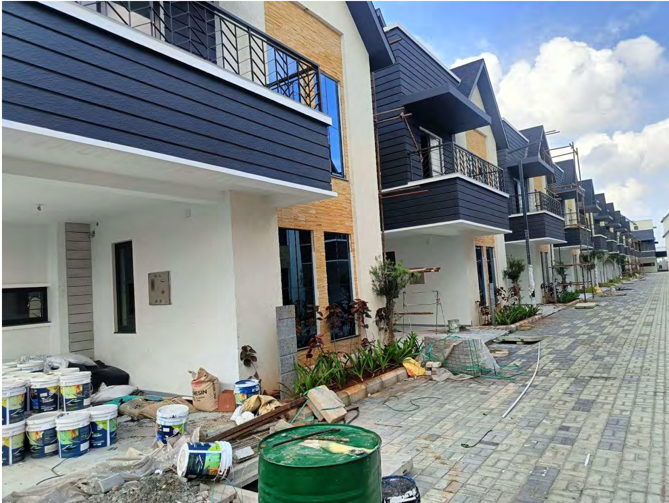
Painting work in progress
