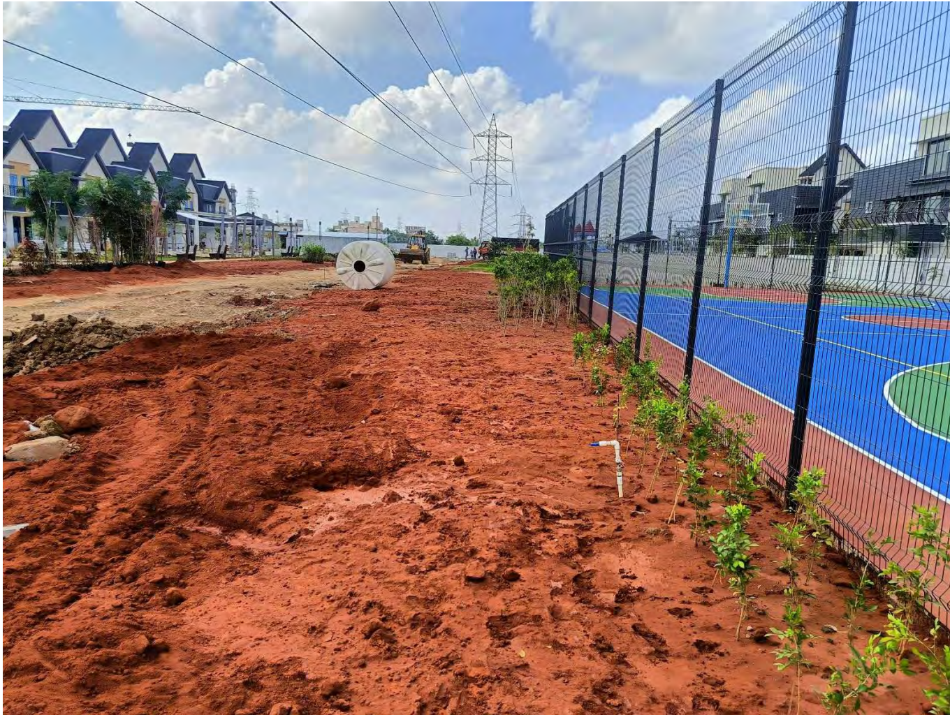
Landscape work in progress
