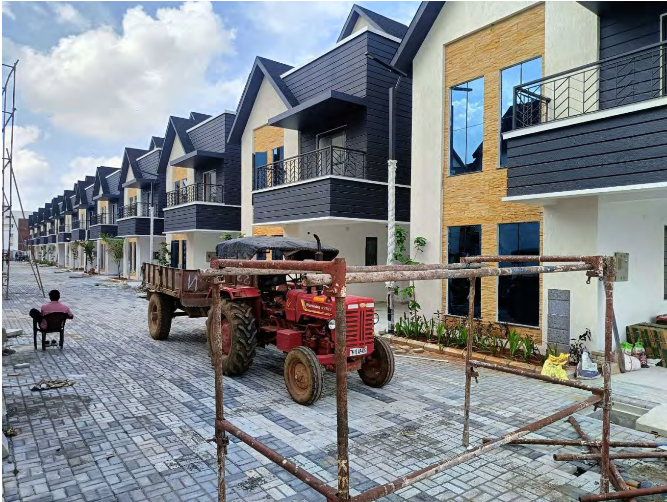
Snag work in progress
