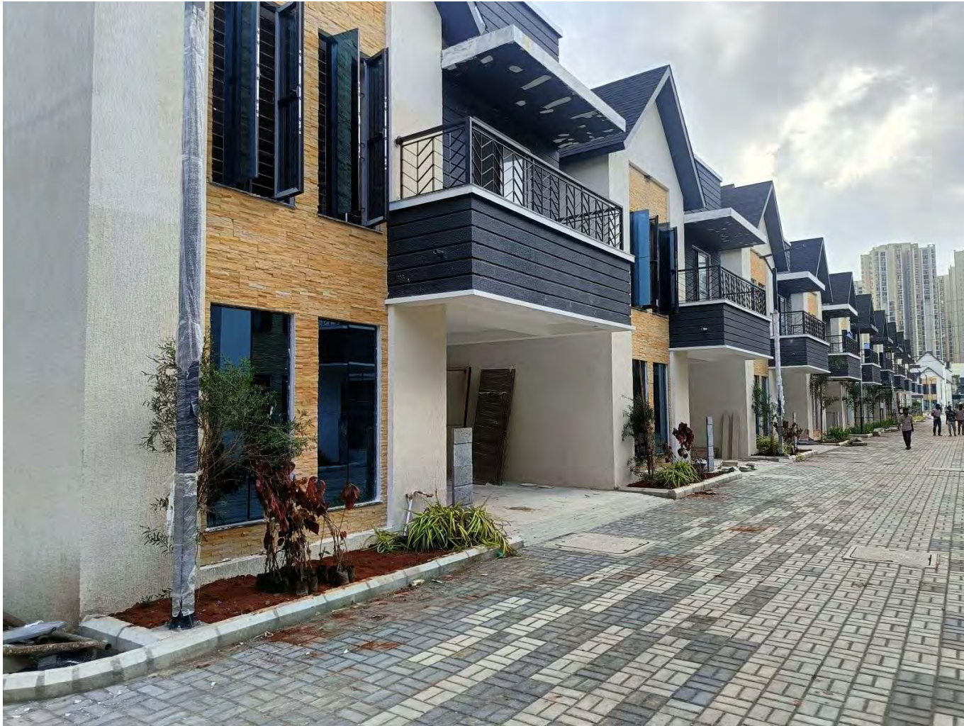
Painting work in progress
