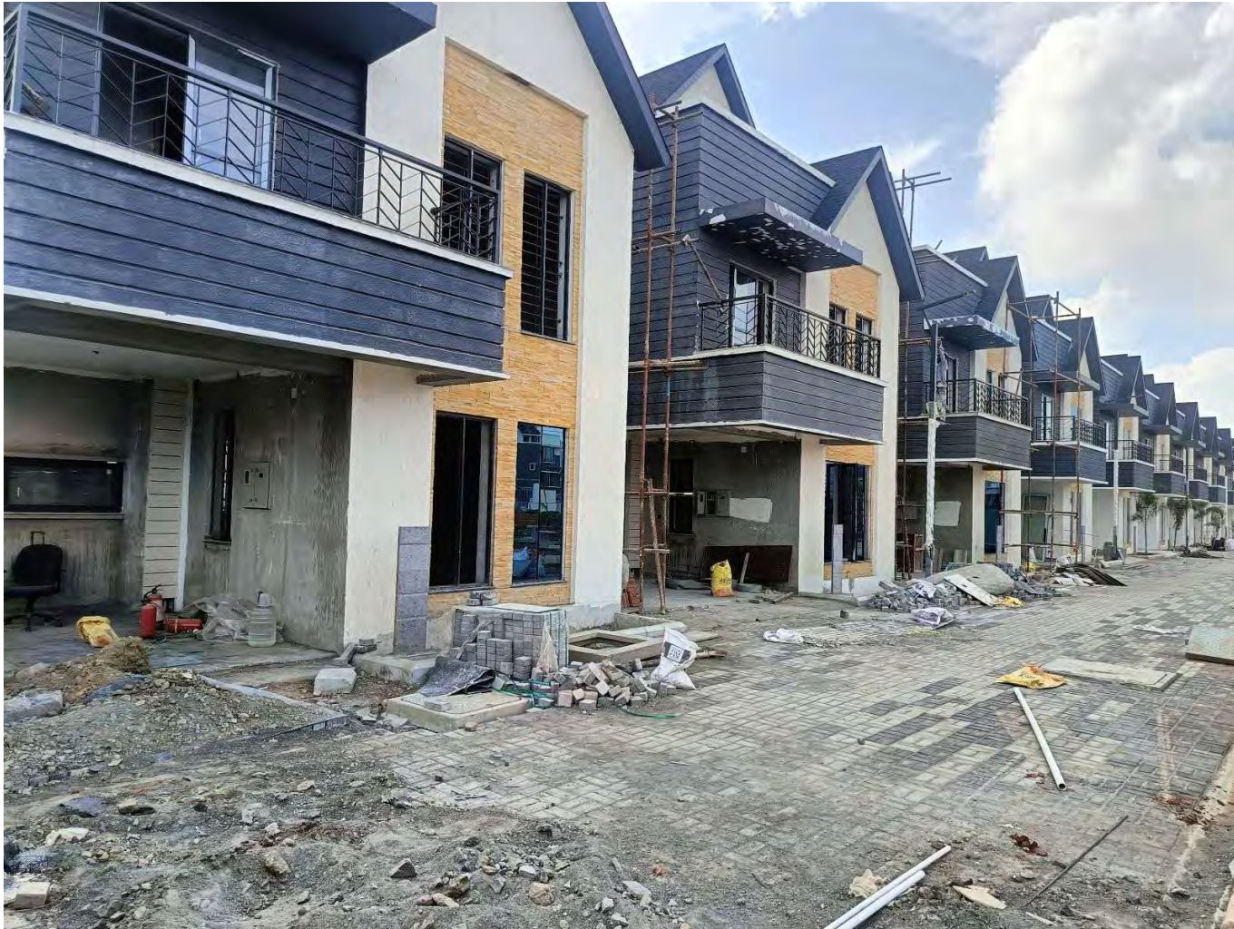
Snag work in progress
