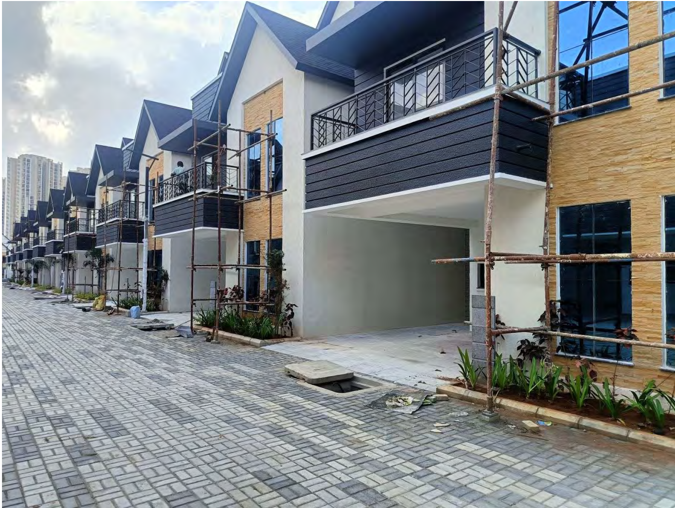
Painting work in progress
