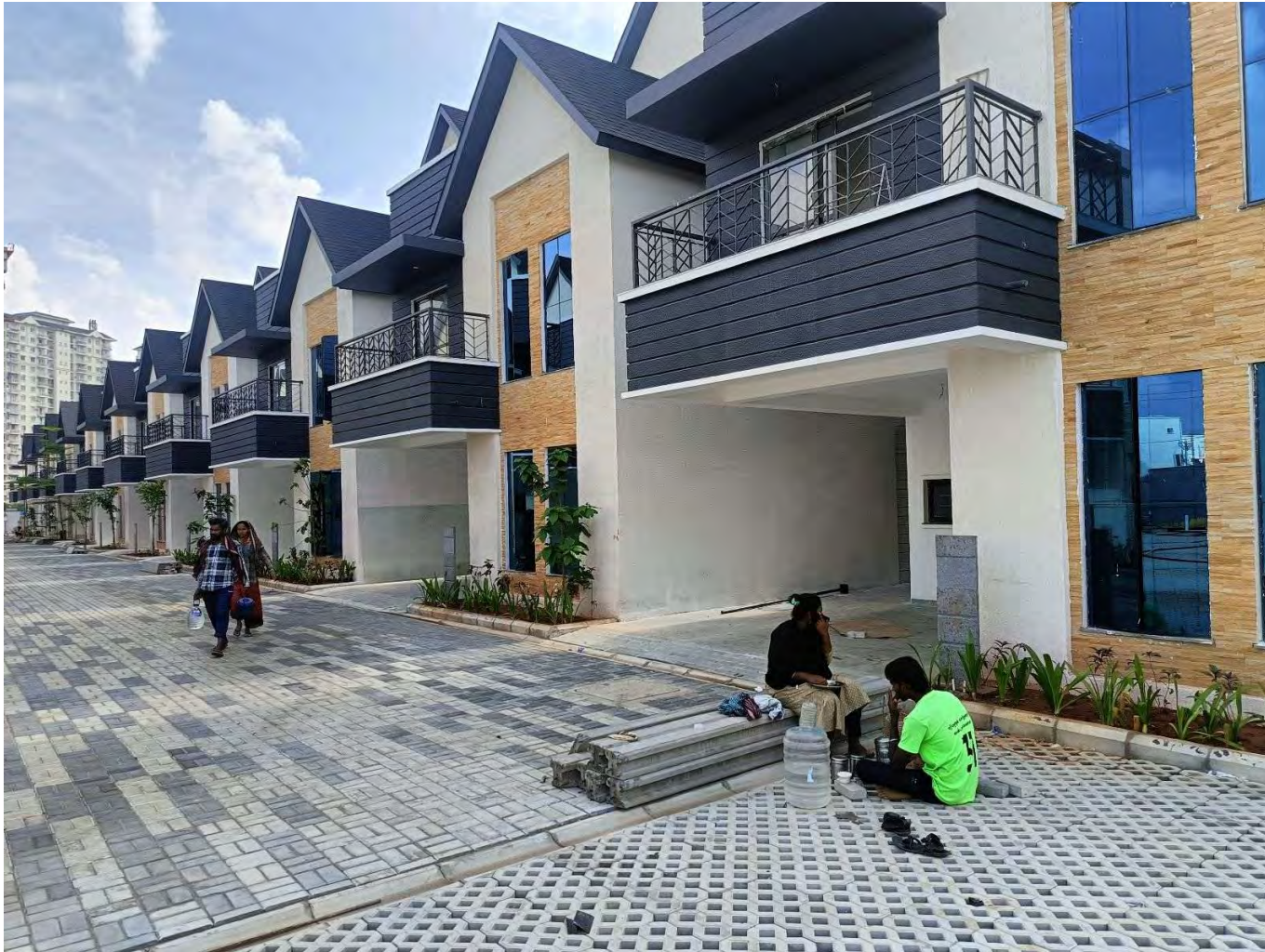
Snag work in progress
