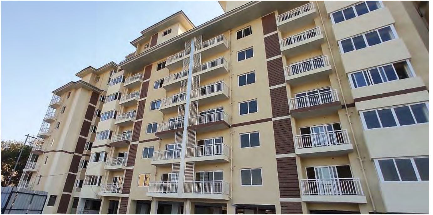
Tower C8 – Pic 2
