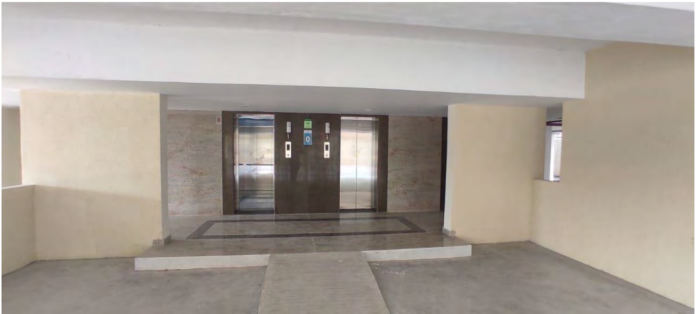
External Infra – Pic 5
