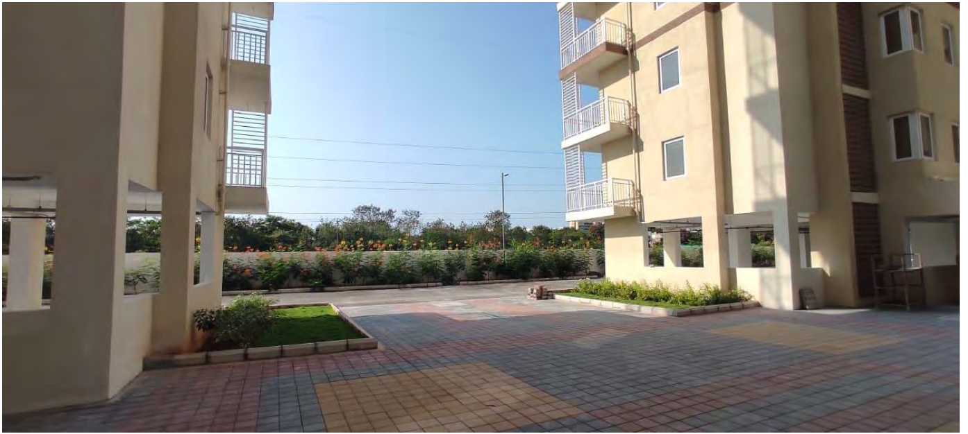
External Infra – Pic 4
