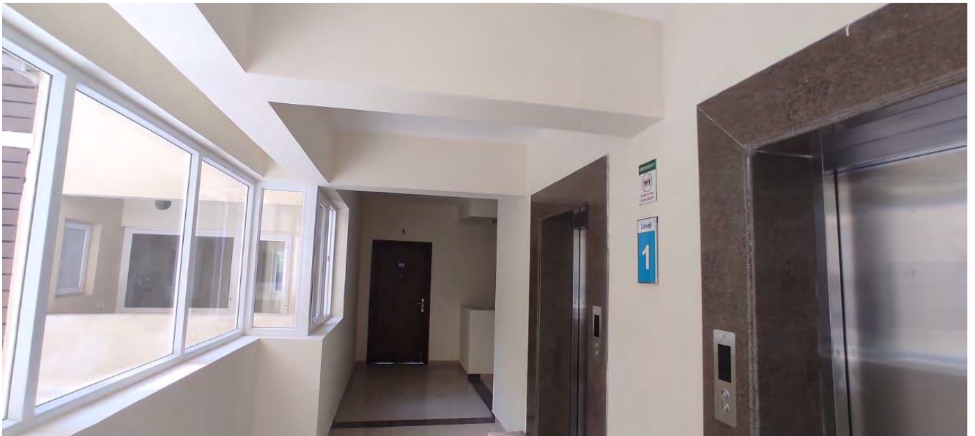
Tower C7– Pic 3
