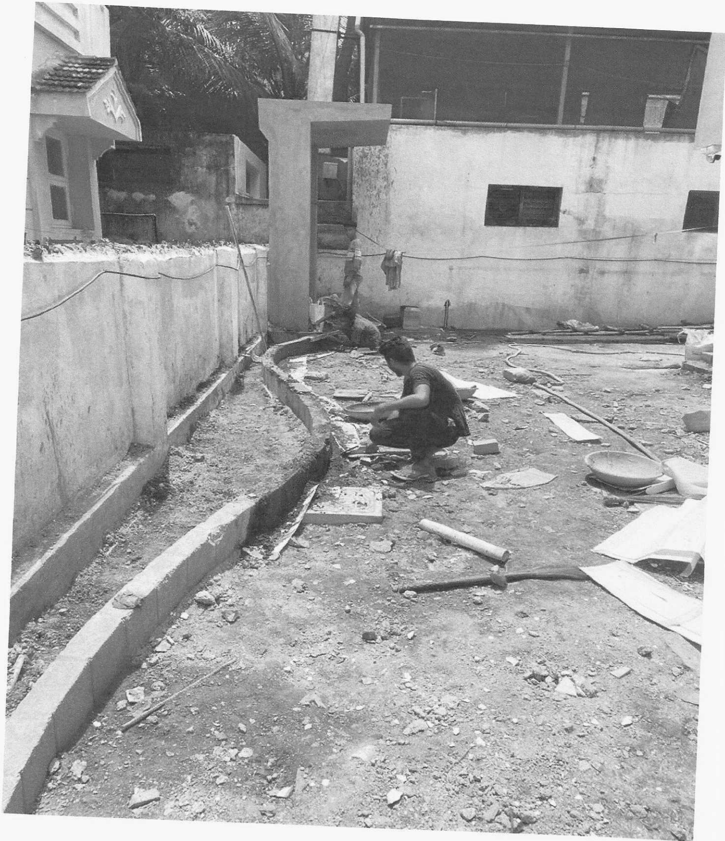
BLOCK 01 – SET BACK AREA EARTH LEVELING WORK
