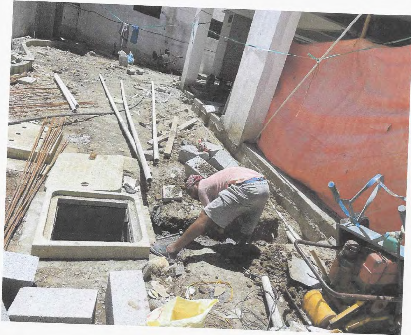
EXTERNAL PLUMBING CHAMBER WORK
