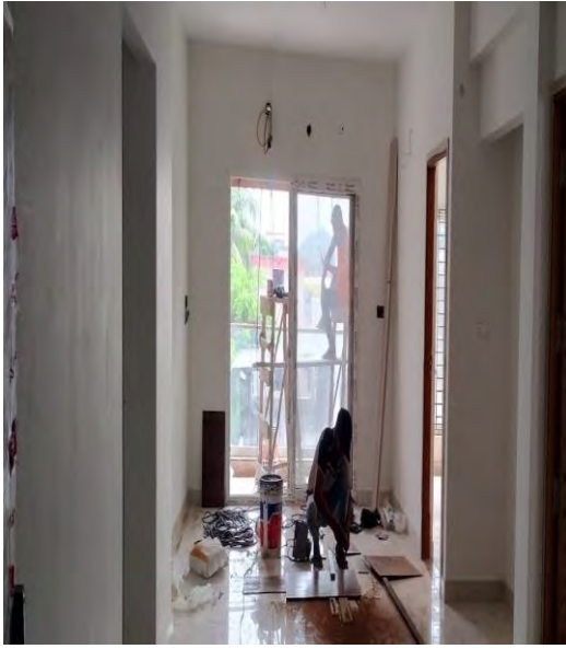
Internal wiring testing work is in progress
