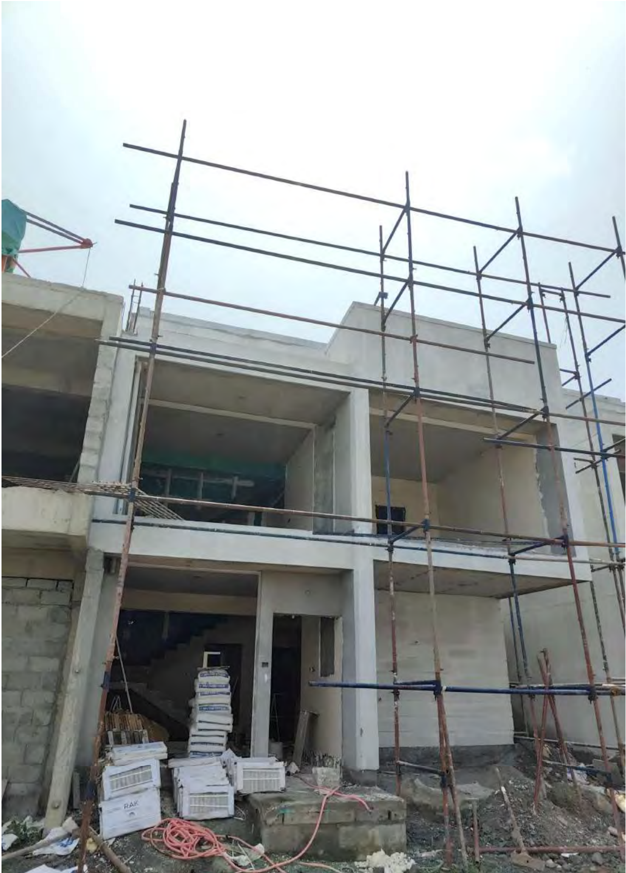
RERA REGISTRATION NO: TN-01-BUILDING-486-22 VILLA – 29 PAINTING WORK IN PROGRESS
