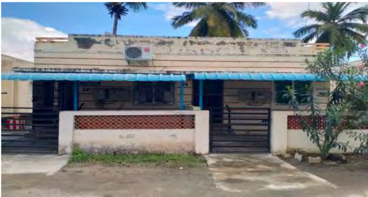
TWIN HOUSES T1 T2 AND T3 ALL 40 NOS COMPLETED & HANDED OVER
