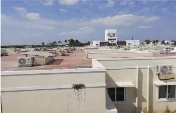
TERRACE OF ROW HOUSES
