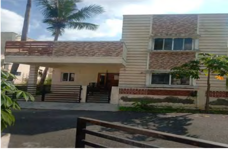
VILLAS V2-1 TO V2-7 COMPLETED & HANDED OVER
