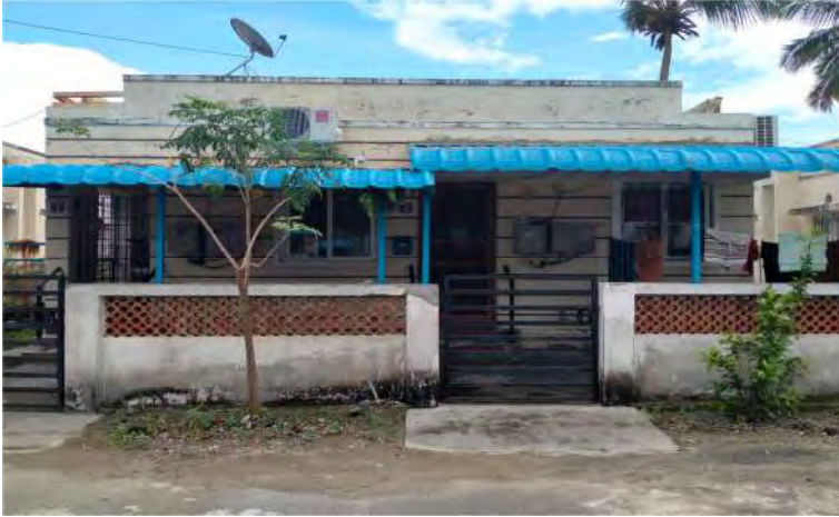
TWIN HOUSES T1 T2 AND T3 ALL 40 NOS COMPLETED & HANDED OVER
