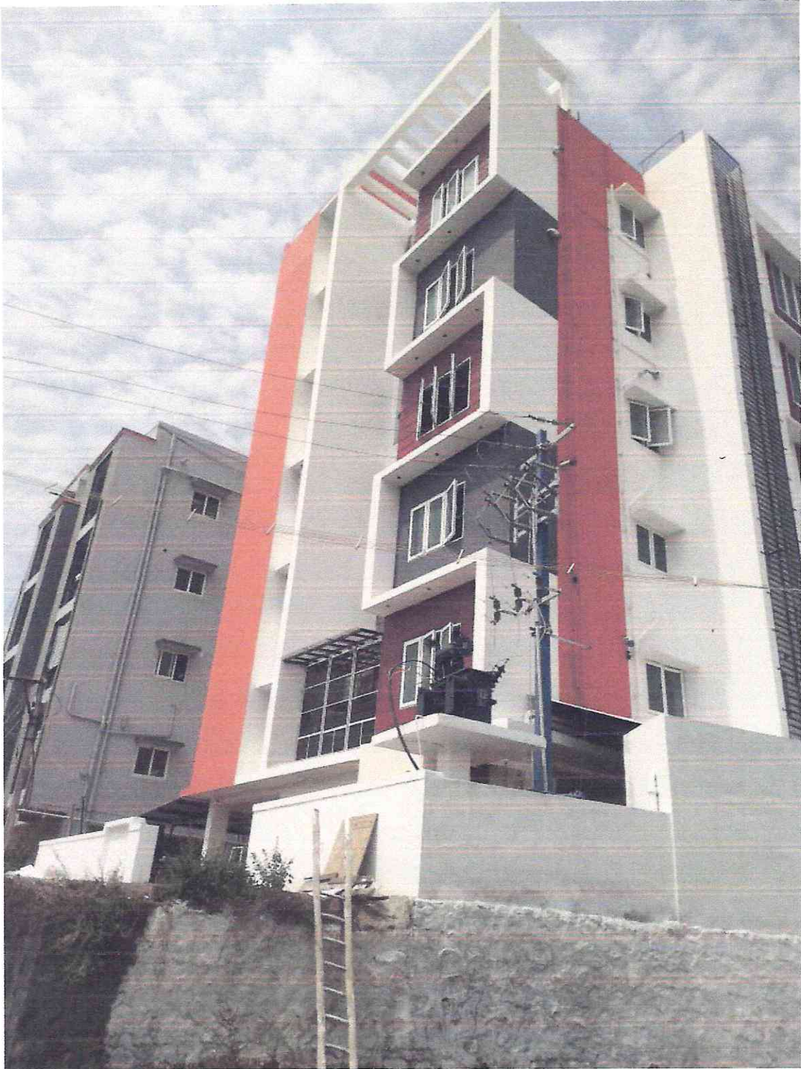
South east corner
