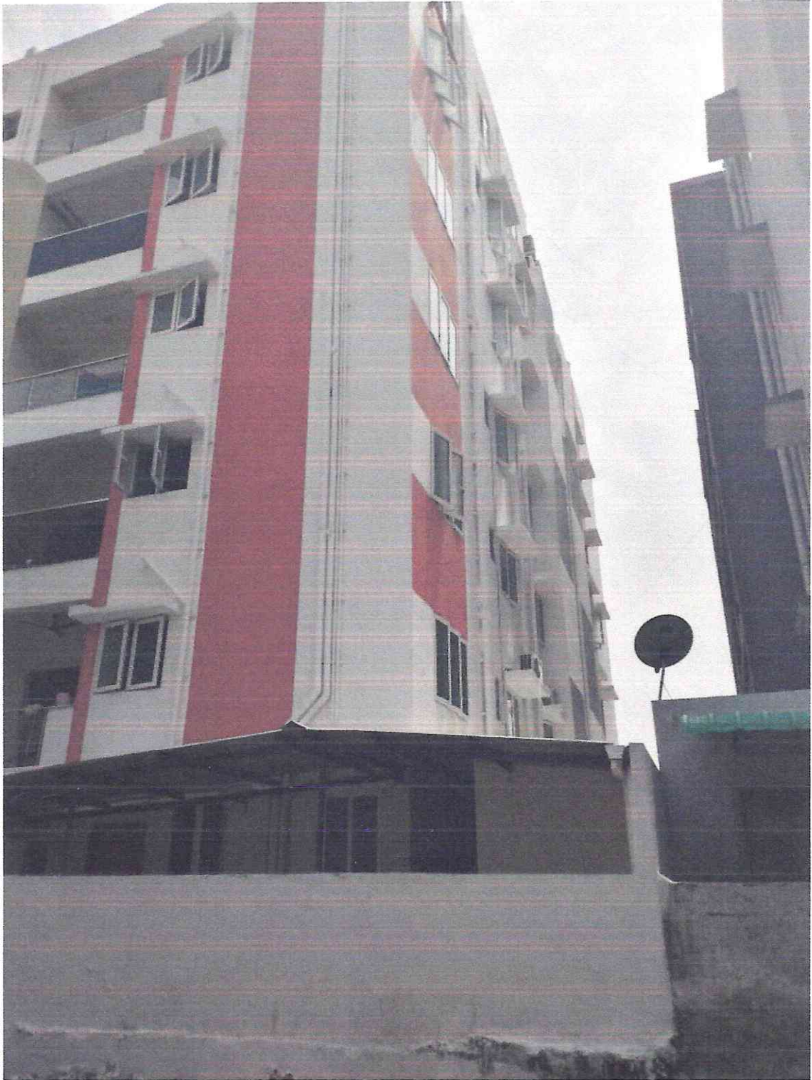
North side ( Back Of building)
